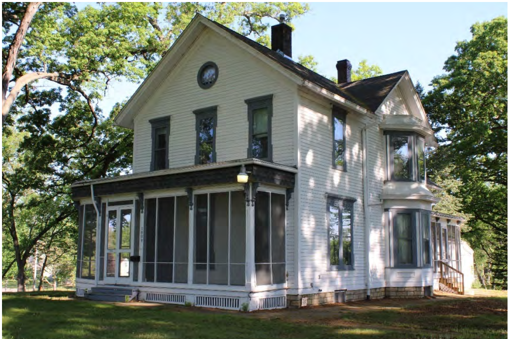
Figure 17. Exterior, façade (north) and east side elevation, facing northwest
