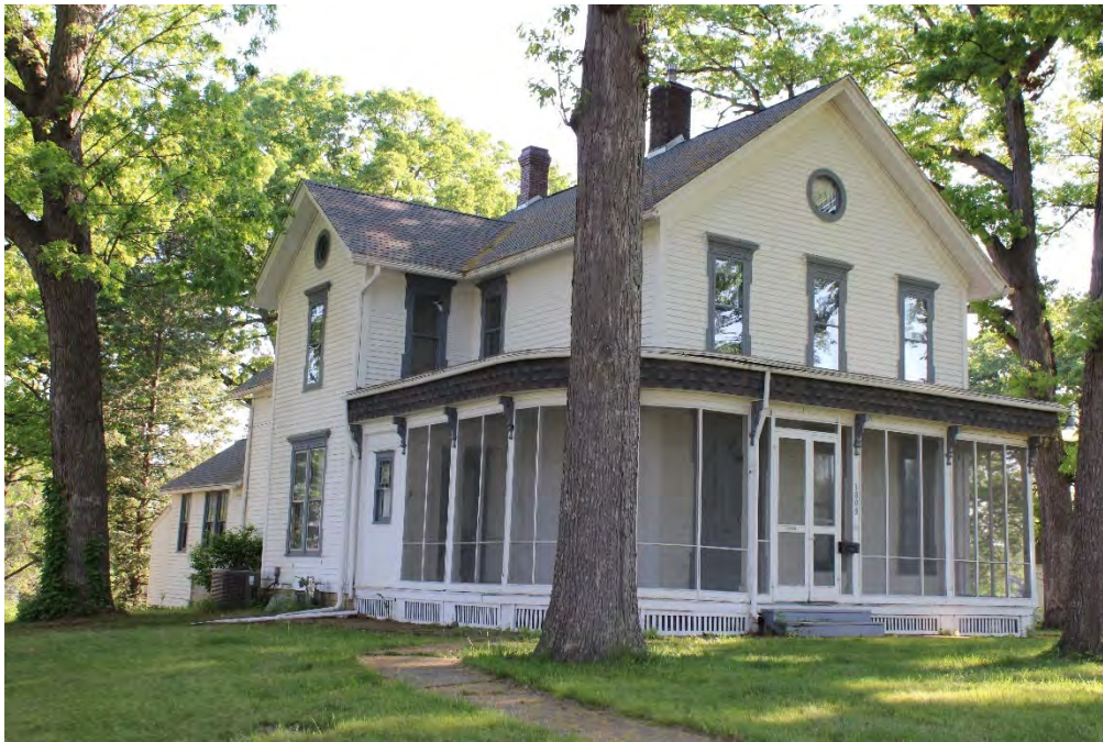
Figure 10. Exterior, façade (south) and west side elevation, facing northeast
