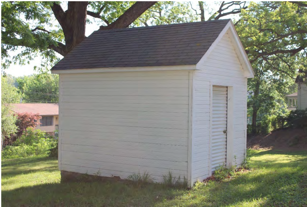
Figure 40. Northeast shed, facing northeast, standing northeast of house
