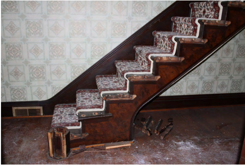
Figure 25. Interior, main stair hall, first floor; Habitat for Humanity removed main post and banister railing, other trim
