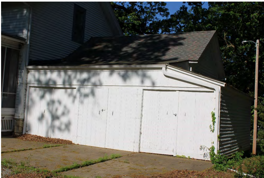
Figure 14. Exterior, east side and rear (north) elevations, one-story garage ell, facing southwest
