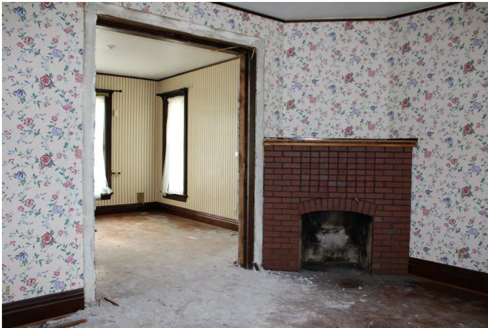
Figure 34. Interior, living room, Habitat for Humanity removed fireplace mantel and framing elements
