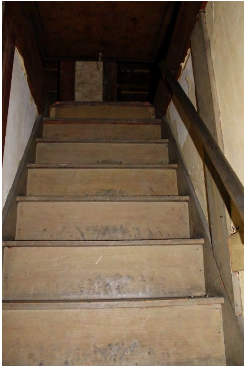
Figure 27. Interior, attic access, accessed in southeast bedroom on second floor
