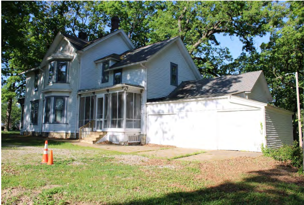
Figure 13. Exterior, east side and rear (north) elevations, one-and-a-half-story ell and rear one-story garage ell, facing southwest
