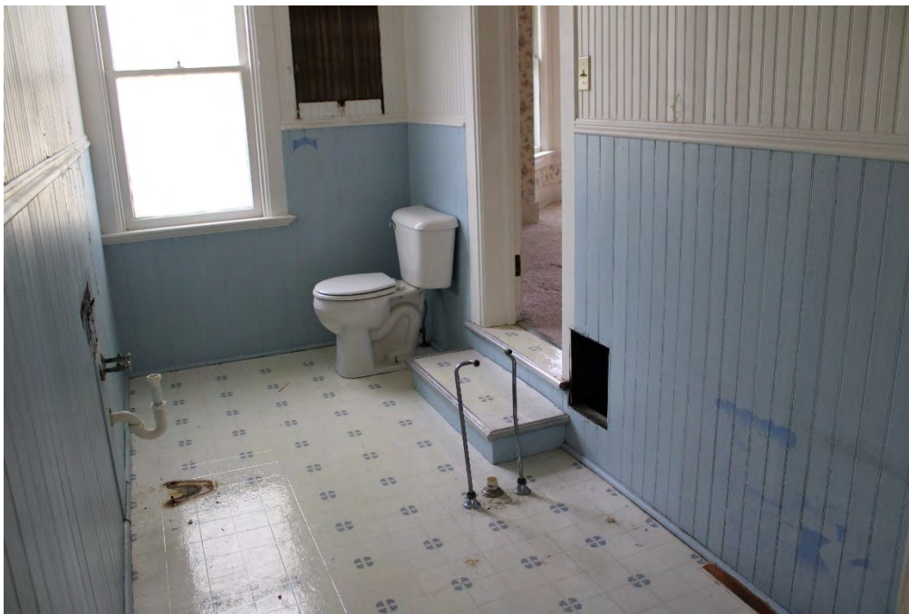
Figure 30. Interior, bathroom, second floor, Habitat for Humanity removed bathtub, sink, any floor cabinetry, floating wall shelf/mirror, other trim
