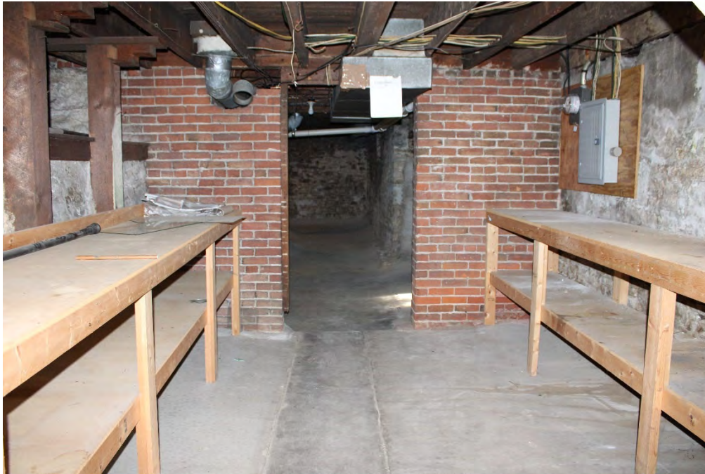
Figure 23. Interior, basement, brick wall spans and coated stone foundation walls, facing north from stairwell
