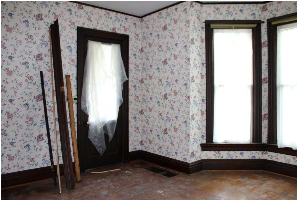
Figure 28. Interior, main living room, examples of wood trim elements removed by Habitat for Humanity. The north-facing wood-and-glass door shown provides access to the east side elevation porch from the main living room
