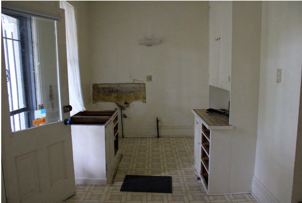
Figure 29. Interior, kitchen, Habitat for Humanity removed appliances, cabinetry, sink, countertops, drawers, other trim
