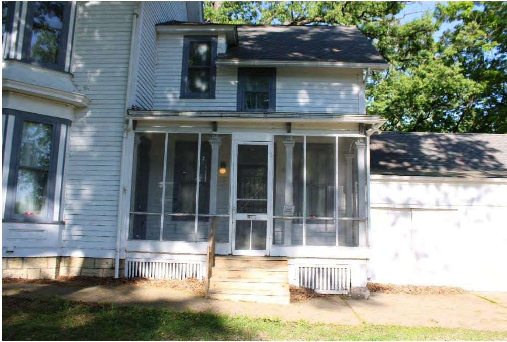
Figure 15. Exterior, east elevation side porch, facing west
