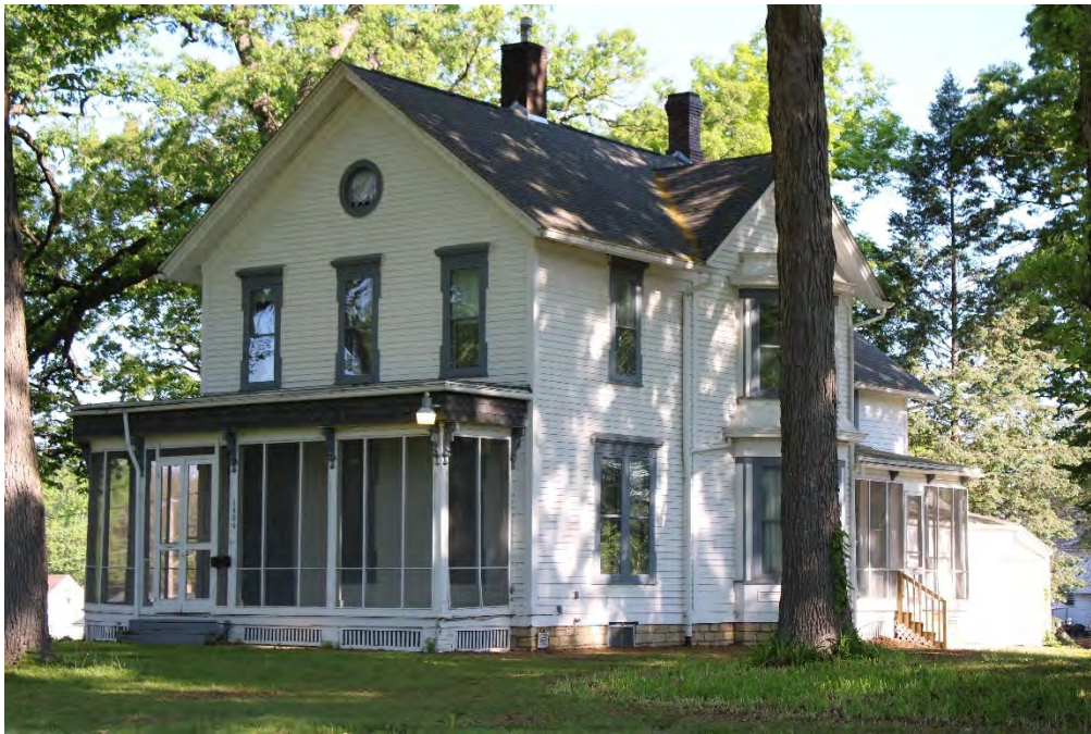
Figure 8. Exterior, façade (south) and east side elevation, facing northwest
