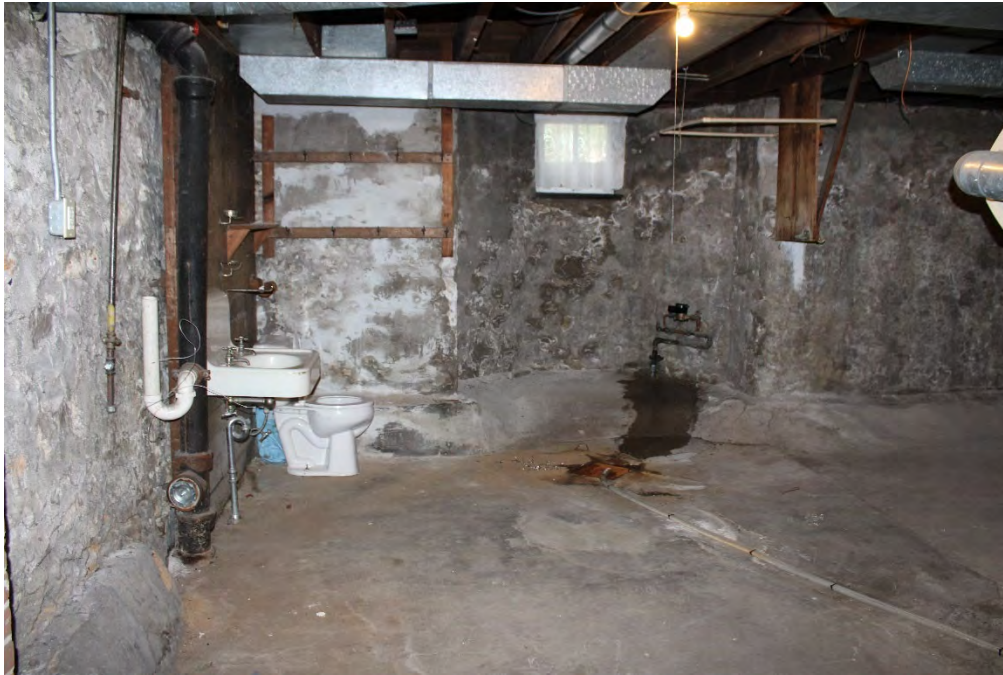
Figure 33. Interior, basement, modern bathroom elements with no walls added
