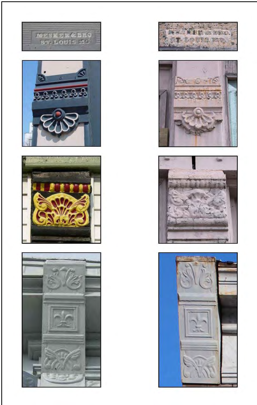
Figure 9: Illustrated in these images are Mesker Brothers ornamentation examples as illustrated in a “got mesker” publication on the left, and the comparable images found in February 2022 on the 14-16 S. Main Street building in Pinckneyville (“got mesker? Identification Guide to Sheet-Metal Facades and Building Components Manufactured by Mesker Brothers Iron Works & George L. Mesker & Company,” Viewed at https://www2.illinois.gov/dnrhistoric/Preserve/Documents/Mesker_identification_guide.pdf in June 2022).
