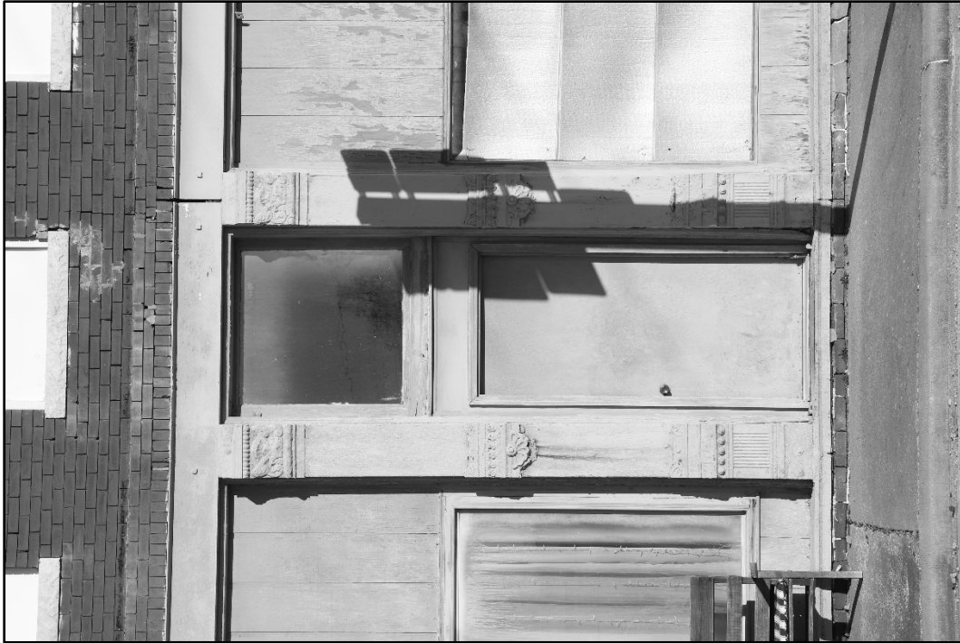
Photo #11 of 30 (turn 90° to the right for viewing)
