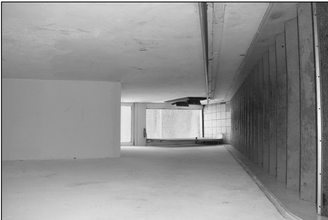
Photo #22 of 30 (turn 90° to the right for viewing)
