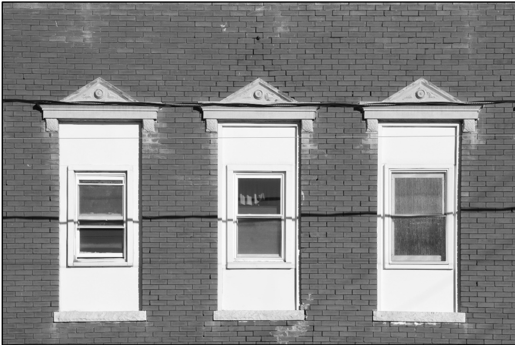
Photo #14 of 30 (turn 90° to the right for viewing)
