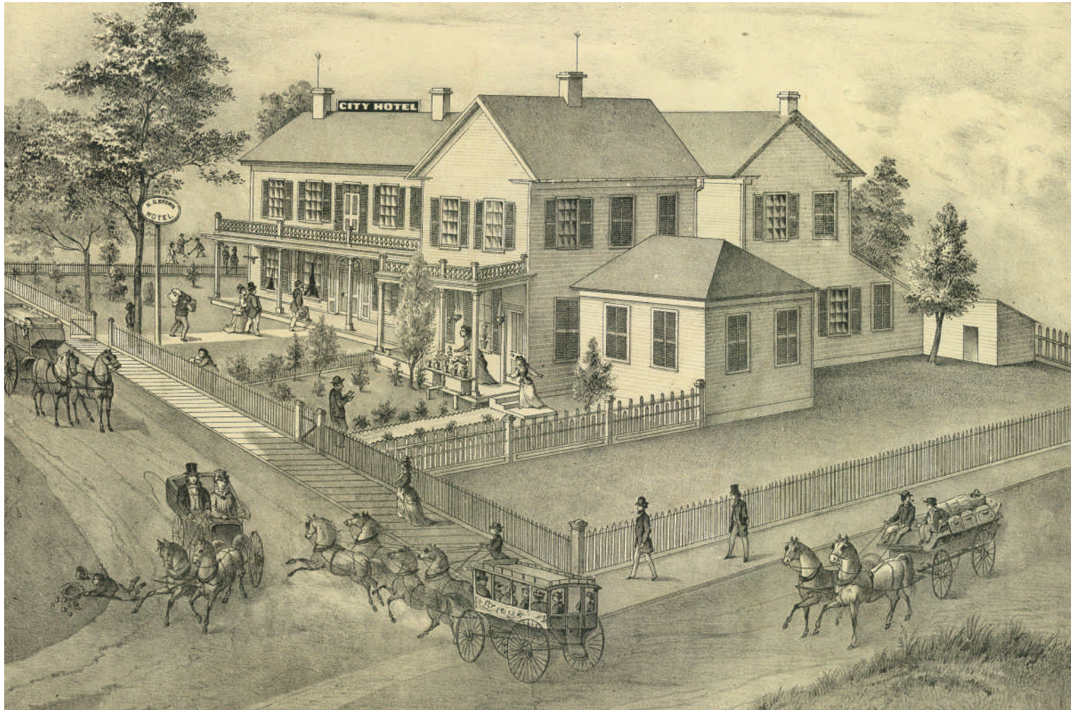
Residence and hotel constructed in Hillsboro, in neighboring Montgomery County, for James Hagee, as depicted in 1874. This is an excellent example of the “house-hotel” building type common during the nineteenth century. This single building resembled a house but incorporated functions of family dwelling, guest accommodations, and possibly a tavern under one roof. The sprawling character of the hotel suggests that it was built in several episodes.
