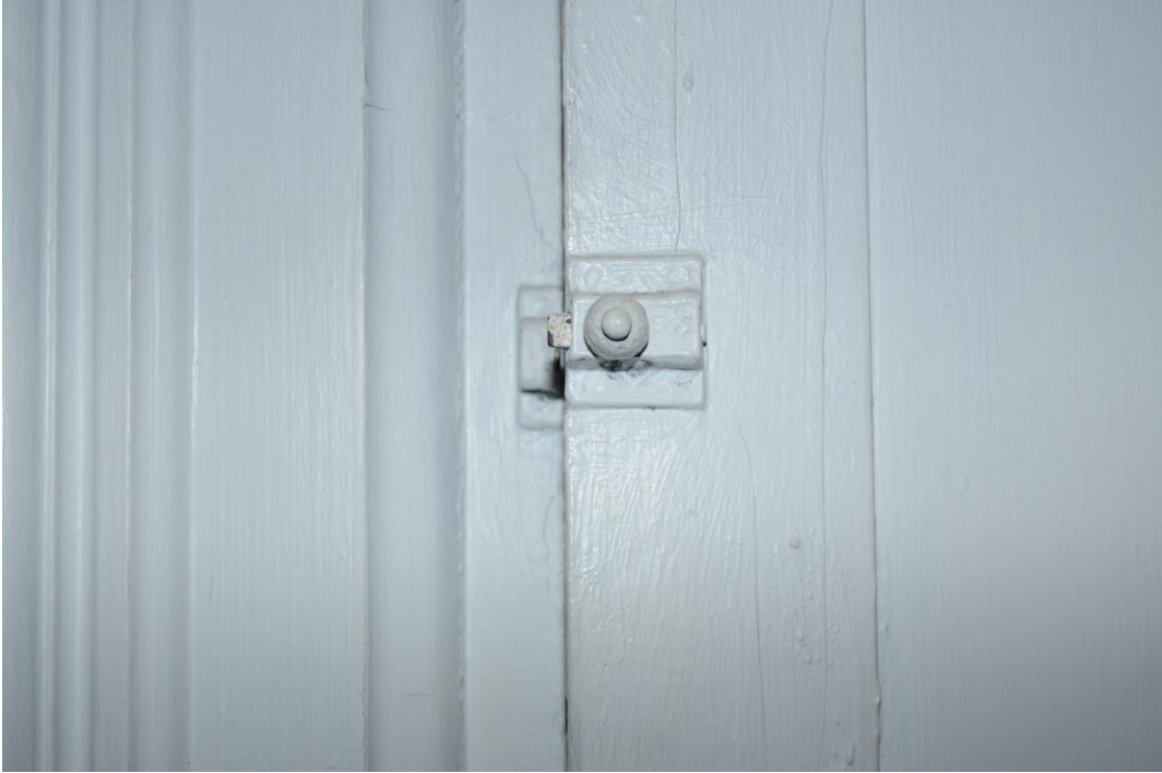
Illinois HABS No. L-2015-01-19. Detail of bedroom cabinet latch (111).
