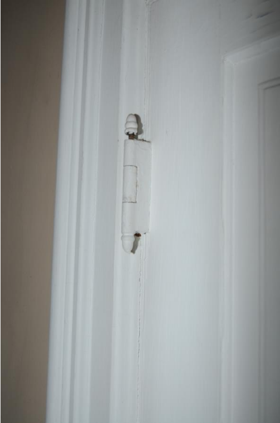
Illinois HABS No. L-2015-01-23. Detail of door pintel (157).
