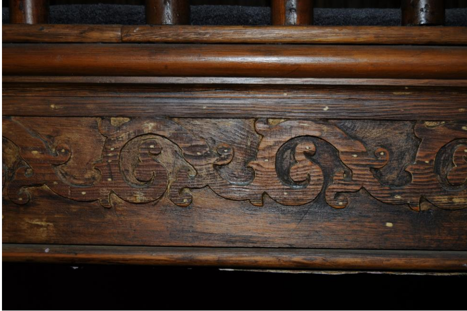
Illinois HABS No. L-2015-01-14. Detail of the skirting on the fascia (102).
