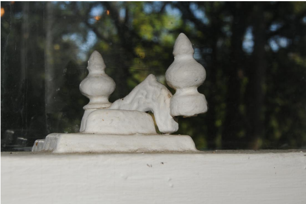
Illinois HABS No. L-2015-01-22. Detail of original window latch (148).
