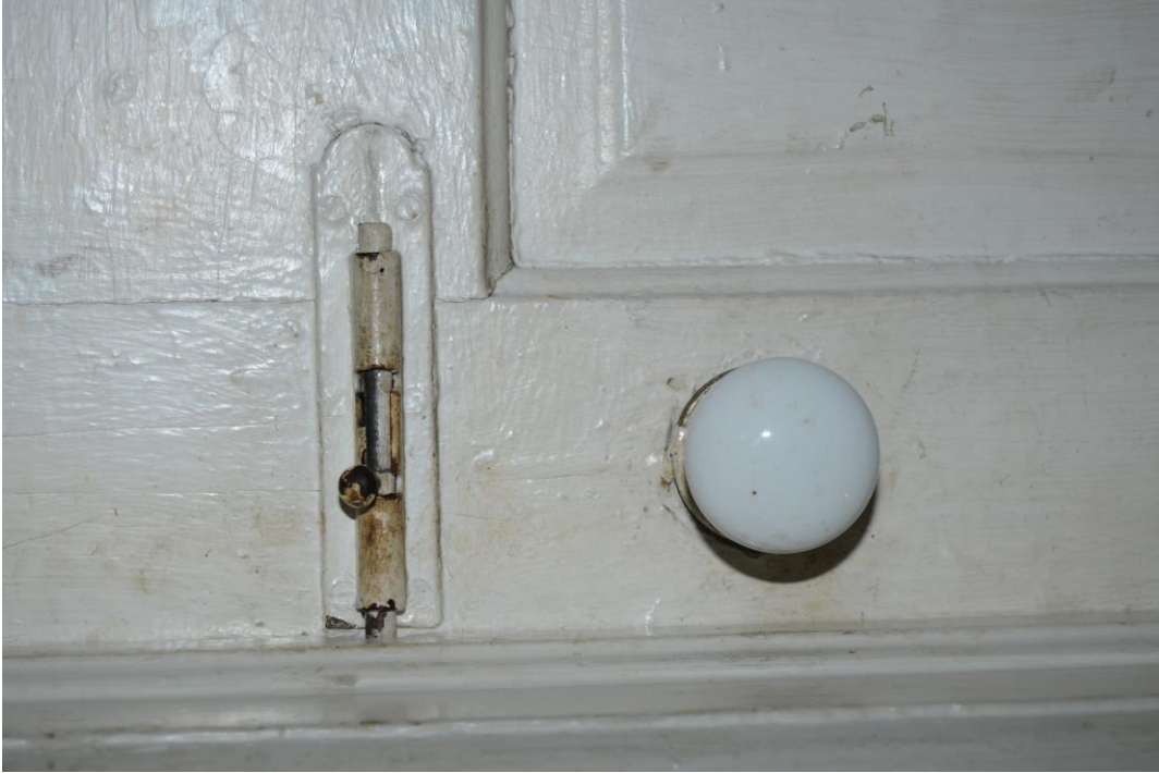
Illinois HABS No. L-2015-01-21. Detail of basement door hardware (130).
