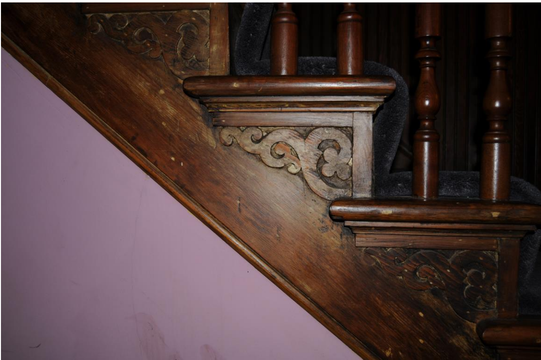
Illinois HABS No. L-2015-01-13. Detail of skirting brackets (95).
