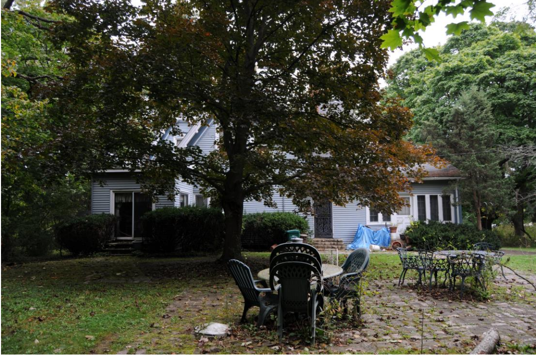
Illinois HABS No. L-2015-01-5. Rear façade (west) of the residence illustrating the relationship between the patio and the residence, and showing the two gable ends partially obscured by the tree foliage (65).
