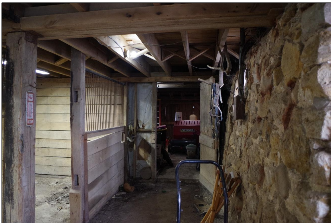
Photograph 23: Interior view of barn, lower level, looking east.
