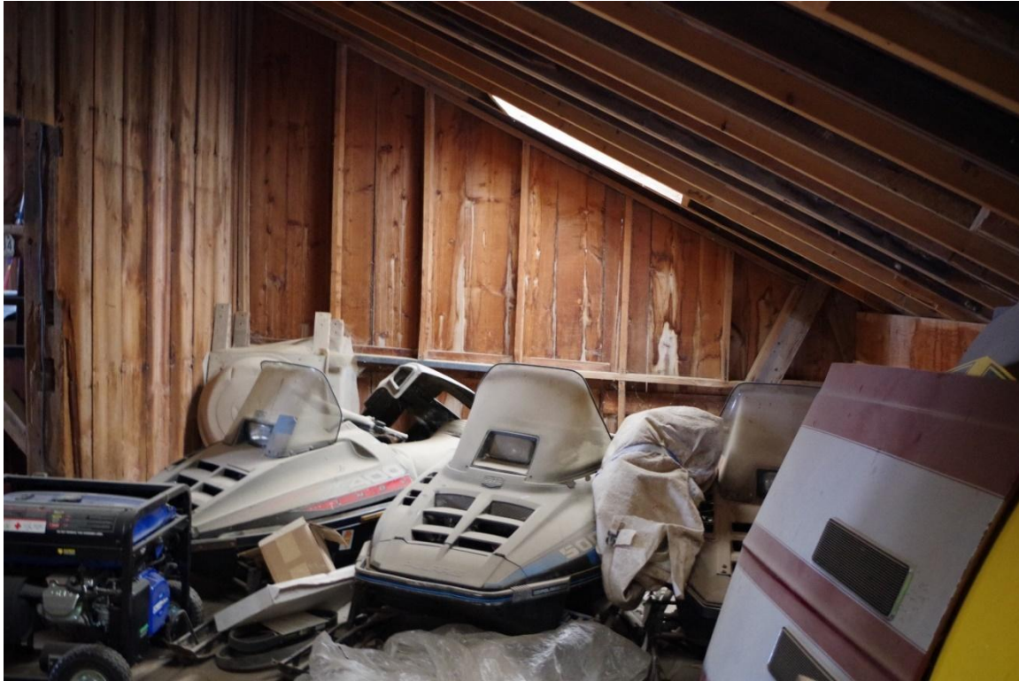
Photograph 35: View of the barn interior, second level, east addition, camera facing northeast.
