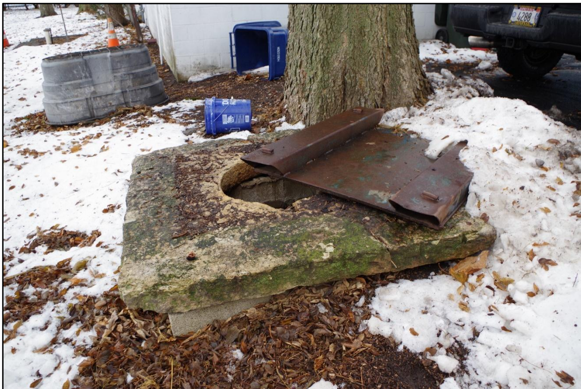
Photograph 12: View of the ca. 1860 cistern, camera facing south. December 2025.
