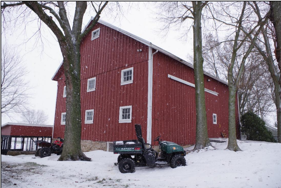
Photograph 22: View of the barn, camera facing southeast. December 2025.
