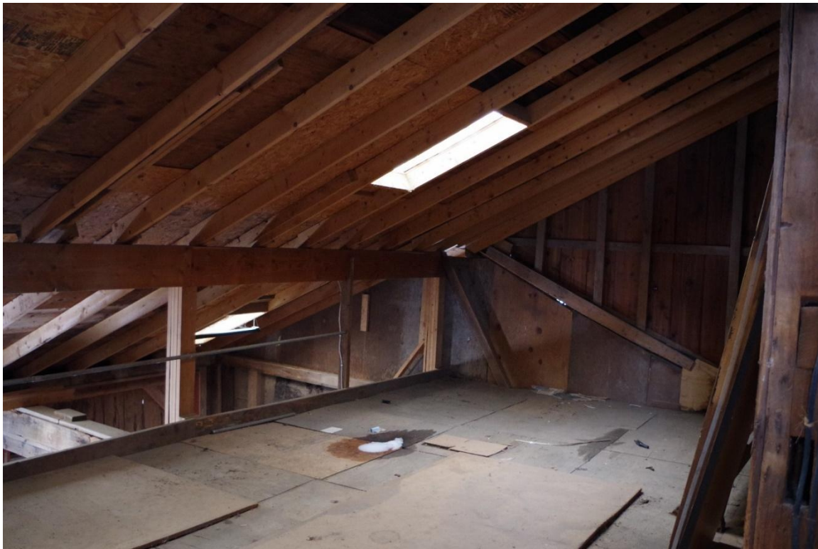
Photograph 36: View of the barn interior, second level, east addition, camera facing southeast.
