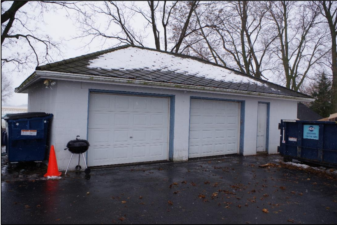
Photograph 45: View of the garage, view looking southeast.
