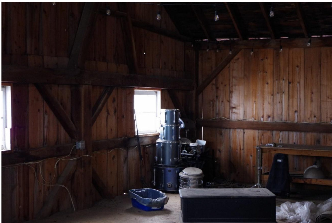
Photograph 42: View of barn interior, third level, camera facing southwest.
