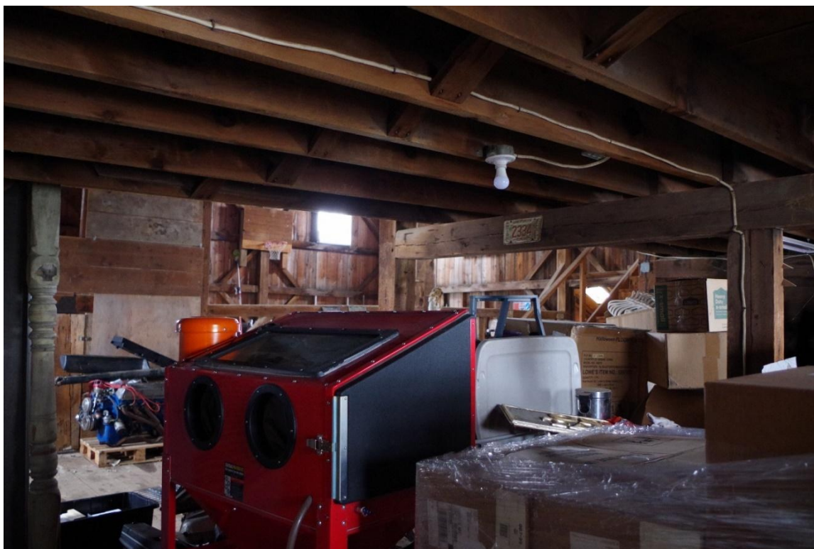
Photograph 32: View of barn interior, second level, camera facing northeast.
