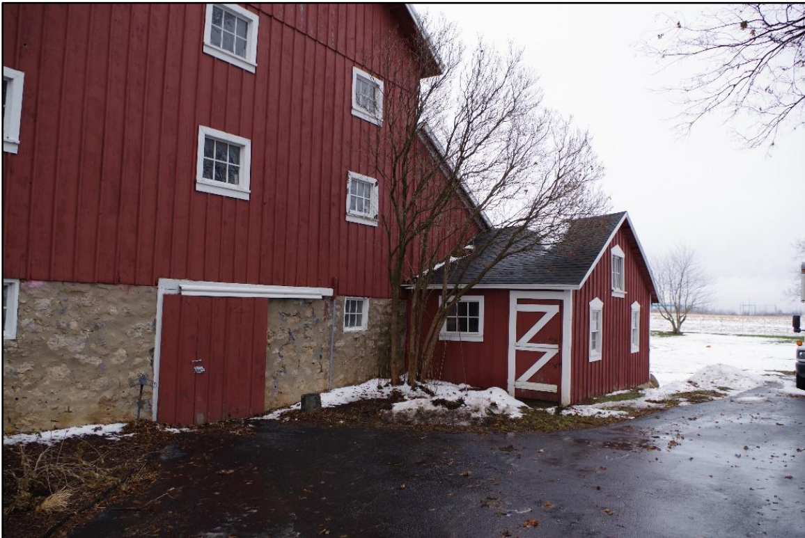
Photograph 16: View of the barn, camera facing northeast. December 2025.
