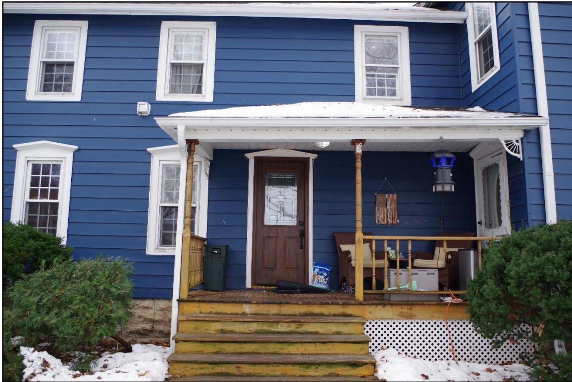
Photograph 11: View of the ca. 1860 dwelling, porch detail, camera facing south. December 2025.
