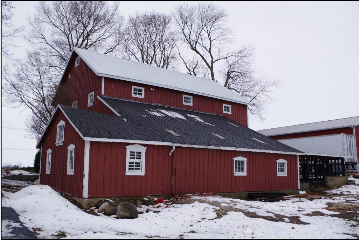
Photograph 19: View of the barn, camera facing west-northwest. December 2025.
