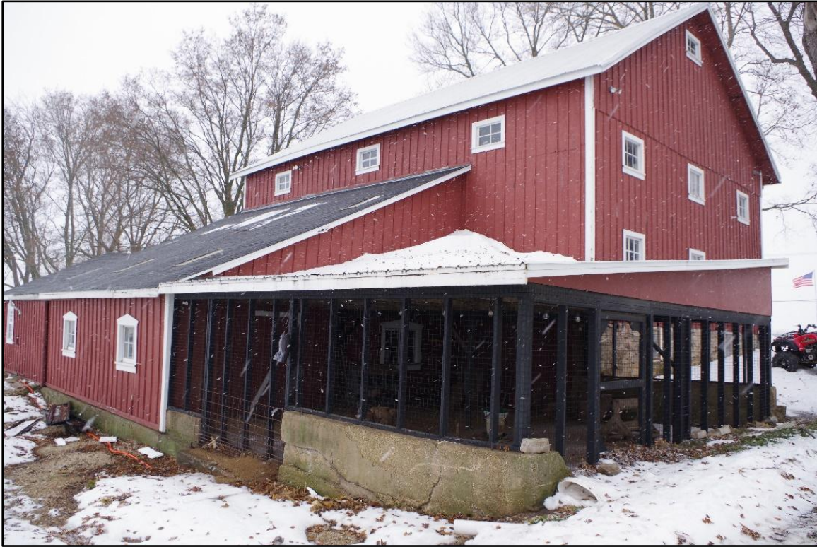
Photograph 21 View of the barn, camera facing southwest. December 2025.
