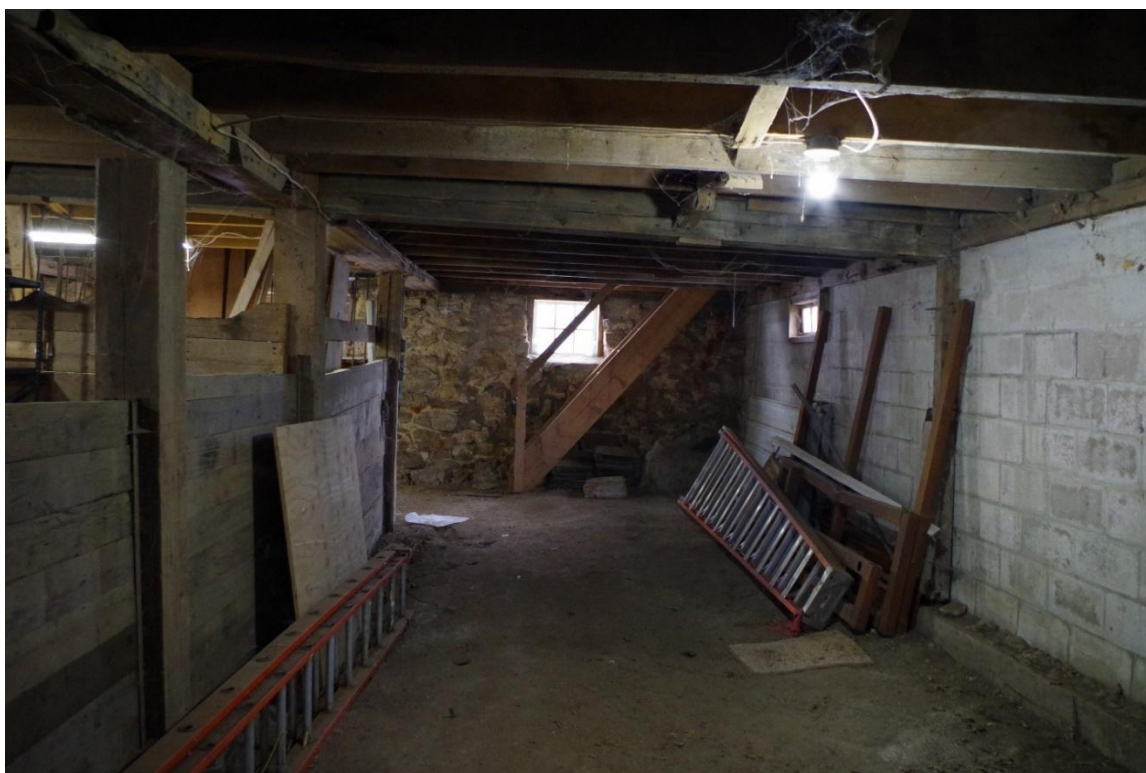
Photograph 29: View of barn interior, lower level, camera facing south.
