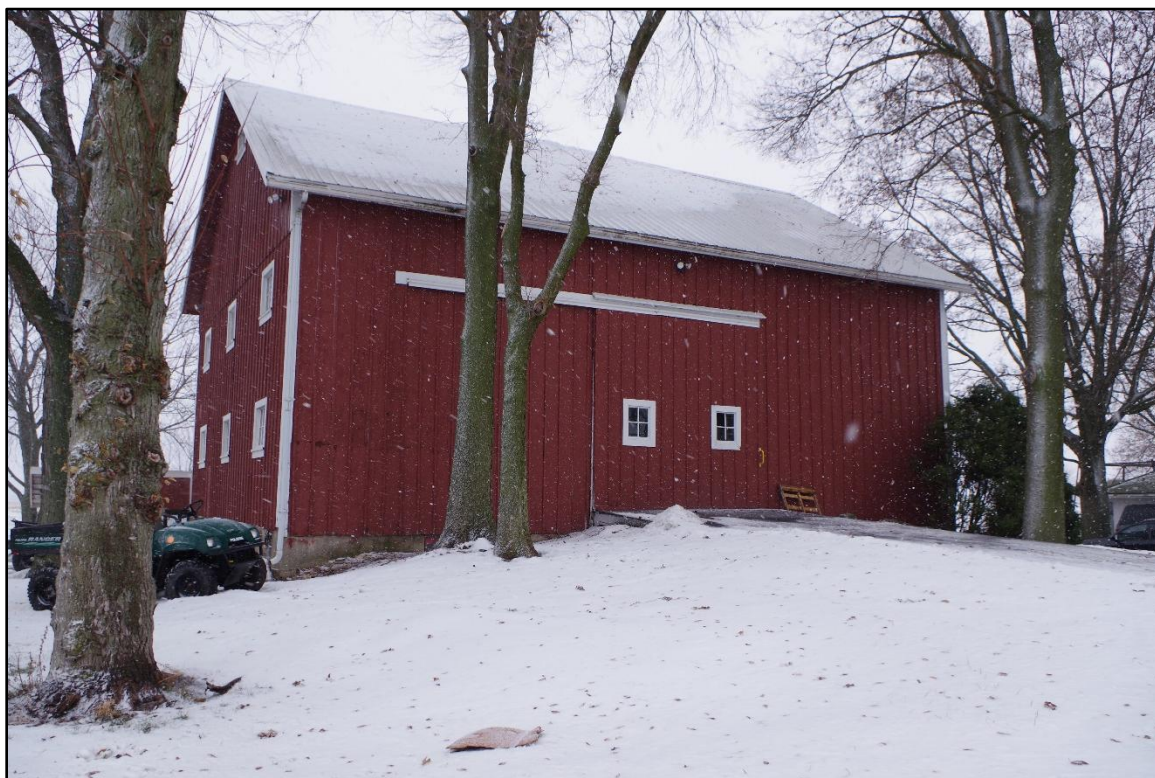
Photograph 14: View of the barn, camera facing northeast. December 2025.
