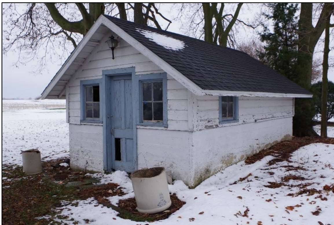
Photograph 52: View of the cold storage building, looking southeast.
