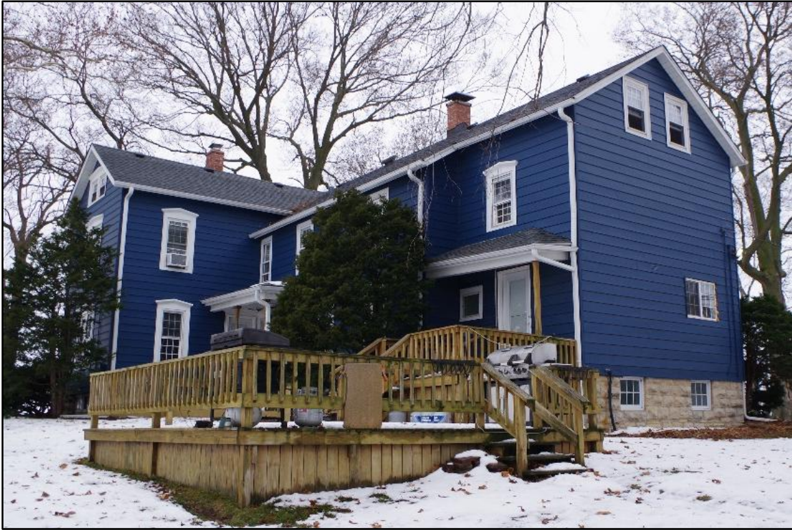
Photograph 9: View of the ca. 1860 dwelling, camera facing northwest. December 2025.
