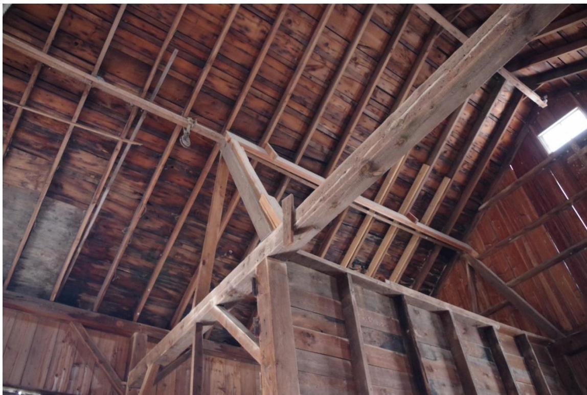
Photograph 39: View of barn interior, truss detail from second level, looking northwest.
