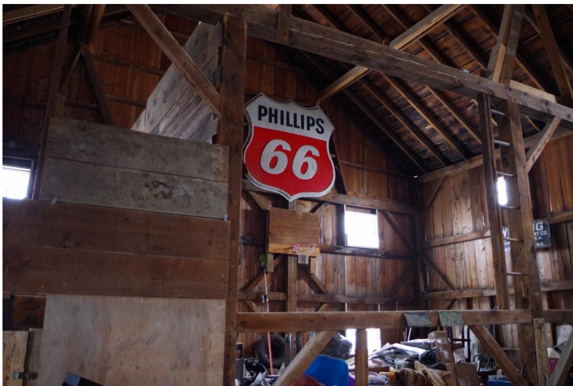
Photograph 30: View of barn interior, second level, camera facing northeast.
