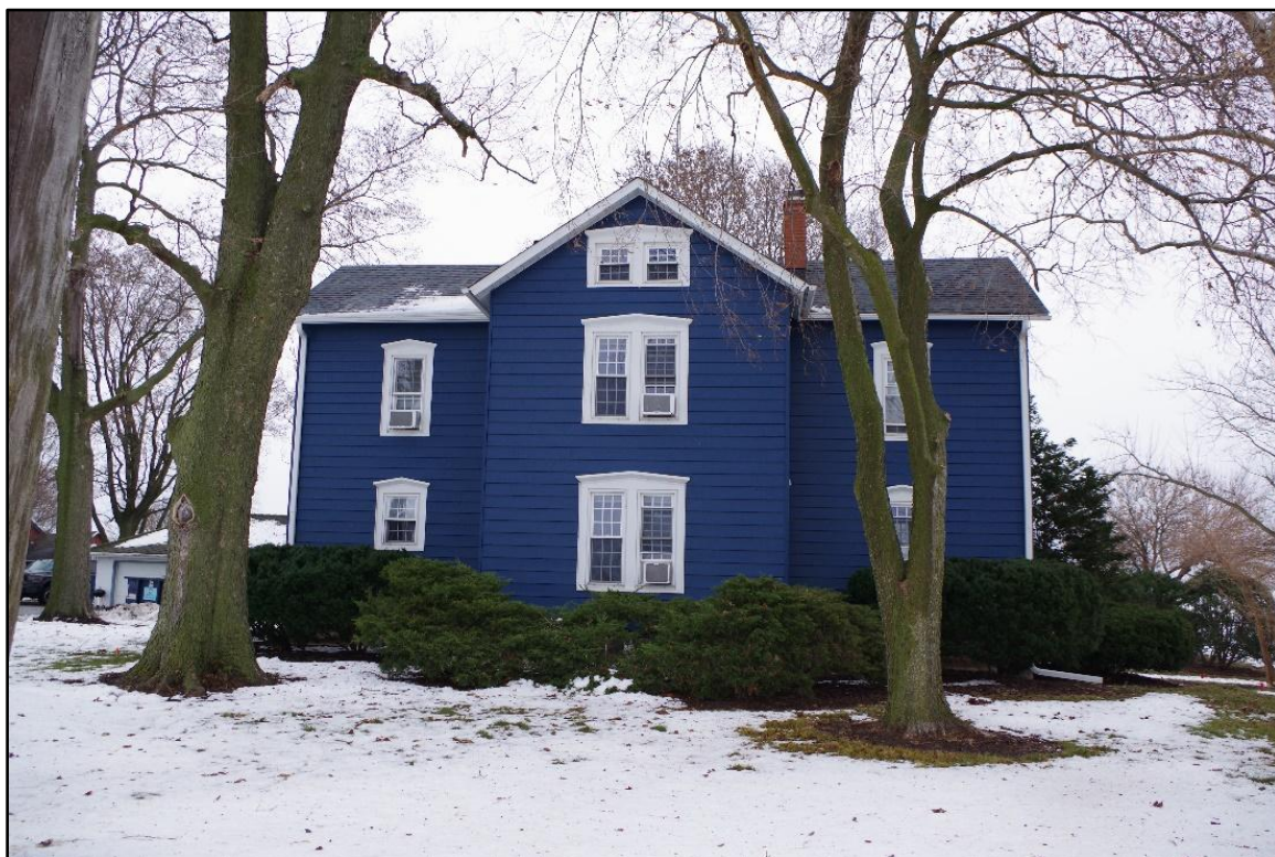
Photograph 6: View of the ca. 1860 dwelling, camera facing east. December 2025.
