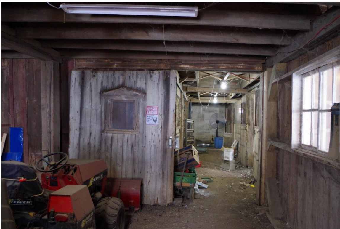
Photograph 27: View of barn interior, lower level, east addition, looking west.
