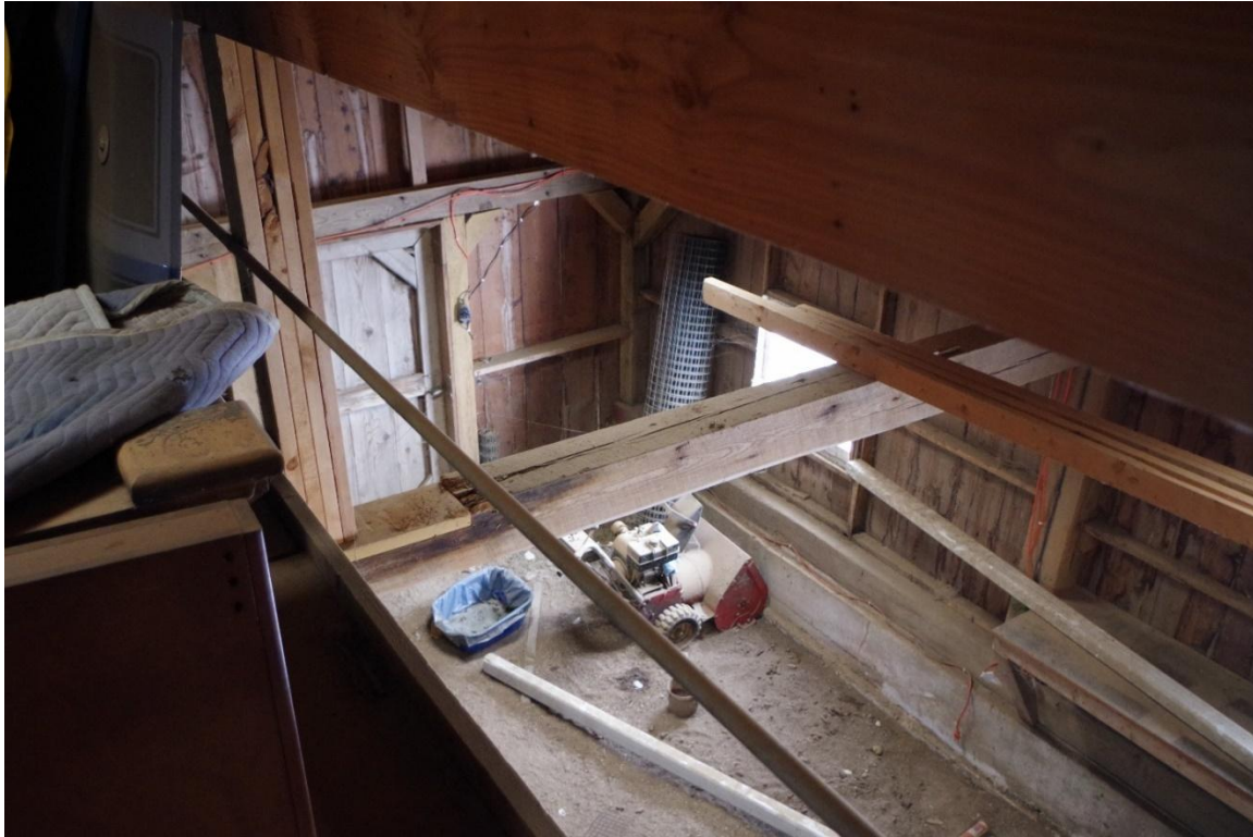
Photograph 37: View of the barn interior, looking northeast at the first floor of the east addition from the second level.
