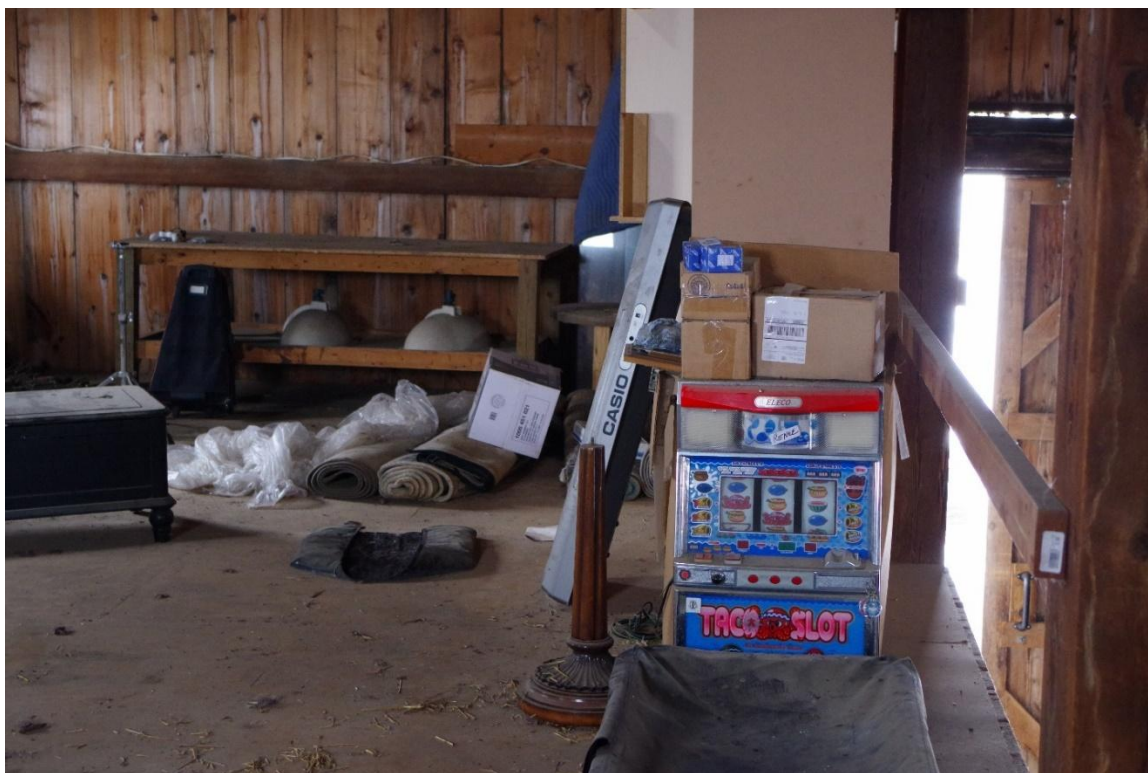
Photograph 40: View of barn interior, third level, camera facing west.
