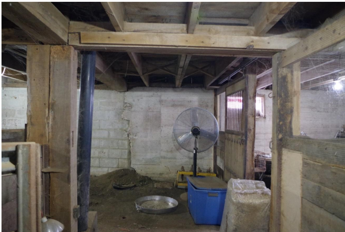
Photograph 28: View of barn interior, lower level, looking west.
