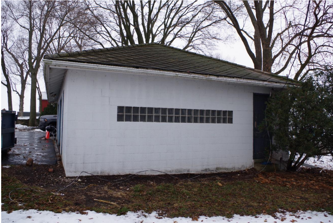
Photograph 47: View of the garage, view looking north.
