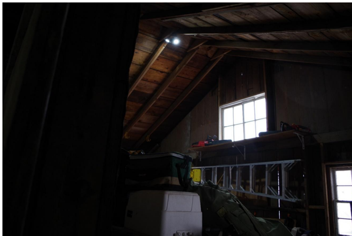
Photograph 24: Interior view of barn, south addition, lower level, looking southeast.
