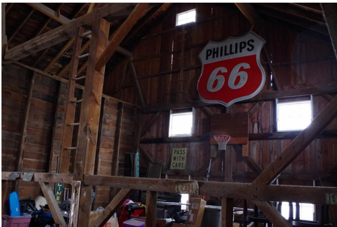
Photograph 31: View of barn interior, second level, camera facing northwest.
