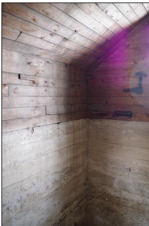
Photograph 56: Interior view of the cold storage building, camera facing southeast.
