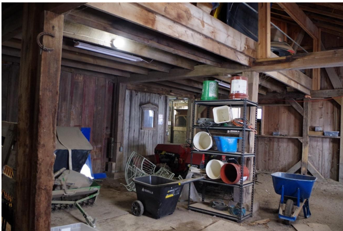
Photograph 26: View of barn interior, east addition, lower level, looking northwest.
