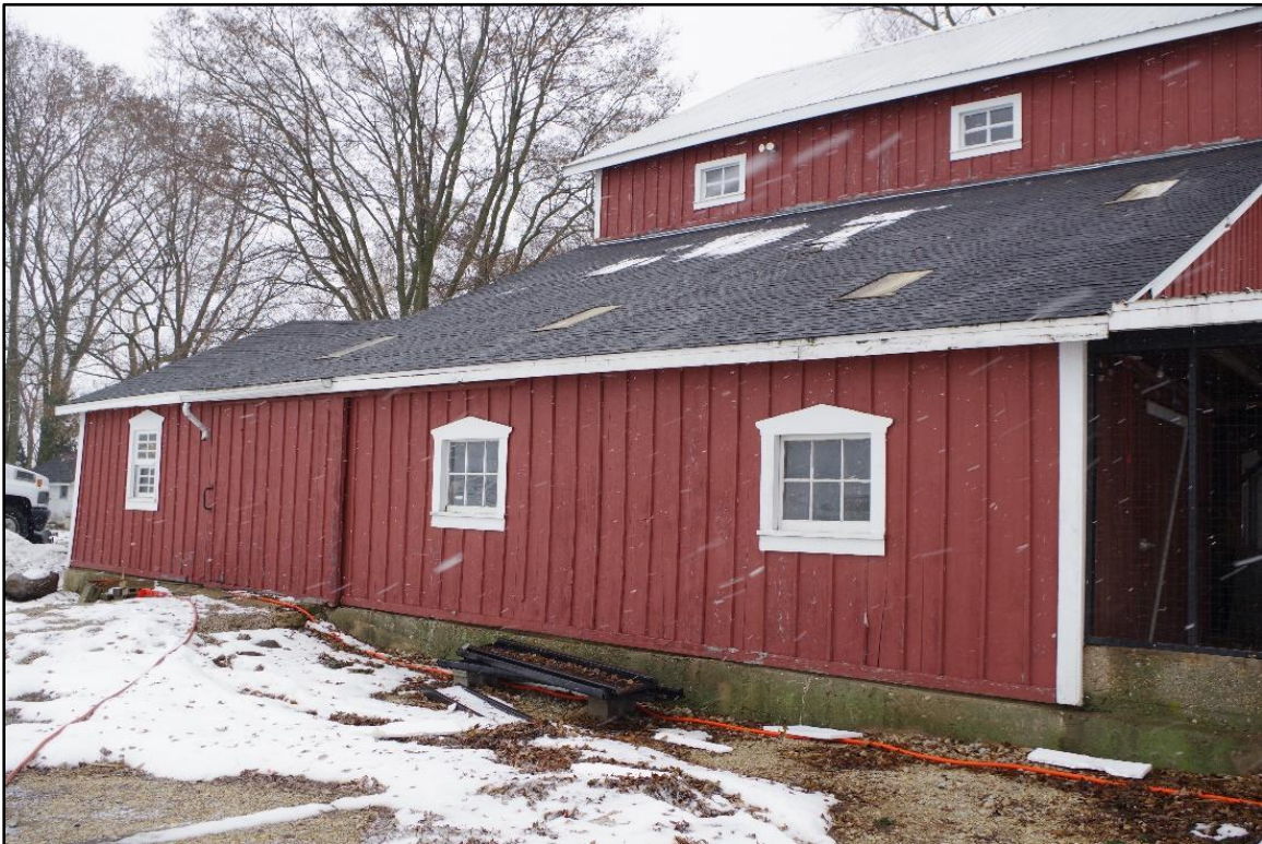
Photograph 20: View of the barn, camera facing southwest. December 2025.
