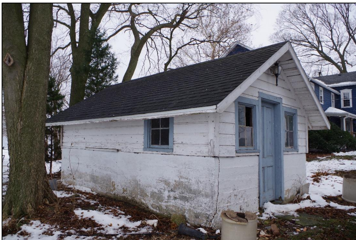
Photograph 51: View of the cold storage building, looking southwest.
