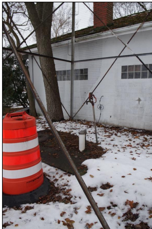
Photograph 44: View of windpump base, detail showing later pump and concrete slab, camera facing southwest.
