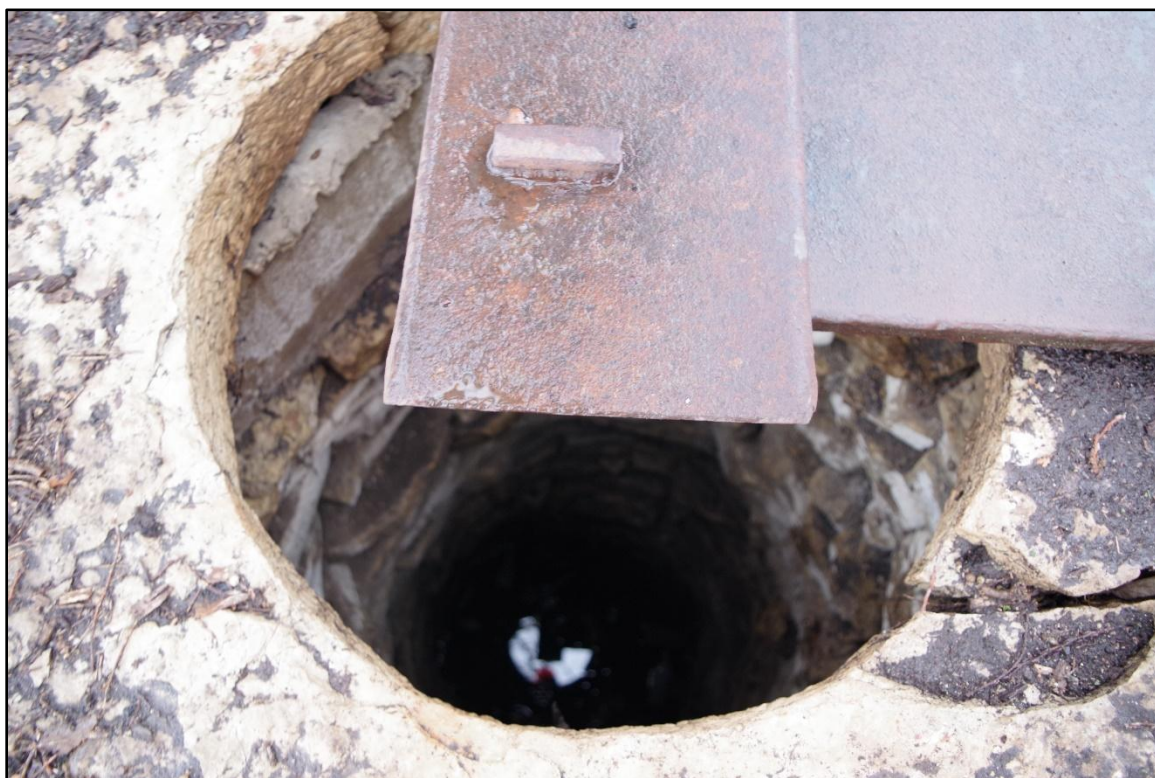
Photograph 13: Cistern, detail. December 2025.
