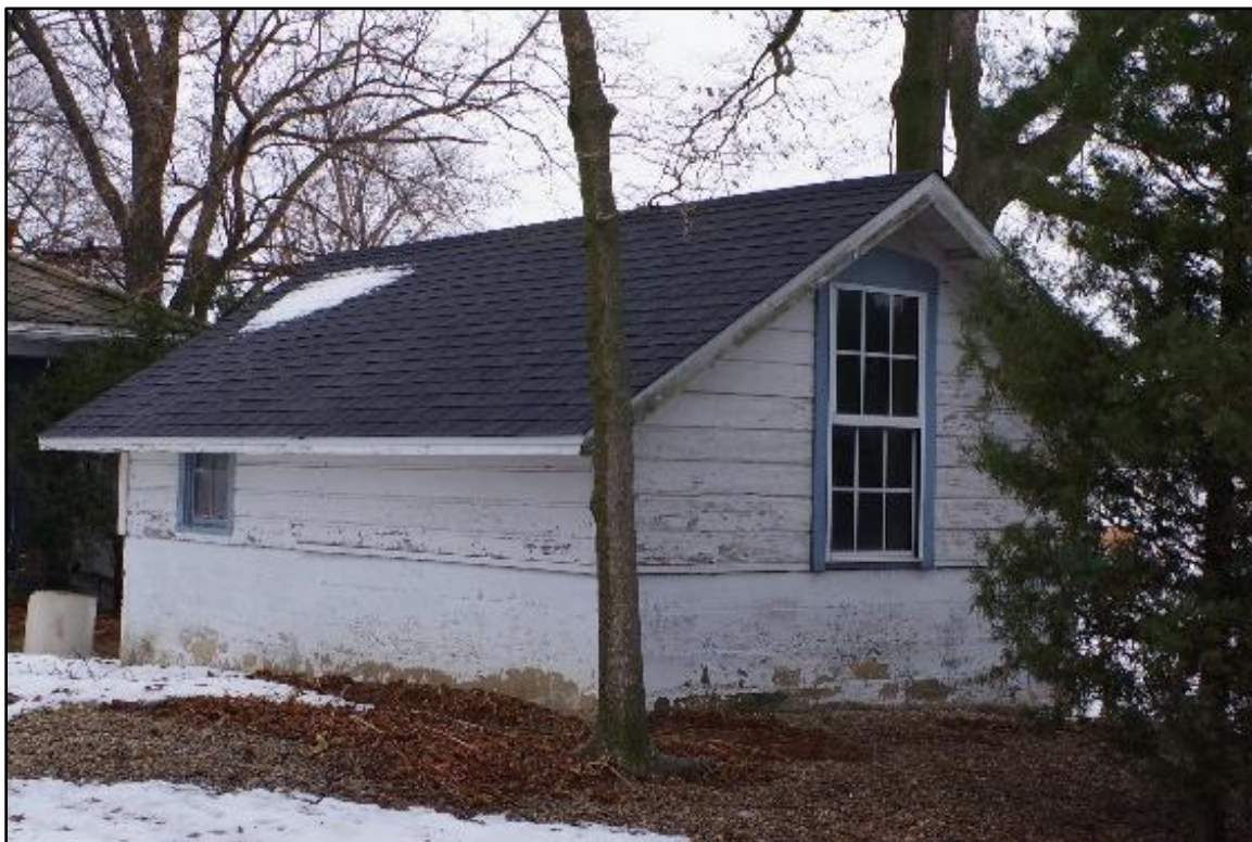
Photograph 53: View of the cold storage building, camera facing northeast.
