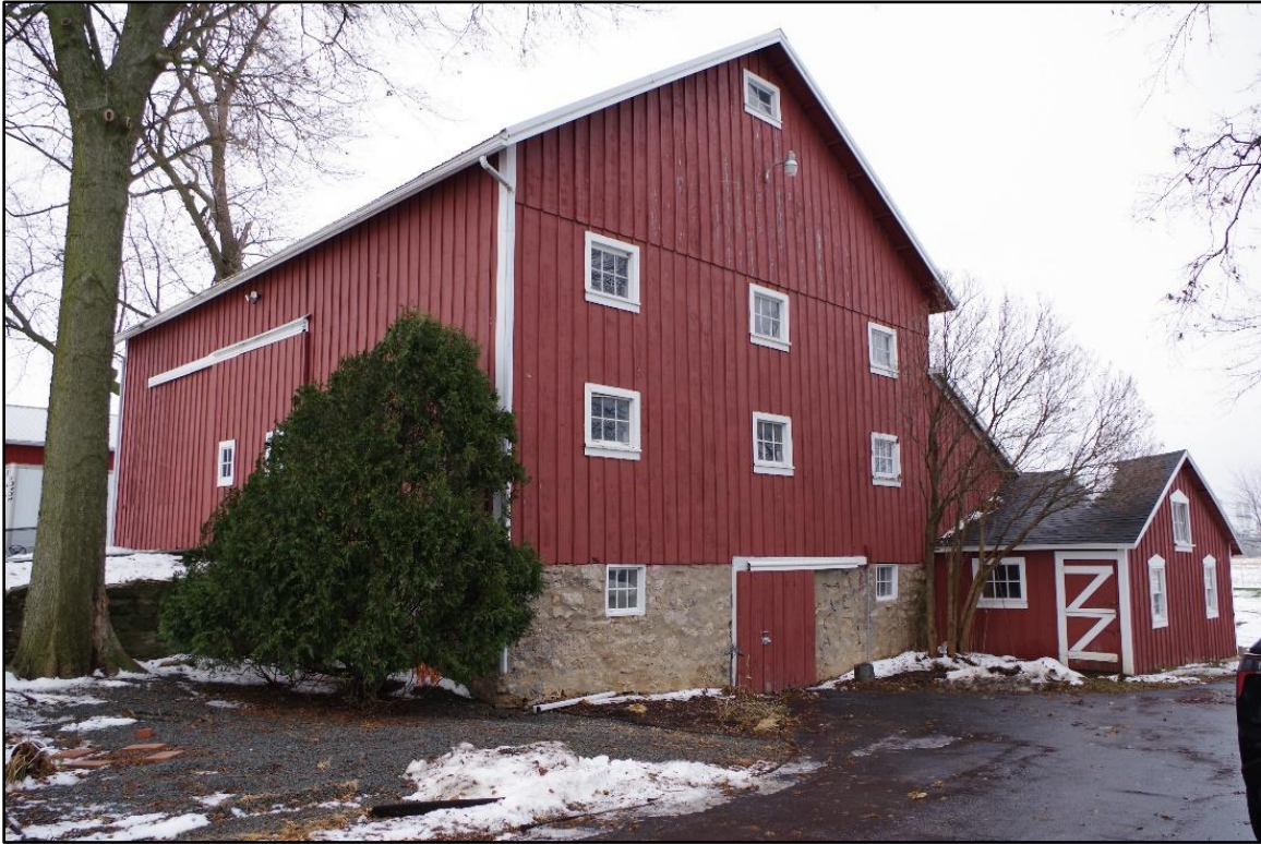
Photograph 15: View of the barn, camera facing northeast. December 2025.
