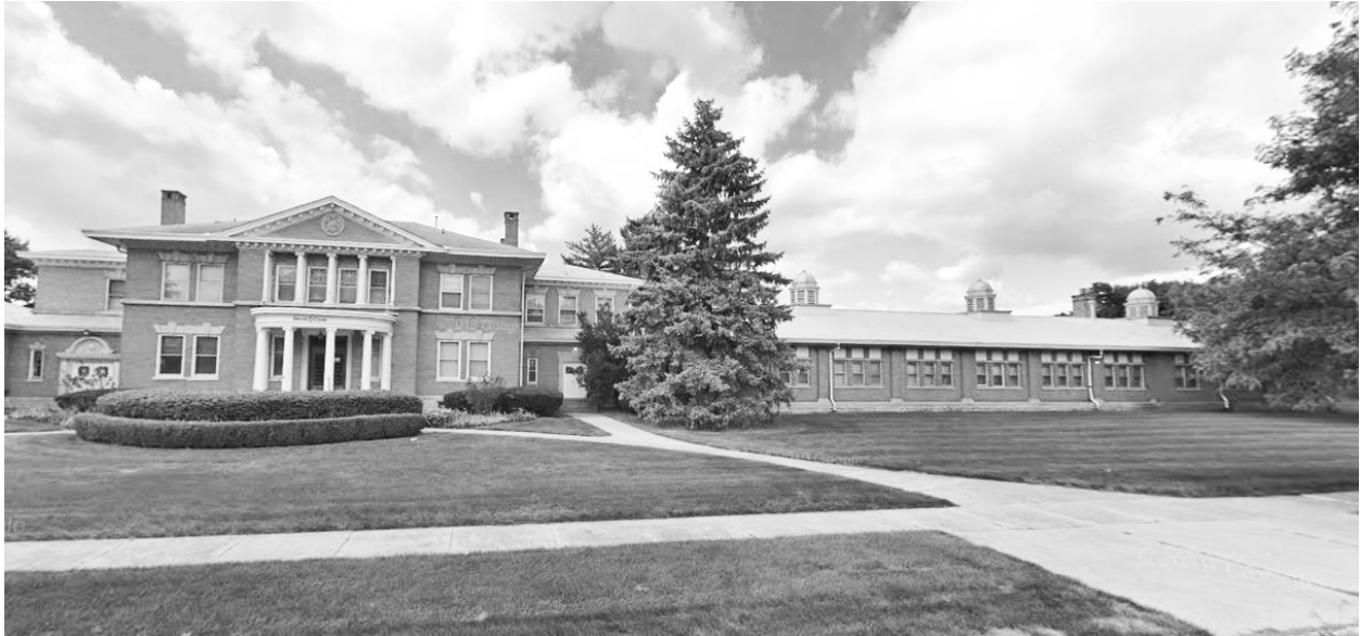
Figure 31. Main building and north wing, (Source: Google images, as shown in City of Elgin Application for Individual Landmark Designation, David C. Cook Publishing House )
