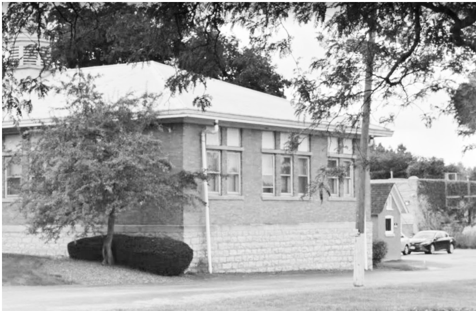
Figure 32. North elevation of north wing, 2018. (Source: Google images, as shown in City of Elgin Application for Individual Landmark Designation, David C. Cook Publishing House )
