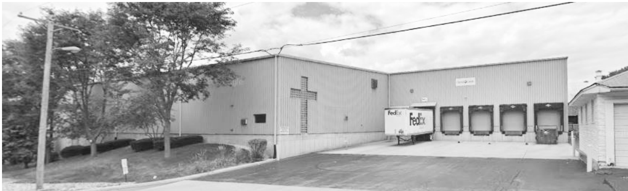
Figure 36. Truck garage/warehouse, 2018. (Source: Google images, as shown in City of Elgin Application for Individual Landmark Designation, David C. Cook Publishing House )
