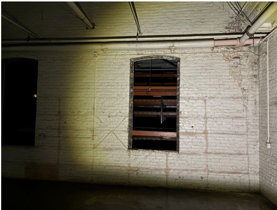
Figure 43. A window opening in the former exterior wall, with the west addition beyond, 2026. (Source: Wiss, Janney, Elstner Associates, Inc.)
