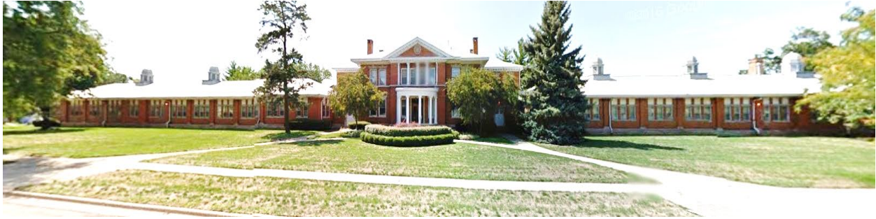
Figure 29. Front elevation of the main building, 2018. (Source: Google images, as shown in City of Elgin Application for Individual Landmark Designation , David C. Cook Publishing House)
