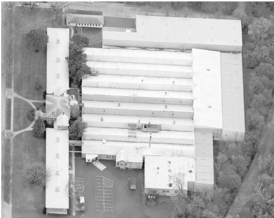
Figure 39. Aerial view of the complex, looking south, 2019. (Source: City of Elgin Application for Individual Landmark Designation , David C. Cook Publishing House)
