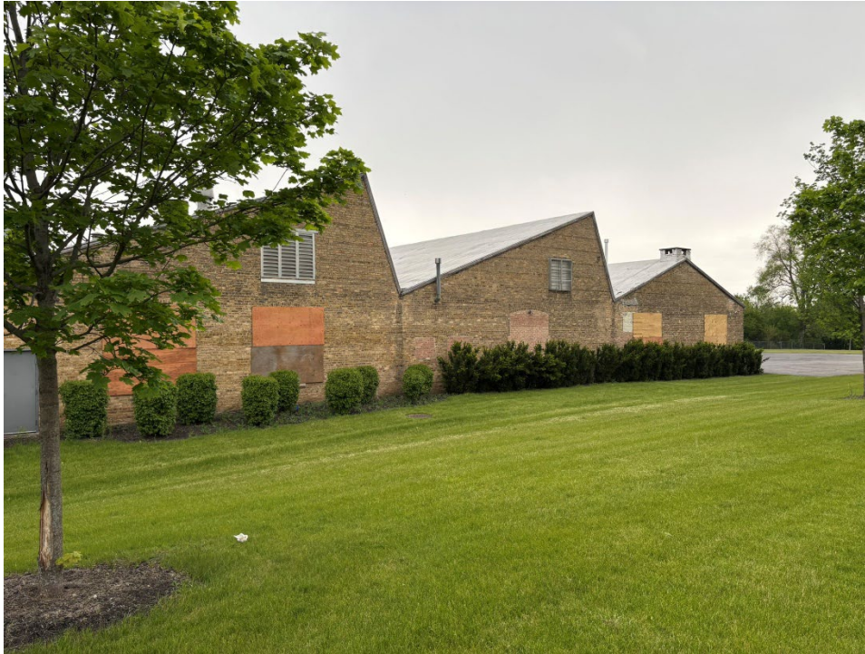
Figure 44. Partial east elevation of the factory building showing the saw-tooth roofs, 2026. (Source: Wiss, Janney, Elstner Associates, Inc.)
