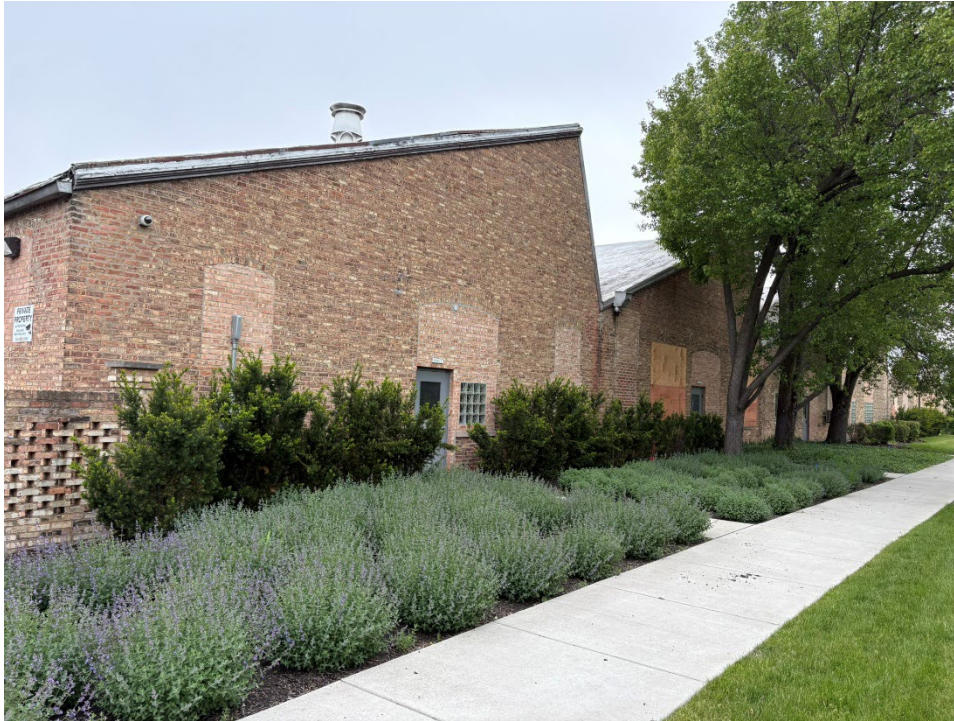
Figure 48. Partial east elevation of the 1911(right) and 1914 (left) additions to the factory building, 2026. (Source: Wiss, Janney, Elstner Associates, Inc.)
