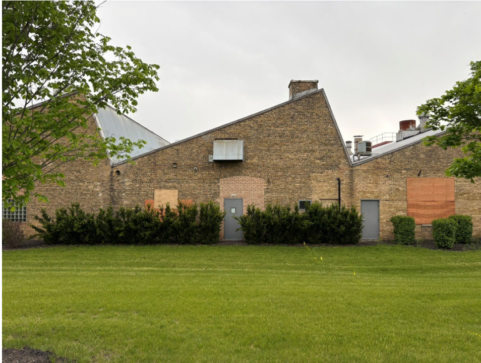
Figure 42. Partial east elevation of the factory building showing infilled openings, 2026. (Source: Wiss, Janney, Elstner Associates, Inc.)
