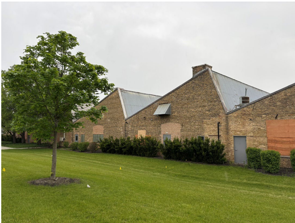
Figure 47. A brick chimney at the peak of a saw-tooth roof, along the north facade, 2026. (Source: Wiss, Janney, Elstner Associates, Inc.)
