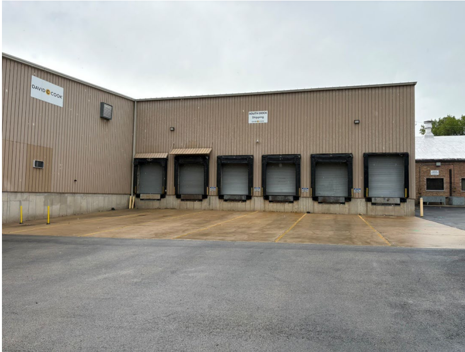
Figure 52. Loading dock at the south facade of the warehouse addition, 2026. (Source: Wiss, Janney, Elstner Associates, Inc.)
