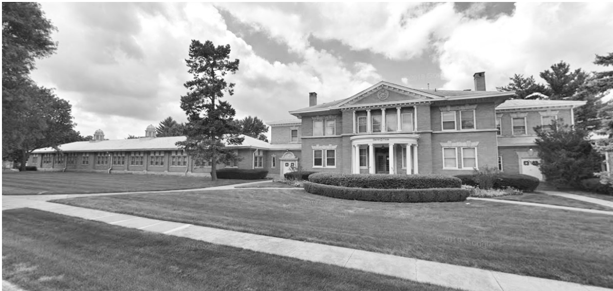
Figure 30. Main building and south wing, 2018. (Source: Google images, as shown in City of Elgin Application for Individual Landmark Designation , David C. Cook Publishing House)
