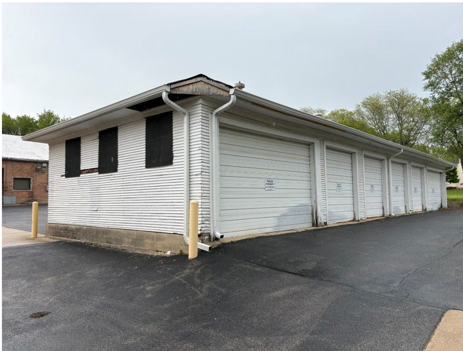
Figure 53. Southwest corner of the private garage, 2026. (Source: Wiss, Janney, Elstner Associates, Inc.)
