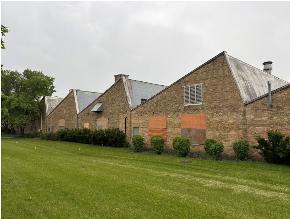
Figure 41. Partial east elevation of the factory building, 2026. (Source: Wiss, Janney, Elstner Associates, Inc. )
