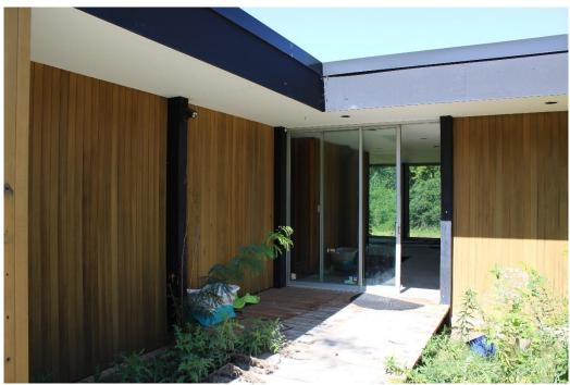
Figure 6: Detail of cedar siding, wood posts, projecting boxed eaves, and main entrance with sliding glass doors approached by wood deck.
