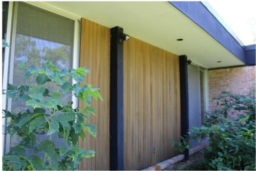
Figure 16: Detail of bedroom wing's north wall, showing wood siding, wood posts, and boxed, overhanging eaves.
