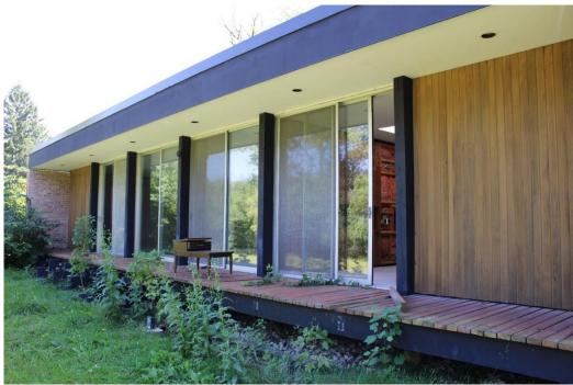
Figure 14: Detailing of living/dining room wall with continuous sliding glass doors and fixed glass panels, cedar siding and wood posts, and wood decking.
