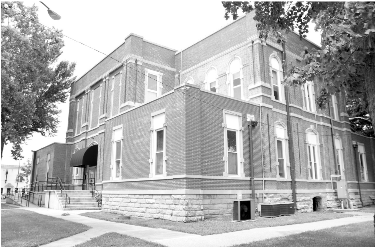
Photograph 75: Facing northwest toward the southeast corner of the building
