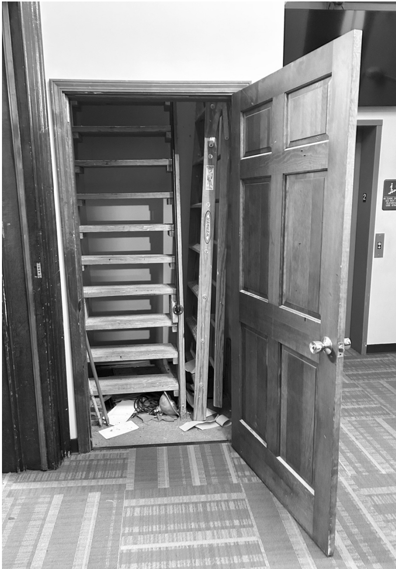
Photograph 62: Standing on the second-floor Elevator Landing with a view of the ladder to the attic
