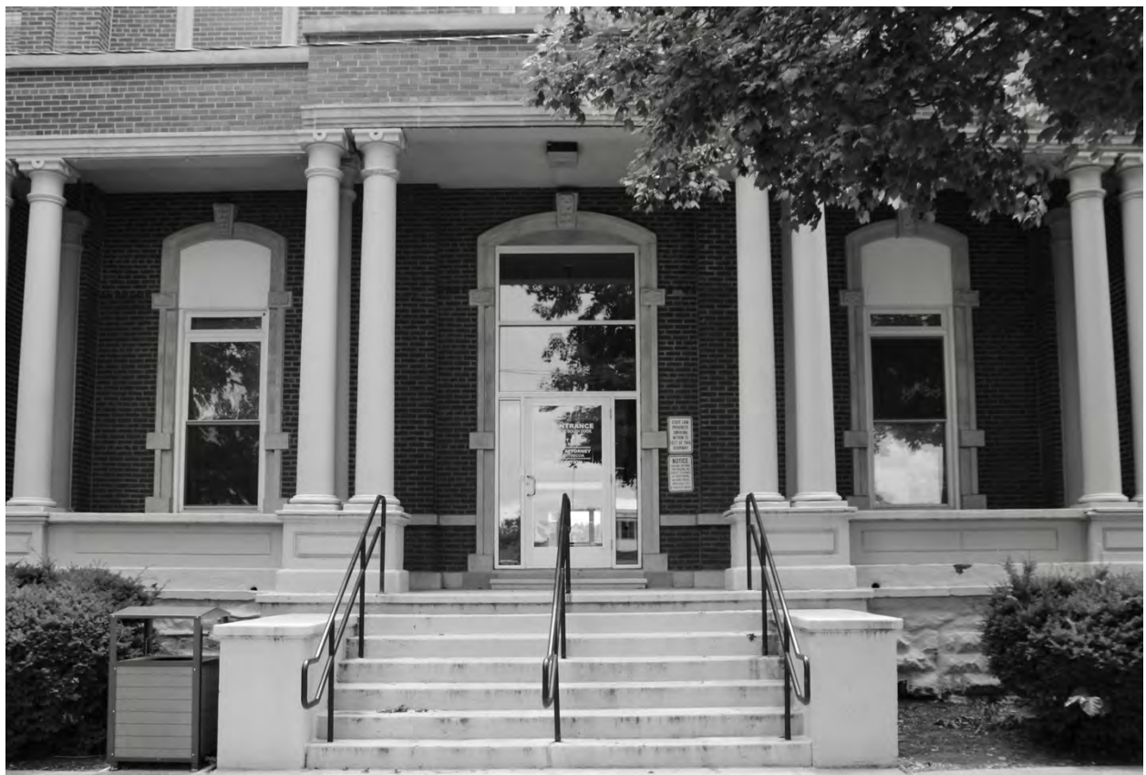
Photograph 90: Facing south toward the north entrance and columns
