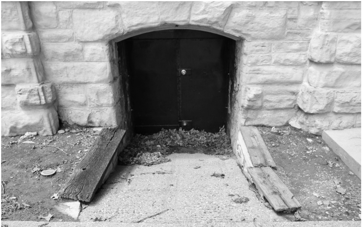
Photograph 68: Facing west toward the exterior of the half-sized double doors used for service access to the basement on the east elevation of the building
