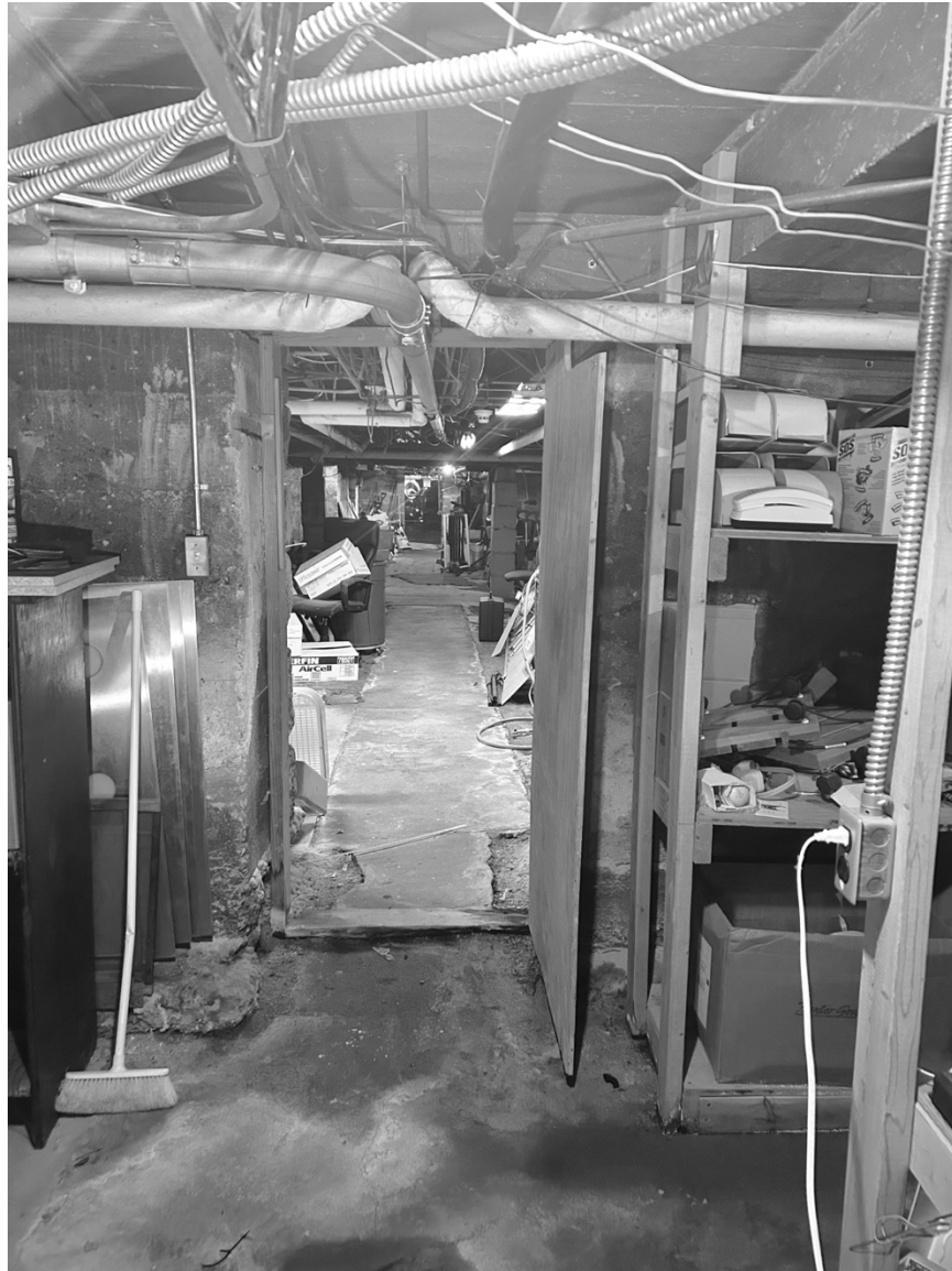
Photograph 66: Standing in the west side of the basement, facing east
