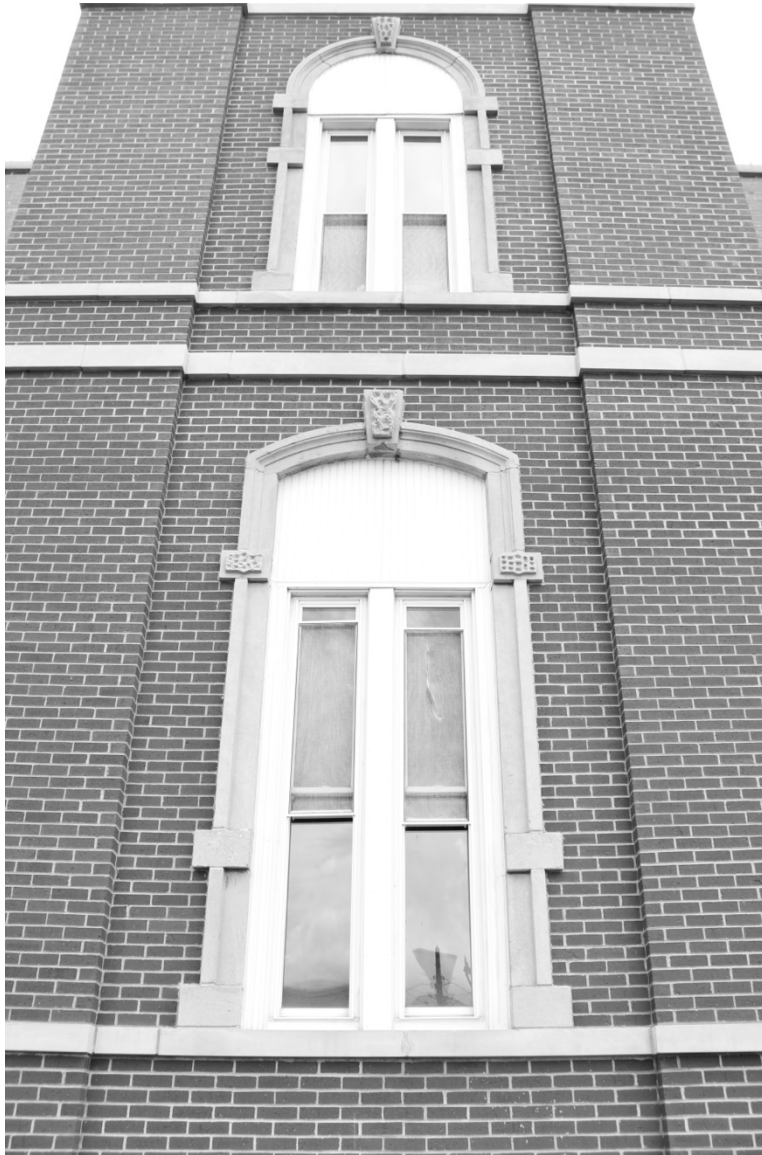
Photograph 87: Facing east toward the West Addition
