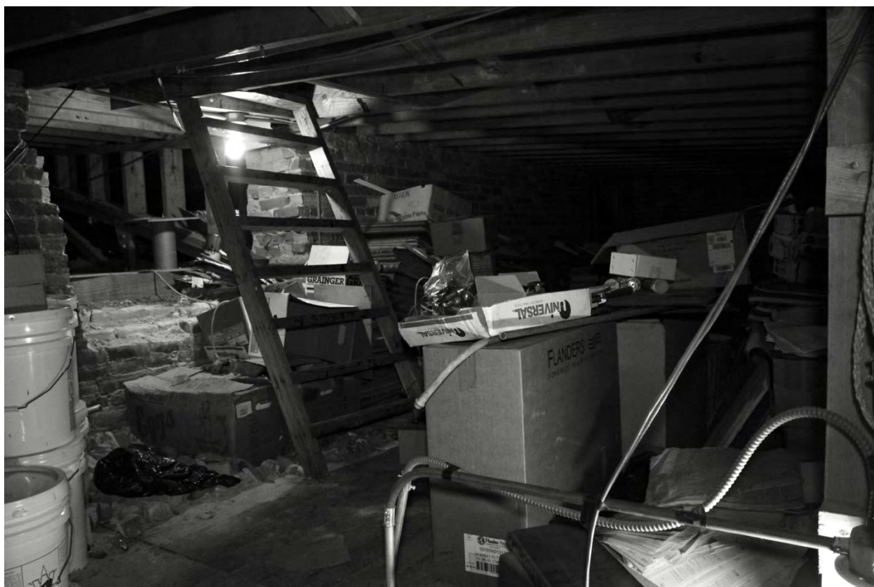
Photograph 63: Standing in the attic facing the trap door to the roof, facing southeast
