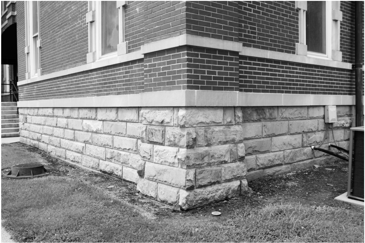
Photograph 76: Facing northwest toward the masonry and raised foundation located on the southeast corner of the building
