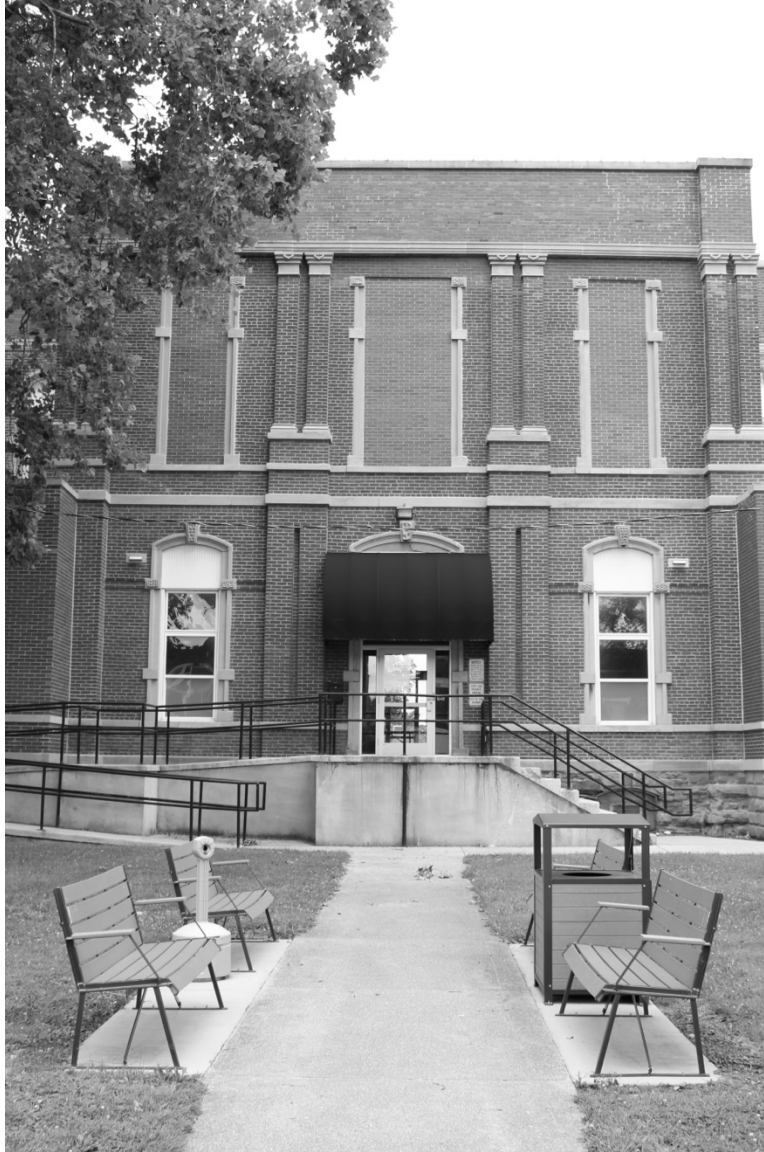
Photograph 78: Facing north toward the south entrance to the building
