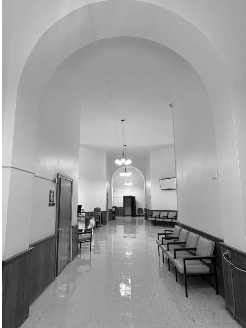
Photograph 22: Facing west in the Lobby with a view of the symmetrical archways in the east-west corridor that forms the apse, nave, and crossing of the cross-shaped courthouse building
