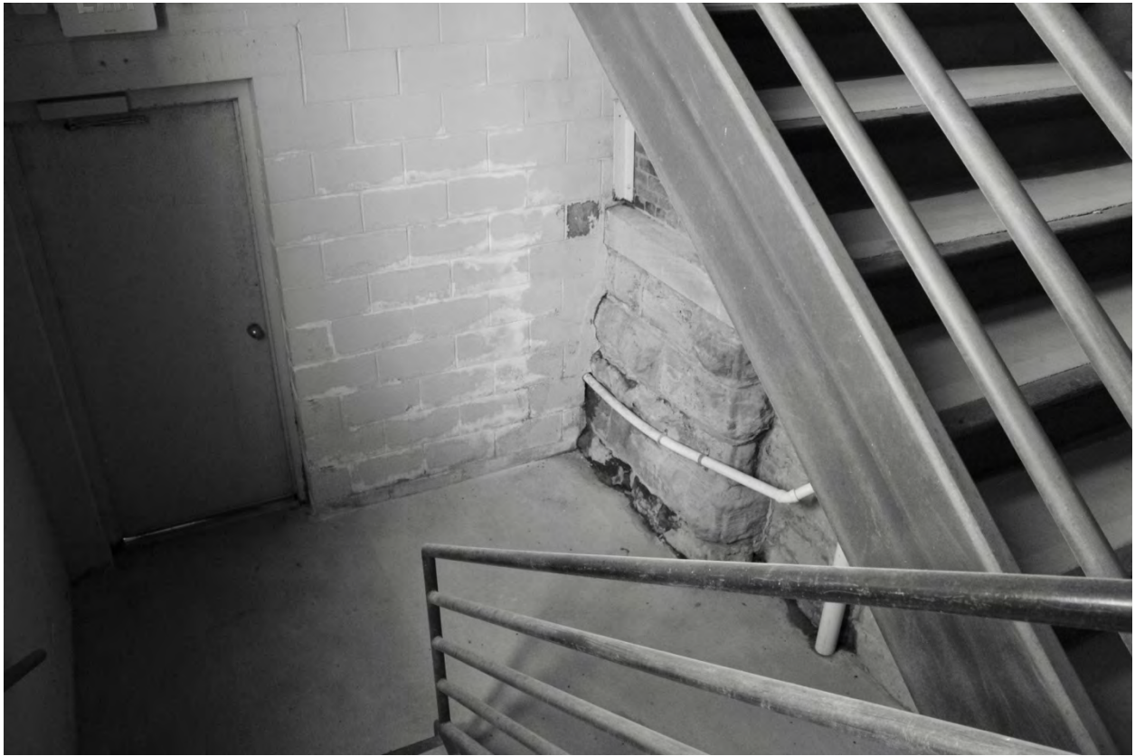
Photograph 61: Facing north toward the bottom of the stairs and ground floor exit from the West Addition
