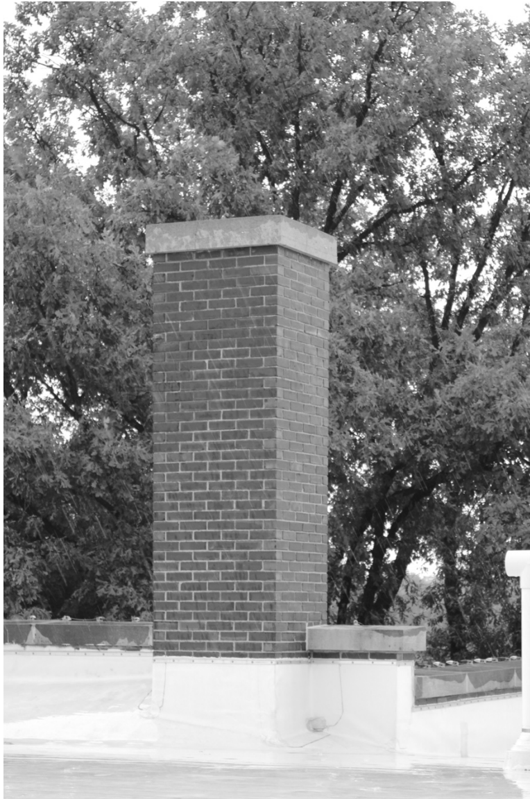
Photograph 65: Standing in the attic trap door, facing northeast with a view of the chimney on the roof
