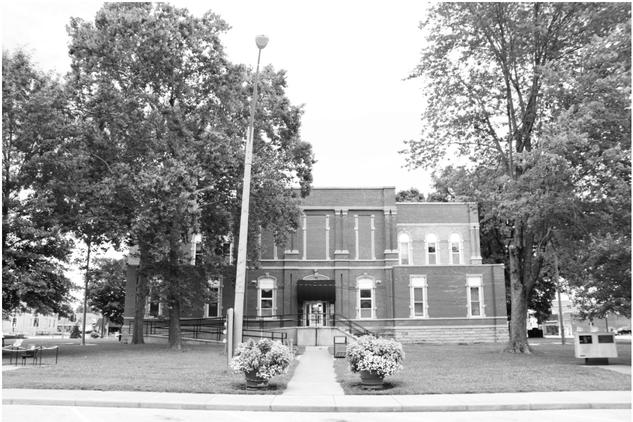
Photograph 79: Facing north toward the south entrance and grounds
