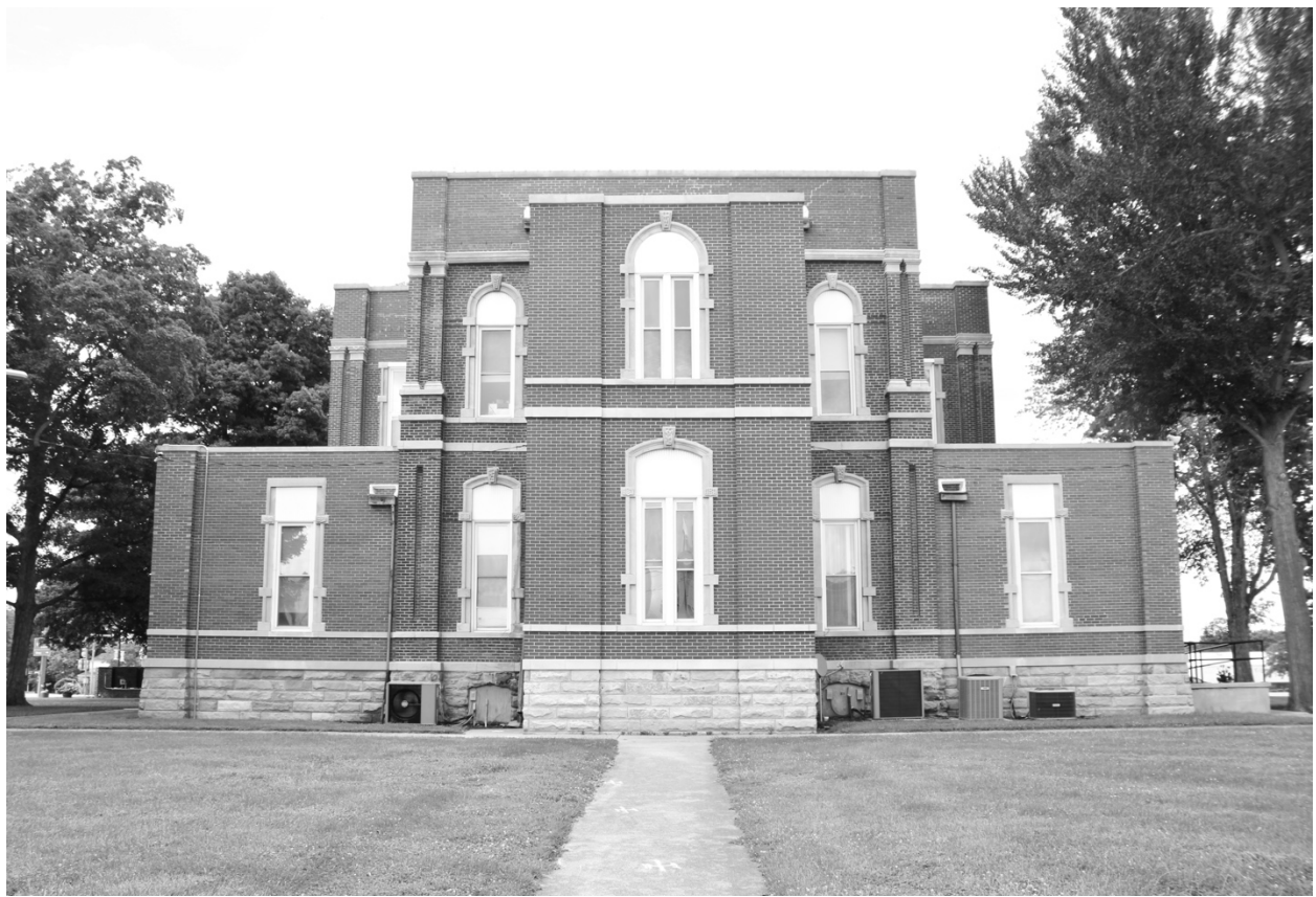
Photograph 86: Facing east toward the west elevation of the building
