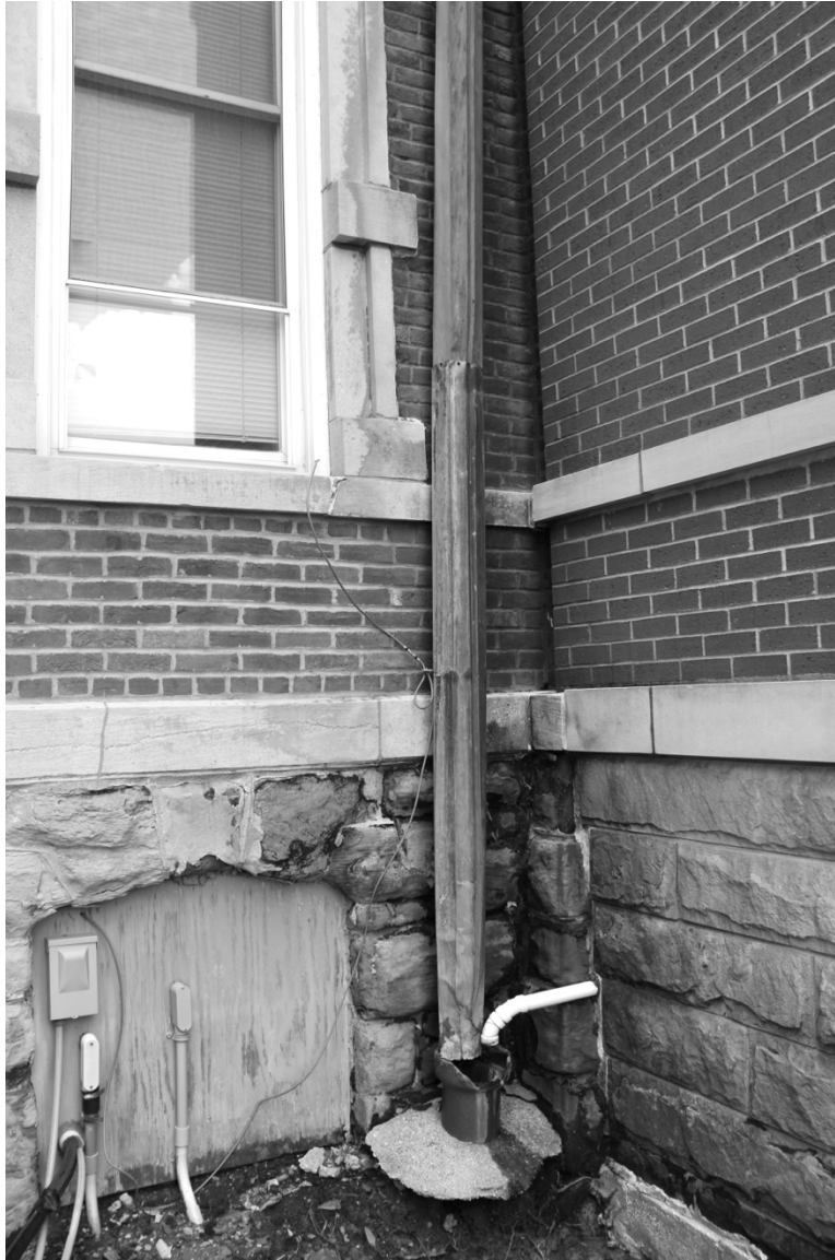
Photograph 88: Facing southeast toward the northeast elevation of the West Addition, where the newer brick veneer in the West Addition meets the older bricks in the west wall
