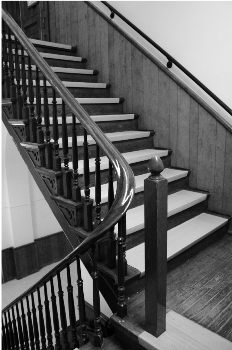
Photograph 33: Facing southwest on the Stair Landing
