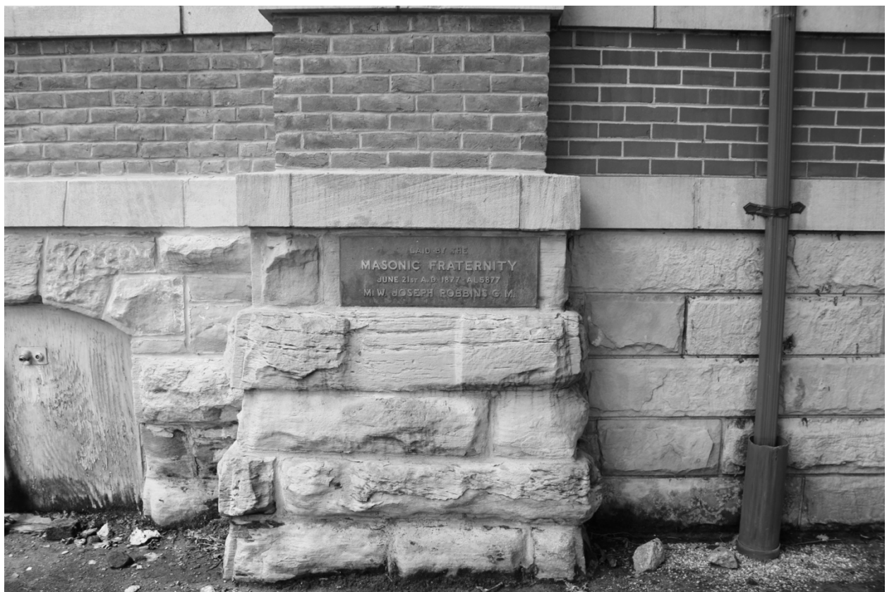
Photograph 73: A distance view of the 1877 plaque giving tribute to the craftsmanship of the Free Masons
