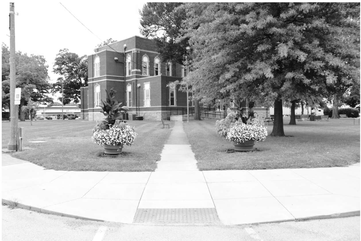
Photograph 85: Facing northeast toward the southwest elevation of the building
