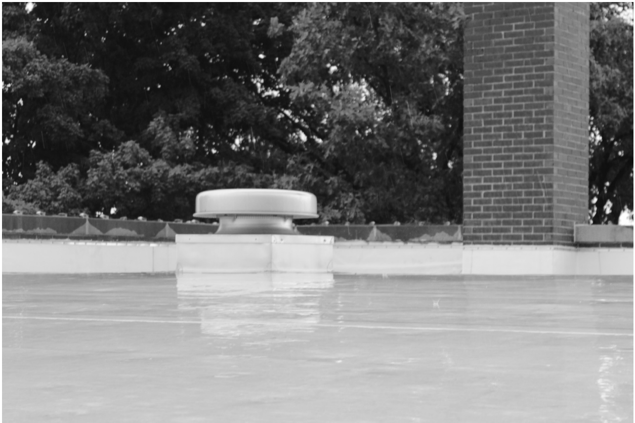
Photograph 64: Standing in the attic trap door, facing southeast with a view of the roof
