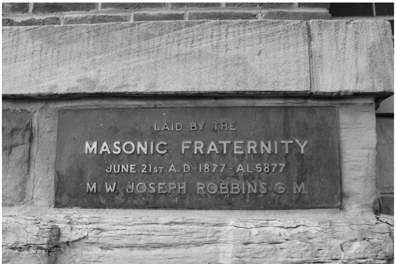
Photograph 72: Facing west toward the east elevation of the building and an 1877 Free Masons plaque
