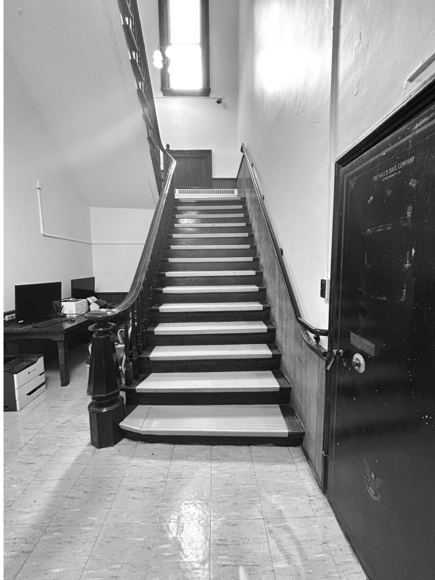
Photograph 32: Facing north toward the stairs
