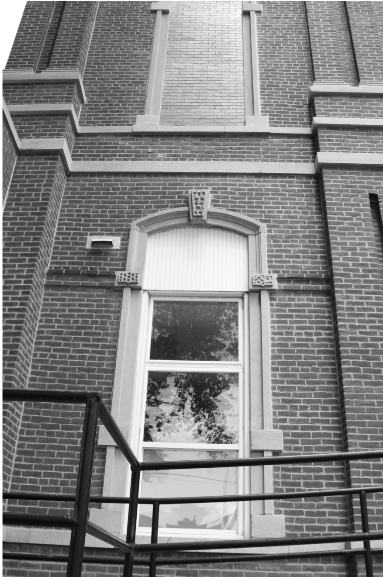
Photograph 80: Facing north toward the south elevation of the building with a view of an arched window
