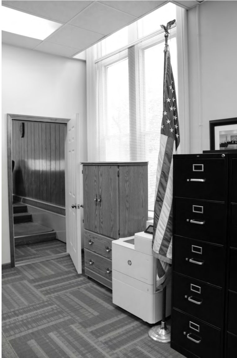
Photograph 50: Facing west/northwest in the Law Library with a view of the low ceilings built to hide ductwork without damaging the arched windows
