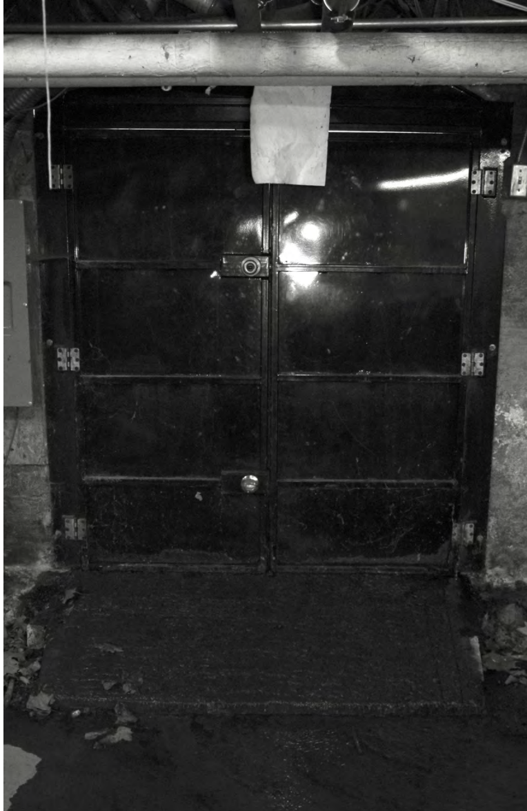
Photograph 67: Facing east in the interior of the east side of the basement as water from a rainstorm leaks through the half-sized double doors used for service
