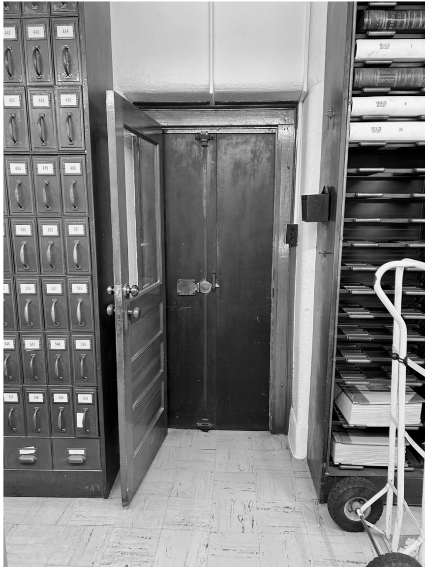
Photograph 13: Facing west toward a vault door that exits from the Clerk's Archives to the Lobby
