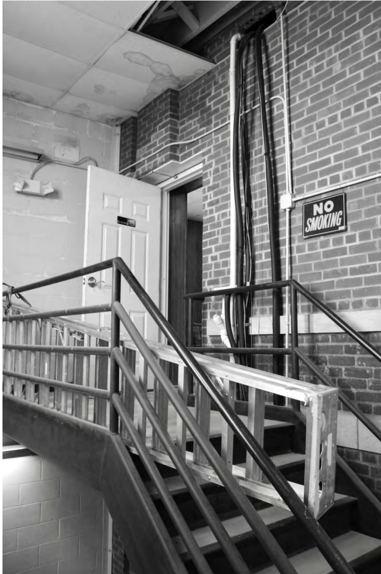
Photograph 59: Standing on the second-floor Landing in the West Addition, facing northeast toward the door to the Jury Meeting Room
