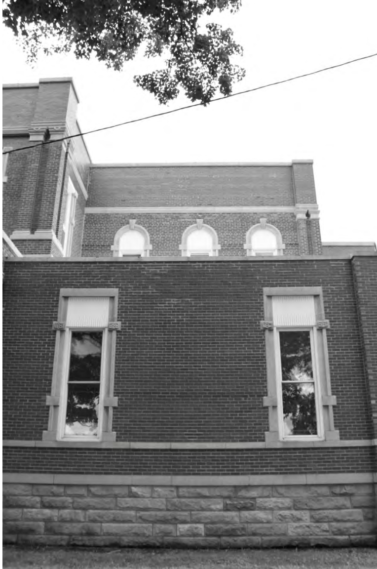
Photograph 77: Facing north toward the south elevation of the building with a view of the windows
