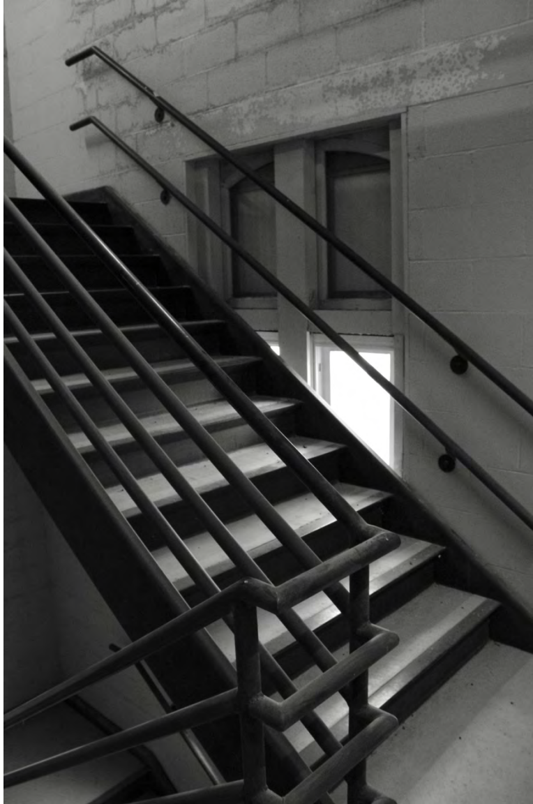
Photograph 60: Standing on the mid-landing in the West Addition, facing south
