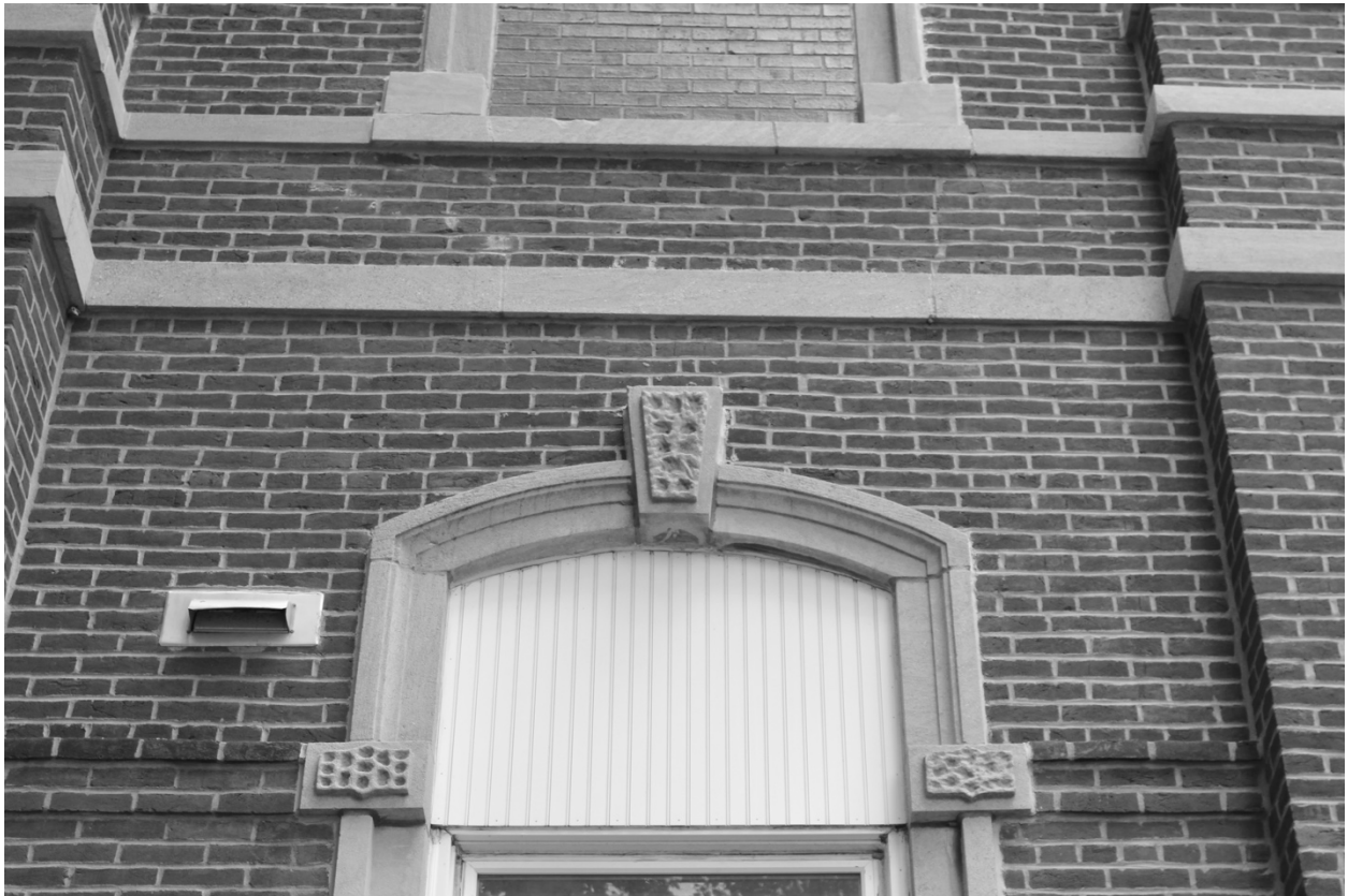
Photograph 81: Facing north toward the south elevation of the building with a view of the wood replacement in the upper fan of the arched window
