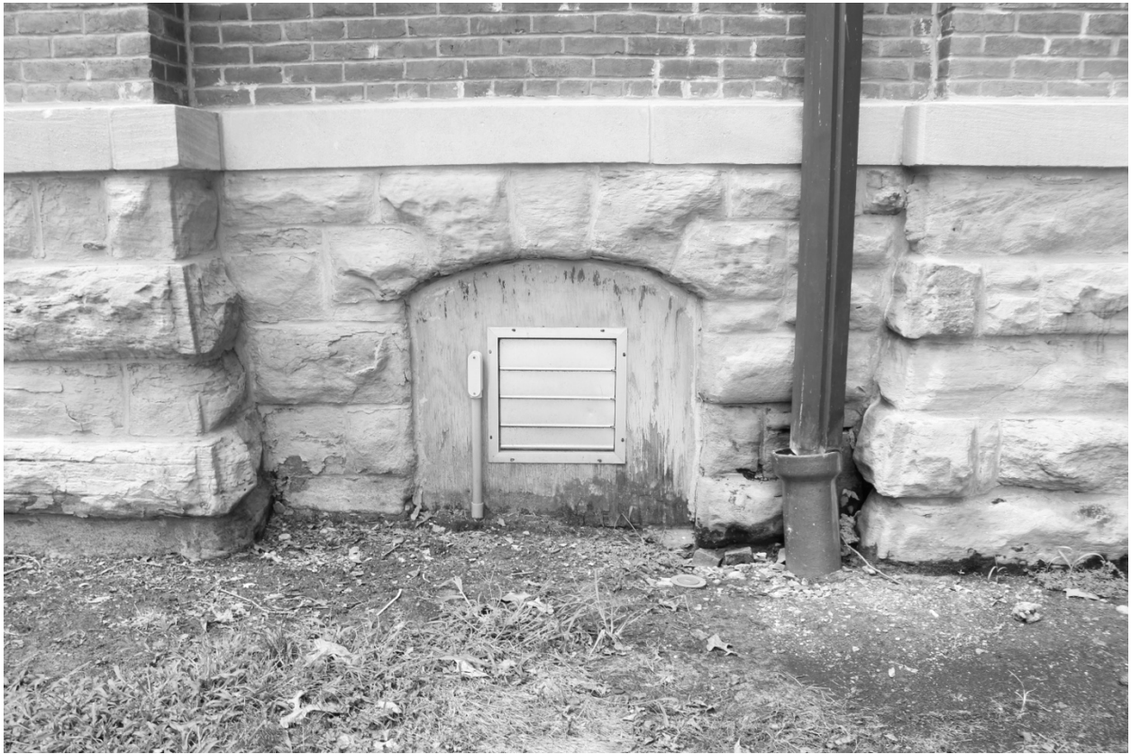
Photograph 70: Facing west toward a vent on the exterior of the east elevation of the building
