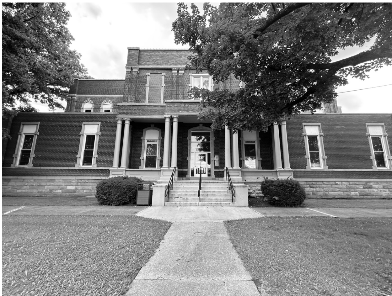
Photograph 91: Facing south toward the north side of the building
