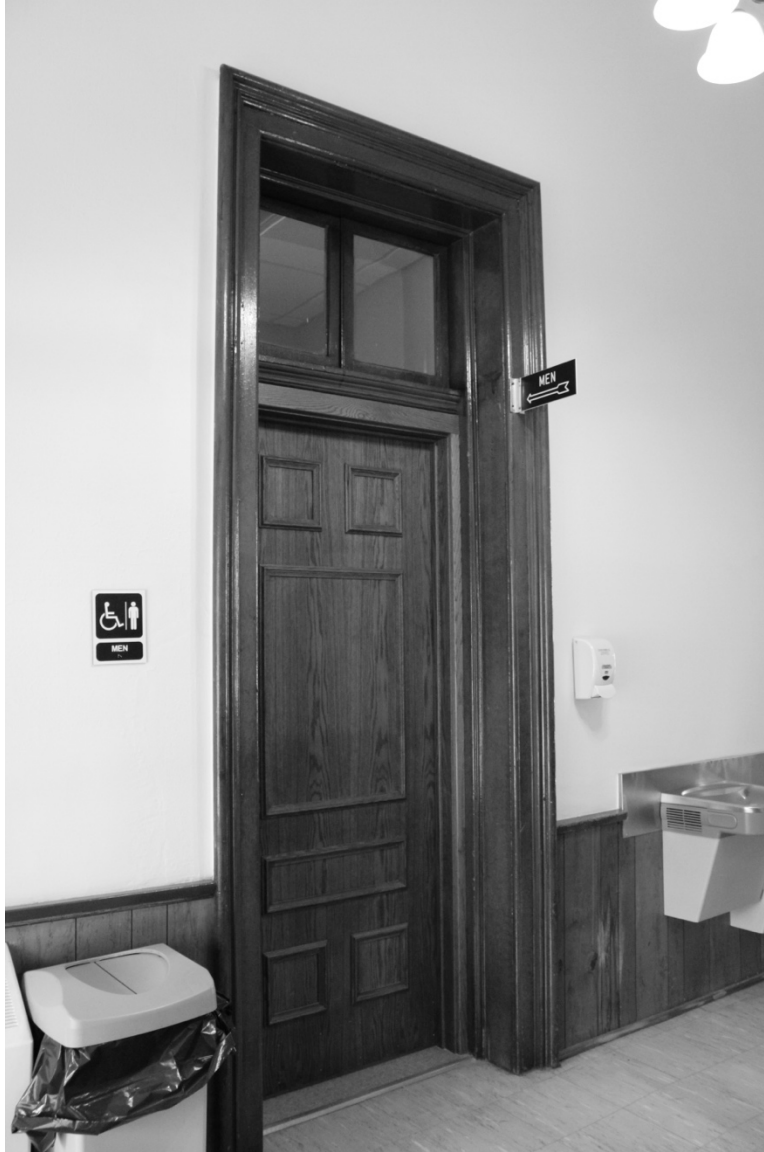
Photograph 27: Facing southwest in the Lobby with a view of the Men's Restroom
