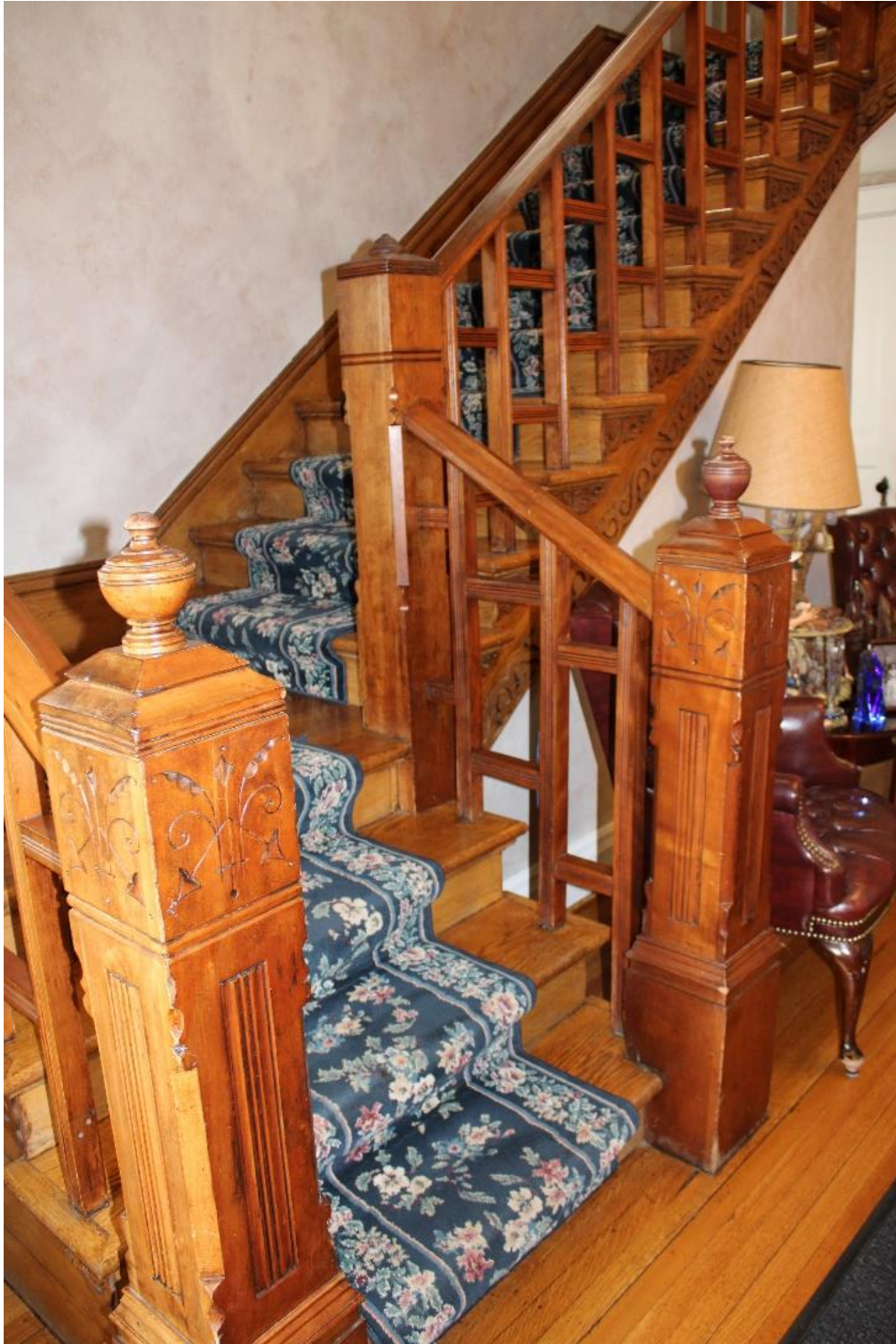
Figure 21: Detail of carved wood newell posts on main staircase.
