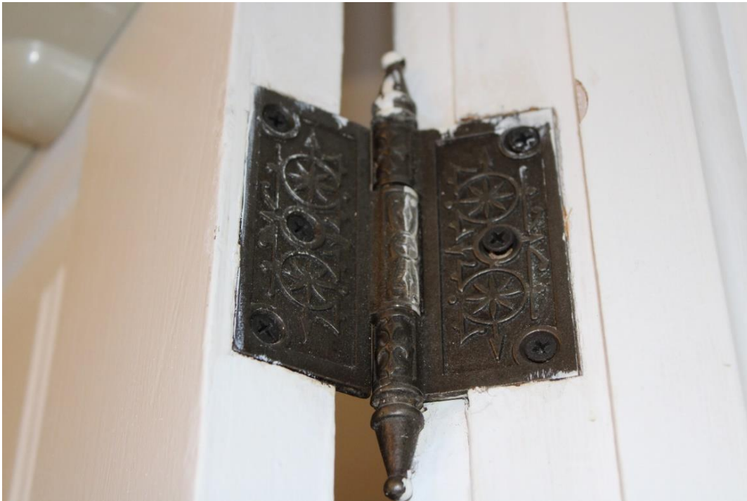
Figure 28: Typical original door hinge.
