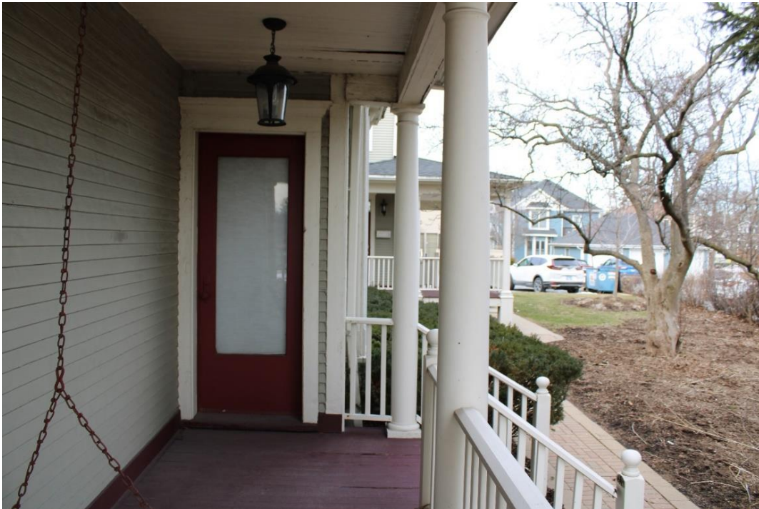
Figure 18: East façade porch entrance, view north.
