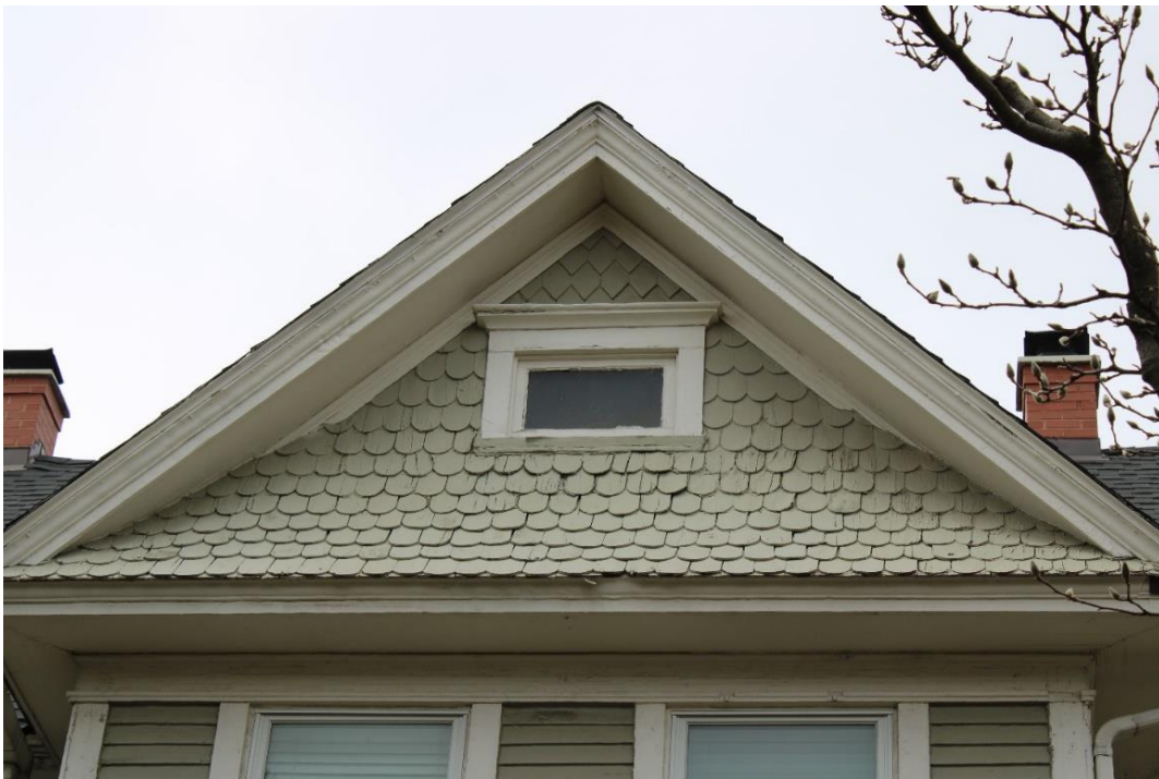
Figure 9: Detail of gable with wood shingles on front facade.
