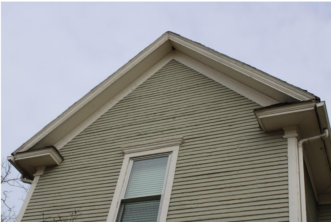
Figure 11: Gable pavilion on west façade showing wood frieze band and cornice returns.
