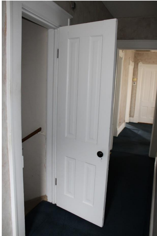
Figure 32: Second floor hallway with doorway to secondary staircase on the left.
