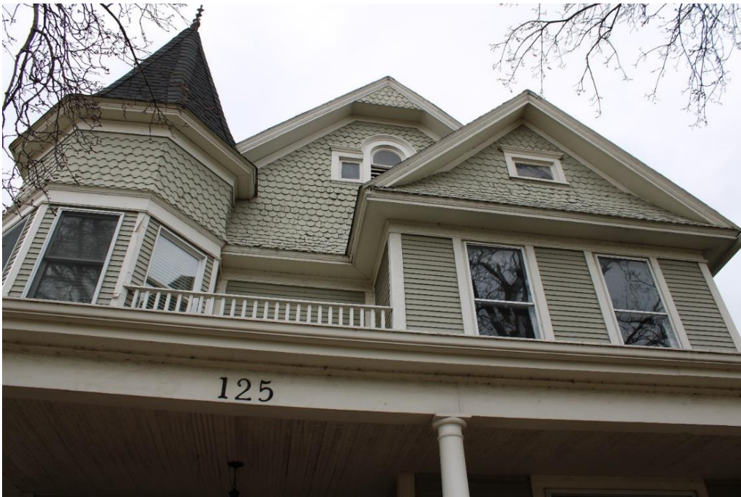
Figure 5: Detail of front façade's second floor, view north.
