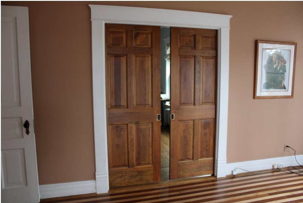
Figure 24: Pocket doors between Offices 2 and 3, view northeast.
