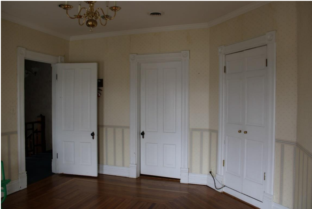
Figure 34: Office 6 on second floor, view north.
