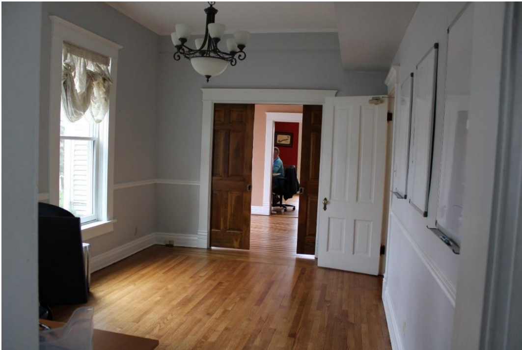
Figure 26: Pocket doors separating Offices 2 and 3, view southeast.
