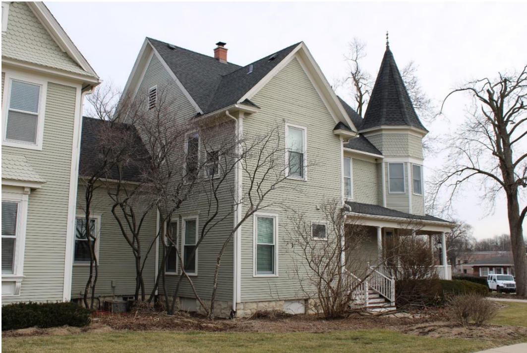
Figure 14: North (left) and west facades of the original house, view southeast.
