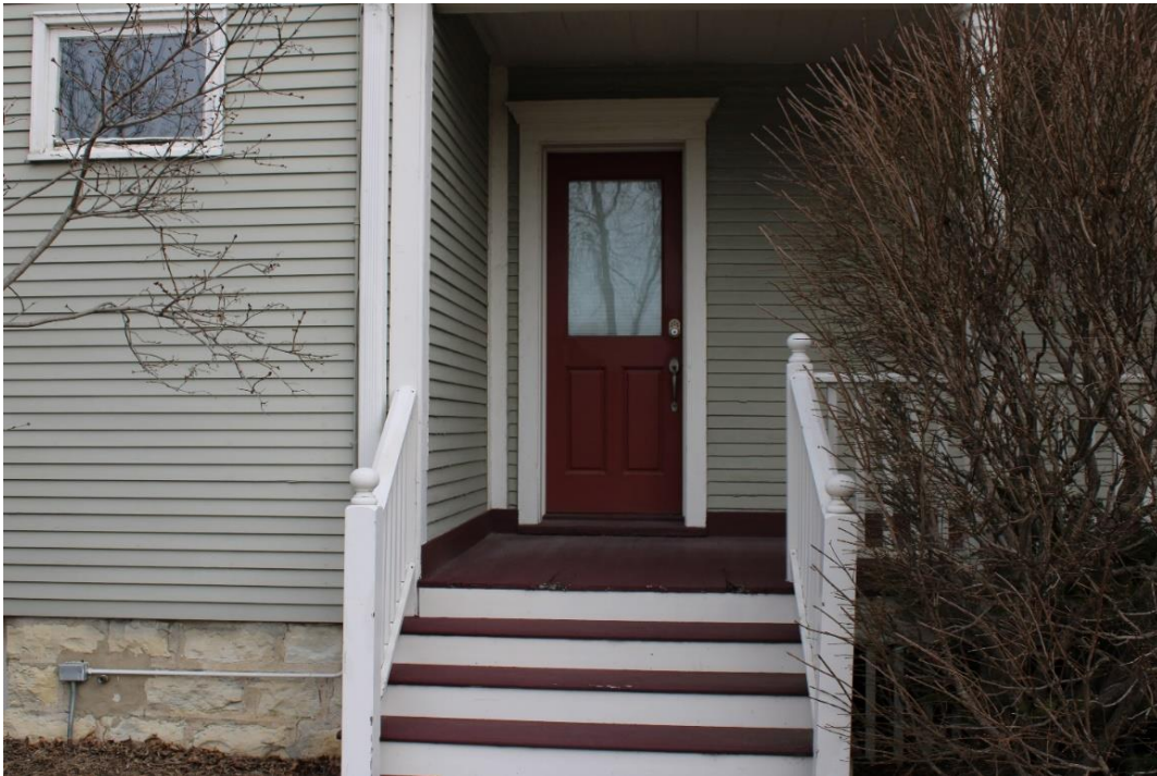
Figure 12: West façade entrance on wraparound porch.
