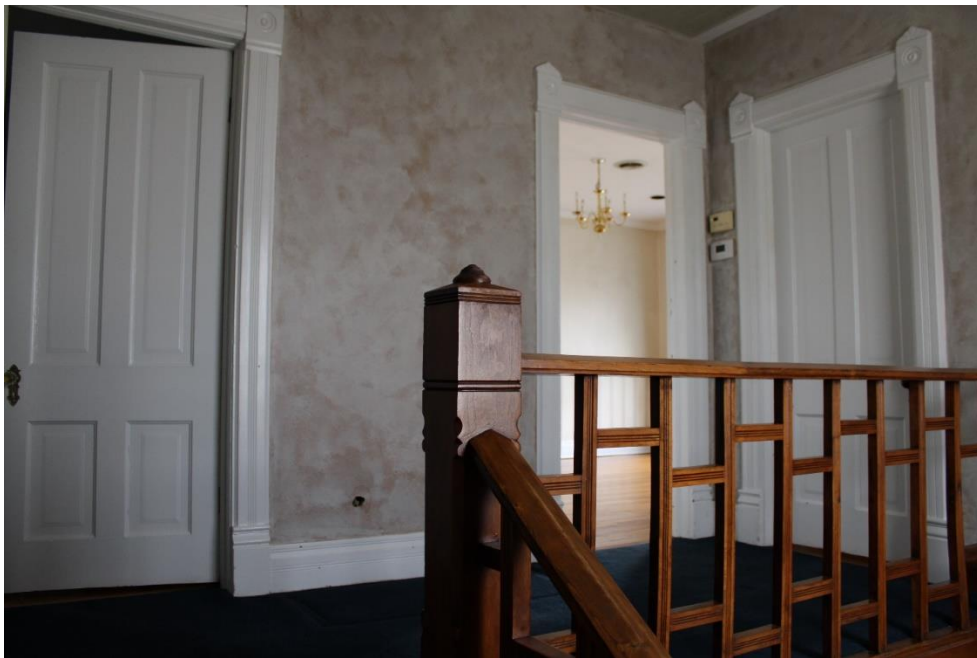
Figure 33: Second floor hallway showing wood railings and newell post of main staircase.
