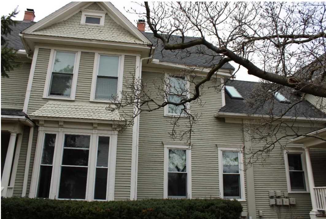
Figure 19: East façade, view west.
