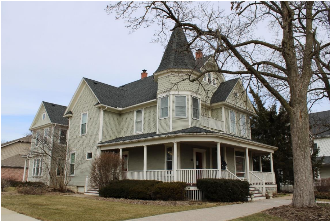
Figure 10: View northeast showing polygonal corner tower with conical roof.
