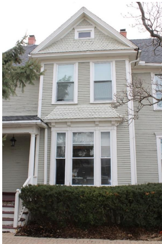
Figure 17: Detail of gable pavilion with bay window on east façade, view west.
