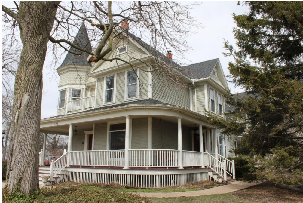
Figure 16: Front (south) and east facades, showing wraparound porch, view northwest.
