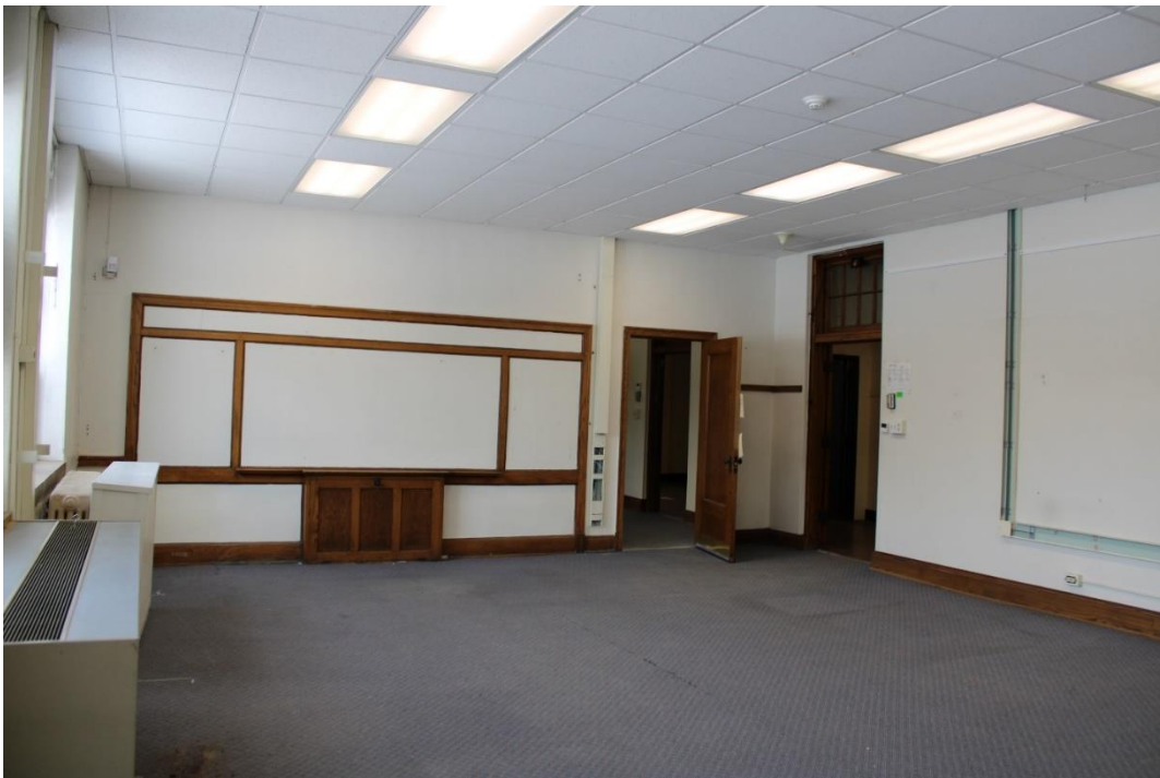
Figure 32: Classroom near the southwest corner of the school, looking northeast.
