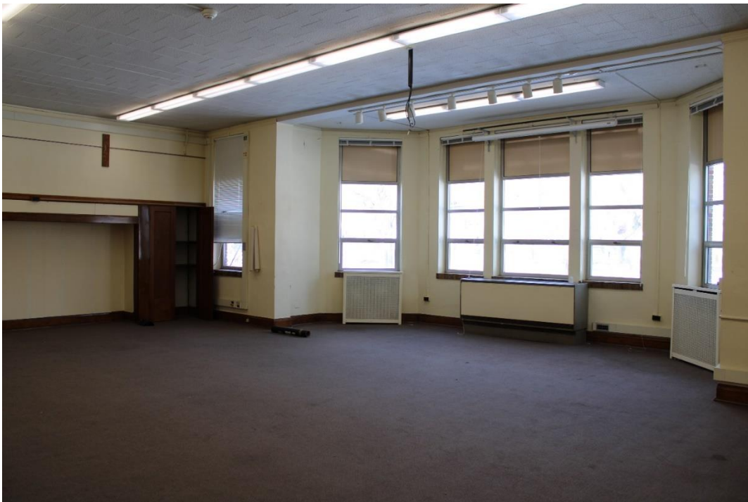
Figure 24: Kindergarten, looking northwest.
