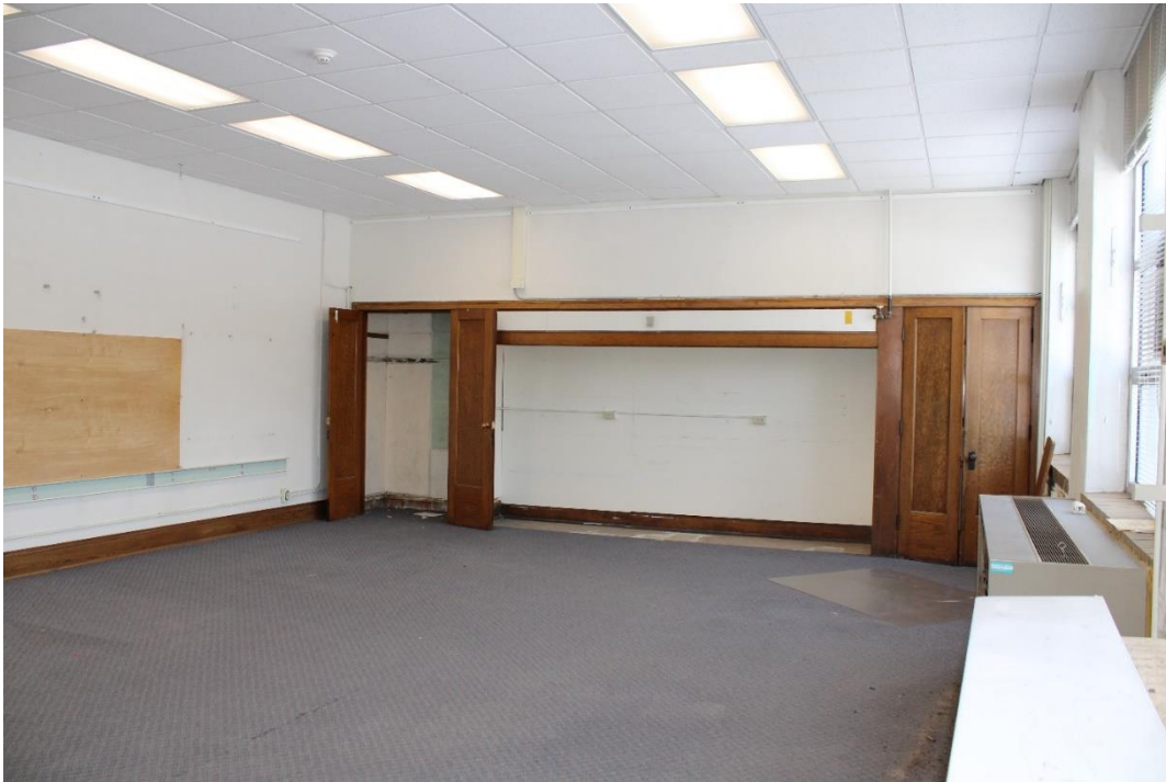
Figure 33: Classroom near the southwest corner of school, looking southeast.
