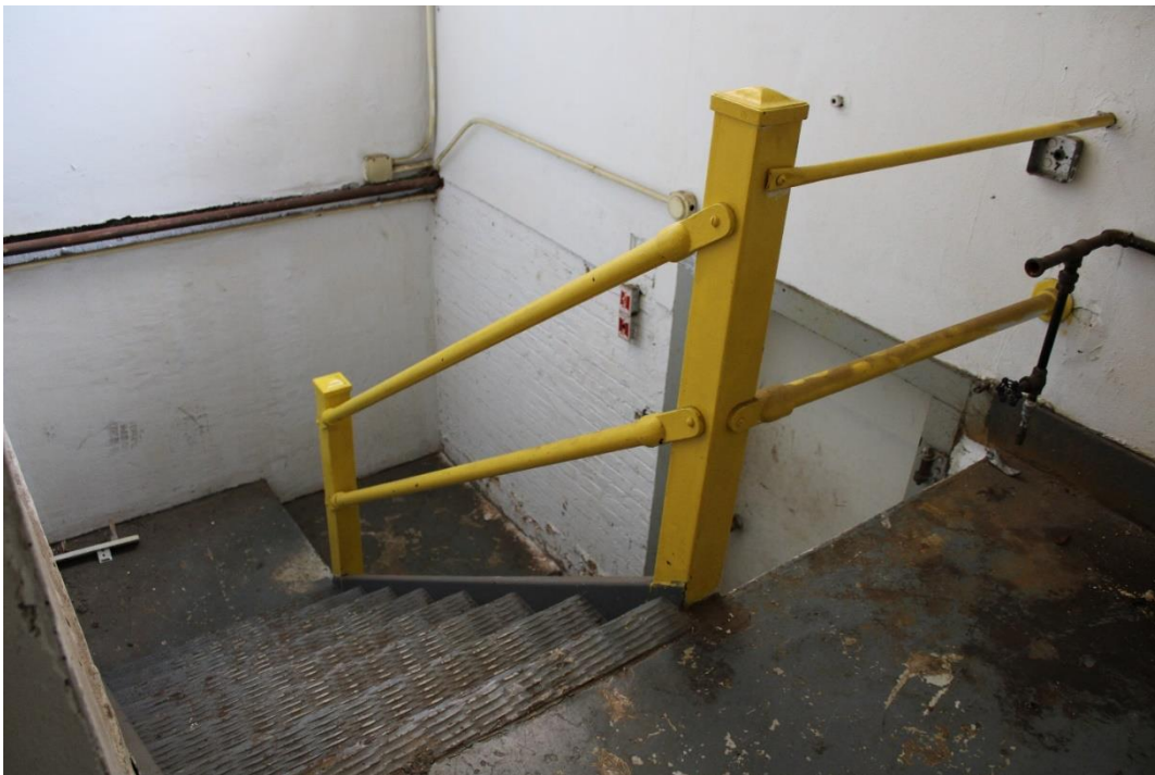
Figure 34: Staircase to basement boiler room.
