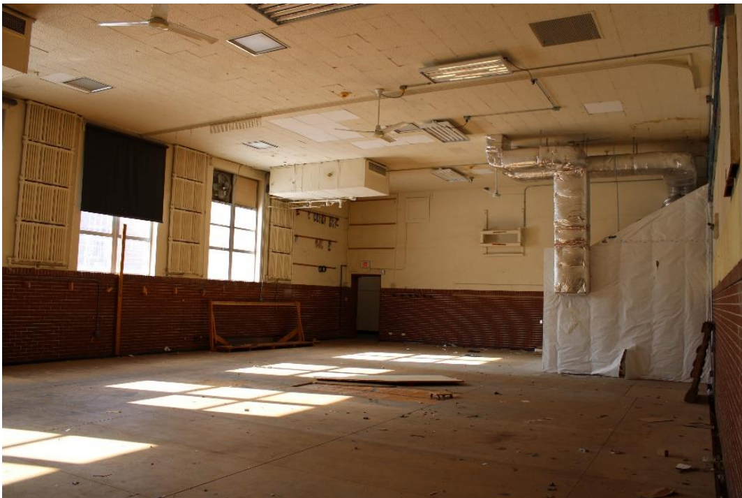
Figure 16: Gymnasium, looking southwest.
