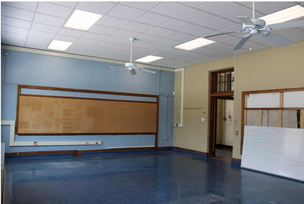
Figure 30: Classroom at the northwest corner of school, looking northeast.
