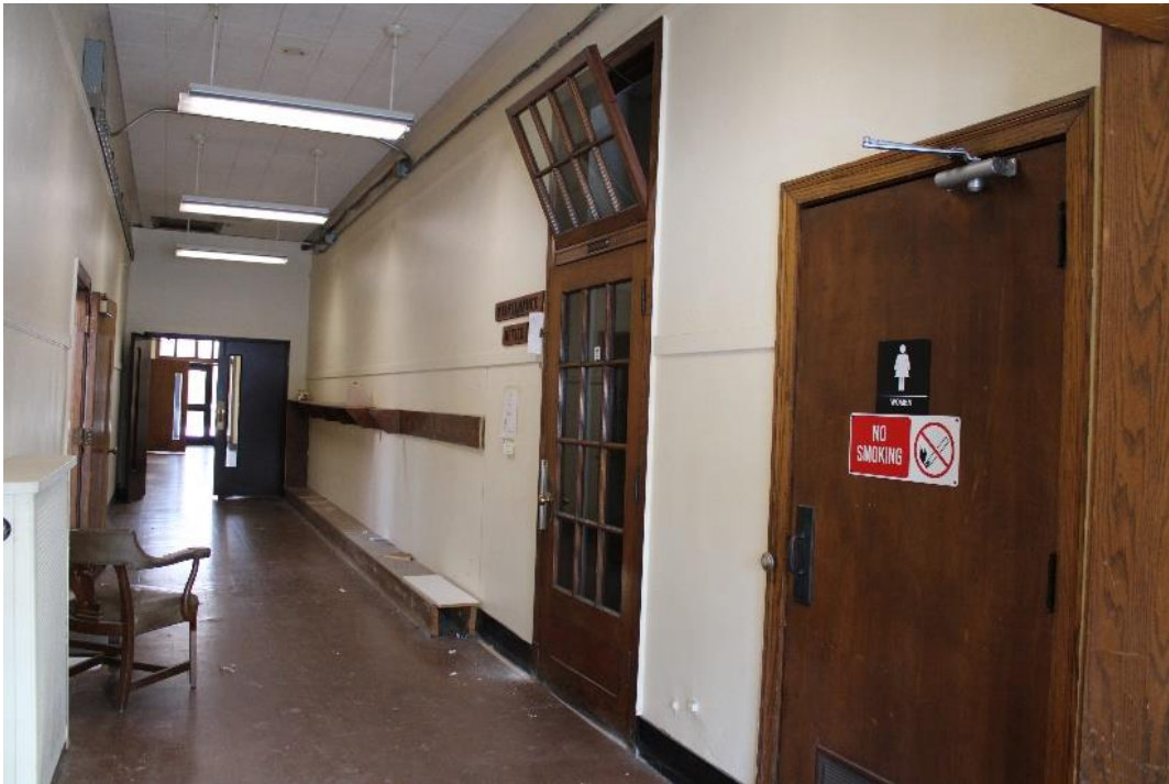
Figure 13: East corridor, looking northeast.
