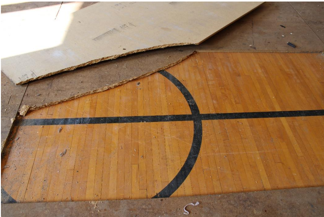
Figure 18: Original maple flooring in gymnasium.
