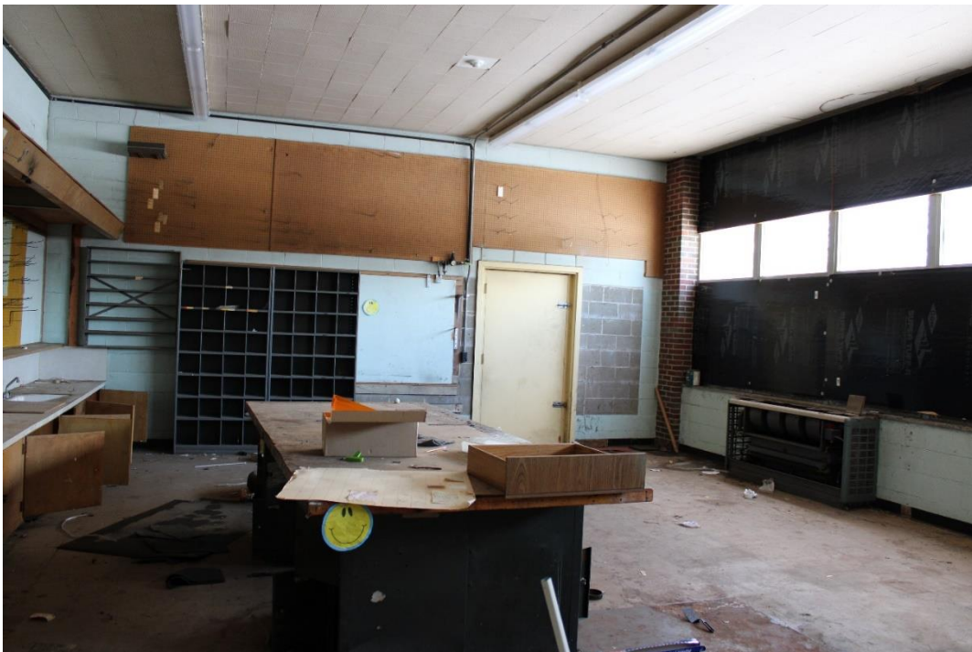
Figure 38: Workshop on the west side of the south addition.
