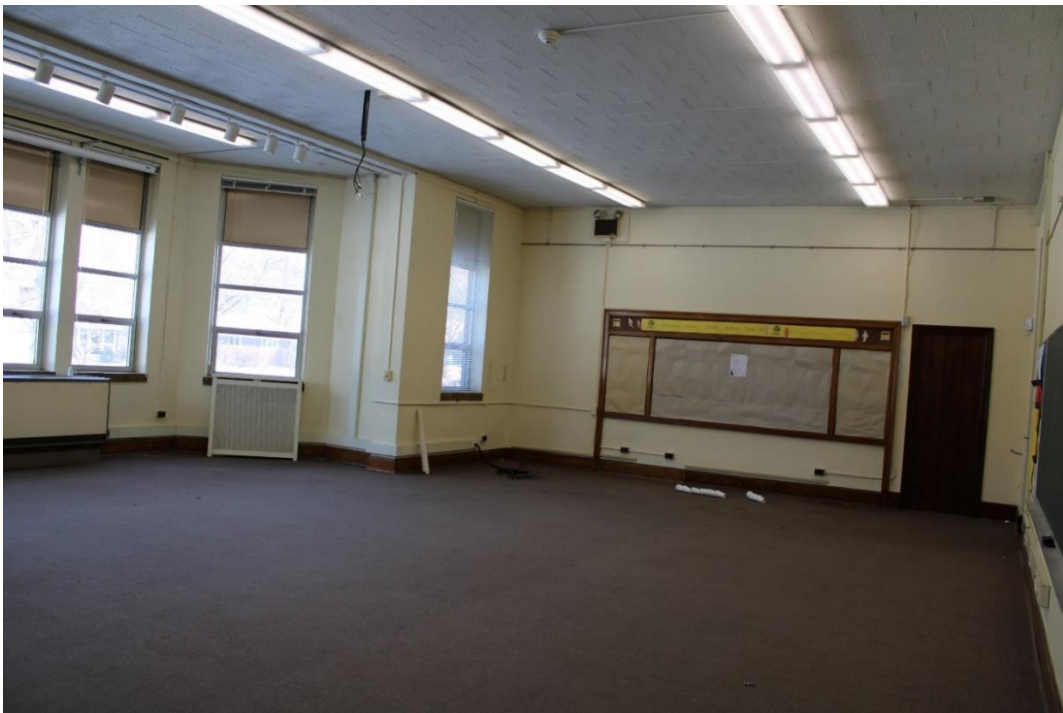
Figure 26: Kindergarten, looking northeast.
