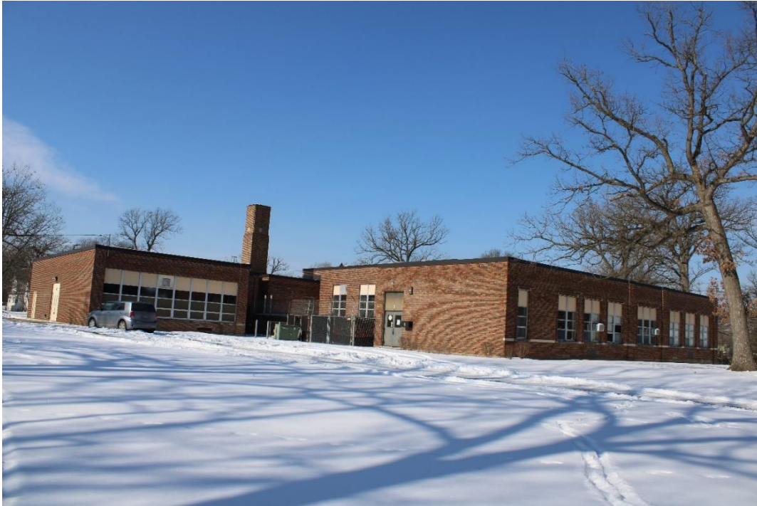
Figure 11: View looking northwest.
