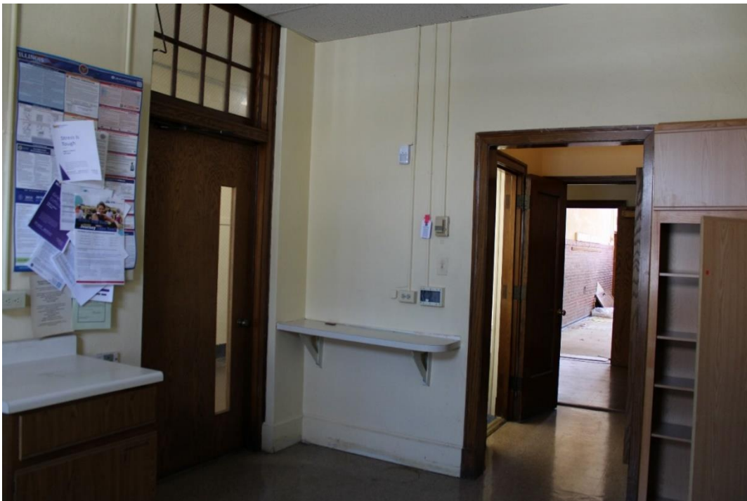
Figure 22: Nurse's room, looking southeast towards north corridor and gymnasium.
