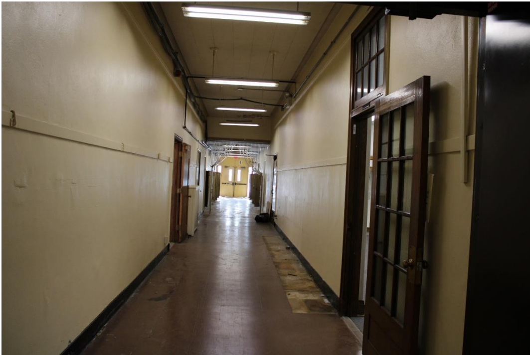
Figure 29: West corridor, looking south.
