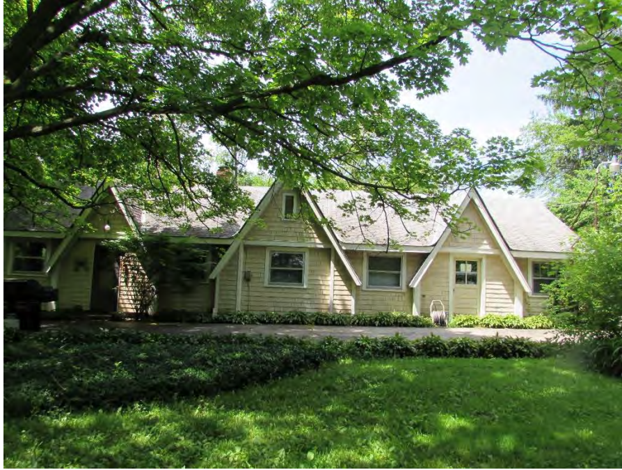
IL HABS No. DU-2016-1.19: Toolhouse, view looking west.
