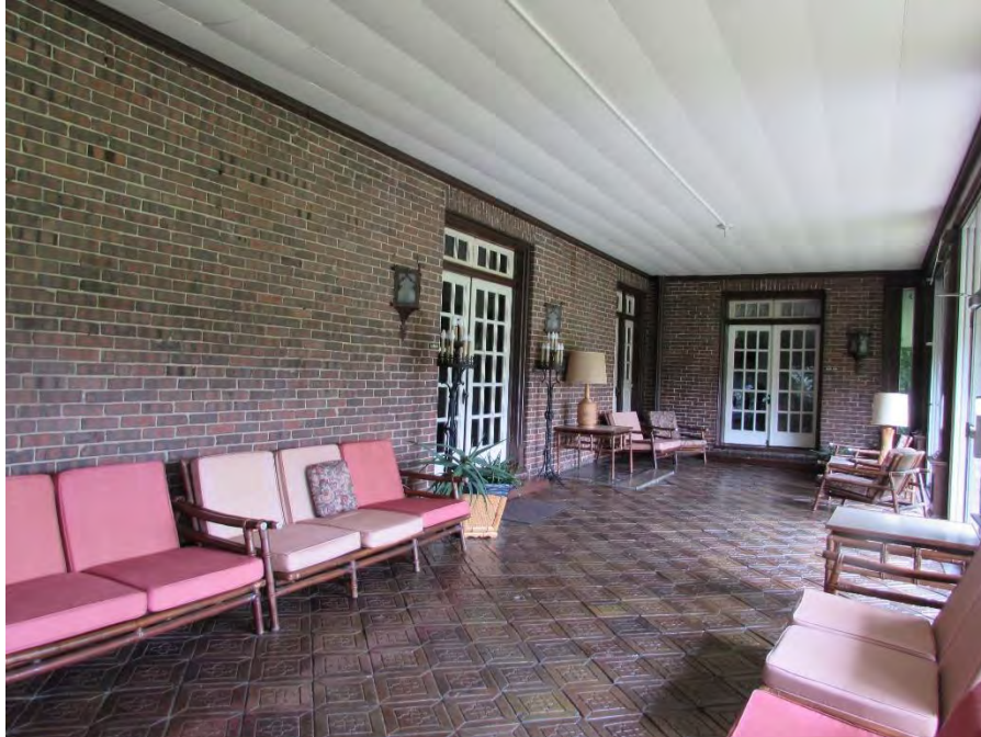
IL HABS No. DU-2016-1.15: House of Seven Gables, glass-enclosed porch along rear (south elevation).
