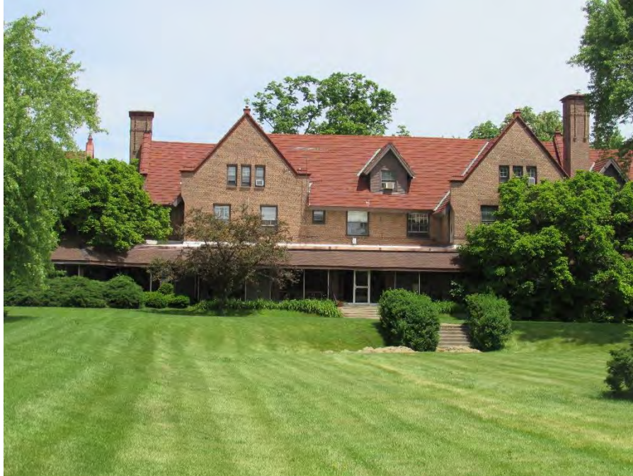
IL HABS No. DU-2016-1.5: House of Seven Gables, rear elevation, view looking north.
