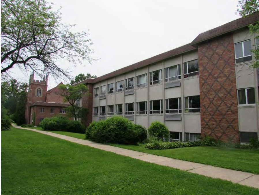
IL HABS No. DU-2016-1.27: North wing of Mary Ward House of Studies Building (foreground) with Loretto Chapel in distance, view looking southeast.
