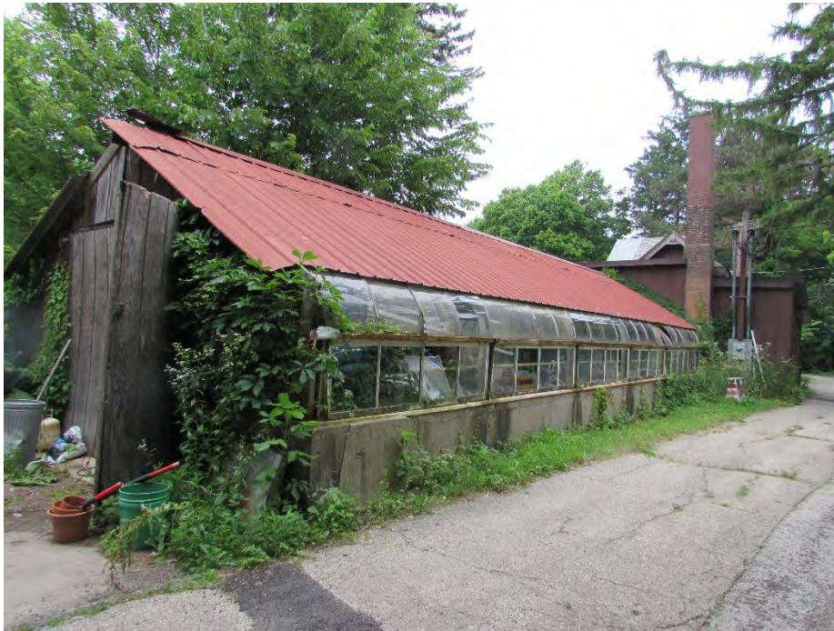
IL HABS No. DU-2016-1.20: Greenhouse, view looking northwest.
