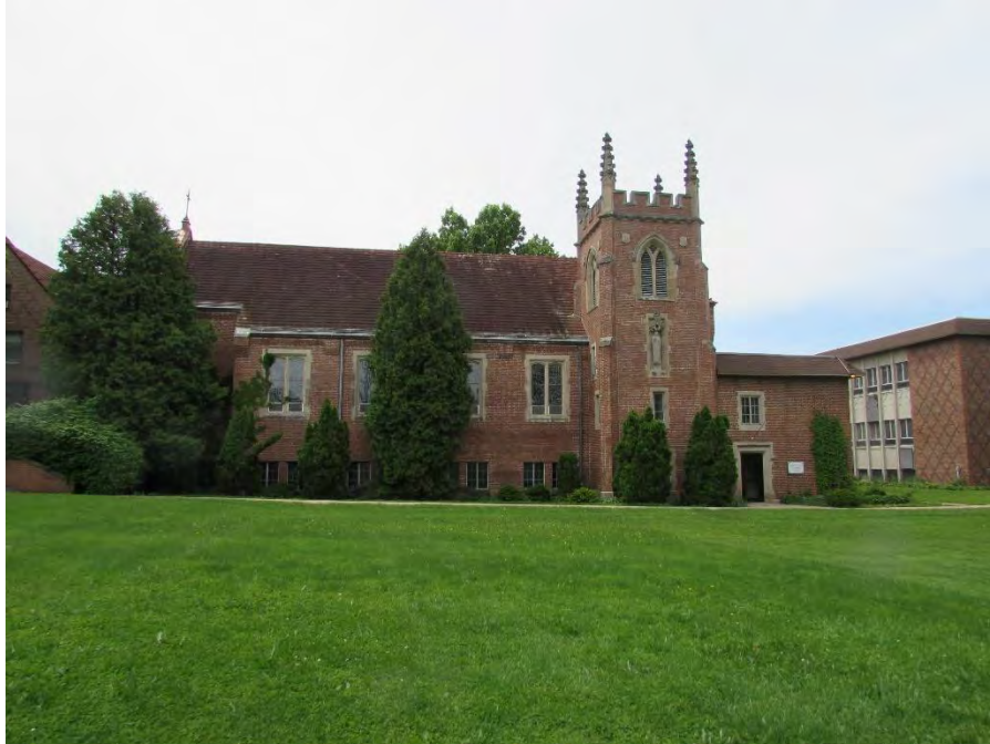
IL HABS No. DU-2016-1.23: Loretto Chapel and Mary Ward House of Studies (right), view looking southwest.
