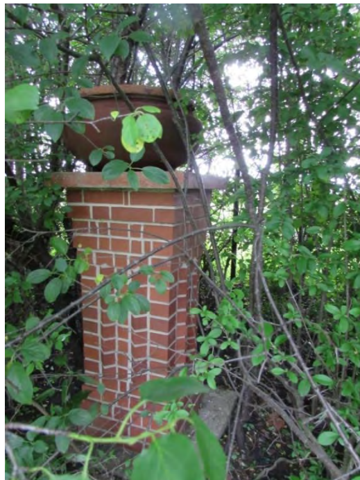
IL HABS No. DU-2016-1.34: One of two extant gateposts at north border of property that originally marked the entrance to Seven Gables Farm from a path that bisected the Chicago Golf Course.
