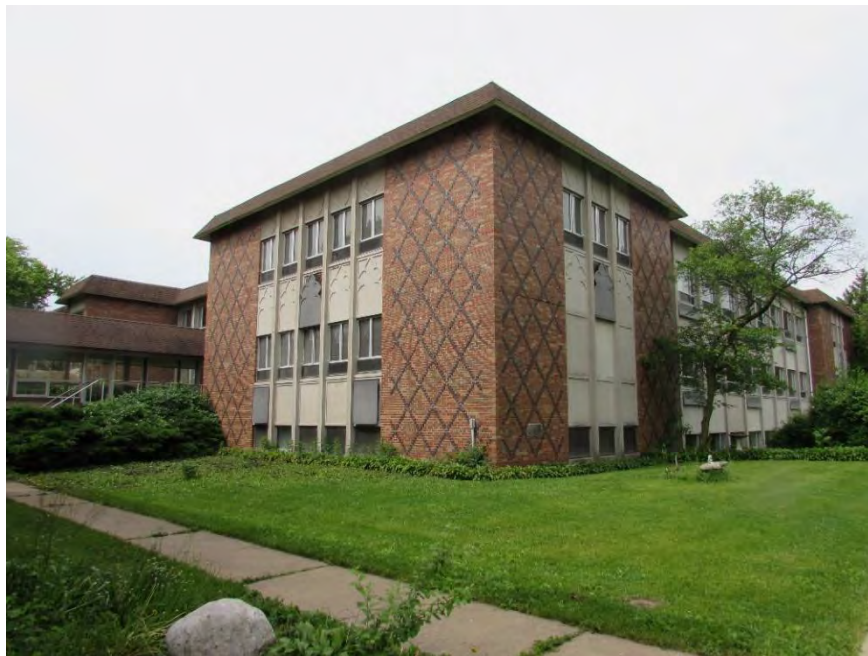
IL HABS No. DU-2016-1.28: Mary Ward House of Studies Building, north wing, view looking southwest.
