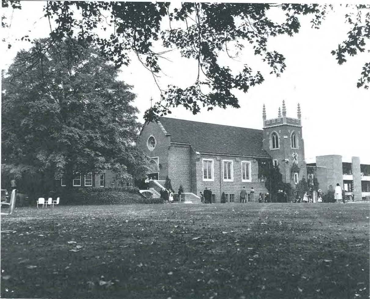
North elevation of Loretto Chapel and corner of Mary Ward House of Studies Building under construction, 1962. Source: Loretto Convent Archive, Wheaton, Illinois.
