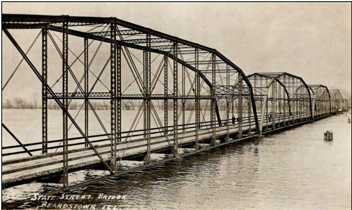
Figure 1: Pictured in this 1914 postcard is the 1898 bridge. Its first three spans were Pennsylvania Through-Trusses, which are the primary components pictured. The swing span is in the distant far right. The bridge's susceptibility to high water is apparent in this image ("State Street Bridge, Beardstown, Ill," Postmarked 10 September 1914, Copy of postcard in possession of ISAS, University of Illinois, Urbana, IL).
