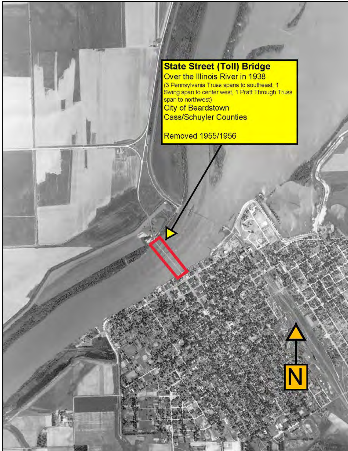
Figure 13: The bridge's agricultural and partially wooded vicinity is evident. Illinois Historic Aerial Photography: 1937-1947, Image SD-12-1009, 06 July 1938, Viewed at http://maps.isgs.illinois.edu/ilhap/ on 30 March 2025.
