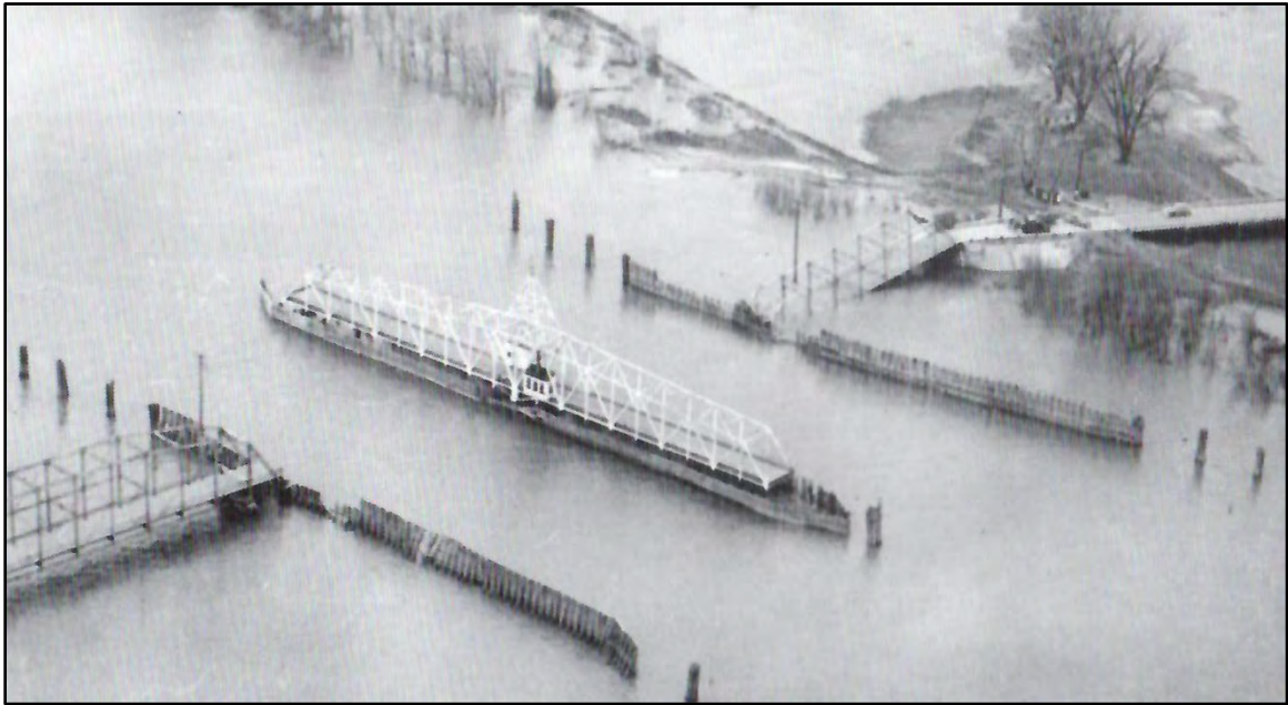
Figure 3: The work of the “Ferdinand” is illustrated in this image. Note that the left (south) end of the north span, seen in the upper right portion of the picture, is off its pier and in the water. The bridge was closed and a ferry carried traffic across the river for about three weeks. Ferries were often used when the bridge was closed for an extended period (Harold Tyson, Beardstown Revisited [Charleston, SC: Arcadia Publishing, 2018]: 99).
