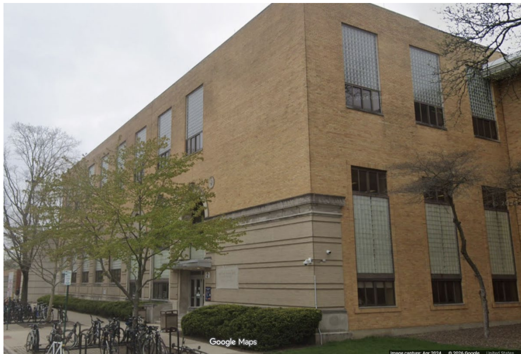
Photograph 4: Girls' Gymnasium Building, view southwest. Source: Google Maps.
