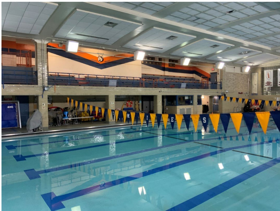
Photograph 12: Girls' pool, view southeast toward balcony along its east wall.
