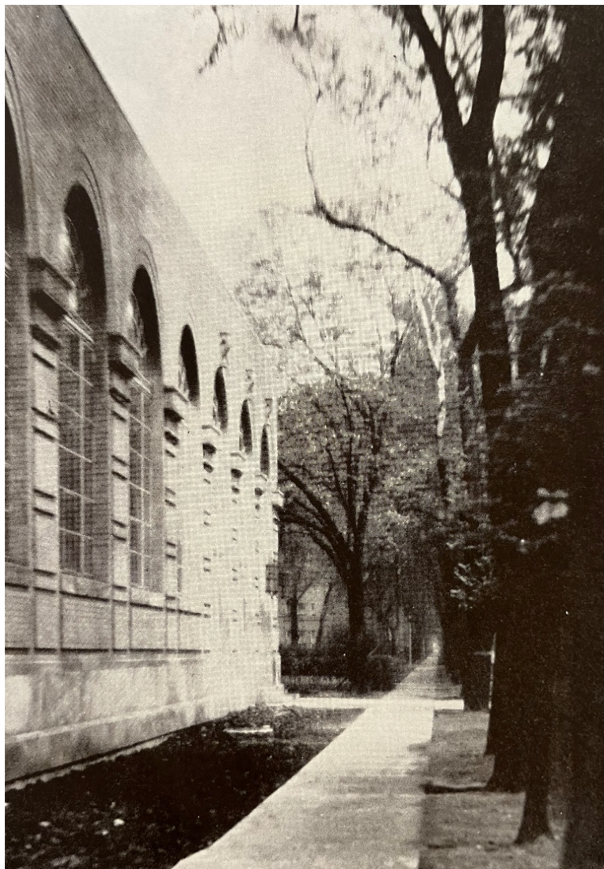
Figure 7: Scoville Avenue façade of the Girls' Gymnasium Building, view north, 1929. Source: Tabula . Oak Park and River Forest High School, 1929.
