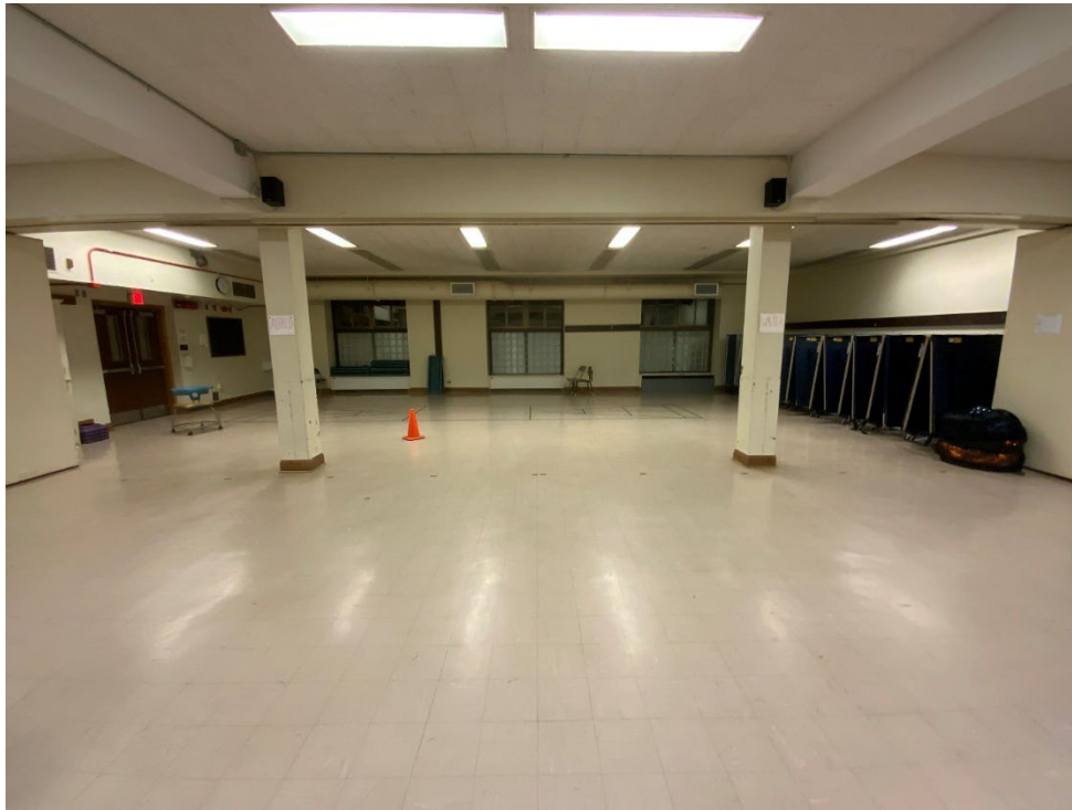
Photograph 20: Second floor gymnasium in the northeast corner of the building, view north.
