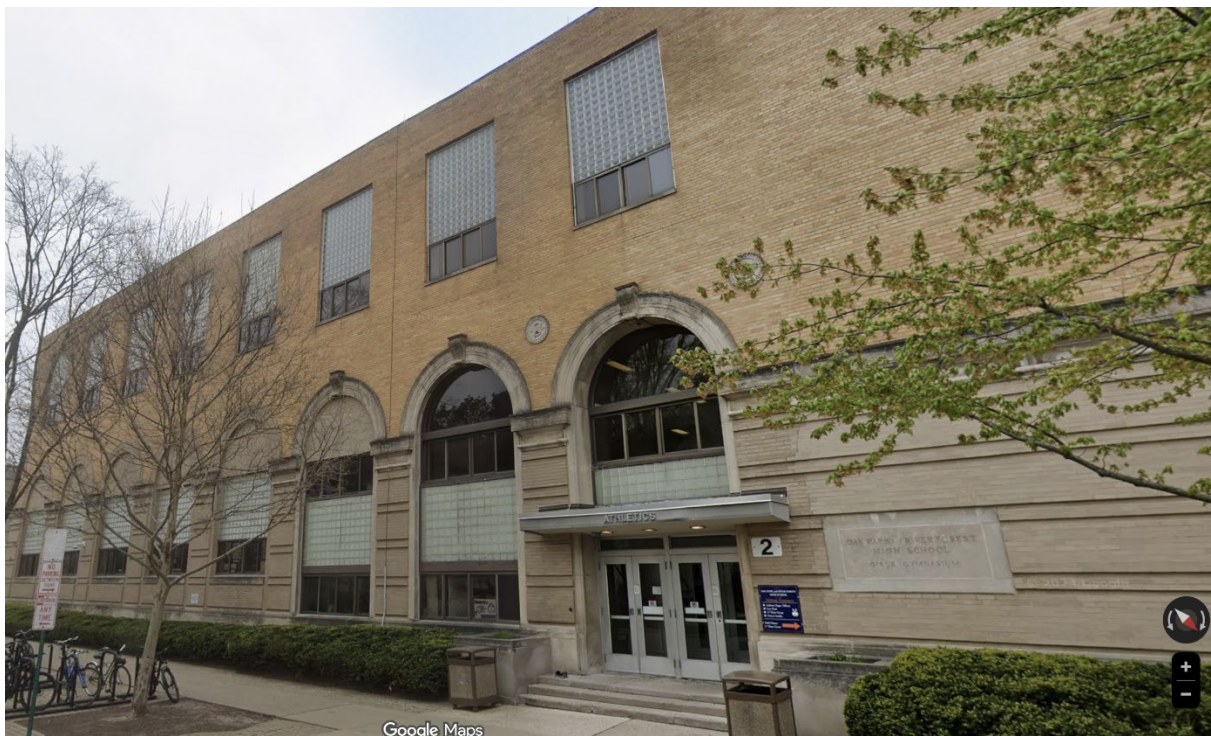
Photograph 2: Girls' Gymnasium Building, view southwest. Source: Google Maps.
