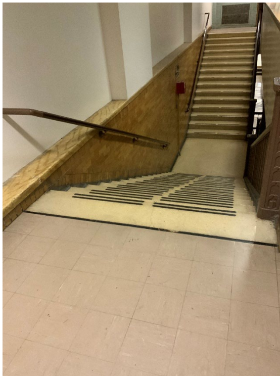
Photograph 21: Stairways to third floor.
