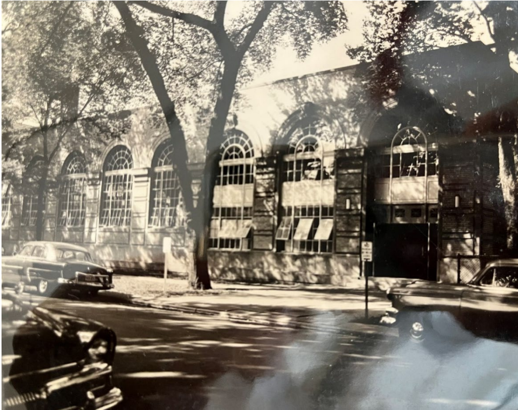
Figure 15: Scoville Avenue façade of Girls' Gymnasium Building. Source: "Pictures and Facts: Oak Park and River Forest High School, November 1957."
