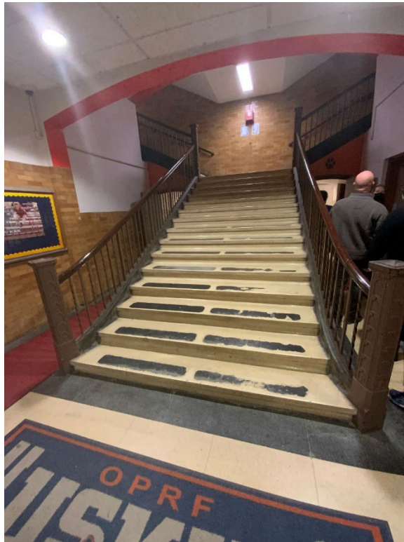
Photograph 7: Main Staircase in the Entrance Hall.
