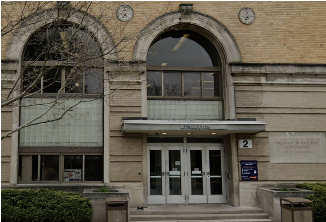
Photograph 3: Scoville Avenue entrance to Girls' Gymnasium Building, view west. Source: Google Maps.
