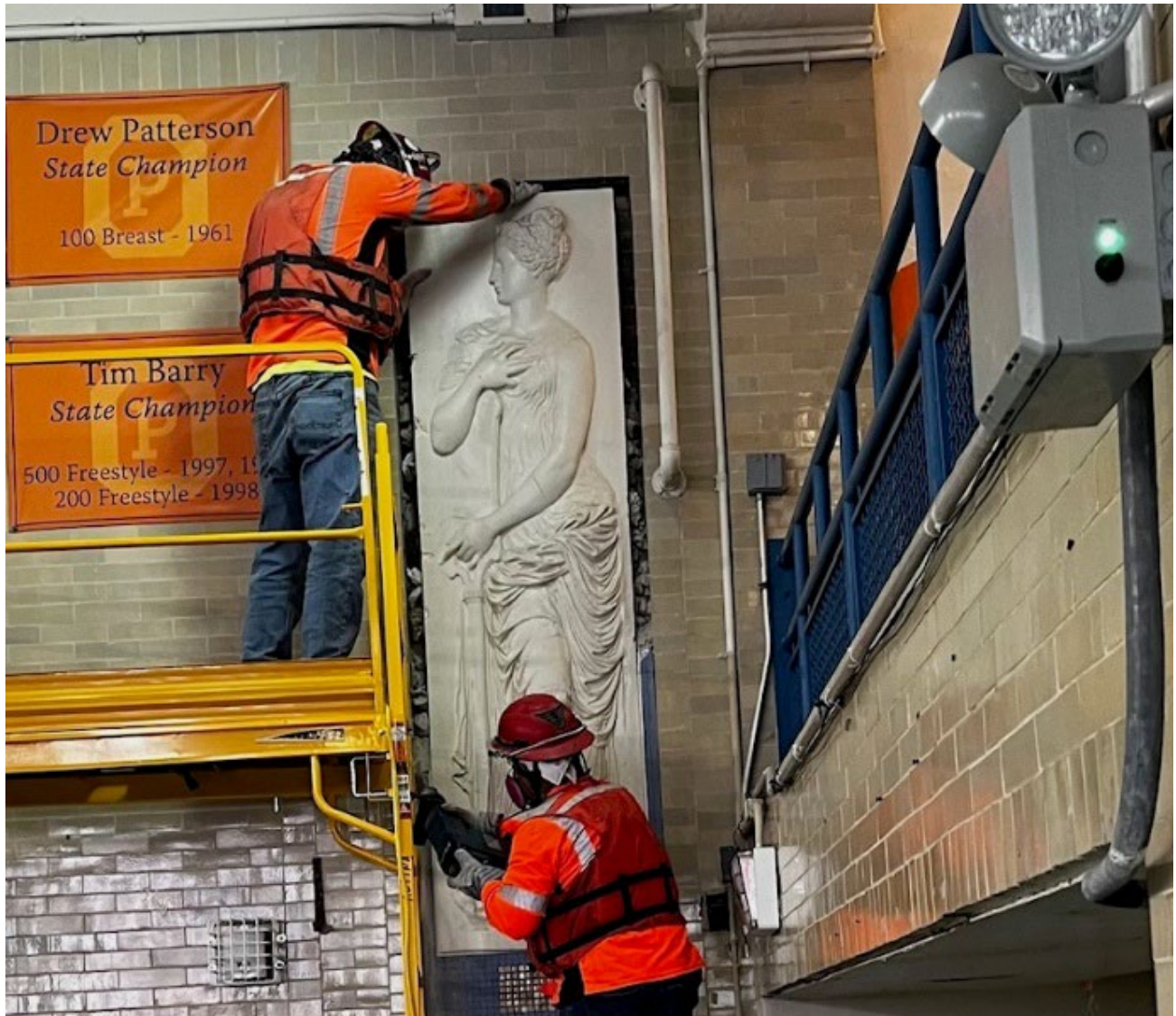
Photograph 15: Removal of bas-relief panel on the wall of the Girls' pool room, prior to the demolition of the Girls' Gymnasium Building.
