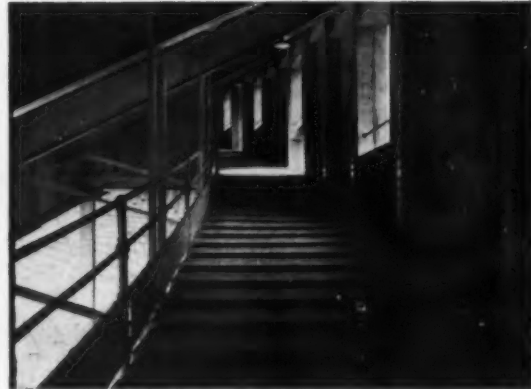
FLOOR OF PASSAGE UNDER SECOND DECK FORMS A RAMP WITH STAIRWAYS AT ENDS WHERE THE SLOPE IS STEEPER. STEPS ARE ABOUT 4" X 22"
