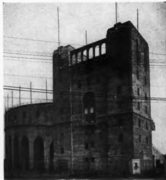
RAMP TOWER OF THE DYCHE STADIUM
