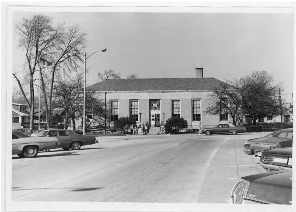
View of former Des Plaines Post Office building from Ellinwood Avenue, 1974, view from east. Note that the cupola above the main entrance is no longer extant. Source: Des Plaines History Center, object number P494.
