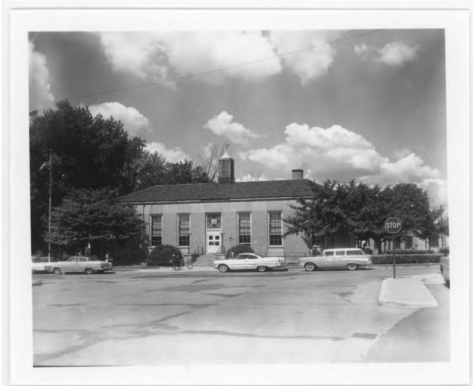
Postcard of Des Plaines Post Office building, 1960, view from east. Note the cupola at the roof over the main entrance. Source: Des Plaines History Center, object number P3858.
