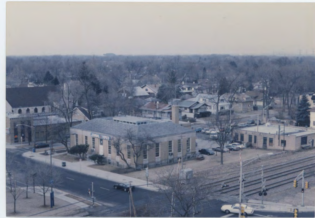
Aerial view of former Des Plaines Post Office building, circa 1996. Note the clerestory is visible at the center of the building. Source: Des Plaines History Center, object number 1996-40-38.
