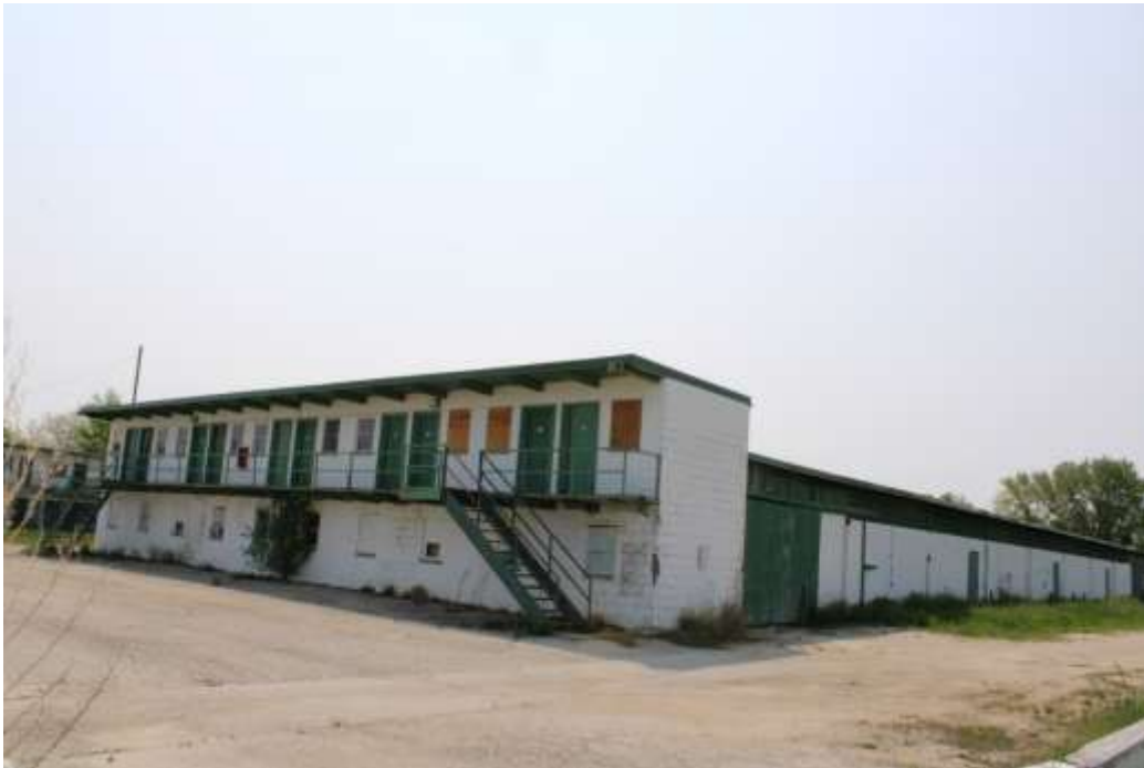
Photograph 47: Stable no. 8 with concrete block walls and dormitory rooms on either end.
