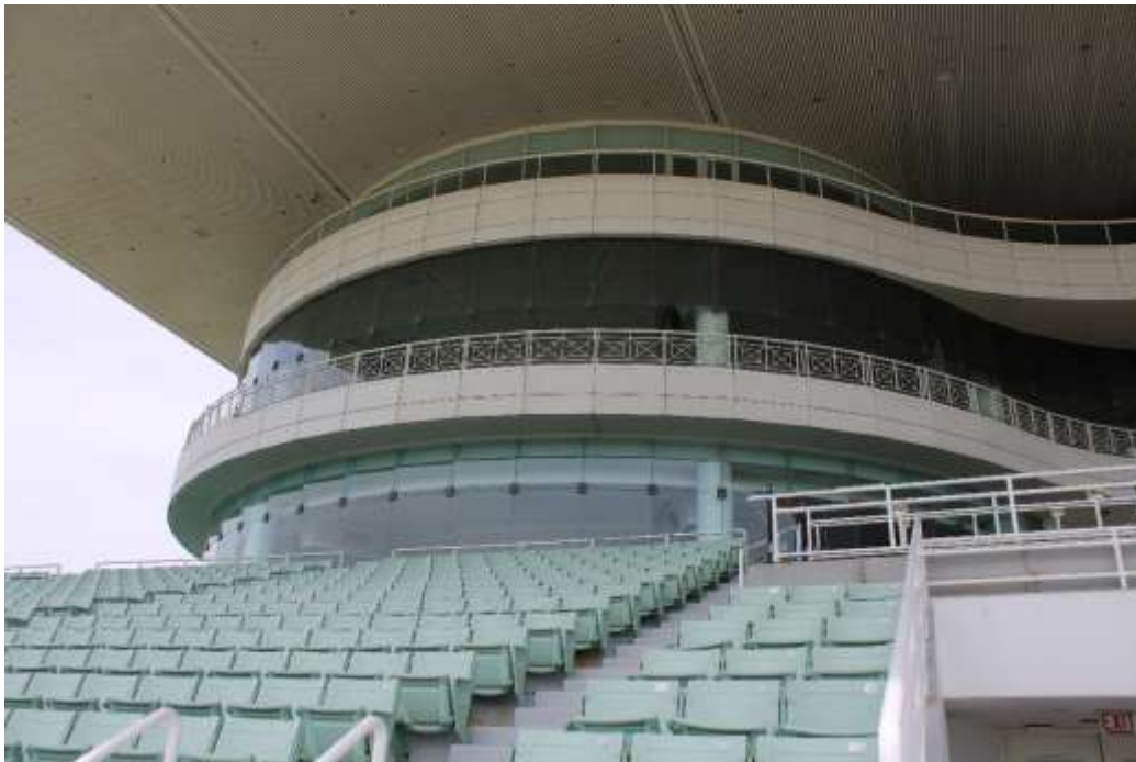
Photograph 4: Detail of grandstand elevation facing racetrack, view north.
