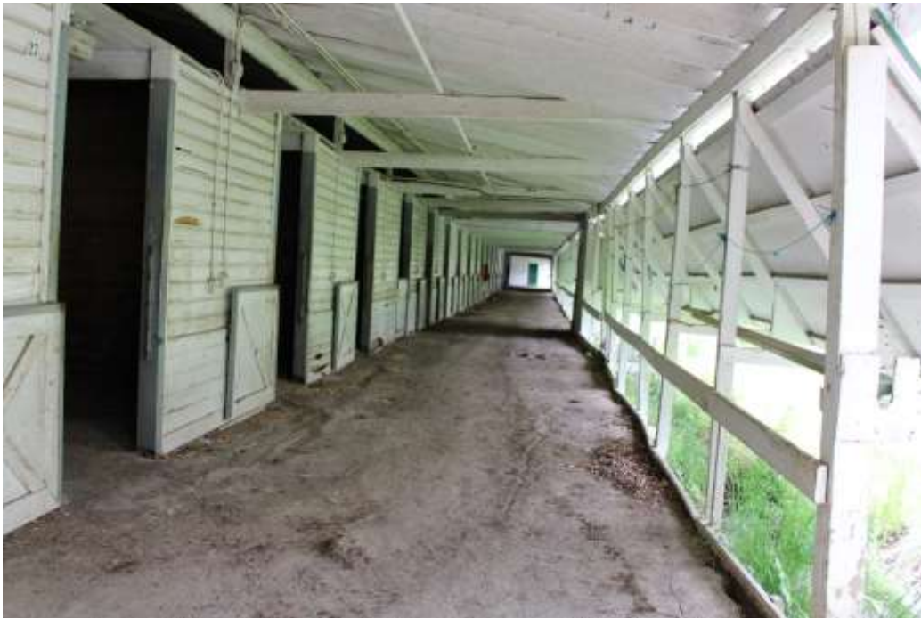
Photograph 45: Typical wood stable with single-loaded aisle.
