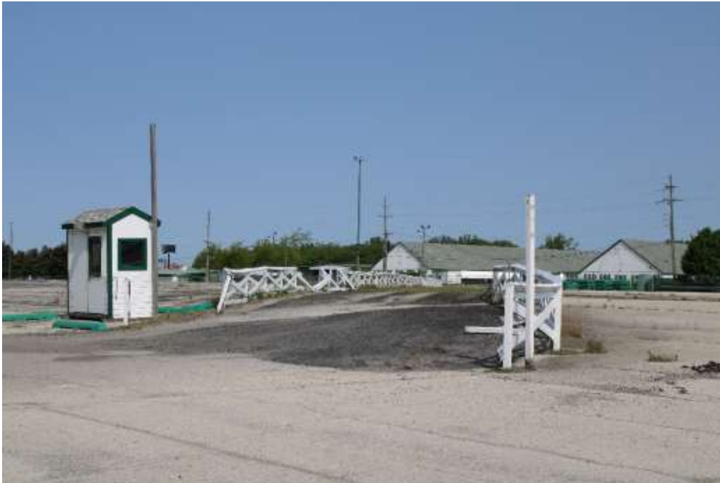
Photograph 39: Path from the paddock area to the backstretch.
