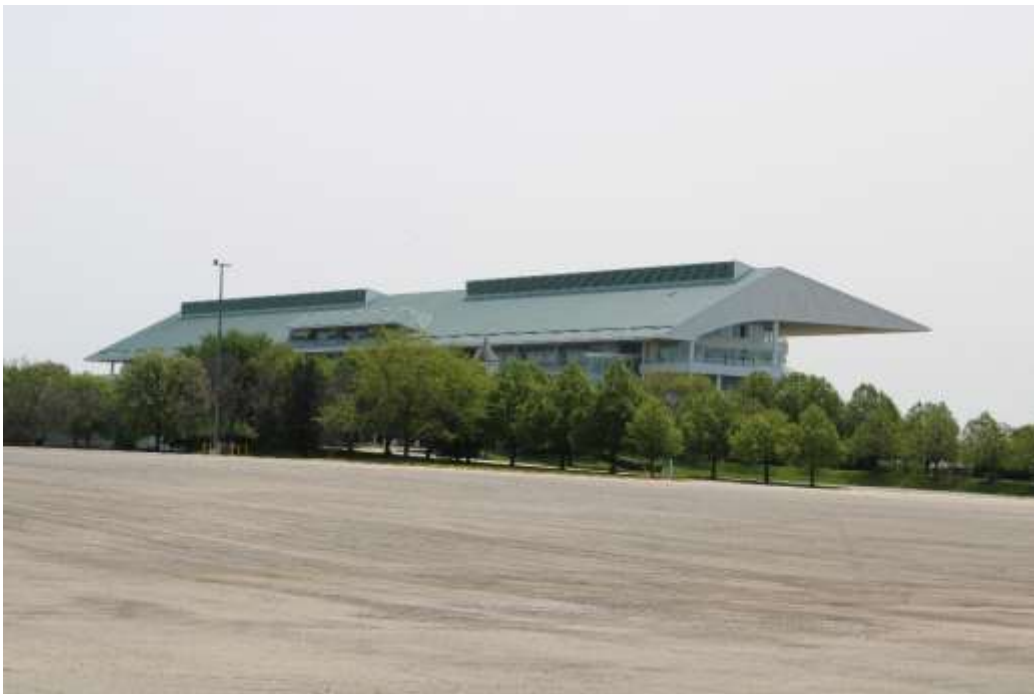
Photograph 12: Rear elevation of the grandstand, view southeast.
