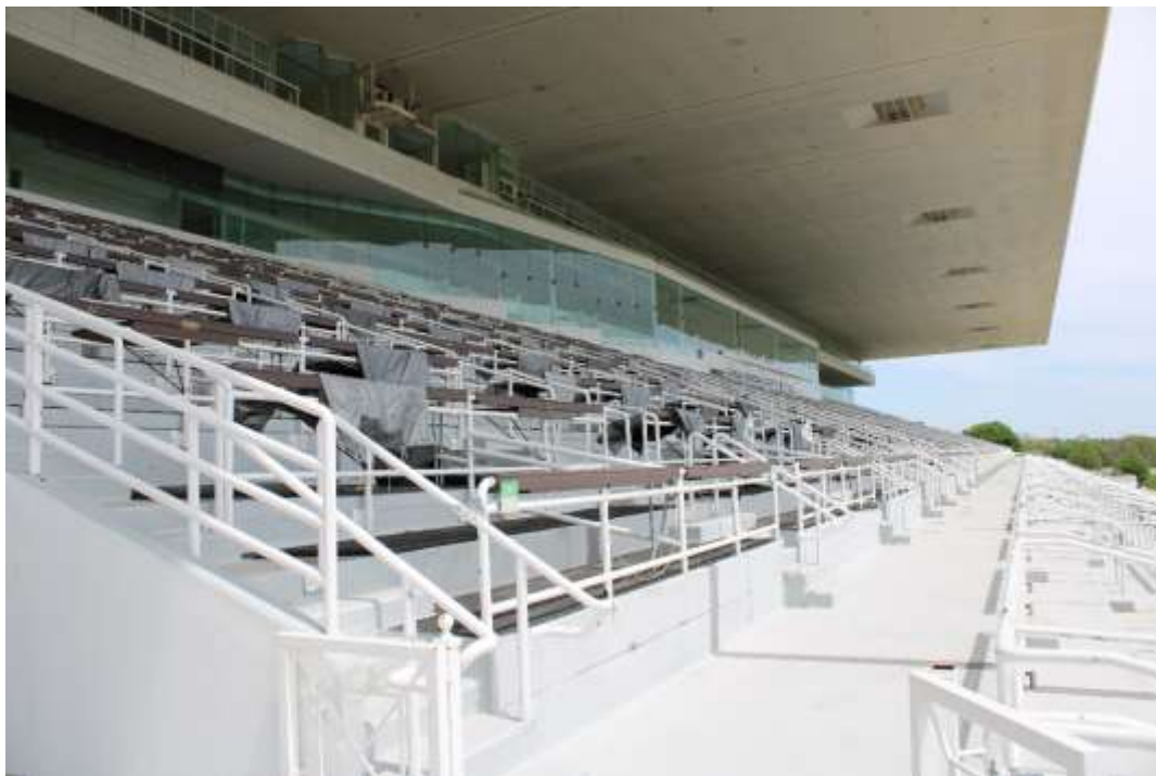
Photograph 6: Grandstand bleacher seating and cantilevered roof, view east.
