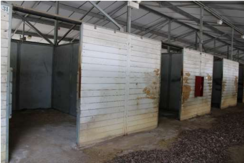
Photograph 62: Entrances to stalls within a typical stable with modular metal construction.
