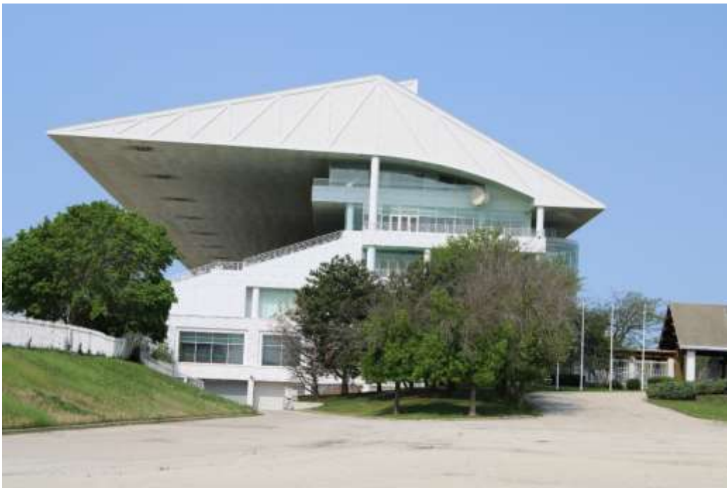
Photograph 10: East elevation of the grandstand showing cantilevered roof, view west.
