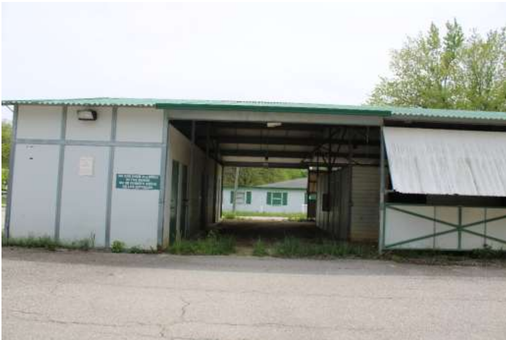
Photograph 60: Entrance to typical stable built with modular metal construction.
