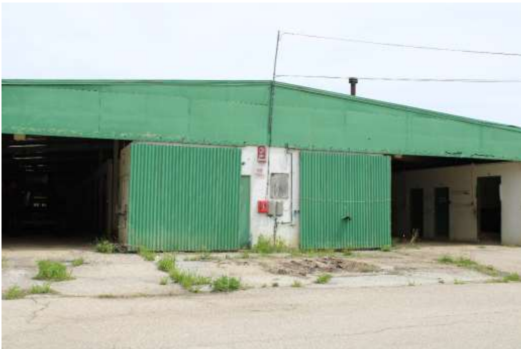
Photograph 54: Entrances to typical stable with precast concrete wall panels and two double-loaded aisles opening onto stalls.
