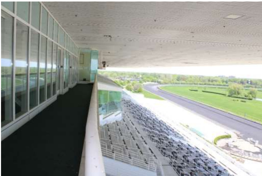
Photograph 8: Bleacher seating and racetrack as seen from the skybox level balcony, sheltered by cantilevered roof, view east.
