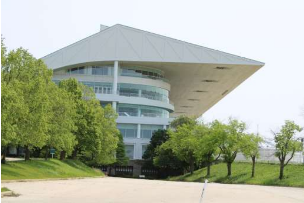
Photograph 11: West elevation of the grandstand showing cantilevered roof, view east.
