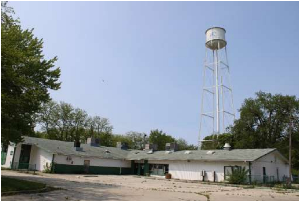
Photograph 74: Auditorium/Kitchen Building for backstretch workers.
