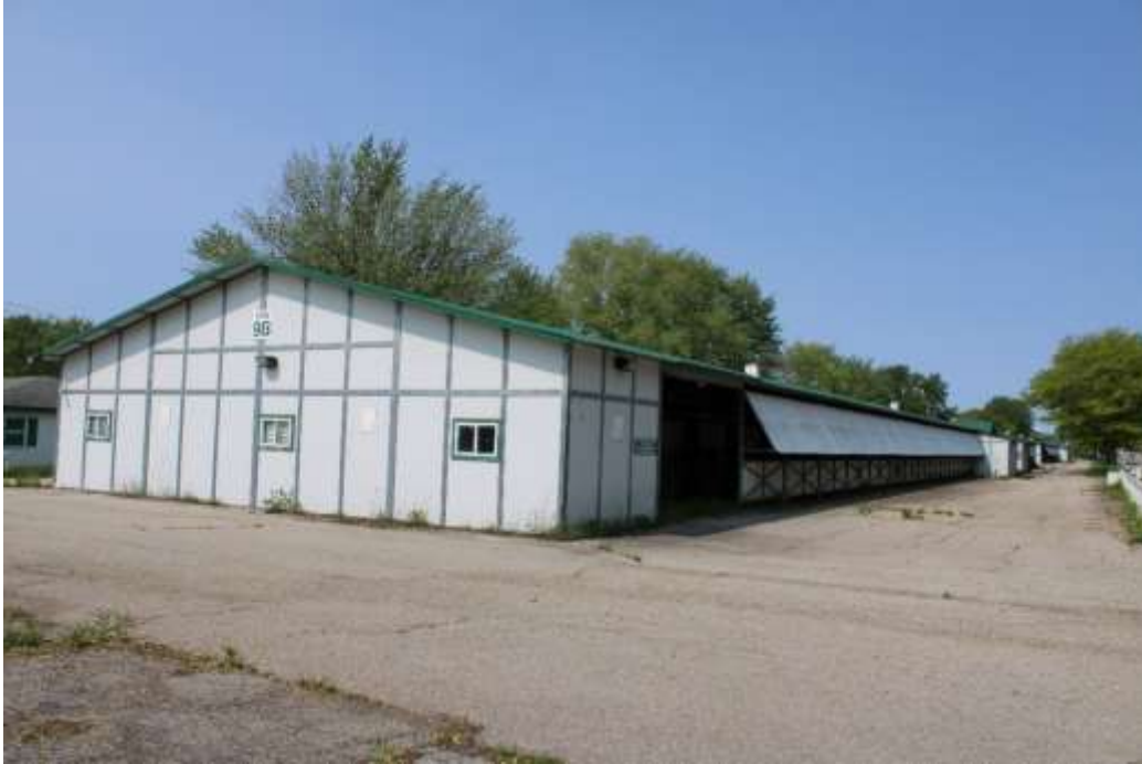
Photograph 59: Typical stable built with modular metal construction.
