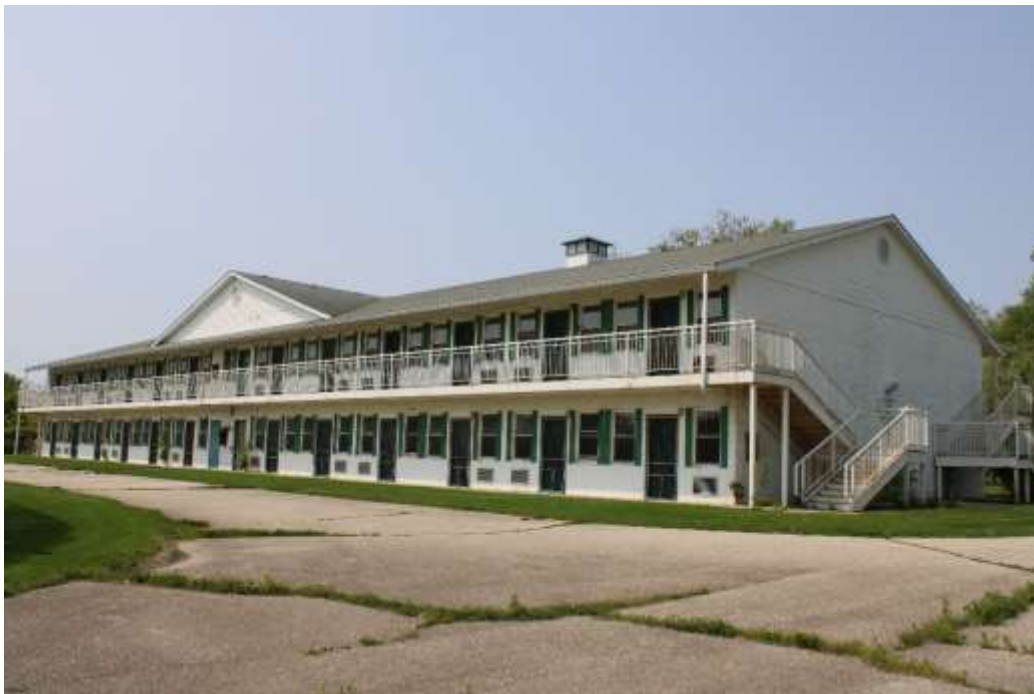
Photograph 70: One of three dormitories with concrete block walls built post-2000 with private bathrooms in each room.
