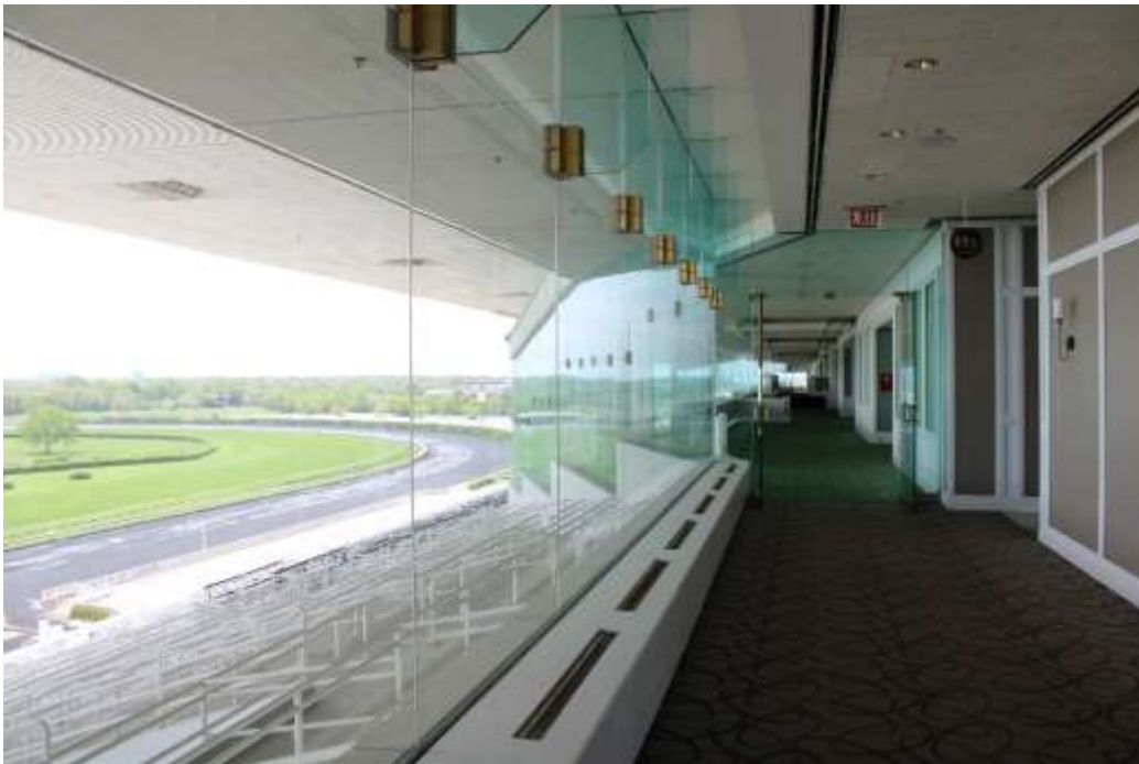
Photograph 30: Grandstand window wall overlooking the racetrack.
