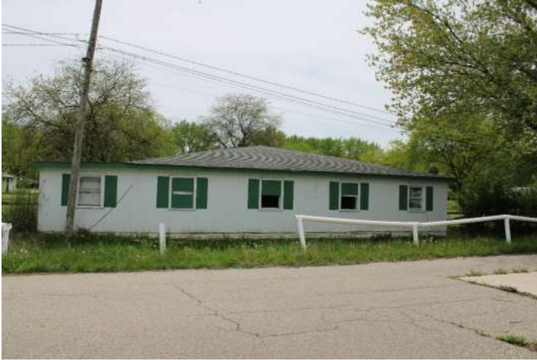
Photograph 41: Typical wood stable showing windows on short end illuminating the tack rooms.
