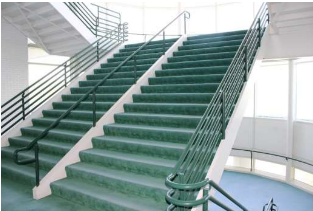
Photograph 24: Typical staircase in one of the grandstand's four semicircular stairwells.
