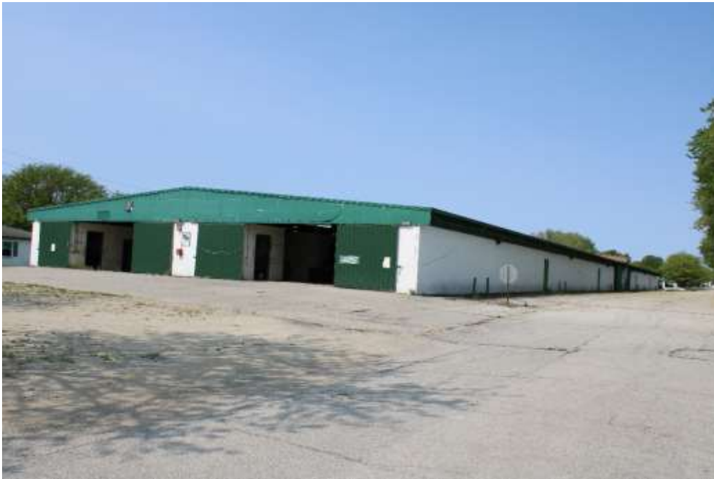
Photograph 53: Typical stable with precast concrete wall panels.
