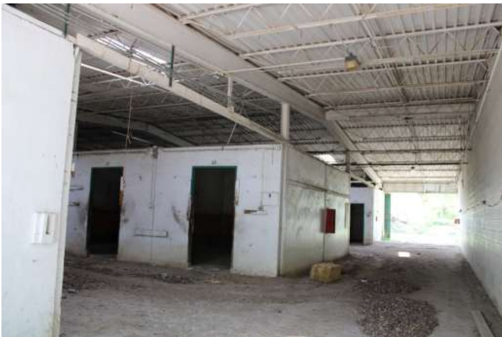
Photograph 56: Typical stable with precast concrete wall panels showing metal truss roof.
