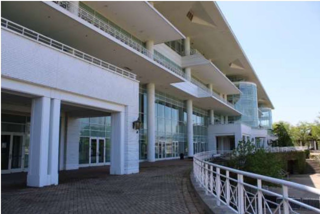
Photograph 15: Grandstand's main entrance from paddock, view southwest.
