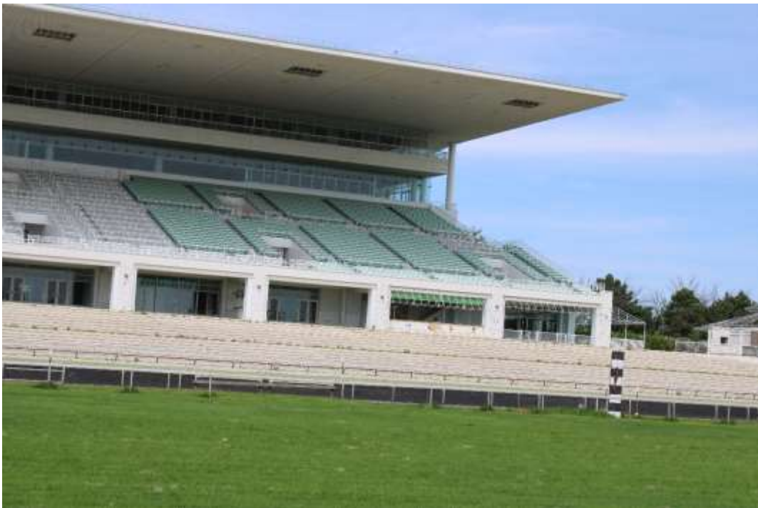
Photograph 2: Grandstand elevation facing racetrack, view northeast.
