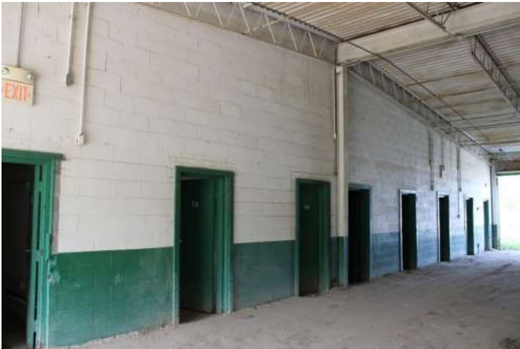
Photograph 50: Tack rooms in stable no. 8.
