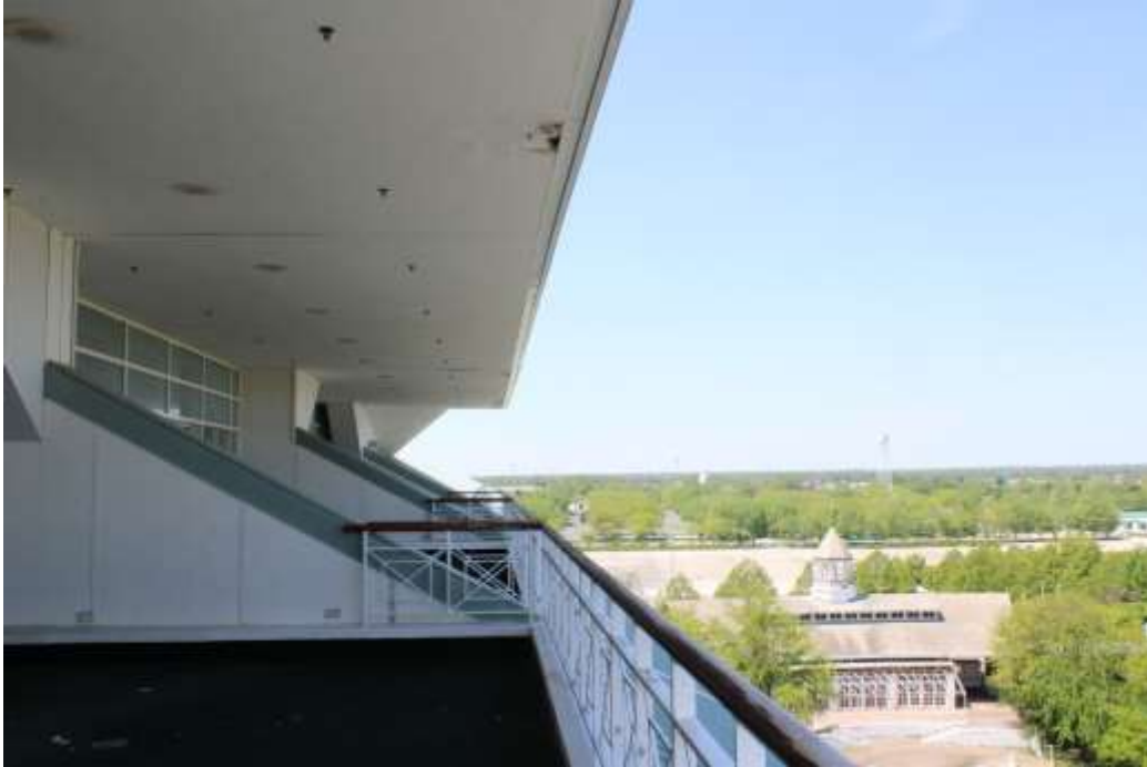
Photograph 37: Grandstand balcony overlooking the paddock.
