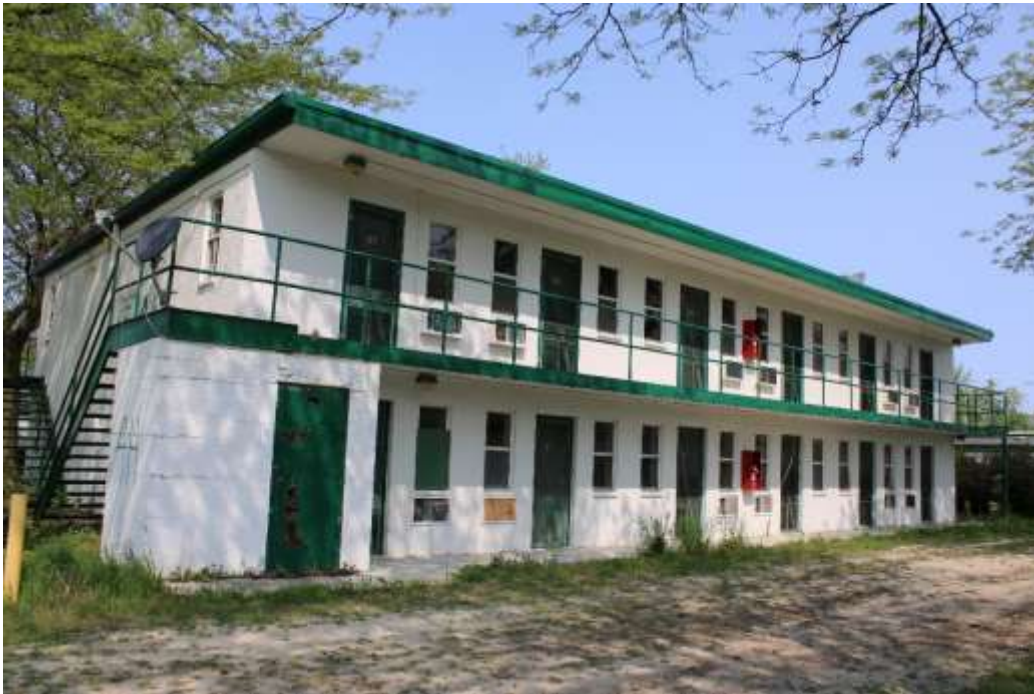
Photograph 65: One of the five concrete block, motel-style dormitories with private bathrooms that were built c. 1985.
