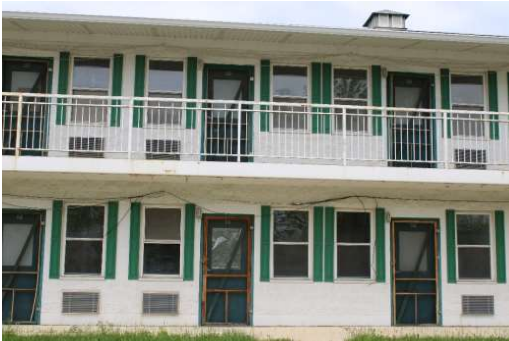
Photograph 71: Detail of a dormitory with concrete block walls built post-2000.
