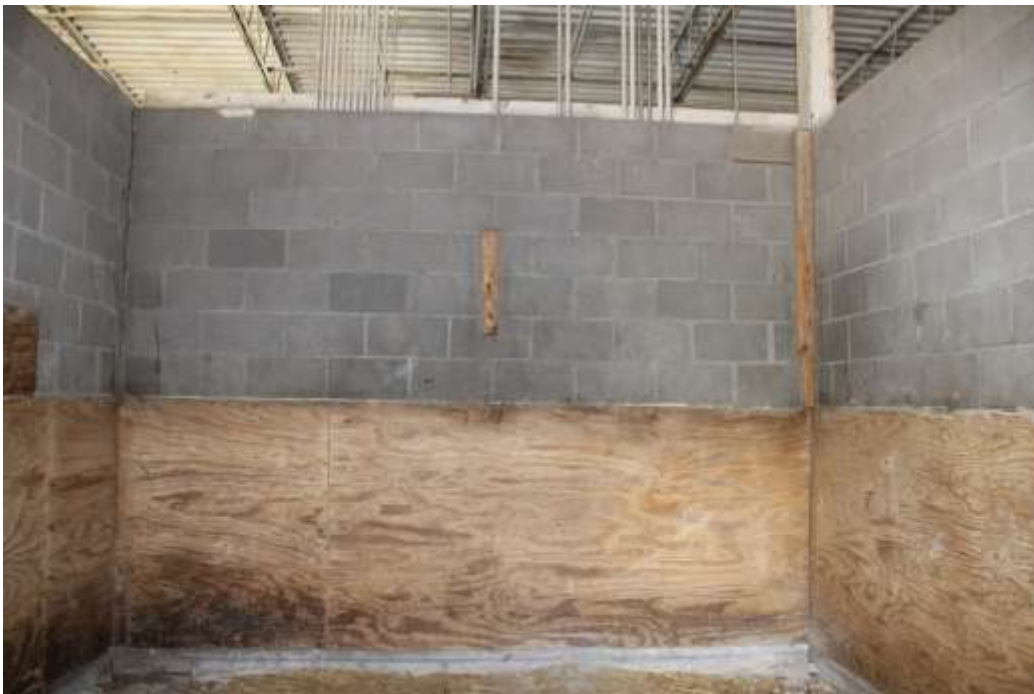
Photograph 52: Stall with concrete block walls in stable no. 8.
