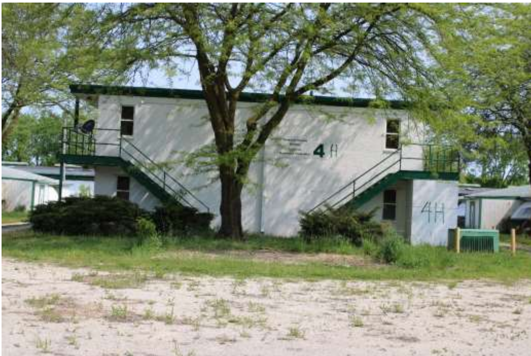
Photograph 66: One of the concrete block, motel-style dormitories that were built c. 1985 showing metal stairways to balconies.
