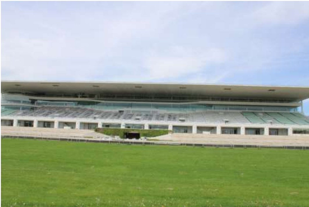
Photograph 1: Grandstand elevation facing racetrack, view north.
