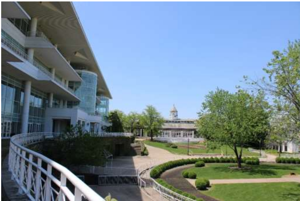
Photograph 16: Paddock with grandstand on the left, looking toward one of the twin entrance gates with cupola, view west.
