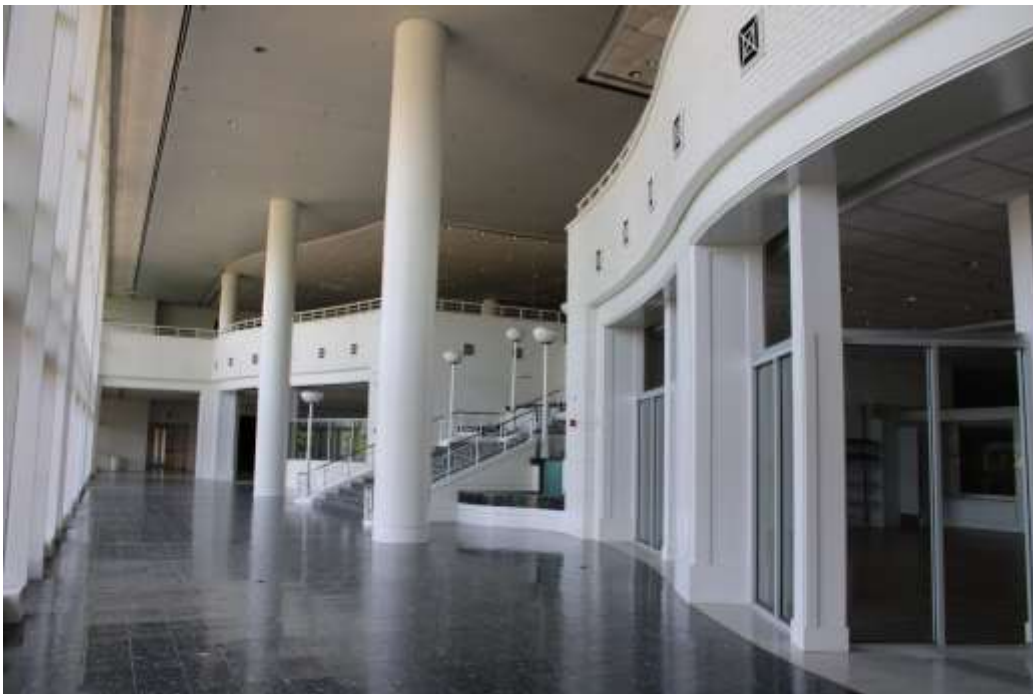
Photograph 18: Apron level of the grandstand looking toward the main entrance staircase on the right.
