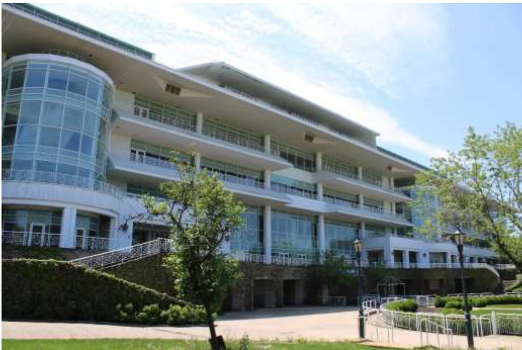
Photograph 14: Grandstand and paddock area, view southwest.
