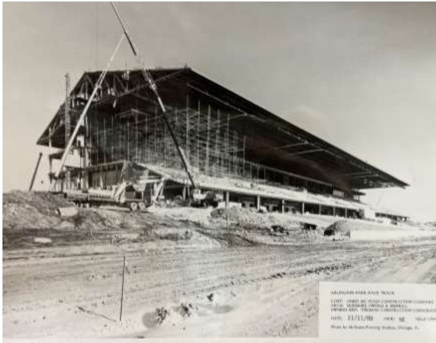
Figure 52: Arlington Park grandstand under construction, November 11, 1988, view northeast. McShane-Fleming Studios, photographer. Source: Arlington Heights Historical Museum.
