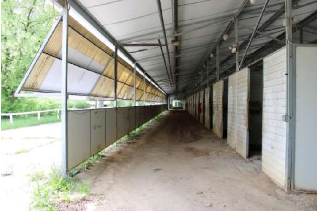
Photograph 61: Single-loaded aisle in typical stable with modular metal construction.
