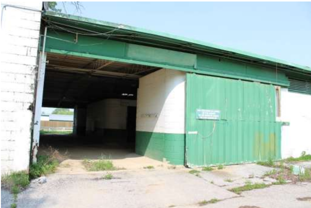
Photograph 48: Entrance to stable no. 8 with concrete block walls.
