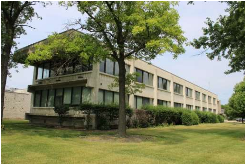
Photograph 16: South wing, view northeast.
