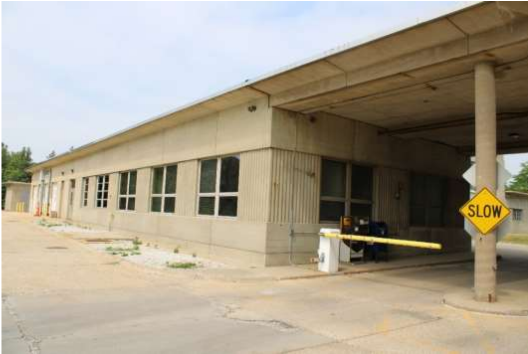
Photograph 15: West façade, view northeast.
