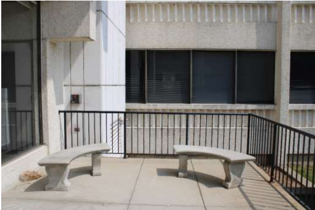
Photograph 3: Detail of entrance terrace with concrete benches, view north.
