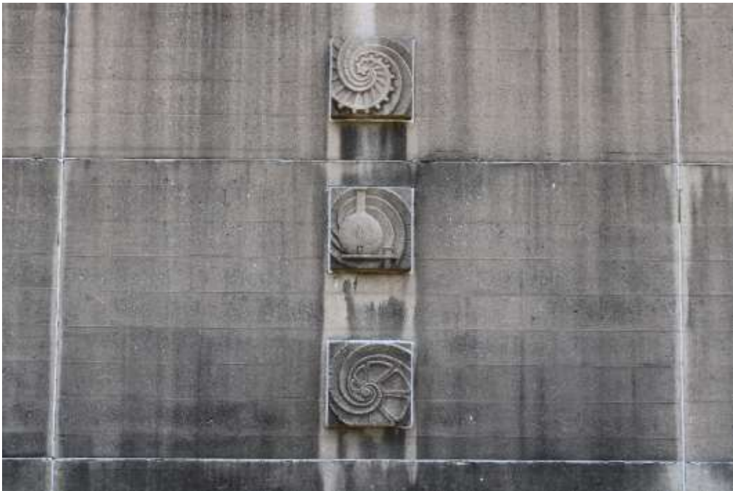
Photograph 10: Decorative concrete inserts on west façade.
