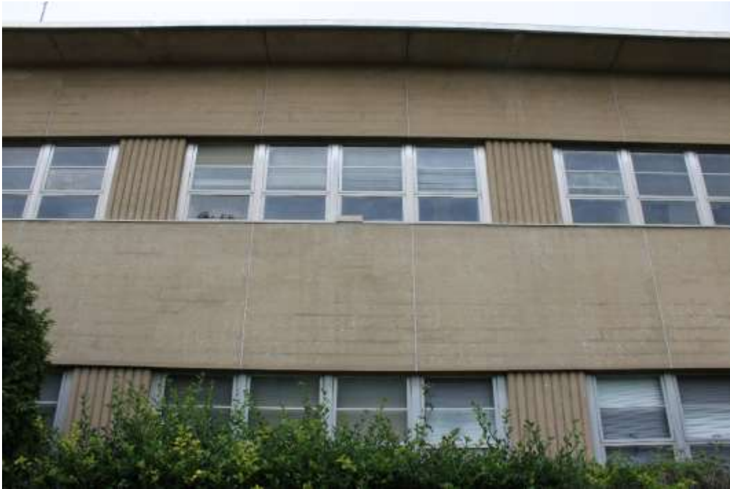
Photograph 31: Detail of precast concrete panels on front façade, view north.
