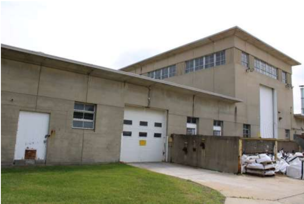
Photograph 9: North façade, view southwest.
