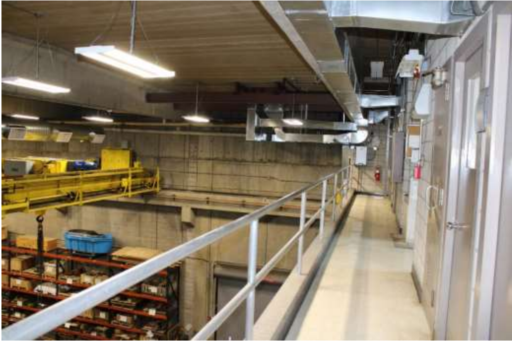
Photograph 21: Third floor balcony spanning east end of laboratory, view north.
