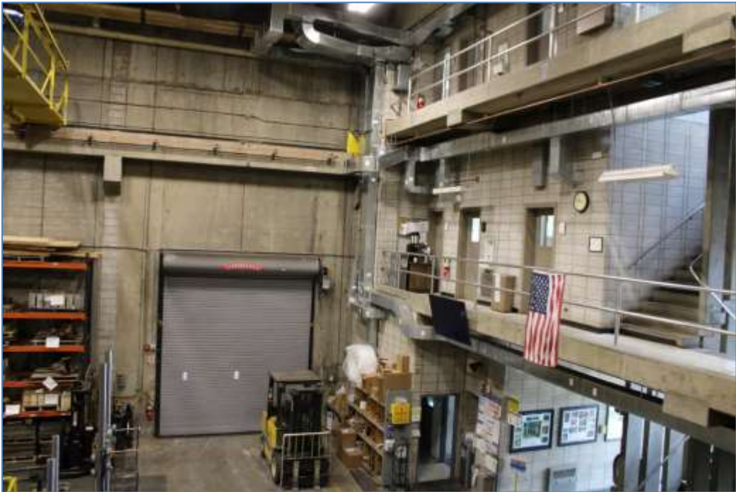
Photograph 26: Laboratory, view north toward steel roll-up door with balconies on the right.
