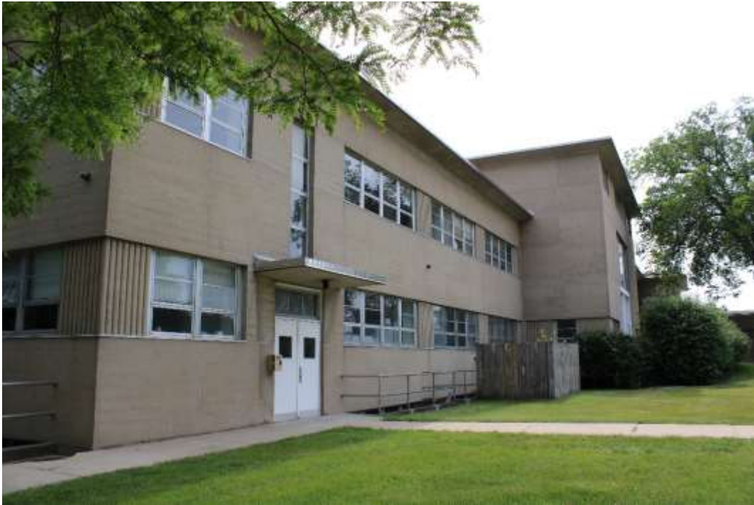
Photograph 25: Rear façade, view southwest.
