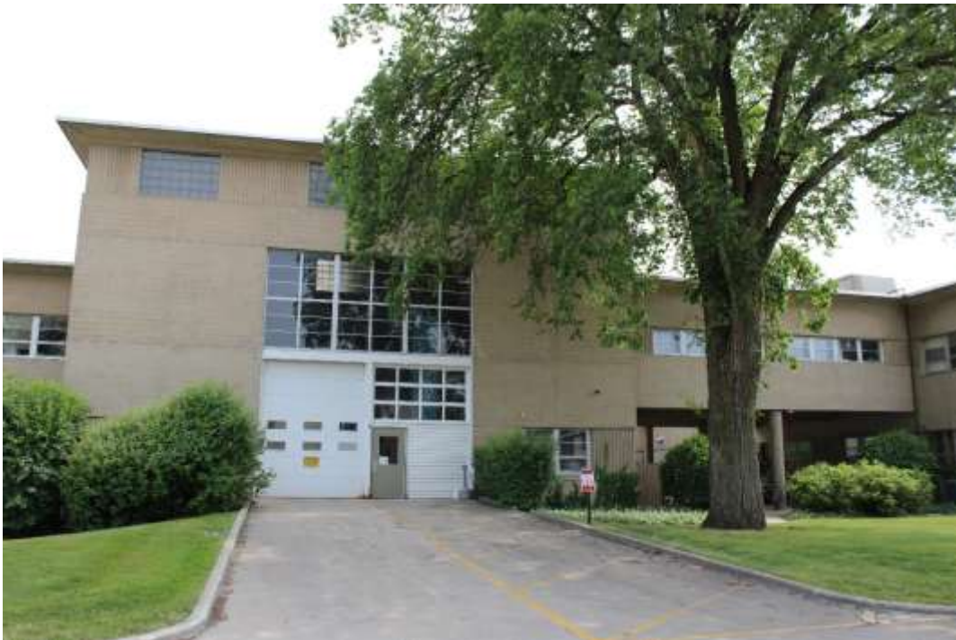
Photograph 24: Detail of high bay that houses the million pound testing machine, view south.
