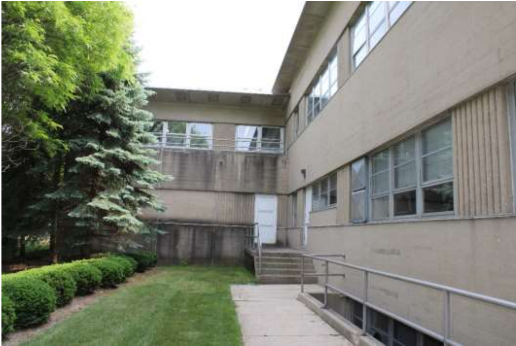
Photograph 27: Rear façade, view south.
