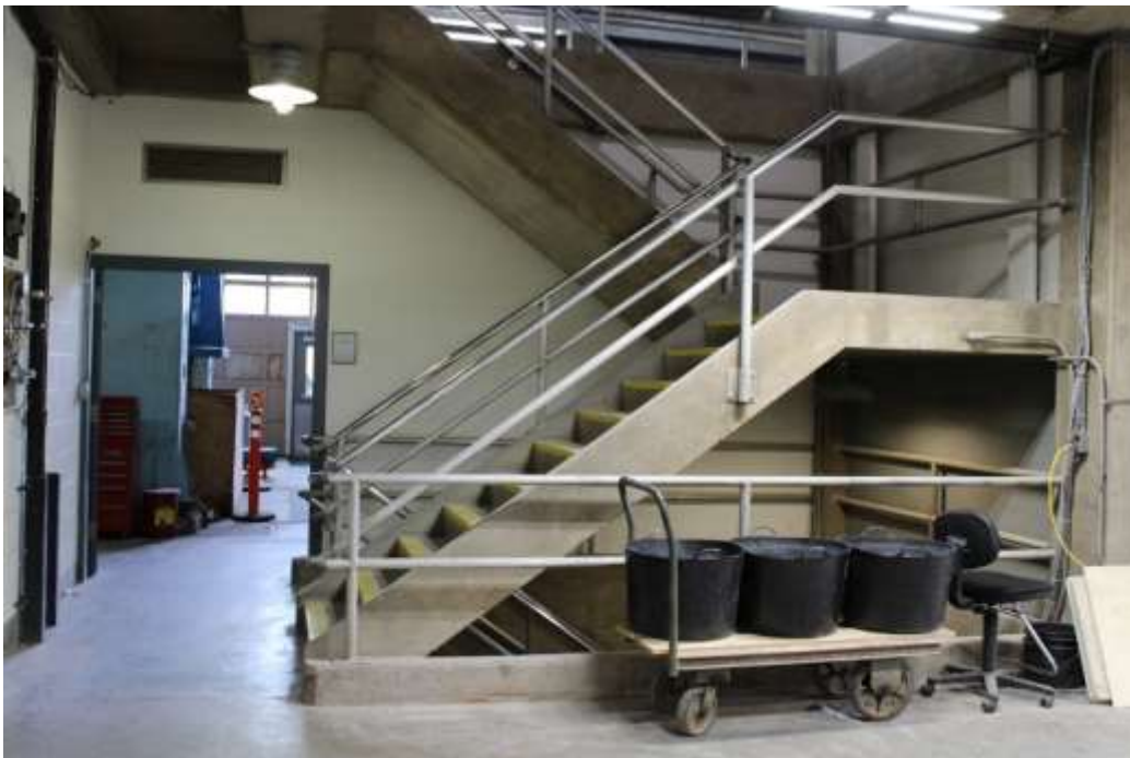
Photograph 38: Stairway in concrete mixing room.
