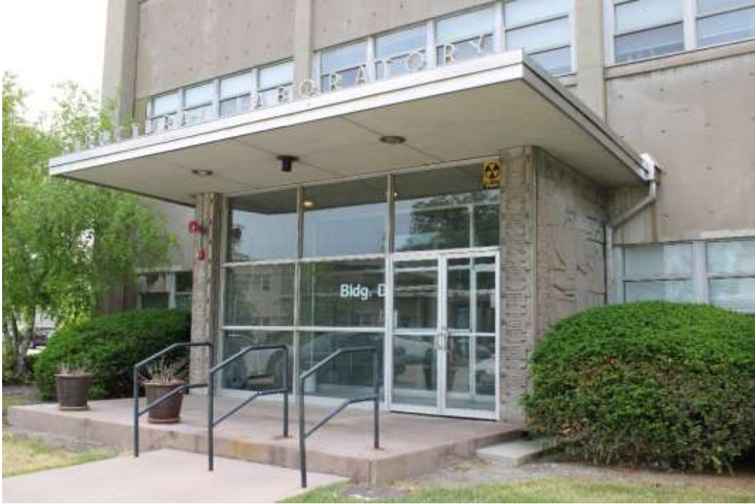
Photograph 2: Front entrance vestibule, view southwest.
