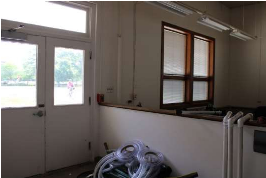
Photograph 21: Office along west side of building.
