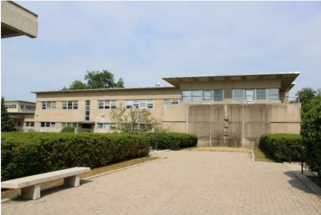
Photograph 9: West façade, view east.
