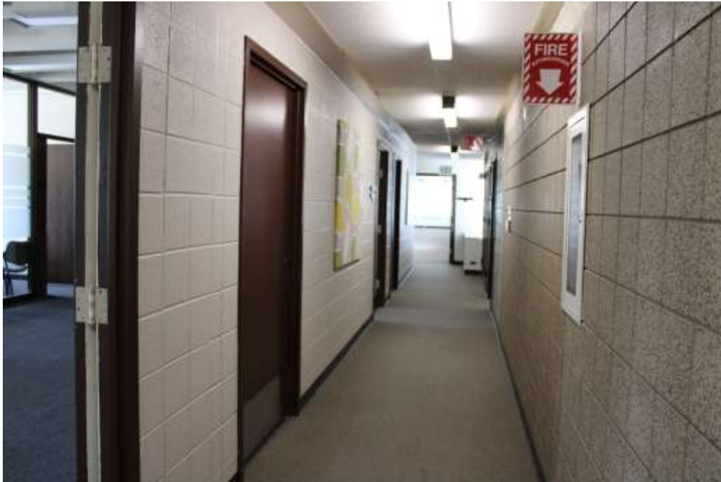
Photograph 36: Second floor corridor.
