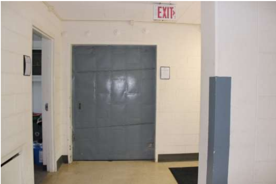
Photograph 51: Insulated door to first floor laboratory.
