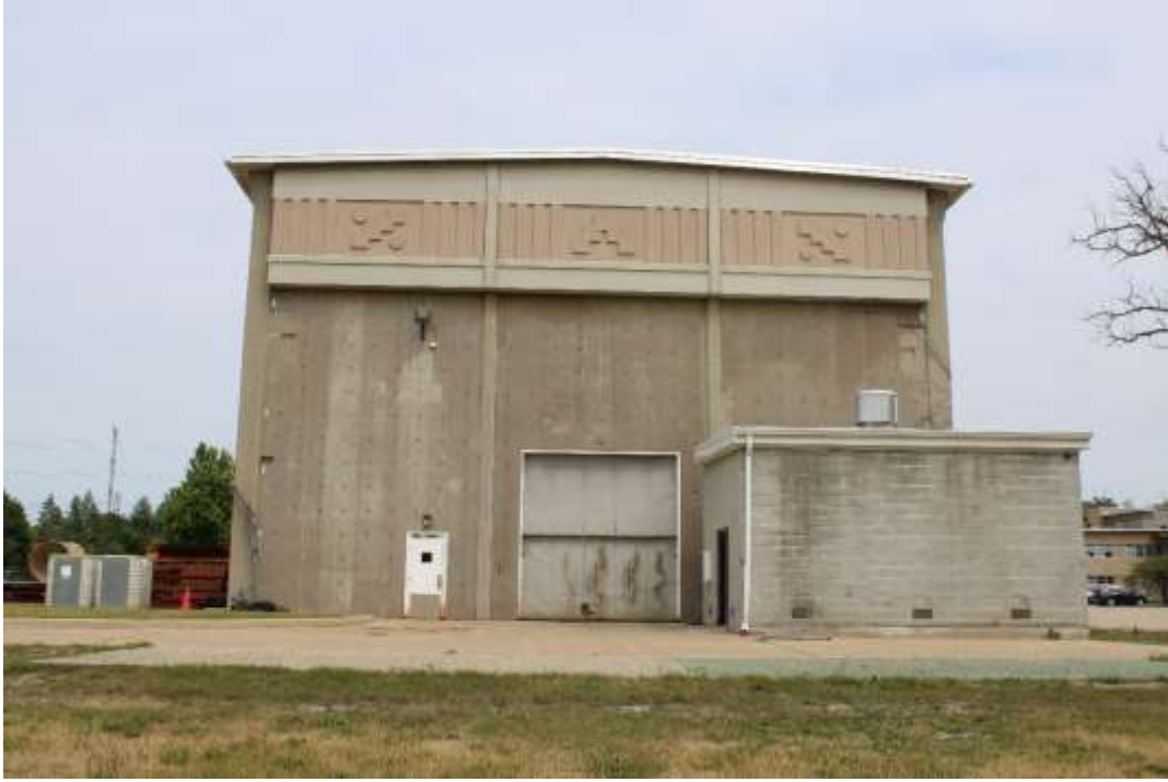
Photograph 8: West façade, view east.
