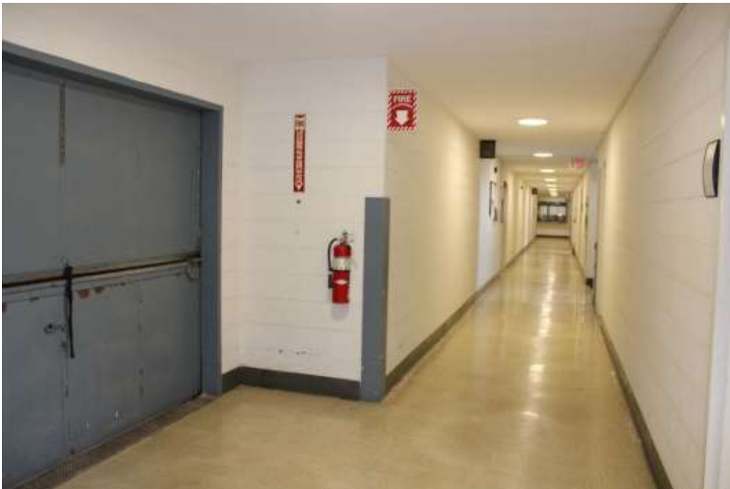
Photograph 49: Freight elevator and first floor hallway, view south.
