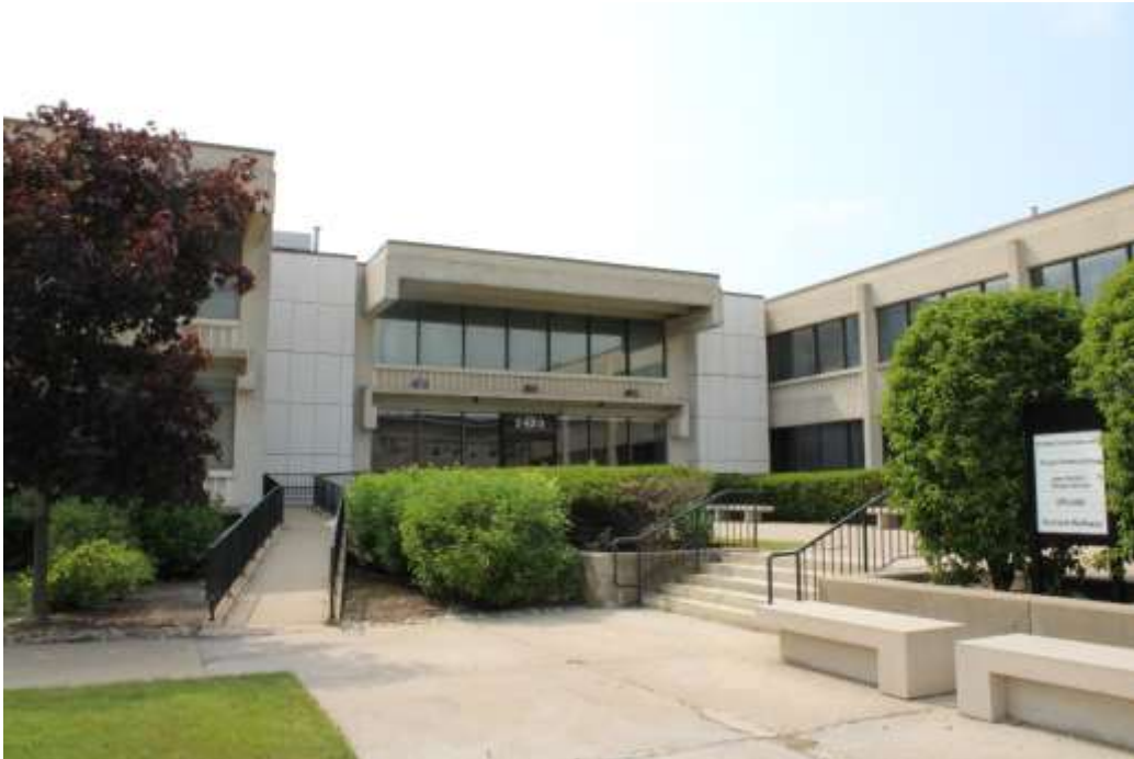
Photograph 1: Central entrance block showing raised terrace and concrete benches, view northwest.
