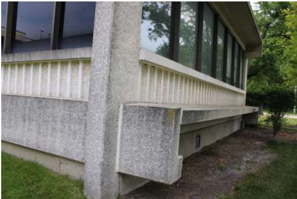
Photograph 14: Detail of south wing, view southeast.
