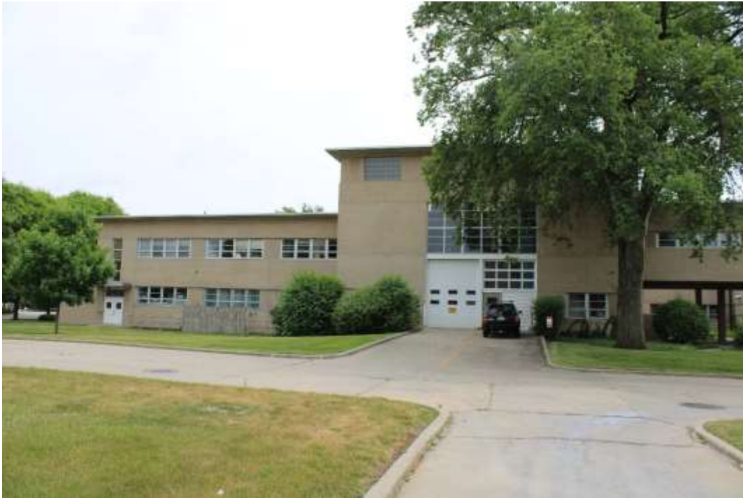
Photograph 23: Rear façade, view south.
