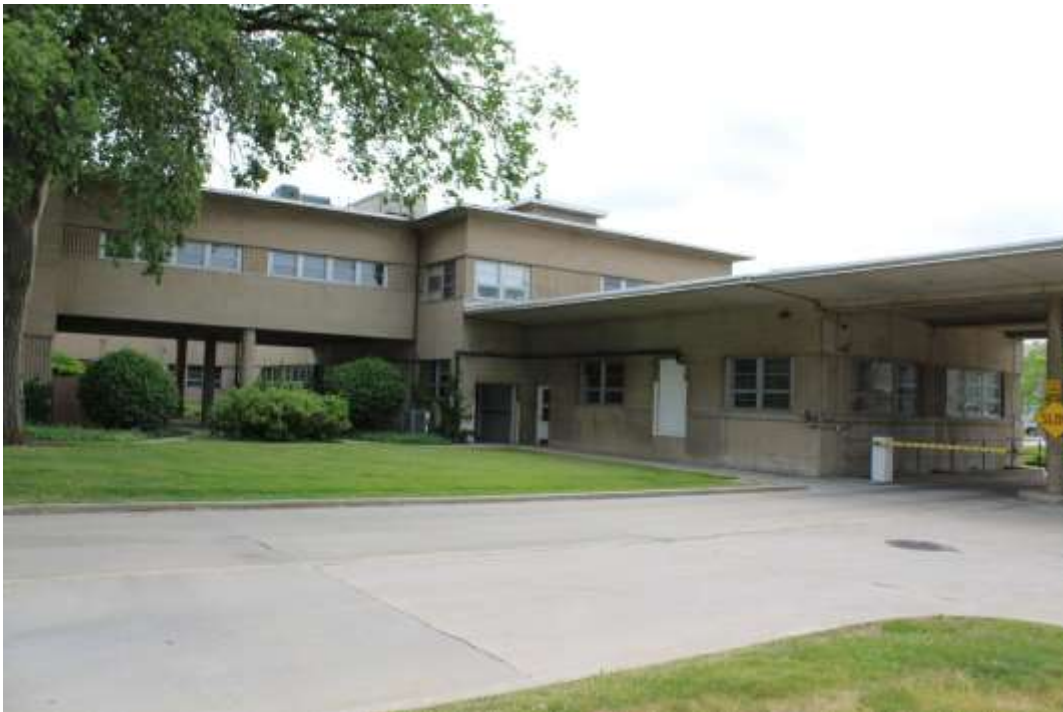
Photograph 18: Rear façade, view southwest toward opening to west courtyard.
