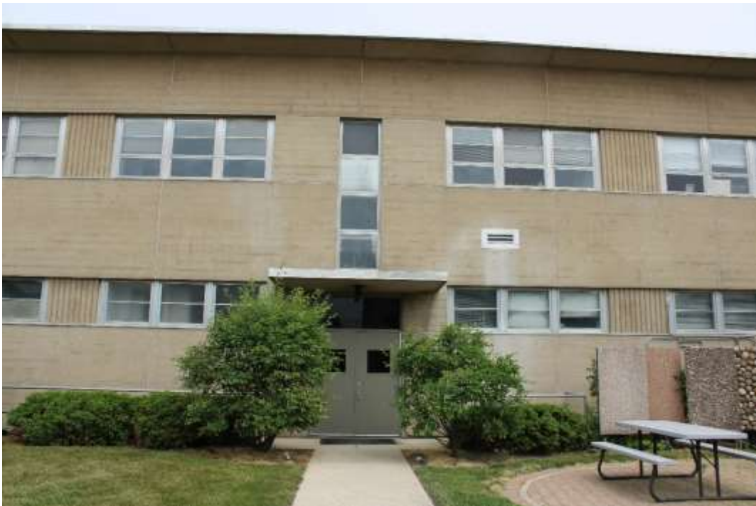
Photograph 14: West façade entrance, view east.
