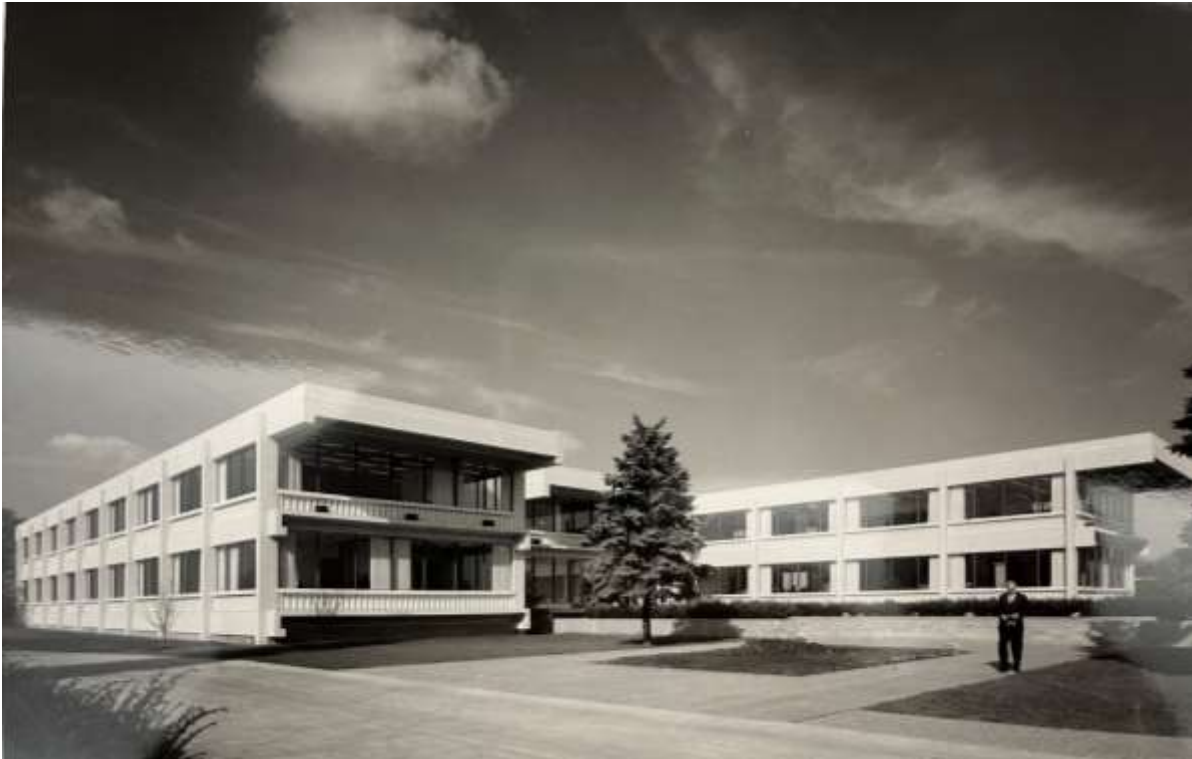
PCA Administration Building, view northwest. Hedrich-Blessing Photograph Collection, Job File HB-32054, Chicago History Museum.
