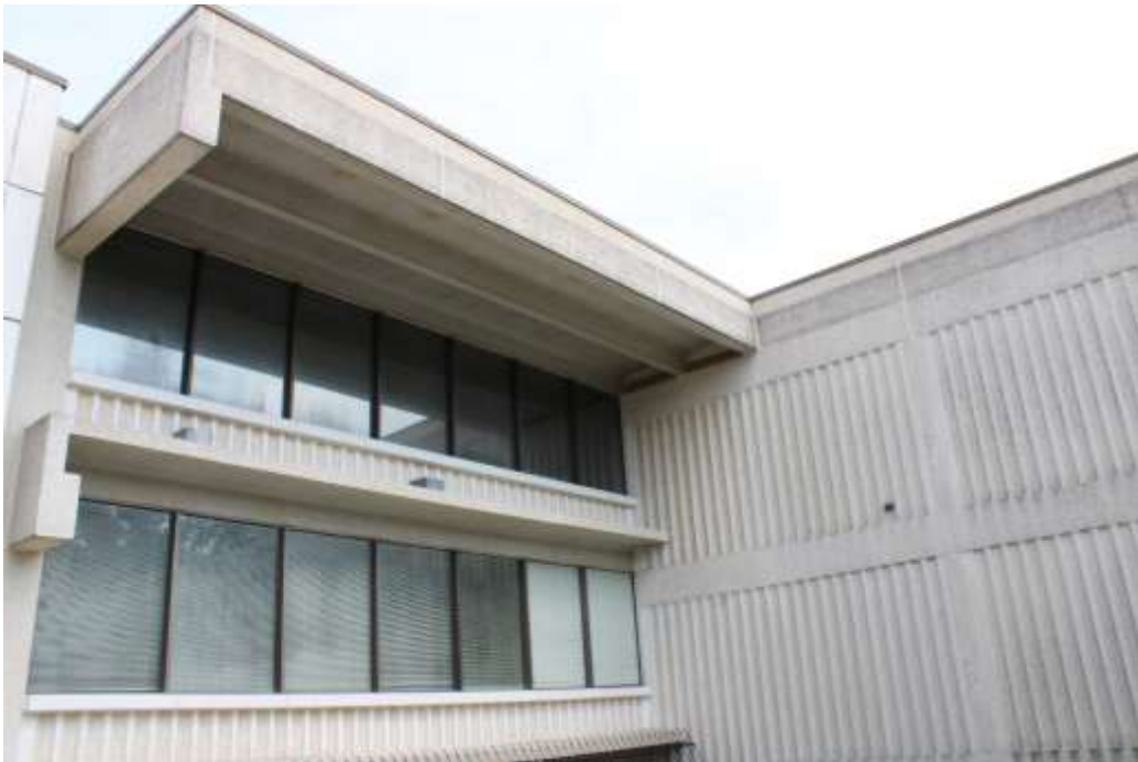
Photograph 10: Detail of central block (left) and stair tower (right), view southeast.
