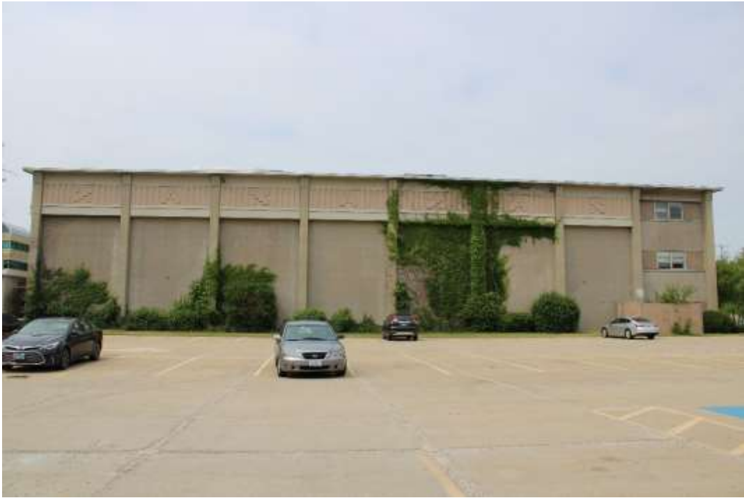
Photograph 11: South façade, view north.
