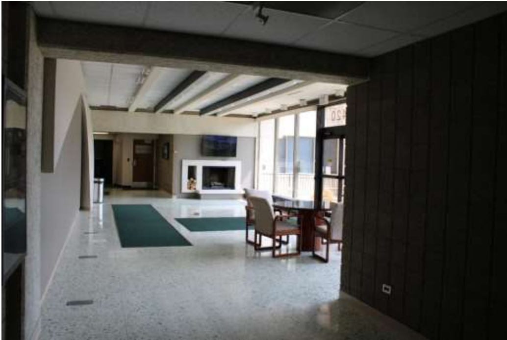
Photograph 17: Lobby with terrazzo flooring, view northeast.
