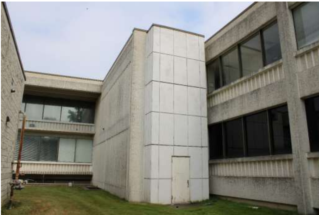
Photograph 12: Stair tower, view east.
