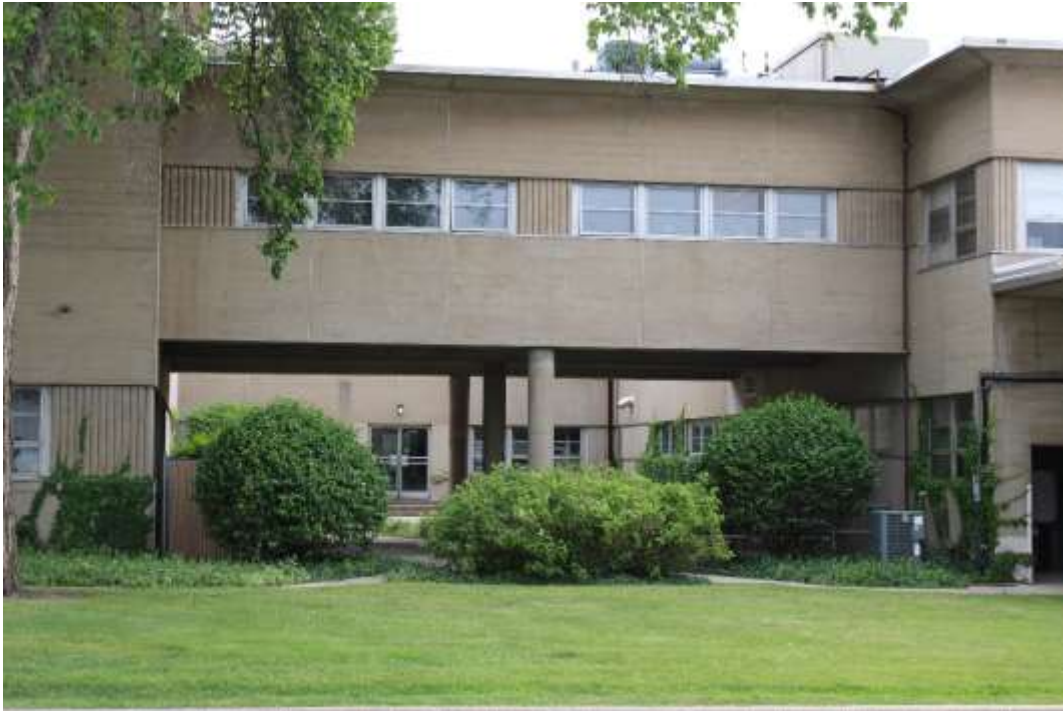
Photograph 19: Opening to west courtyard, view southwest.
