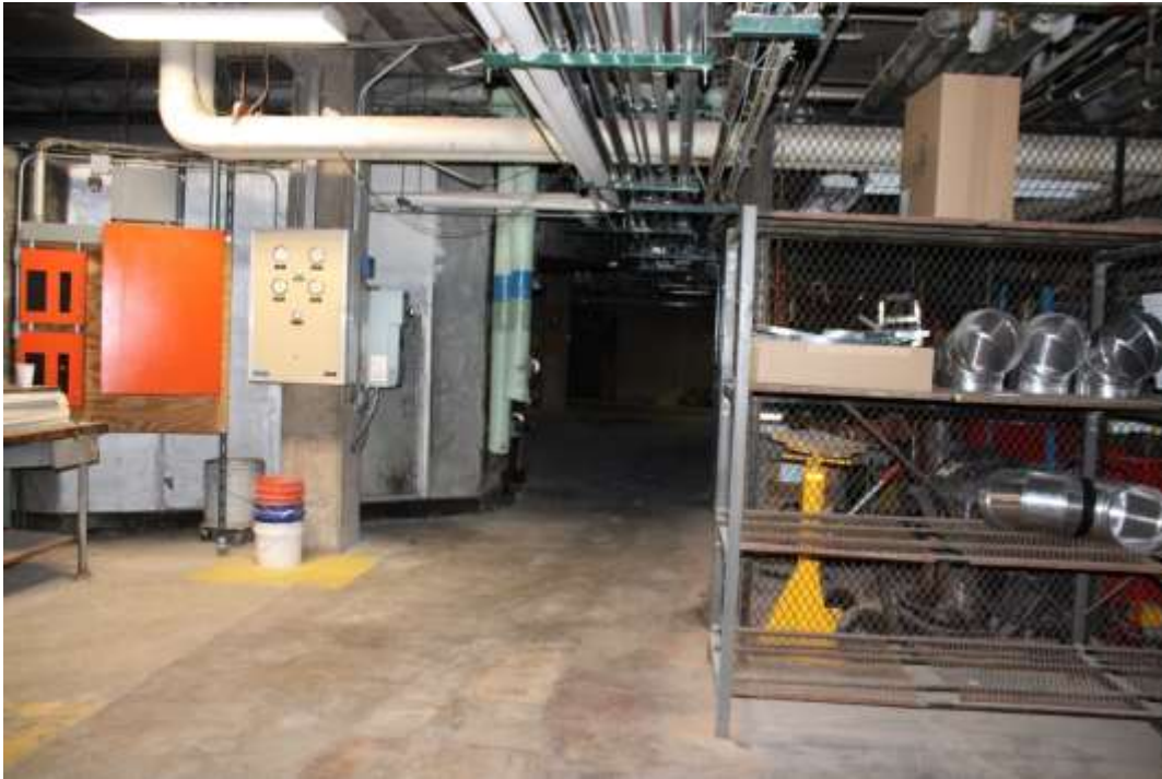
Photograph 64: Basement storage/mechanical space.
