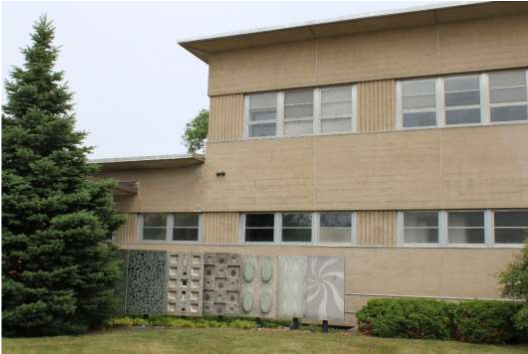
Photograph 15: Detail of west façade, view east.
