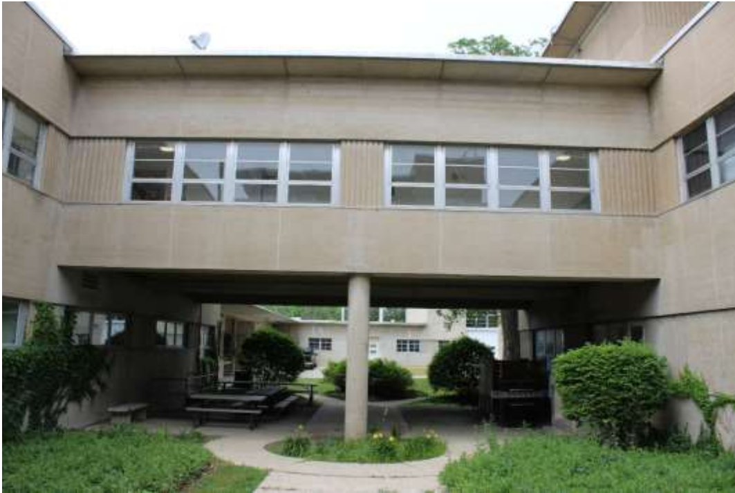
Photograph 21: West courtyard, view north.
