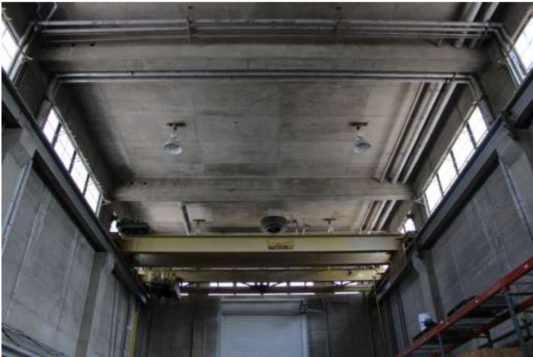
Photograph 27: High bay room ceiling
