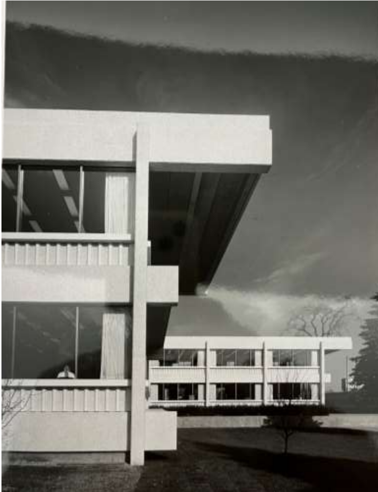
PCA Administration Building, view north. Hedrich-Blessing Photograph Collection, Job File HB-32054, Chicago History Museum.
