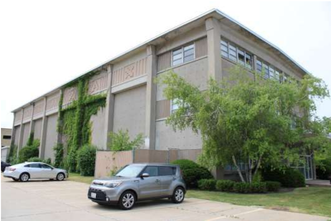
Photograph 12: South (left) and east (right) facades, view northwest.
