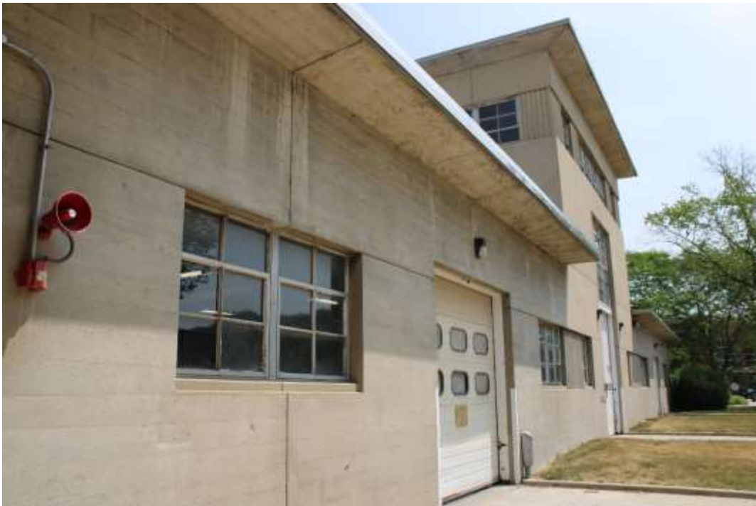
Photograph 4: South façade detail showing precast concrete panels.
