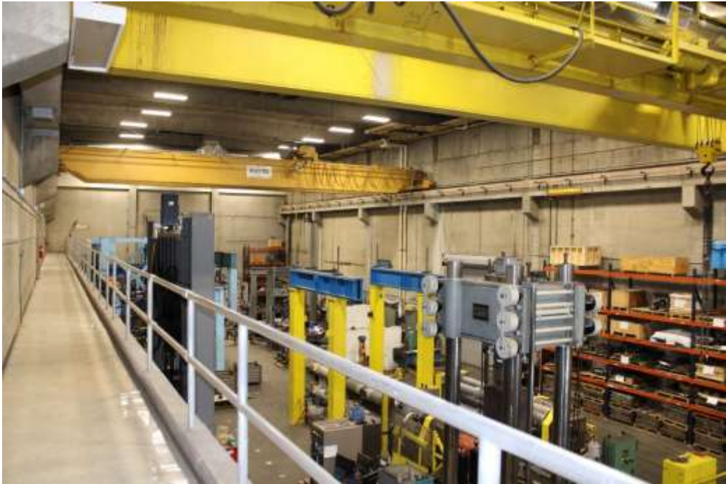
Photograph 28: Laboratory, view northwest from balcony spanning the south wall.
