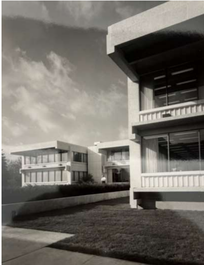
PCA Administration Building, view southwest. Hedrich-Blessing Photograph Collection, Job File HB-32054, Chicago History Museum.
