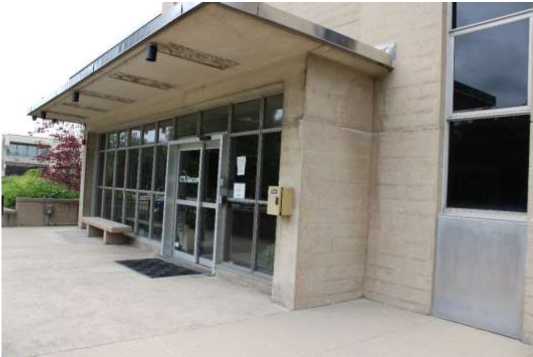
Photograph 4: Main entrance, view northwest.
