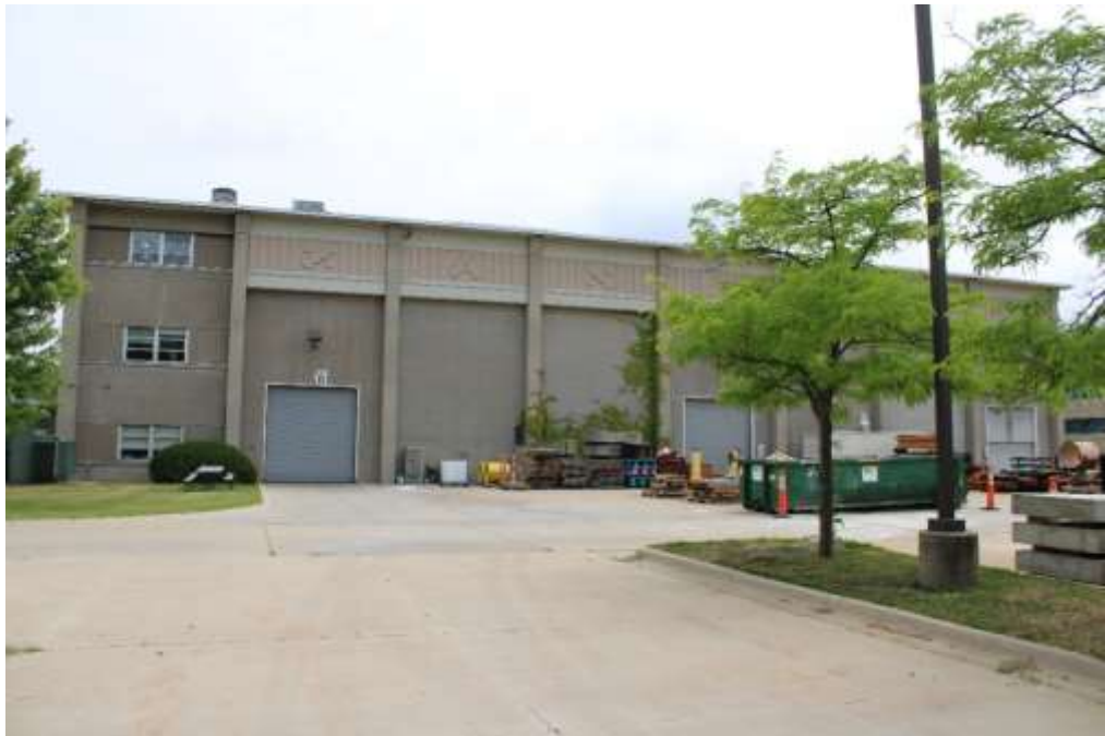
Photograph 6: North façade, view south.
