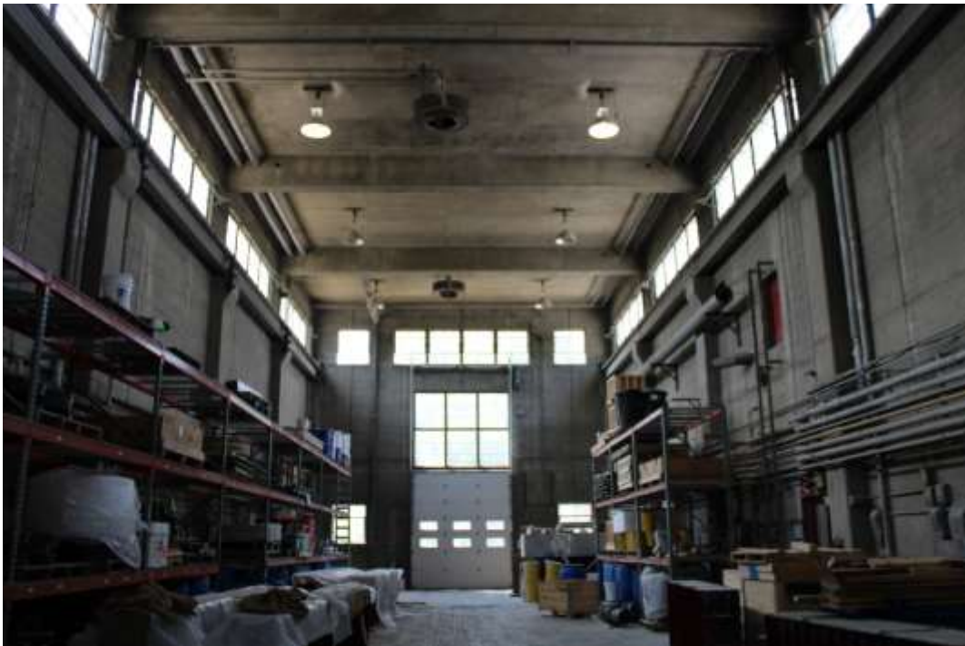
Photograph 24: High bay room, view south.
