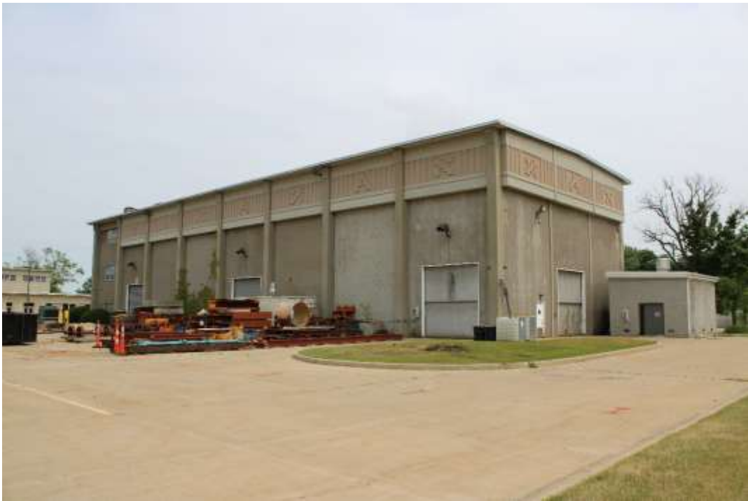
Photograph 7: North (left) and west (right) facades, view southeast.
