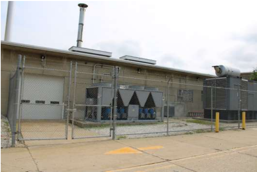
Photograph 11: North façade, view southwest.
