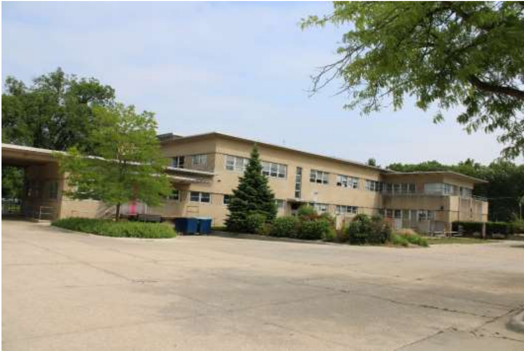
Photograph 11: West façade, view southeast.
