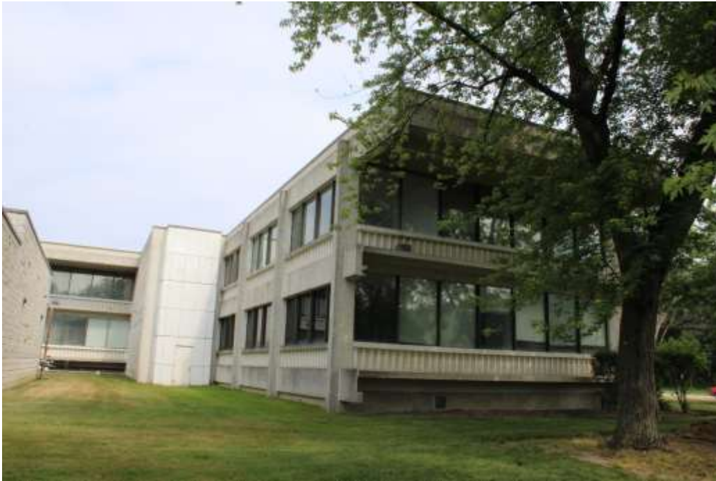
Photograph 15: South wing, view southeast.
