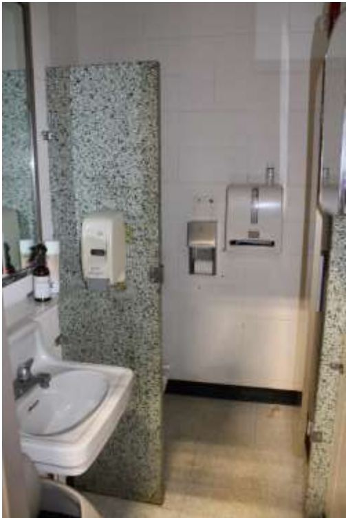
Photograph 25: Toilet room with concrete partitions.
