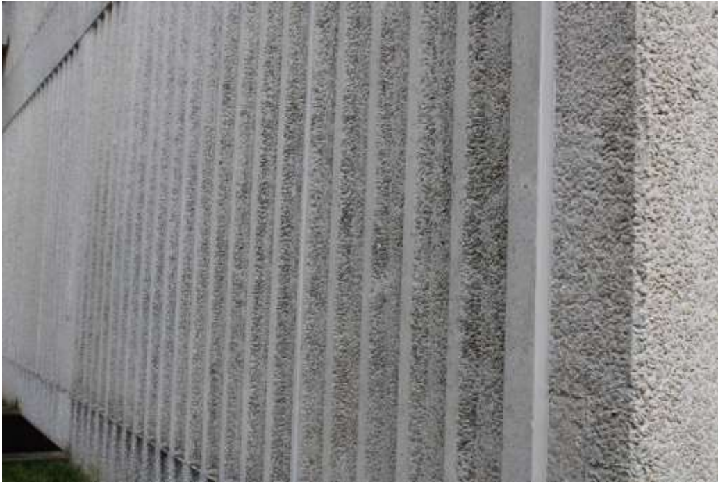
Photograph 11: Detail of stair tower.
