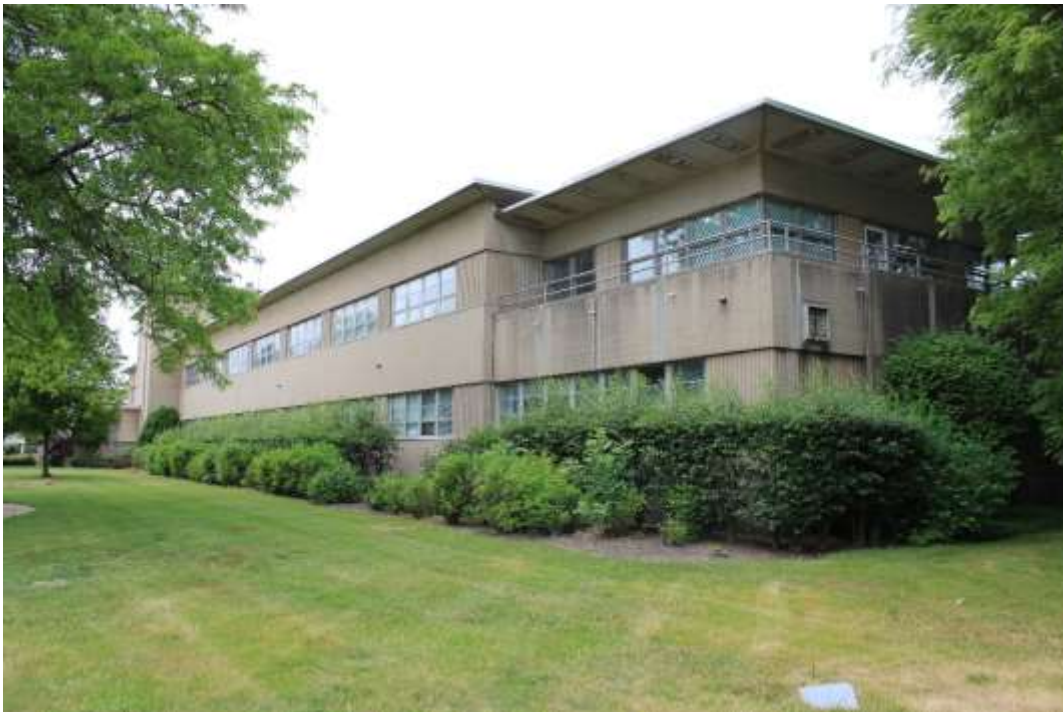
Photograph 28: Front façade, view northeast.
