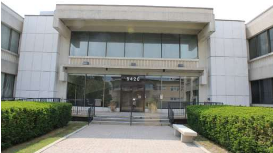
Photograph 2: Central entrance block, view west.
