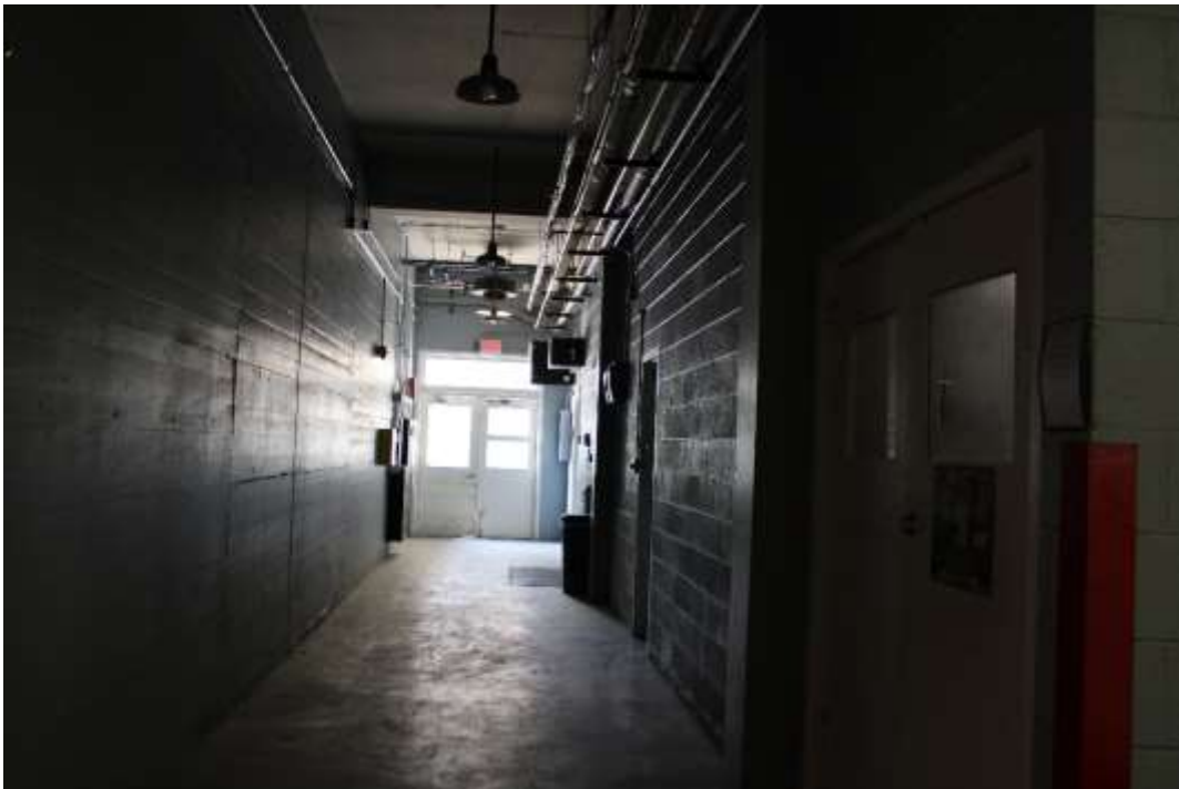
Photograph 16: Corridor, view south.
