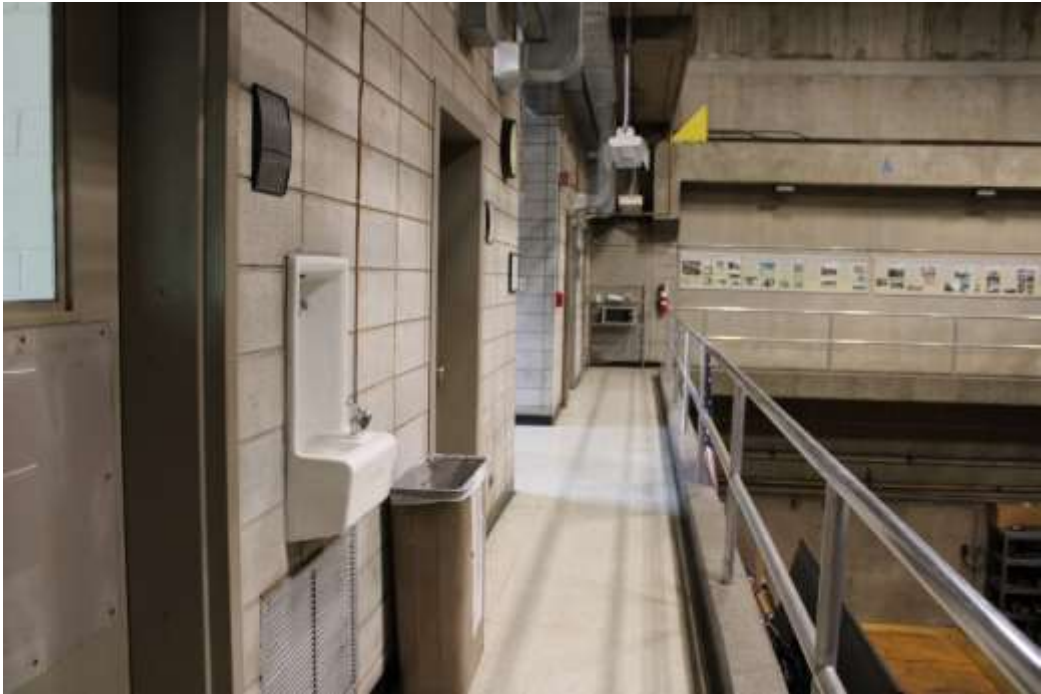
Photograph 20: Second floor balcony spanning east end of laboratory, view south.
