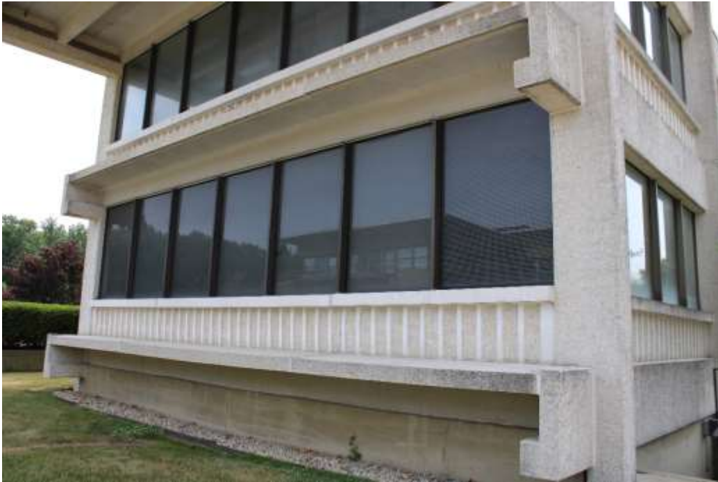
Photograph 7: Detail of north wing, view southwest.
