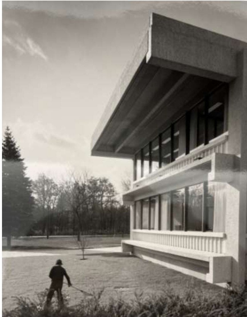
PCA Administration Building, view southwest. Hedrich-Blessing Photograph Collection, Job File HB-32054, Chicago History Museum.
