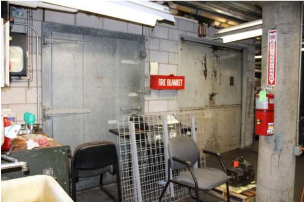
Photograph 37: Basement showing freight elevator and insulated door.
