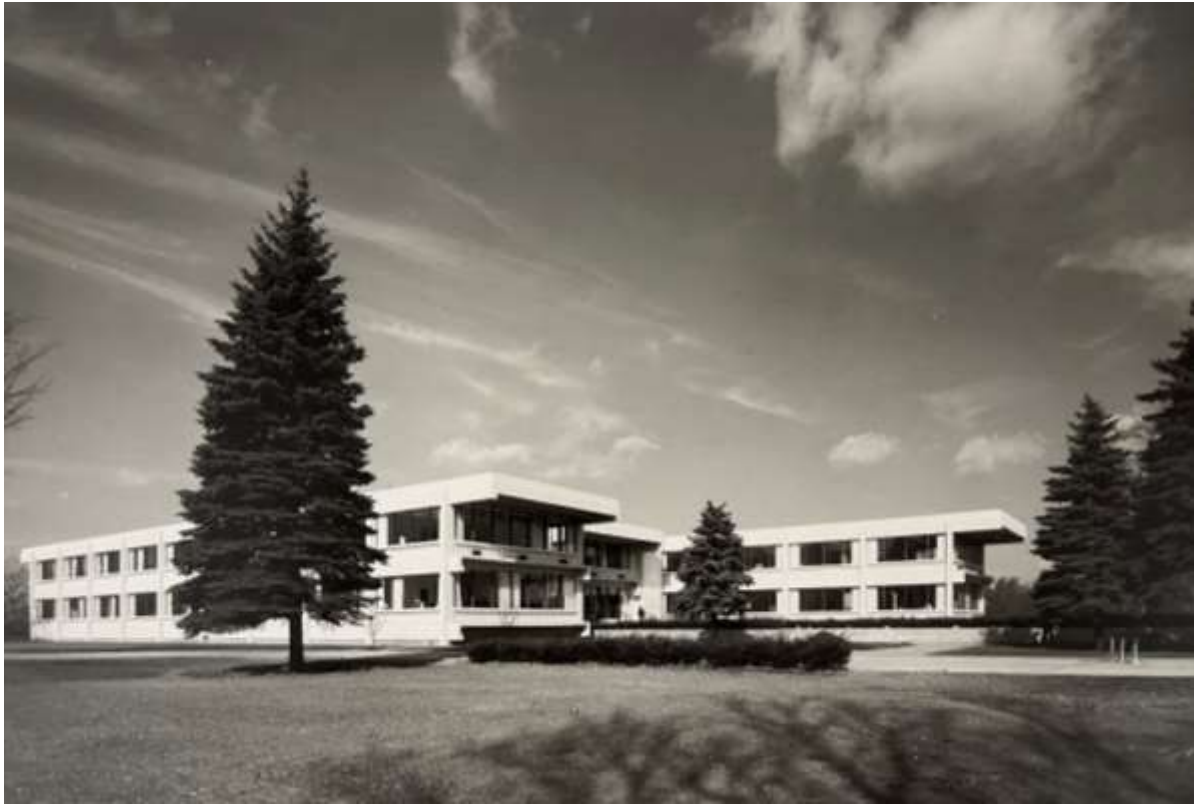
PCA Administration Building, view northwest. Hedrich-Blessing Photograph Collection, Job File HB-32054, Chicago History Museum.
