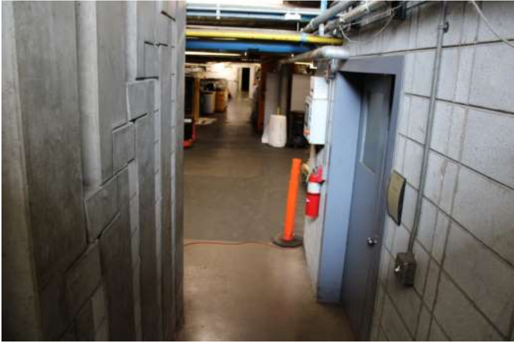
Photograph 35: Corridor leading to basement.
