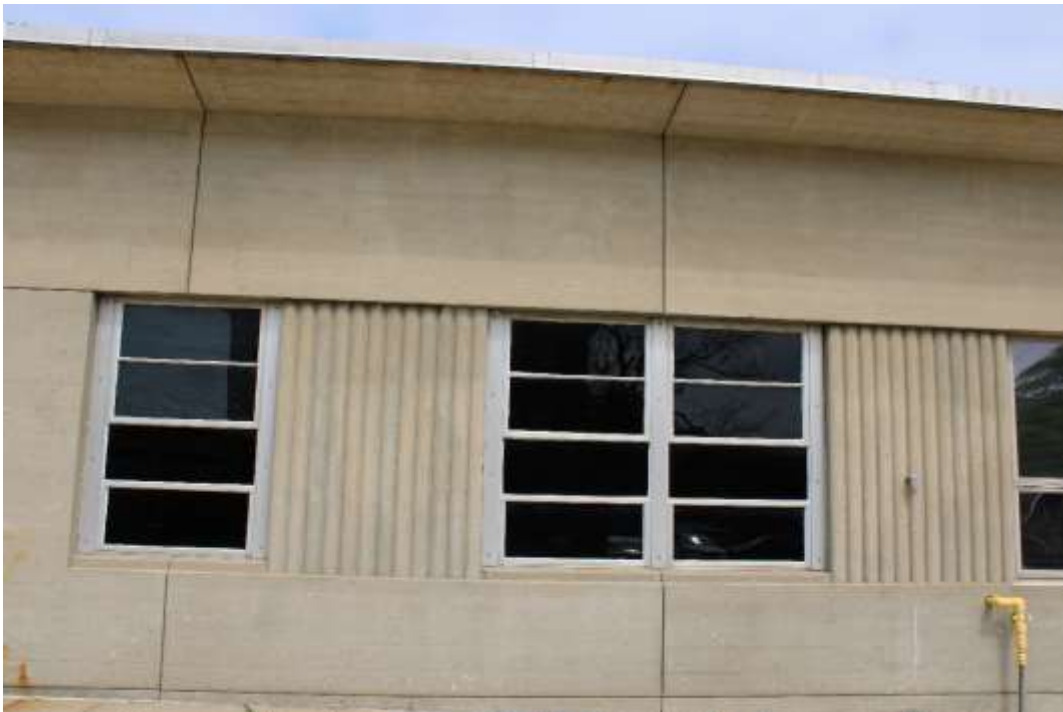
Photograph 14: West façade, detail of windows and precast concrete panels.
