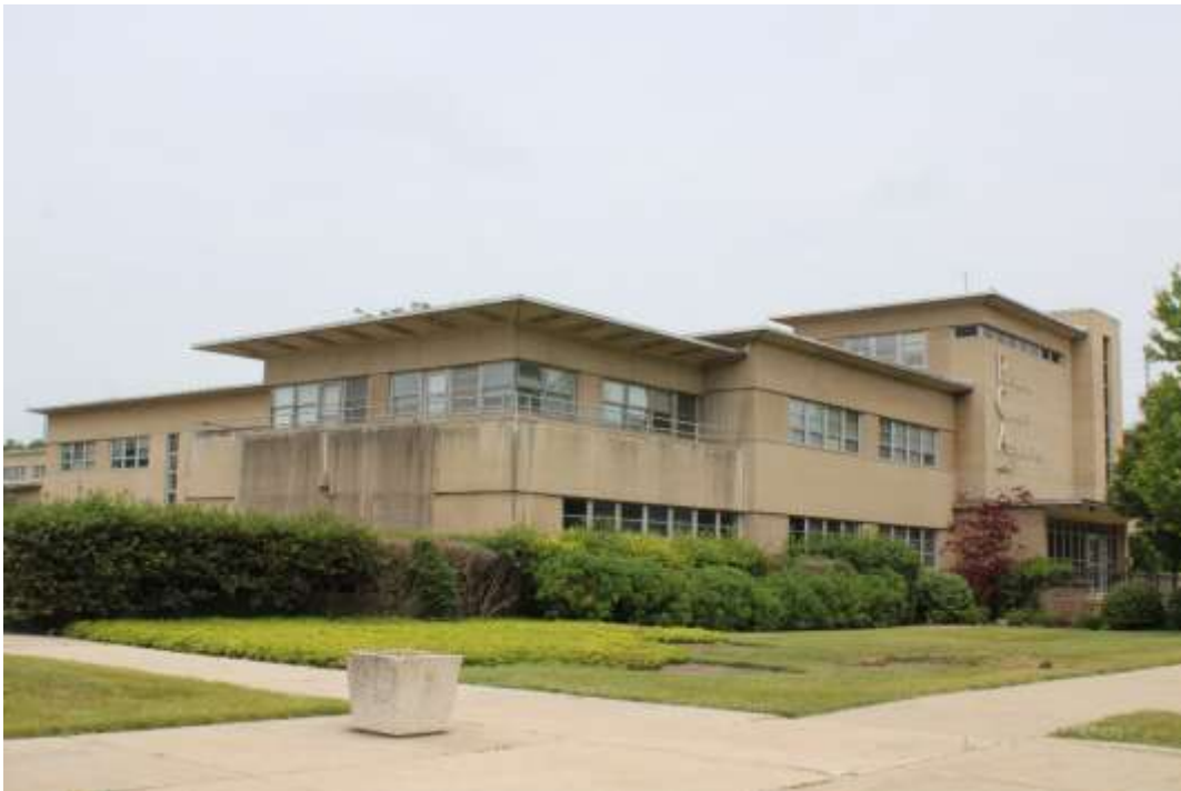
Photograph 8: Front façade, view northeast.
