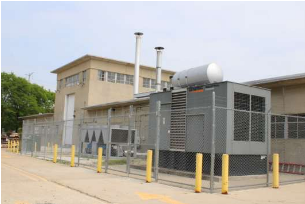
Photograph 8: North façade, view southeast.
