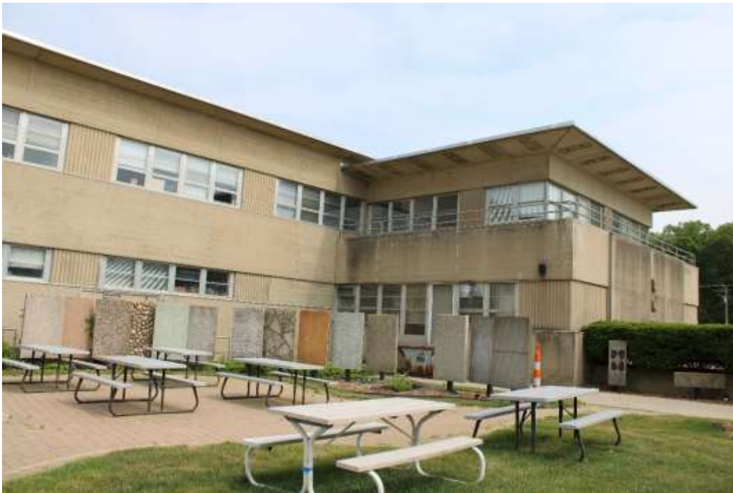
Photograph 12: Detail of west façade, view southeast.
