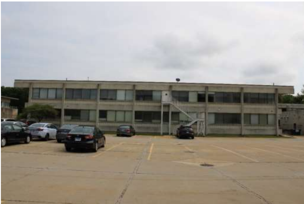
Photograph 8: North wing, view south.
