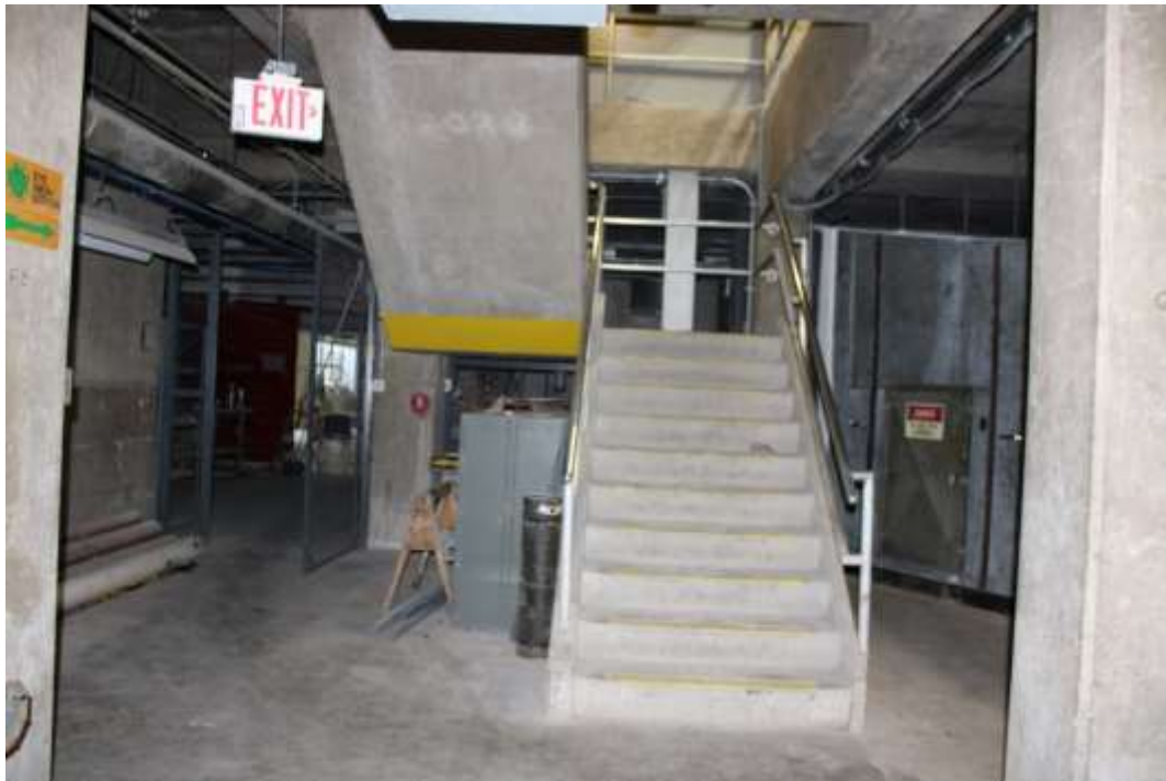
Photograph 63: Concrete stairway in center of building, view from basement.
