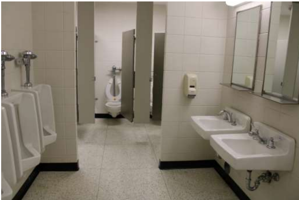
Photograph 26: Typical men's toilet room.
