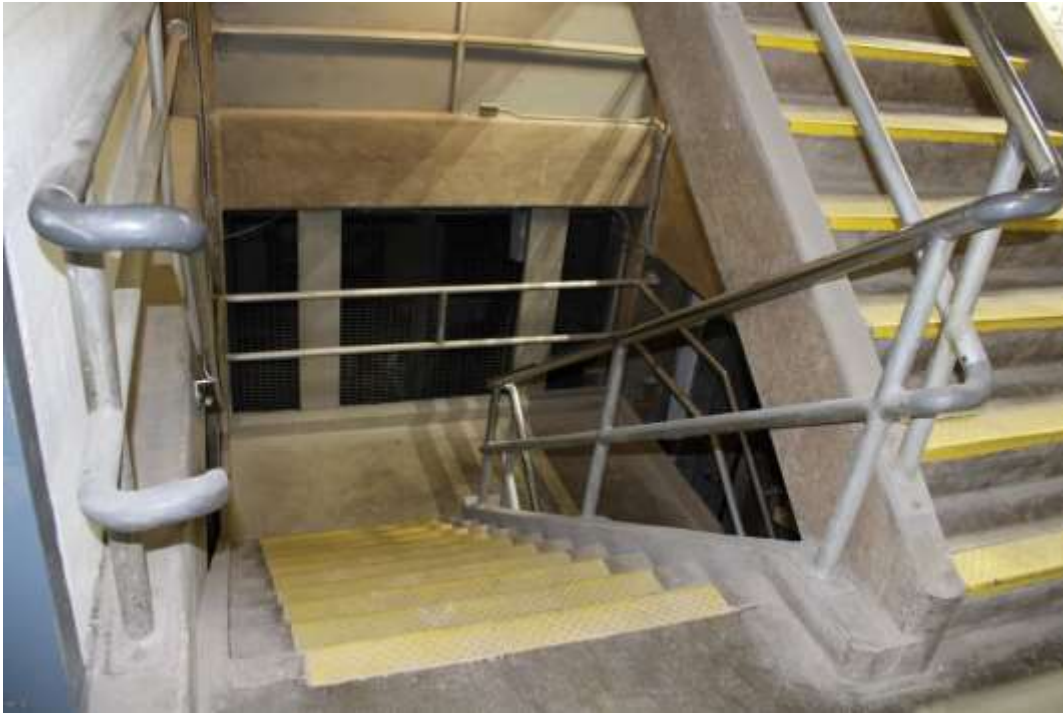
Photograph 62: Concrete stairway in center of building, view toward basement landing.
