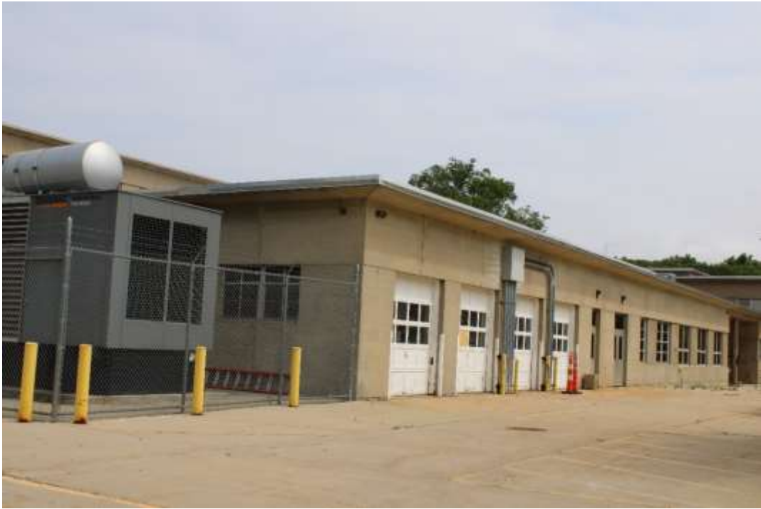
Photograph 12: West façade, view southeast.
