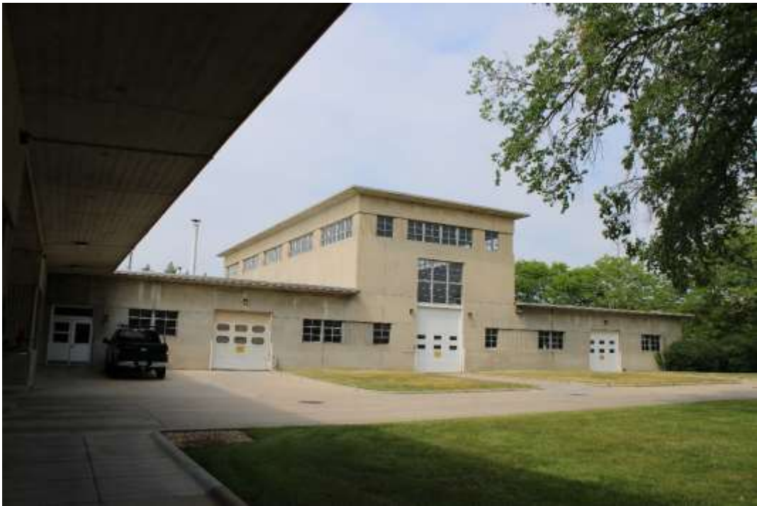
Photograph 1: South façade, view northeast.
