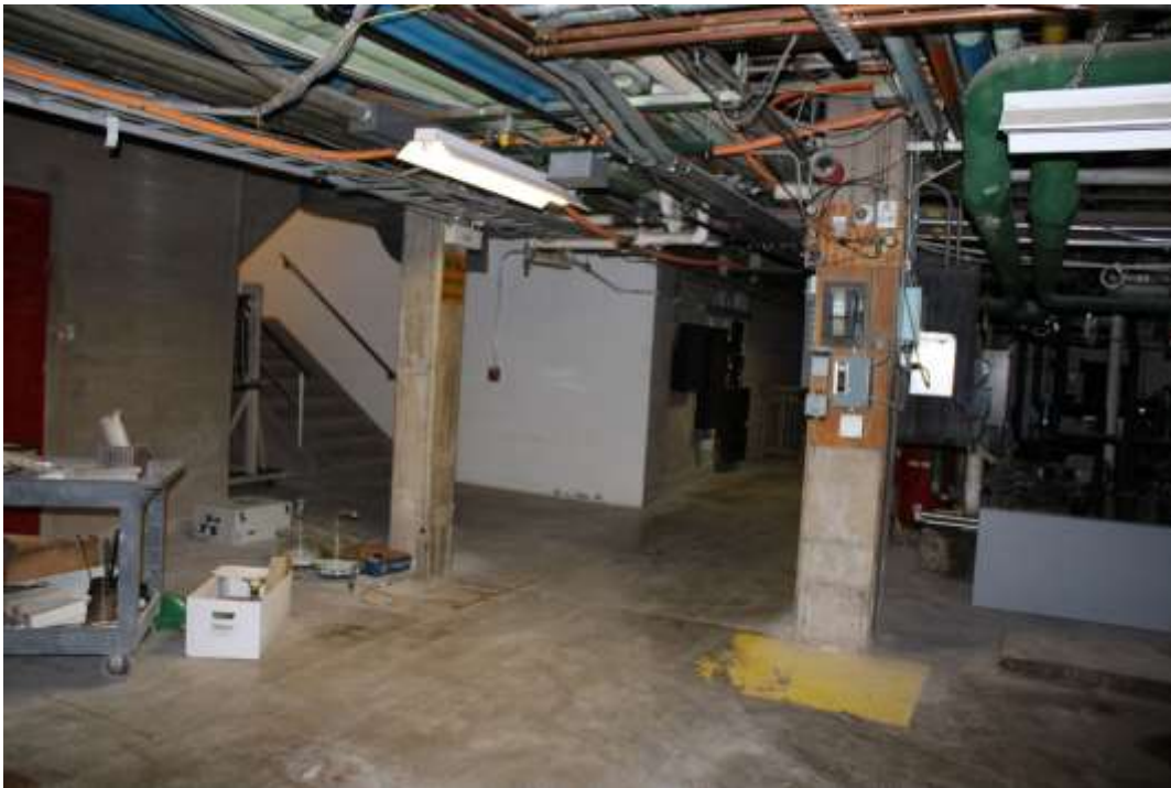
Photograph 65: Basement storage/mechanical space.
