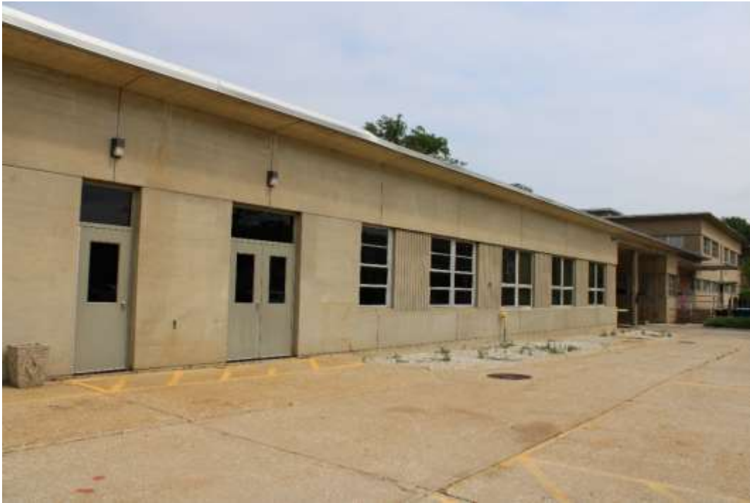
Photograph 13: West façade, view southeast.
