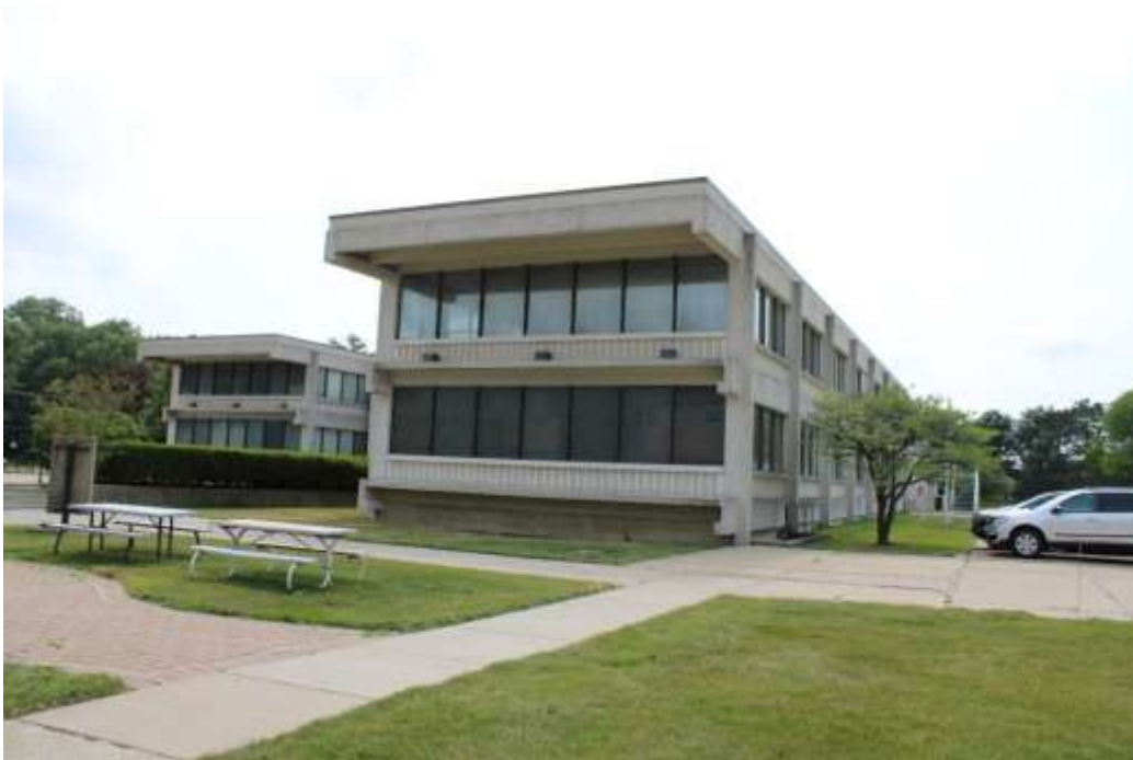
Photograph 6: South wing (left) and north wing (right), view southwest.
