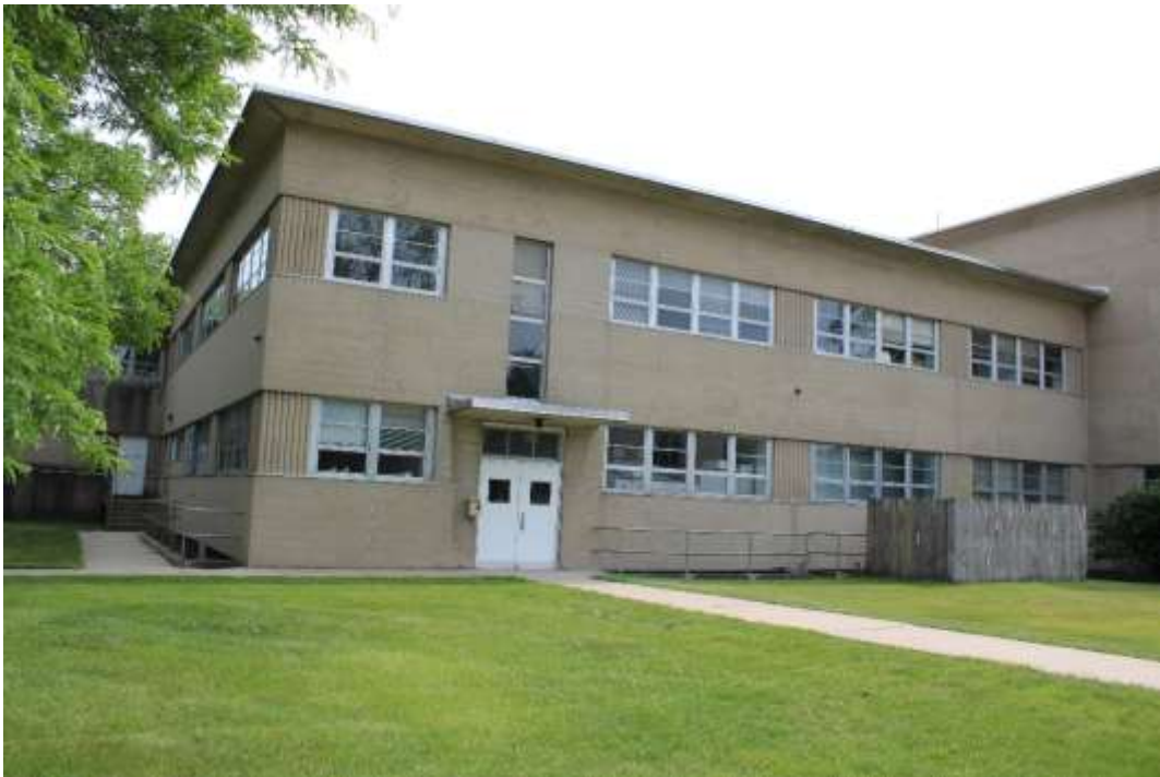
Photograph 26: Rear façade, view southwest.
