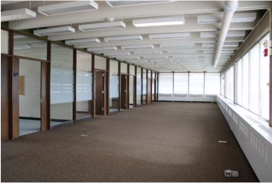
Photograph 28: Second floor workspace separated from perimeter offices by a glass partition wall.
