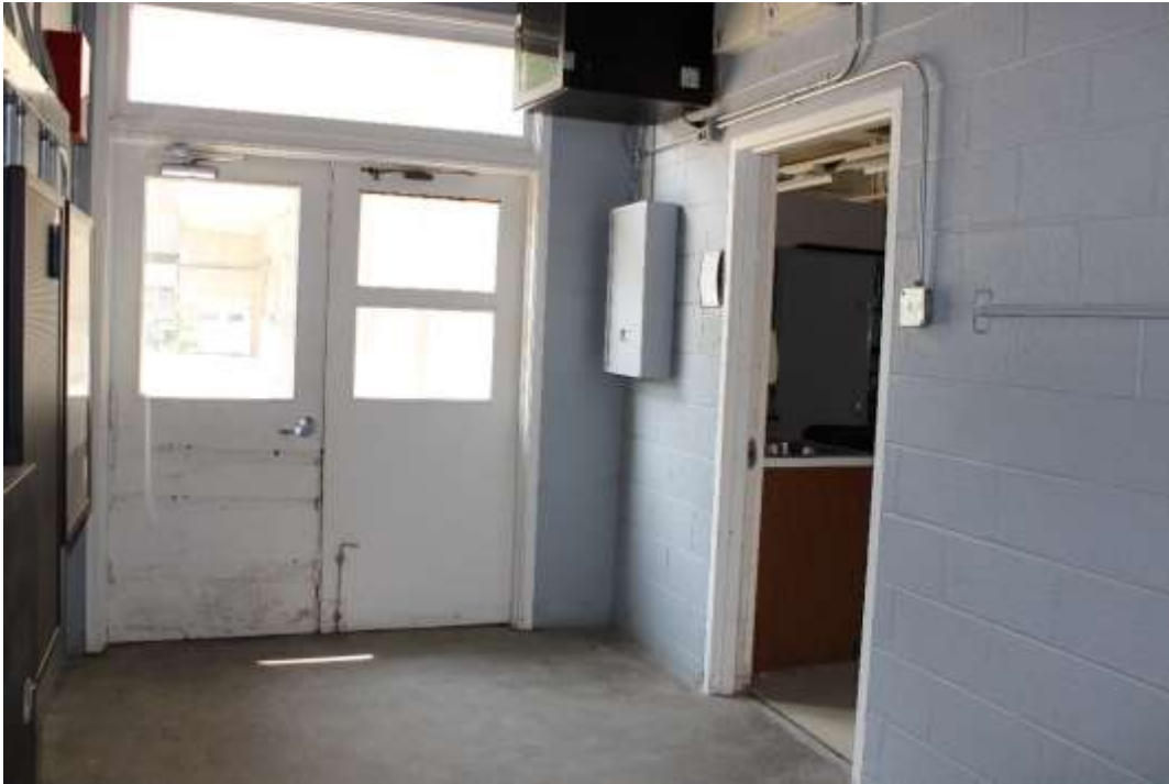
Photograph 17: Corridor, view south toward exterior door.
