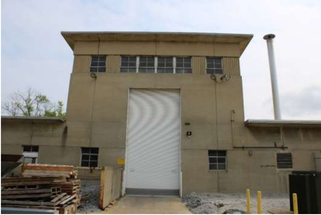
Photograph 10: North façade high bay, view south.
