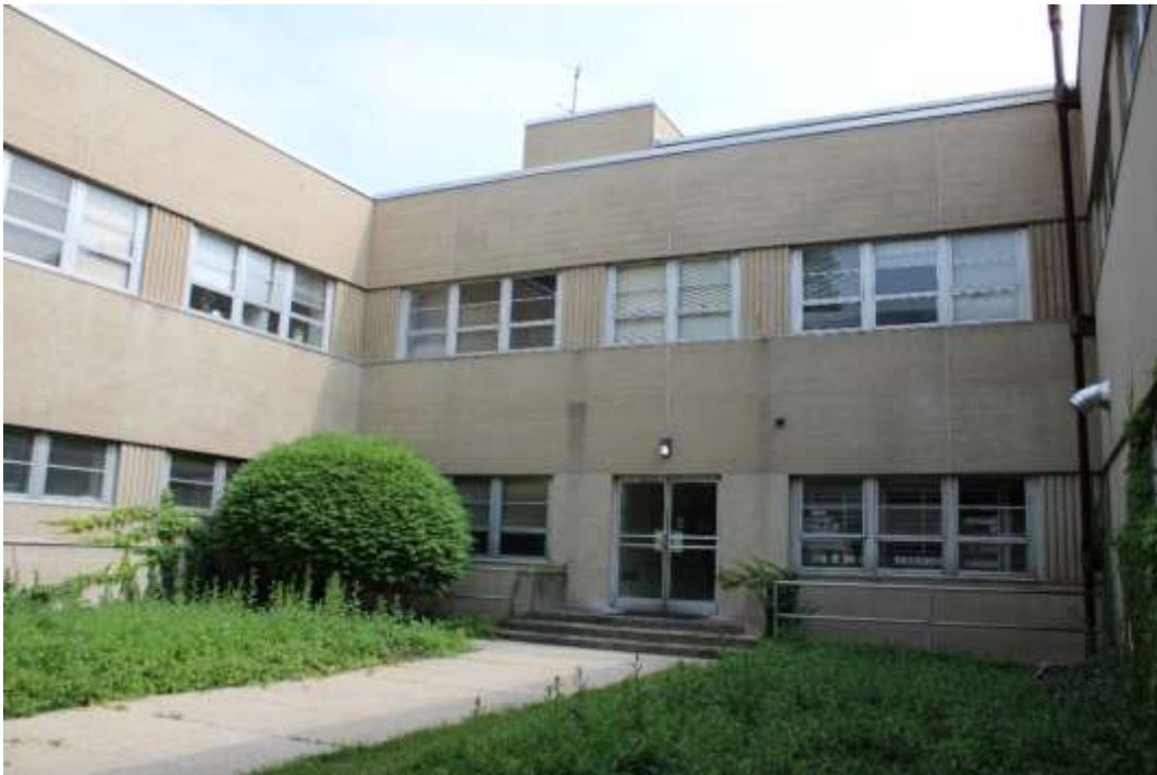
Photograph 20: West courtyard, view southeast.
