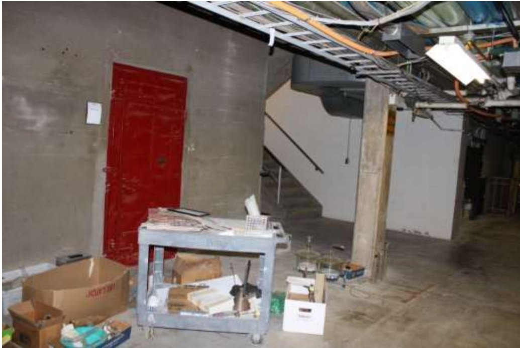
Photograph 66: Basement storage/mechanical space.
