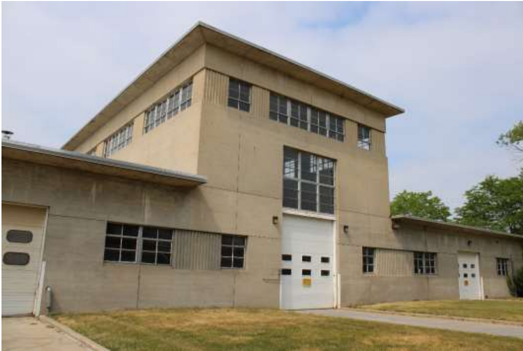
Photograph 3: South façade, view northeast.
