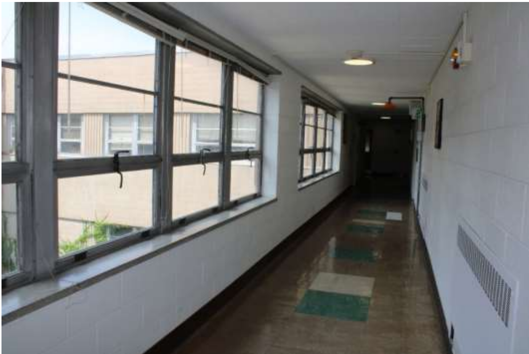
Photograph 59: Second floor walkway overlooking west courtyard.
