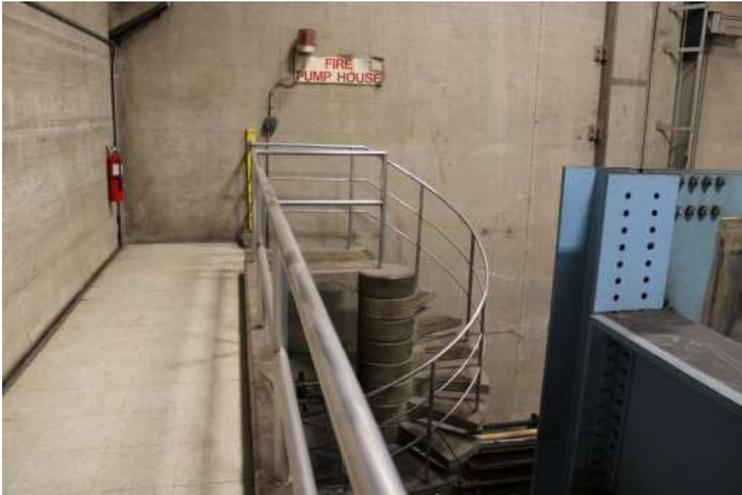
Photograph 32: Spiral concrete staircase in the southwest corner of the laboratory.
