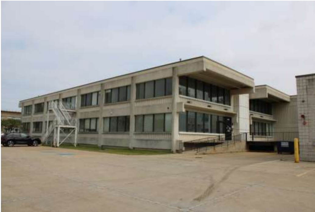
Photograph 9: North wing, view southeast.
