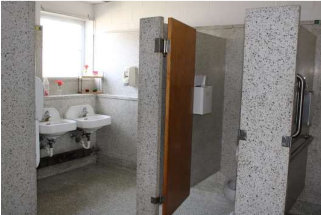
Photograph 48: Women's toilet room with concrete partitions.
