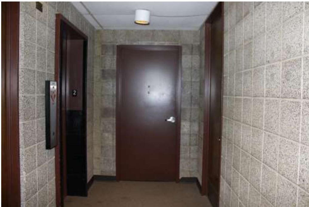
Photograph 35: Second floor elevator lobby.
