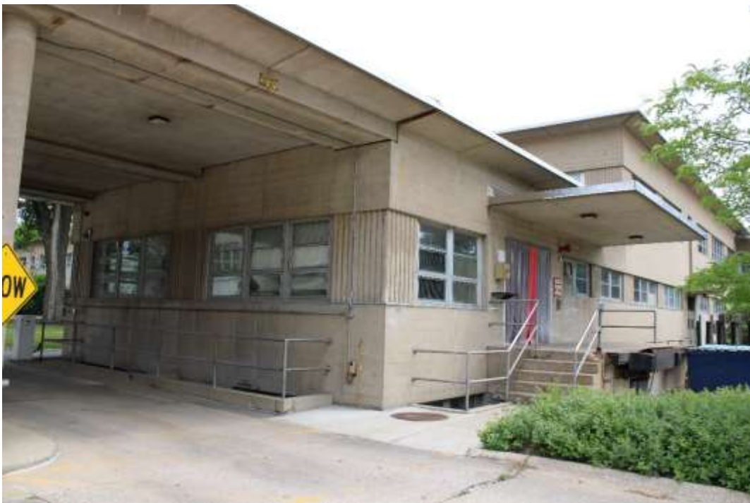
Photograph 16: Detail of canopy linking the Research Building with the Material Storage Building.
