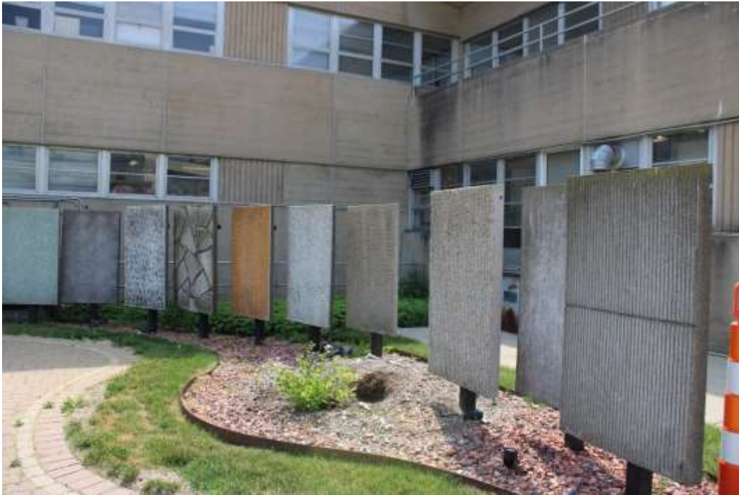
Photograph 13: Concrete panels placed on lawn next to west façade, view southeast.
