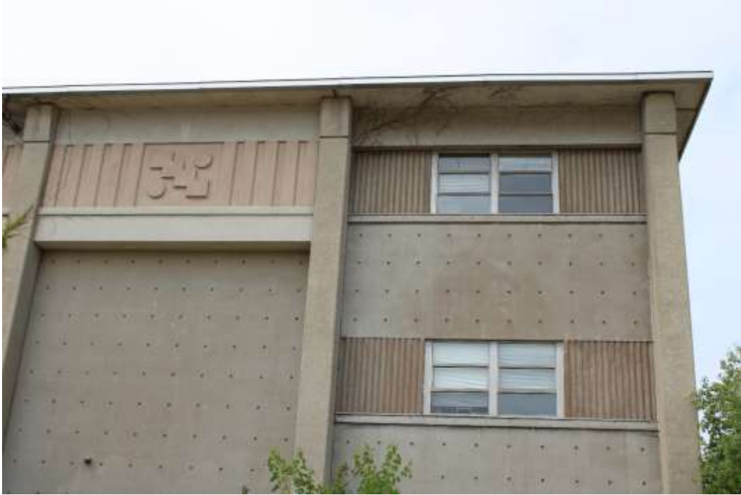
Photograph 13: Detail of precast concrete panels on south façade, view north.
