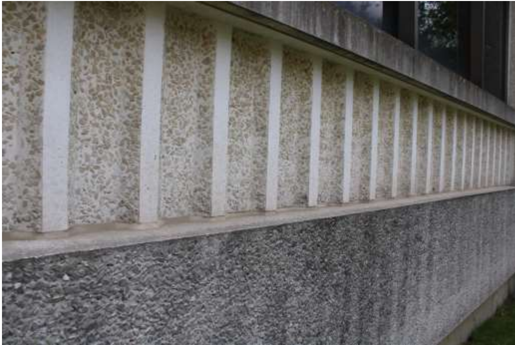
Photograph 13: Detail of concrete spandrel with exposed aggregate.
