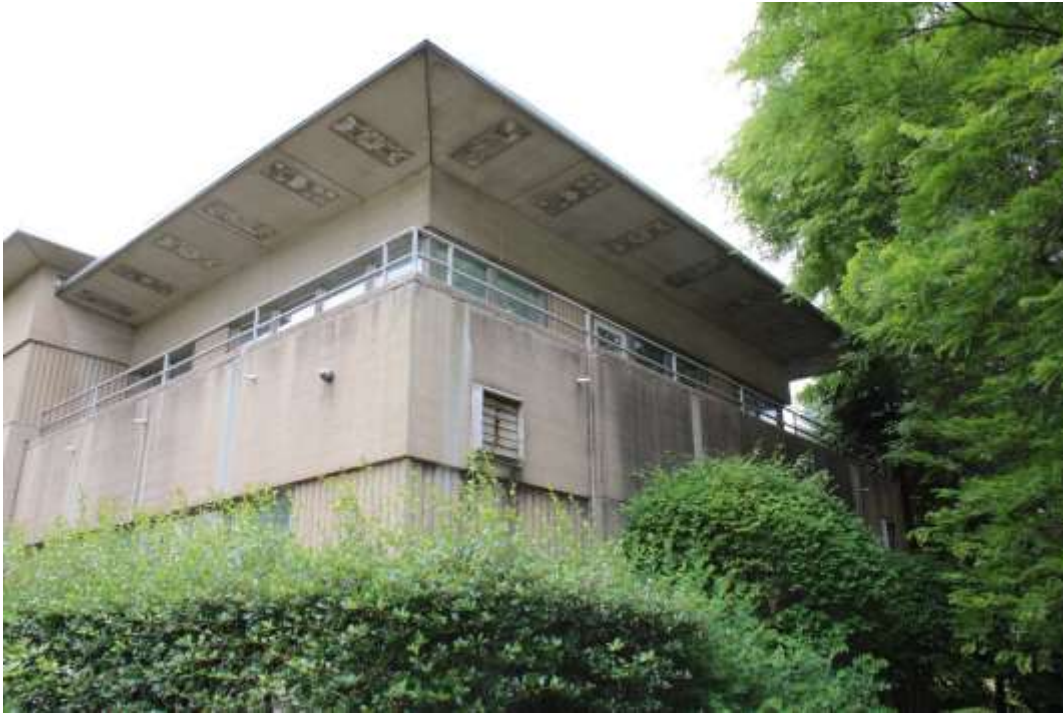
Photograph 29: Southeast corner of the building, showing soffits with decorative concrete panels and aluminum railings.
