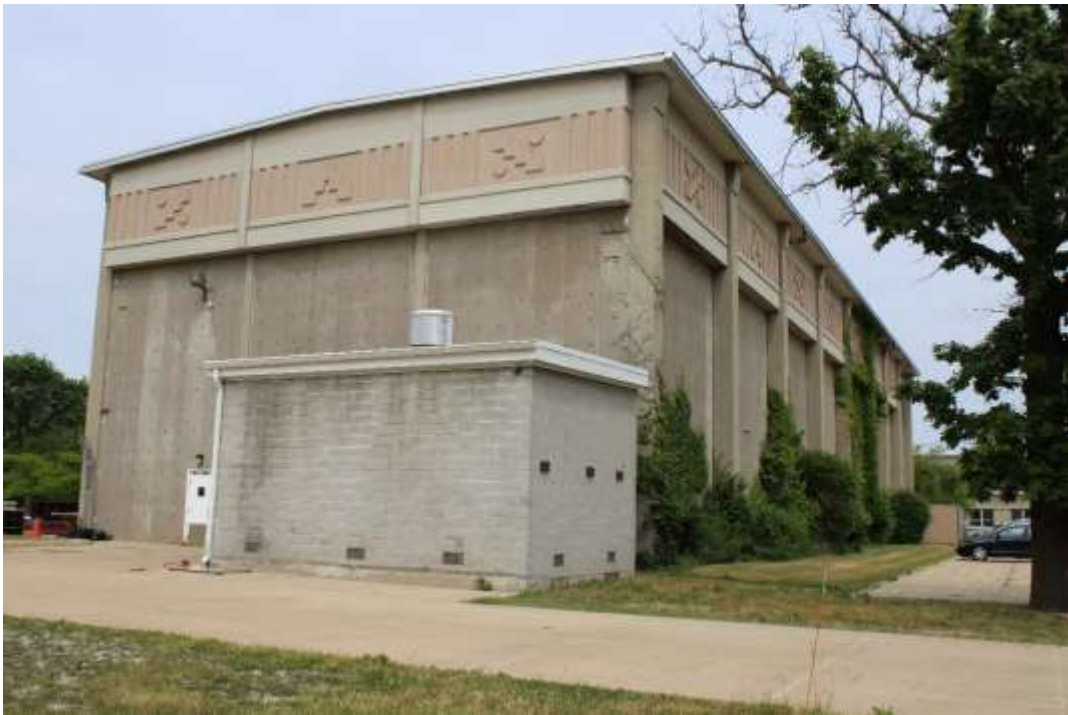
Photograph 10: West (left) and south (right) facades, view northeast.
