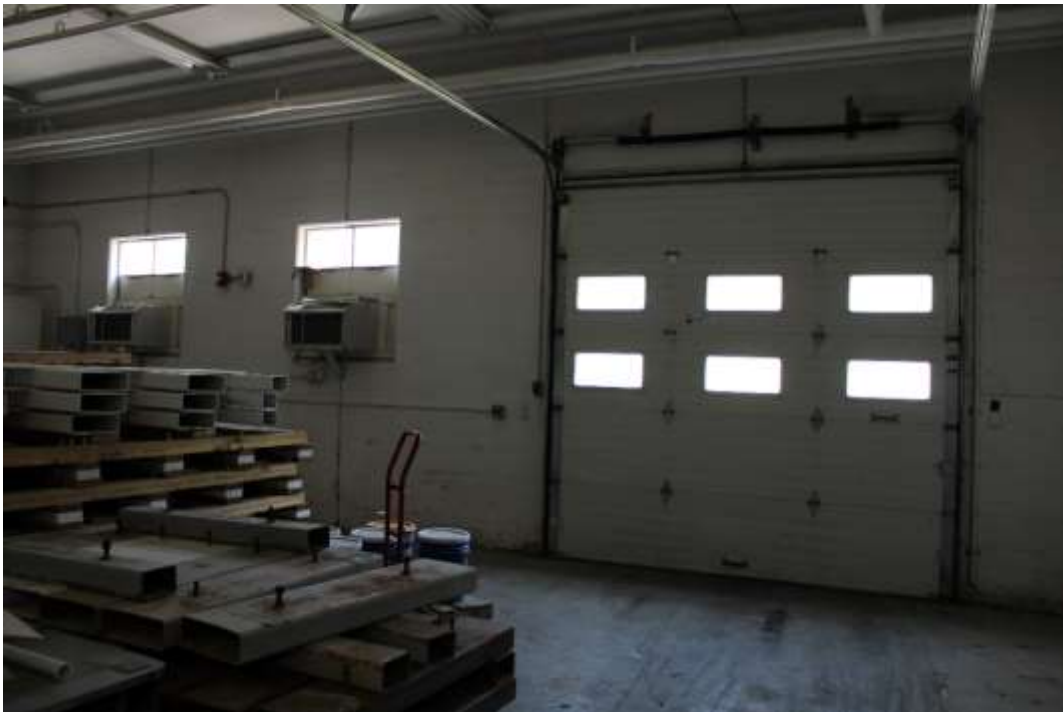
Photograph 32: Storage room, view northwest toward exterior door.
