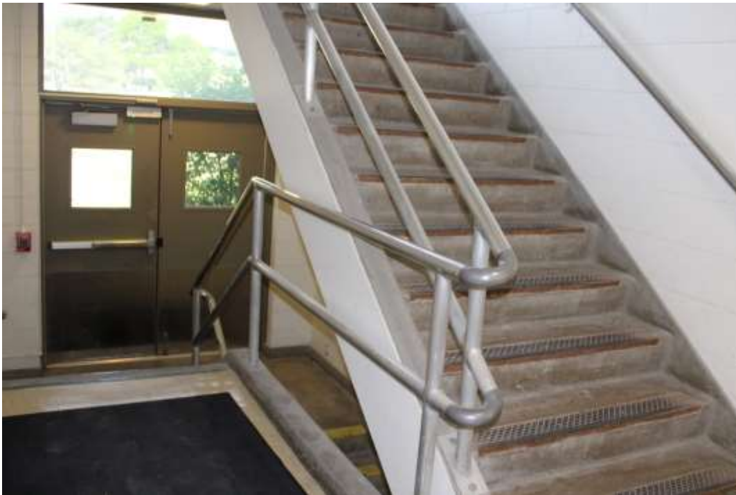
Photograph 47: West concrete stairway with metal pipe railings.
