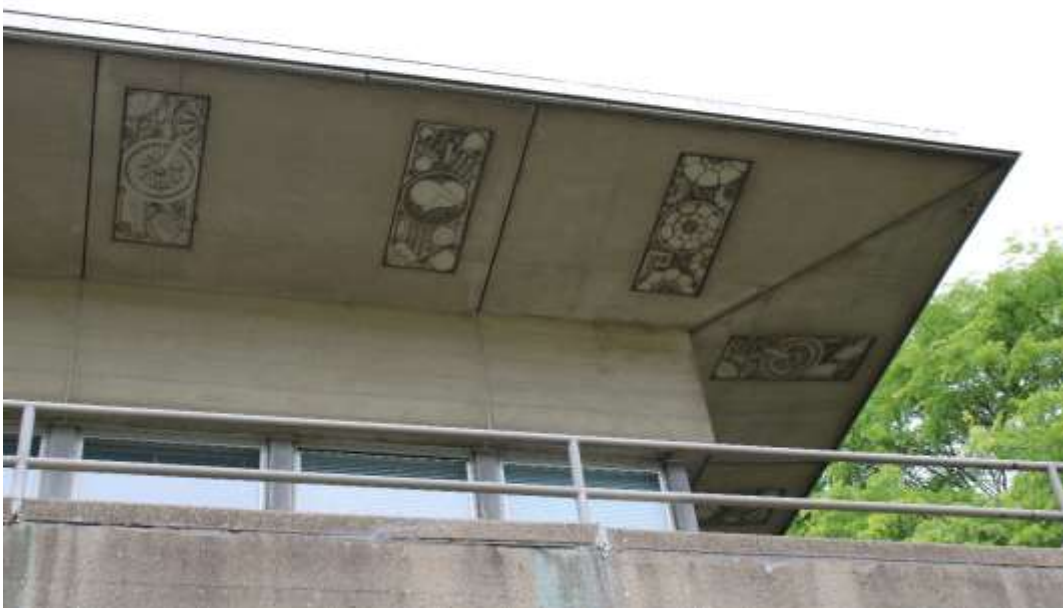
Photograph 30: Soffits with decorative concrete panels.
