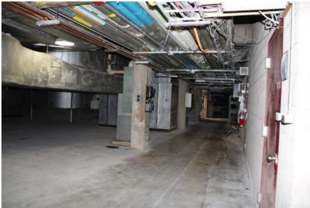
Photograph 67: Basement storage/mechanical space.
