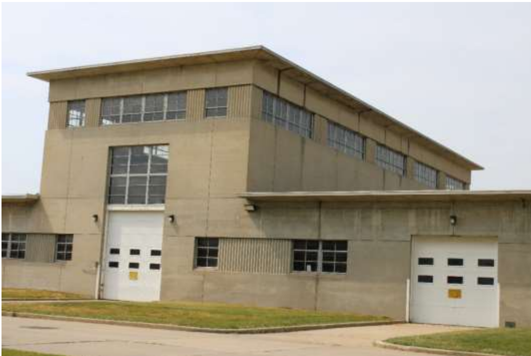
Photograph 6: South façade, detail of high bay, view northwest.
