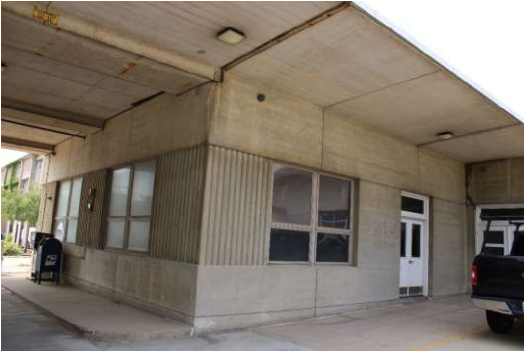
Photograph 2: South wing of building, view northwest.
