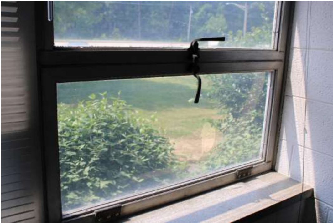
Photograph 46: Interior detail of first floor window.
