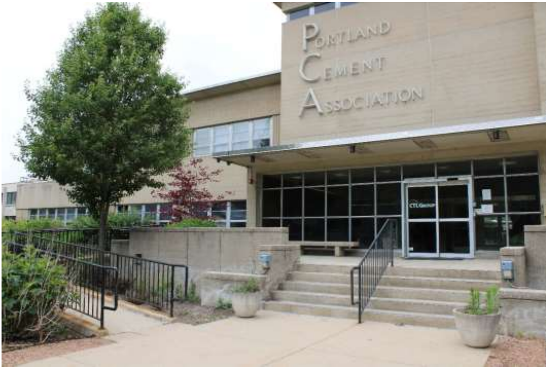
Photograph 3: Front façade, view northwest.
