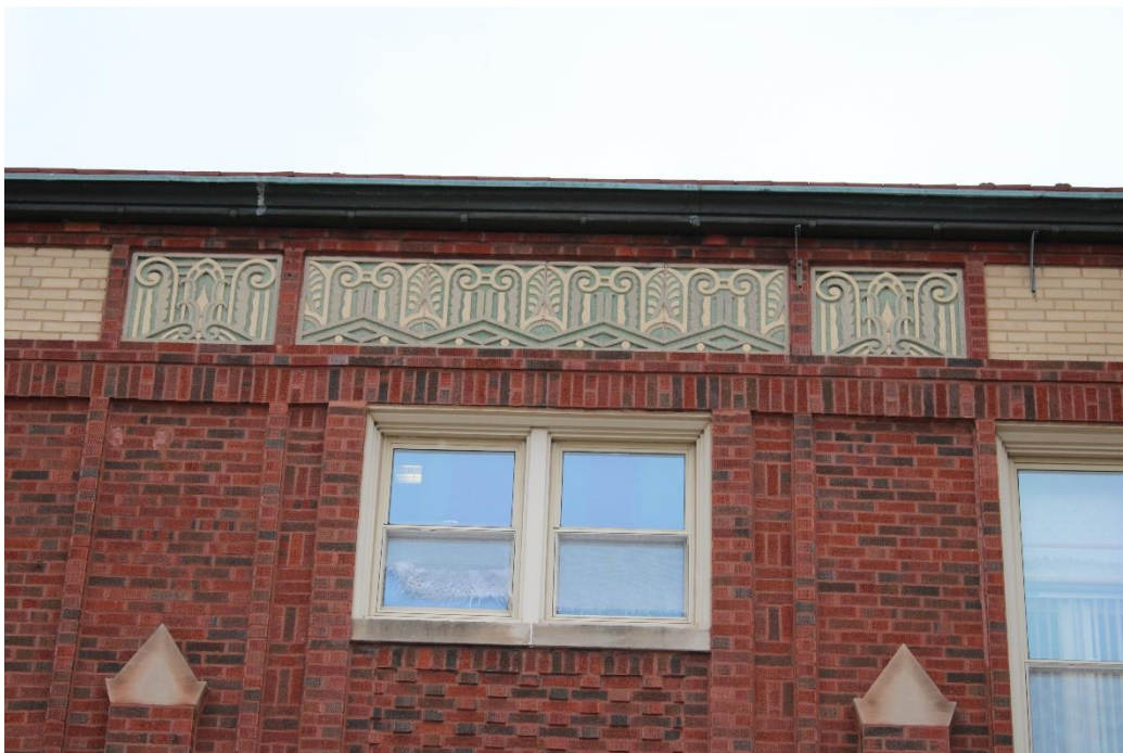
Photo 17: Terra cotta panels at parapet level of south façade, view north.
