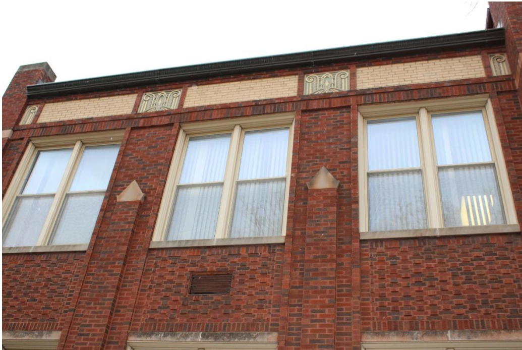
Photo 5: East façade, second floor detail, view west.
