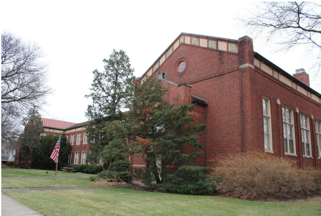
Photo 12: North (left) and west (right) facades, view southeast.
