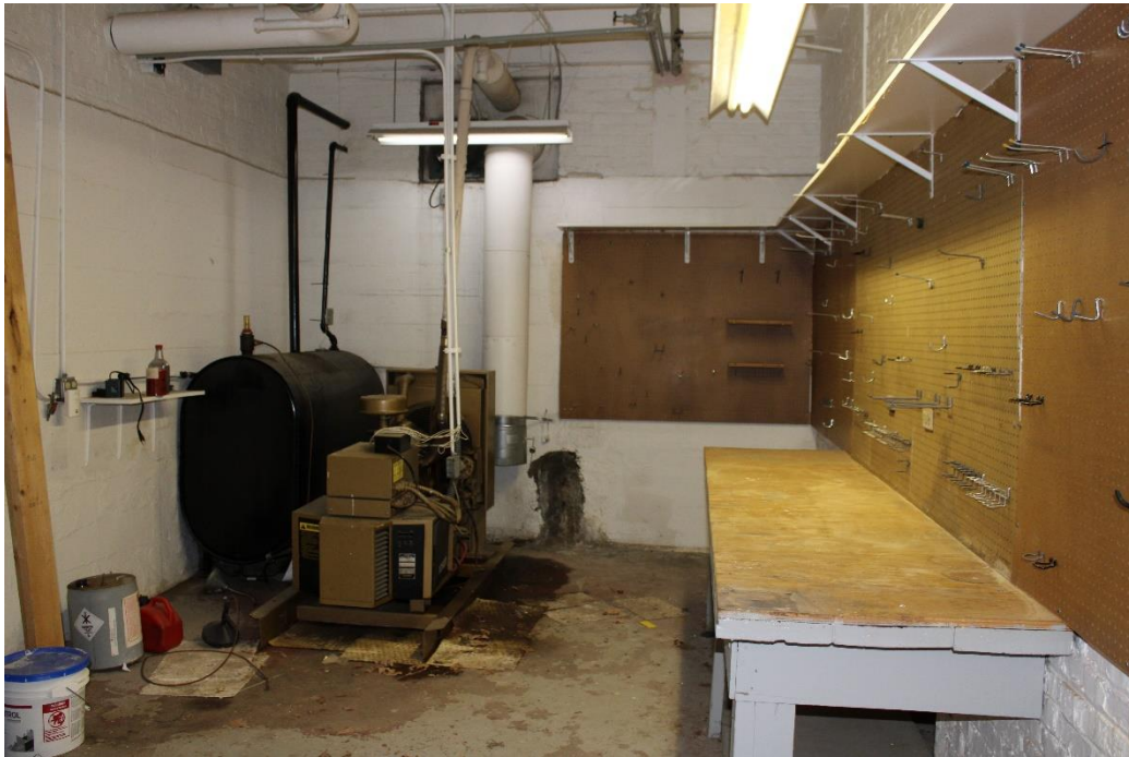
Photo 63: Basement work room.
