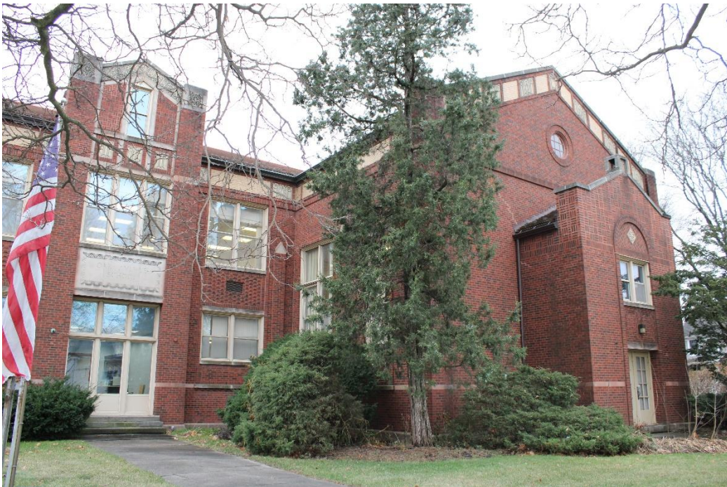
Photo 9: North façade with west wing on the right, view southwest.
