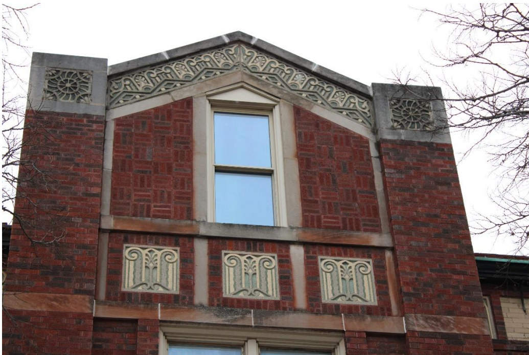
Photo 4: Upper portion of east entrance pavilion.
