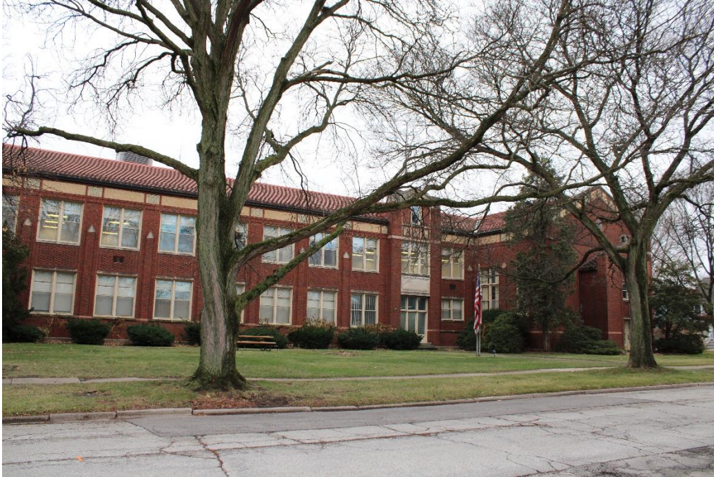
Photo 8: North façade, view southwest from Oak Avenue.
