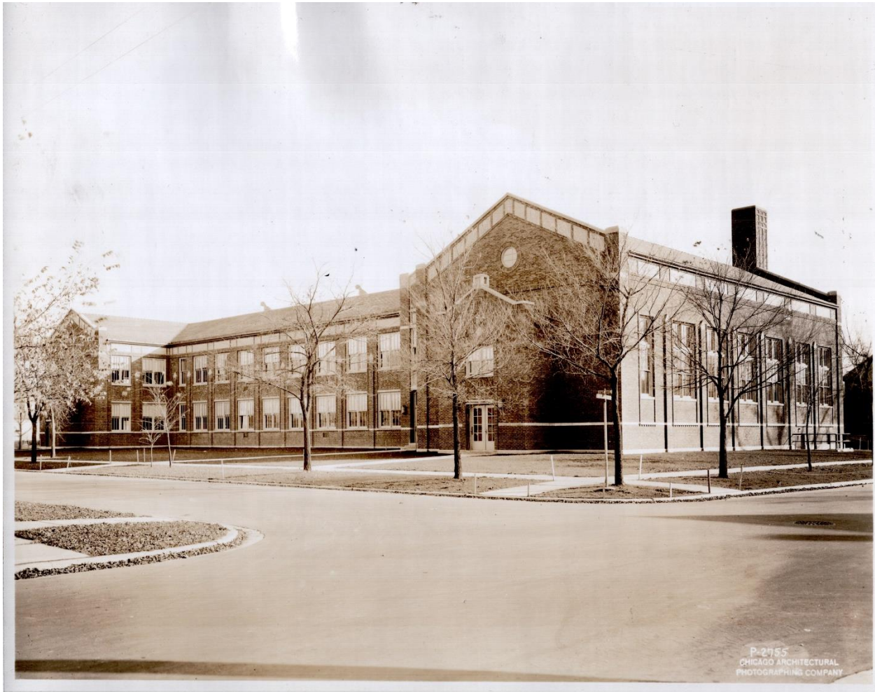
Figure 9: Oak Avenue School, 1930, view southeast, Chicago Architectural Photographing Company. Photo courtesy of the La Grange Area Historical Society.
