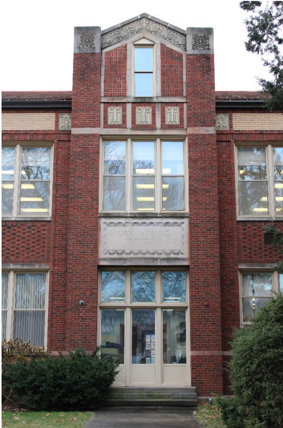
Photo 10: North façade pavilion with “OAK AVENUE SCHOOL” inscribed in concrete spandrel panel above a group of windows that replaced an original entrance, view south.
