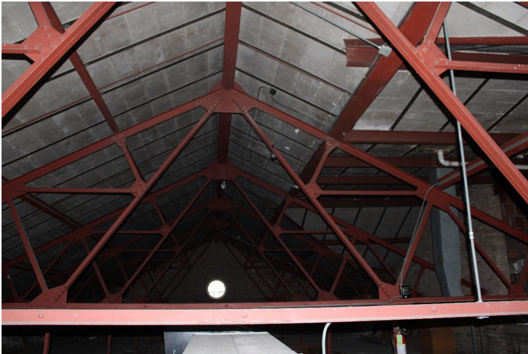
Photo 59: West wing's attic ceiling with steel trusses, view north.
