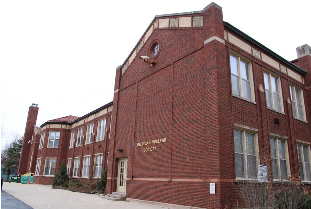
Photo 19: South (left) and east (right) facades, view northwest.
