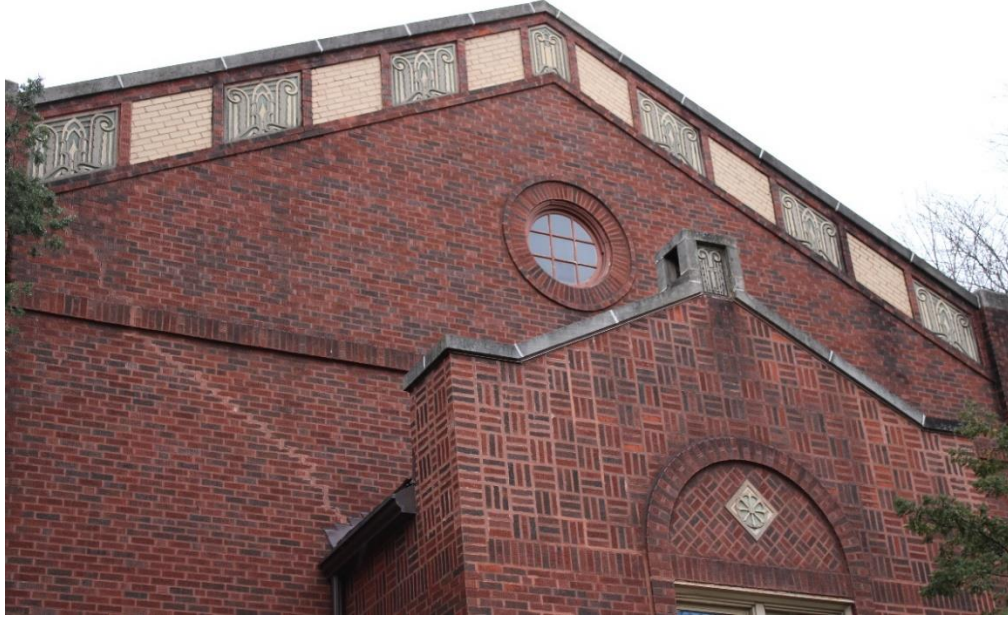
Photo 11: Detail of decorative brickwork and terra cotta panels on the north façade of the west wing, view southwest.
