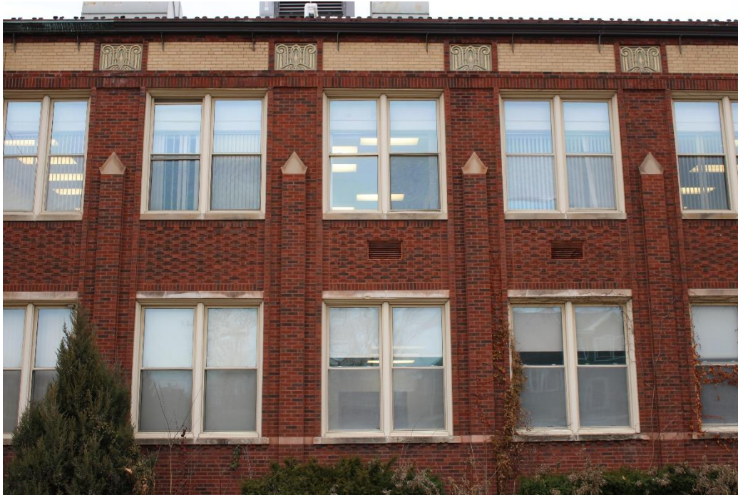
Photo 18: Detail of south façade window bays.
