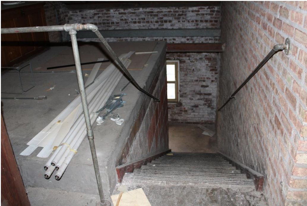
Photo 57: Upper portion of west stairwell leading to attic.
