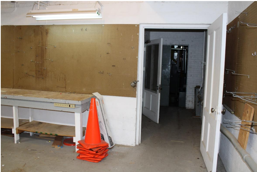
Photo 62: Basement work room.
