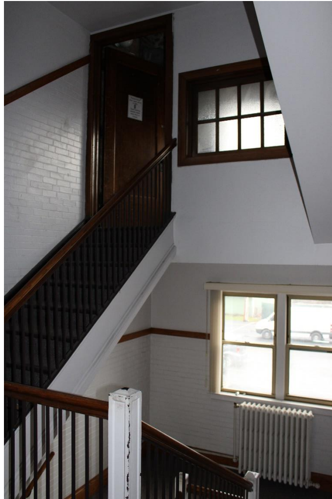
Photo 56: West stairwell showing door to attic level.
