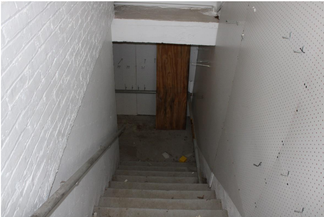
Photo 60: Portion of west wing stairwell leading to basement.
