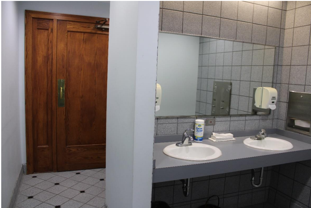
Photo 34: Representative remodeled bathroom.
