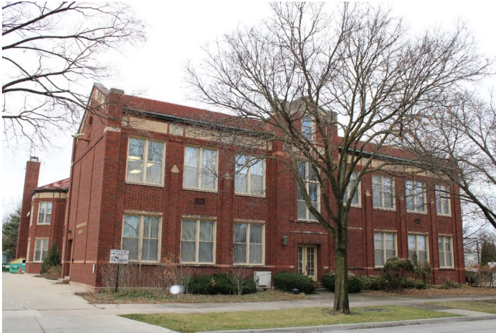
Photo 1: East façade of east wing, view northwest.
