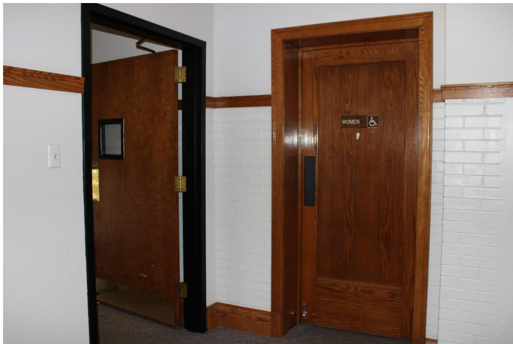
Photo 55: Door to west stairwell (left) and Women's Restroom (right), second floor.
