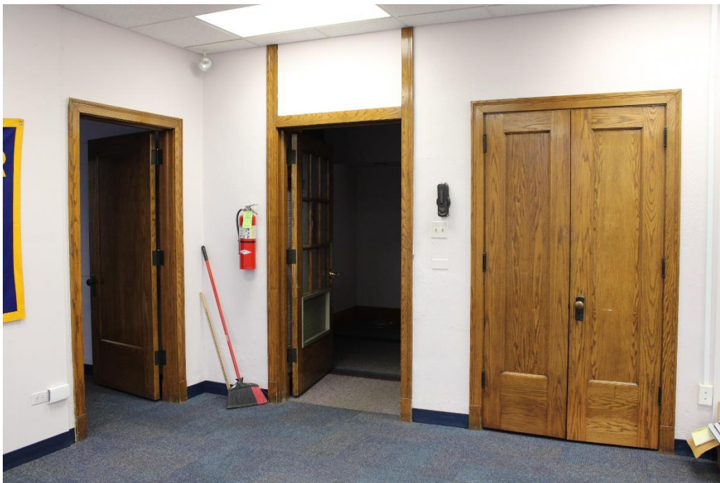
Photo 51: Original closet and wood doors/trim, in former second-floor classroom.
