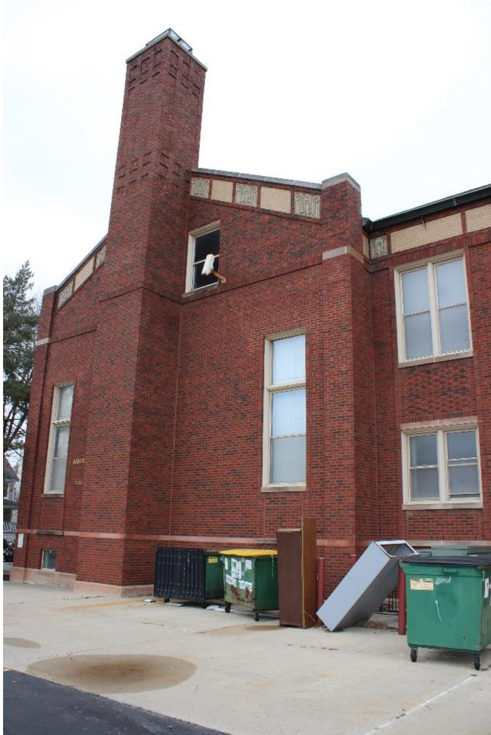
Photo 15: Exterior chimney on west wing's south façade, view northwest.
