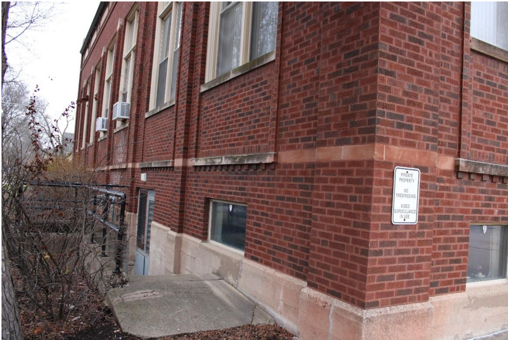
Photo 14: West façade detail showing basement entrance.
