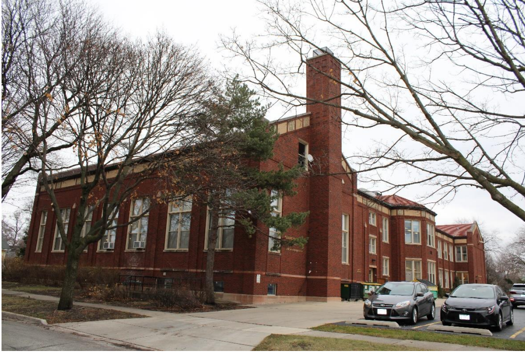
Photo 13: West (left) and south (right) facades, view northeast.
