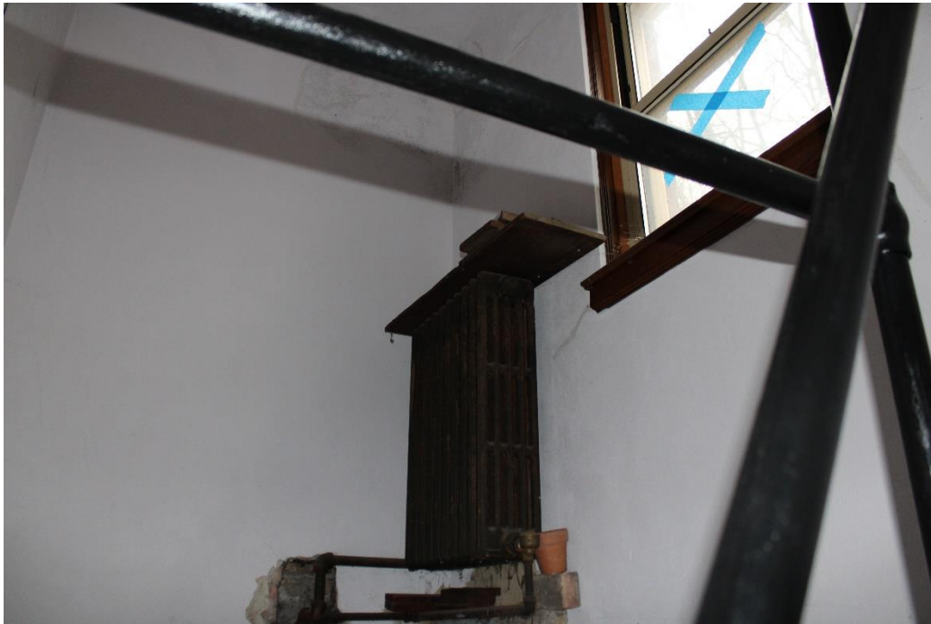
Photo 38: Original projection booth for the auditorium, which is situated above the east wing's north entrance vestibule.
