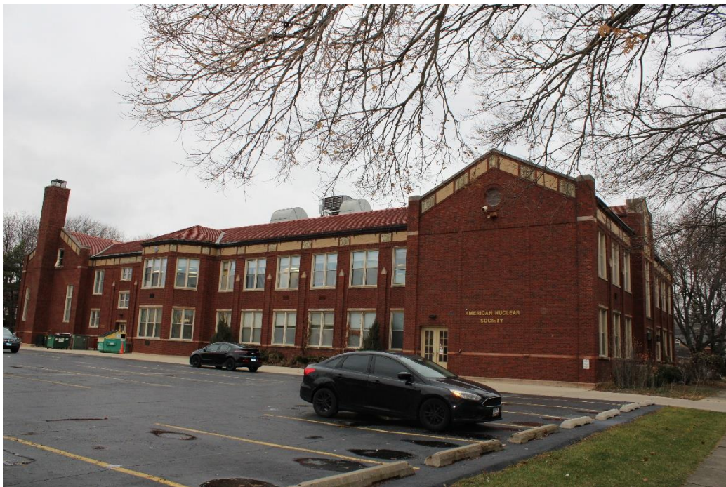
Photo 21: South (left) and east (right) facades, view northwest.
