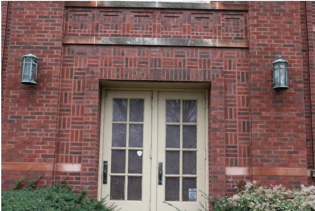
Photo 3: East portal with original doors, basketweave brickwork, and light sconces.
