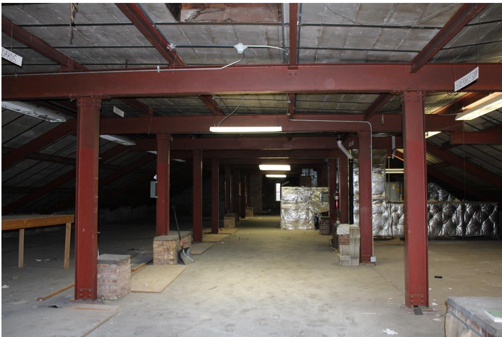
Photo 58: Attic level above main block.
