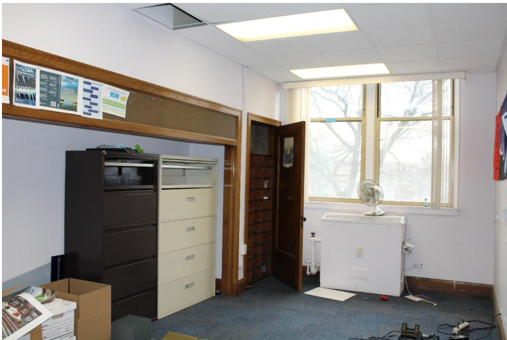
Photo 49: Portion of second-floor classroom converted to office space.
