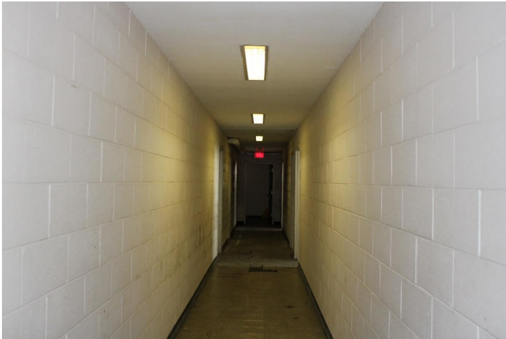
Figure 52: Corridor on lower level, view south.
