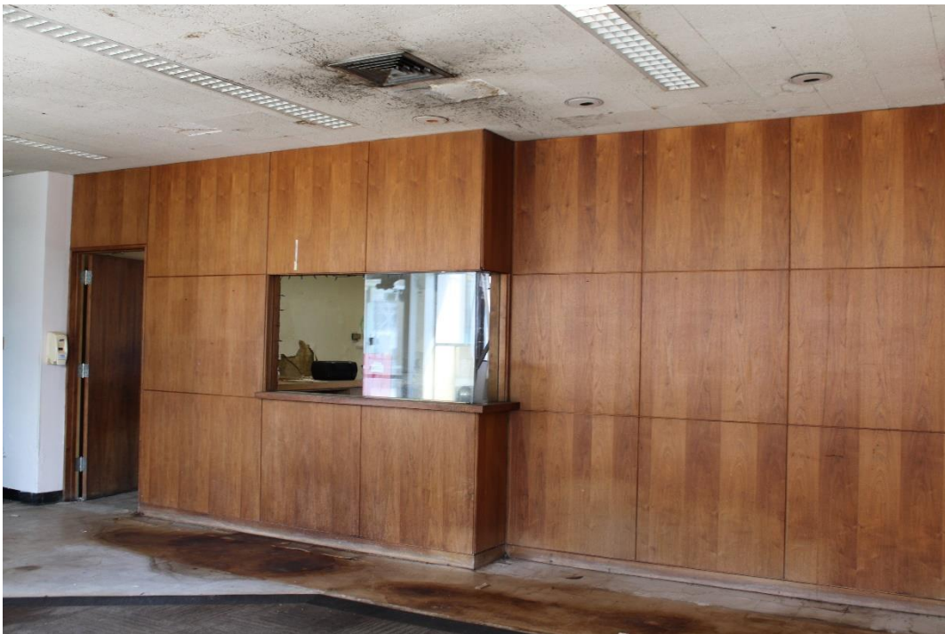
Figure 25: Teakwood paneled wall of main lobby.
