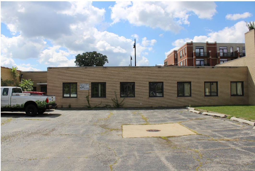
Figure 19: North façade of the Madison Street wing, view south.
