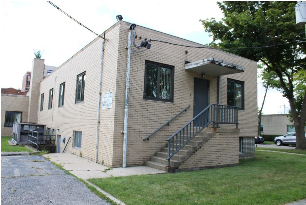
Figure 16: Rear door on west wing, view southwest.
