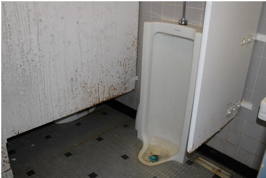
Figure 45: Men's restroom on lower level.
