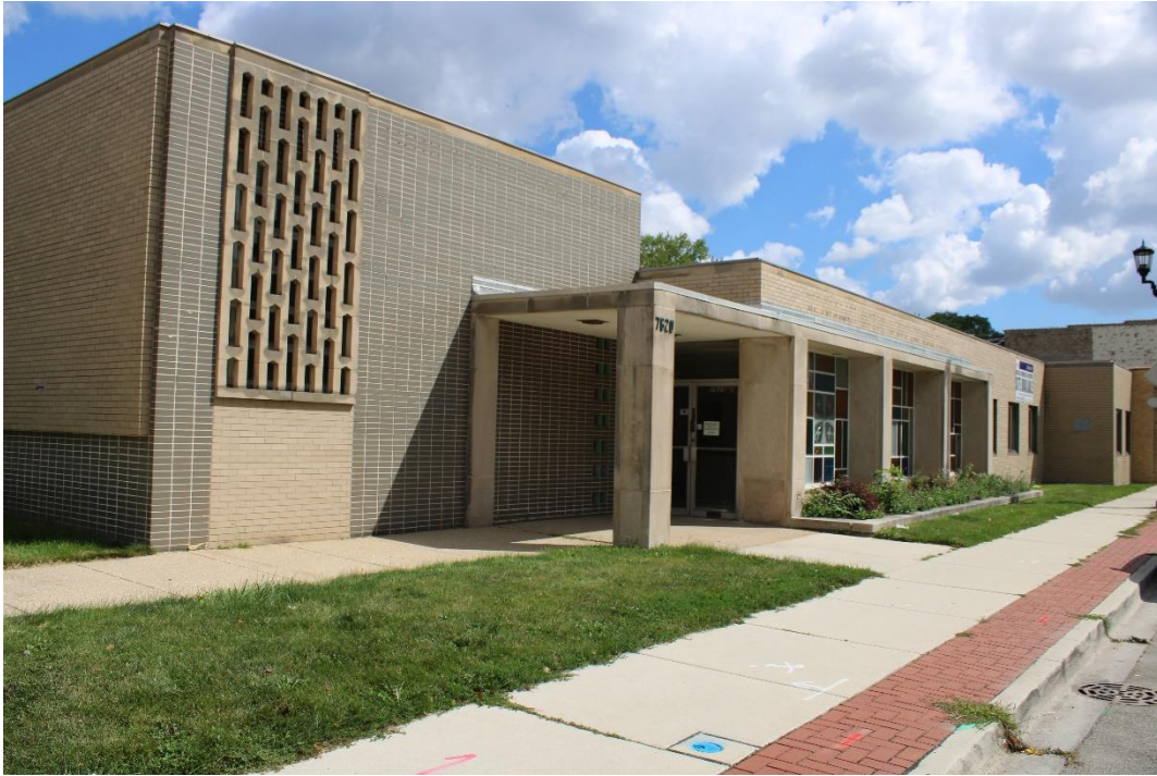
Figure 10: Front façade, view northeast.
