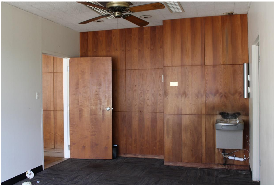
Figure 29: Secondary lobby with teakwood-paneled wall, view north.
