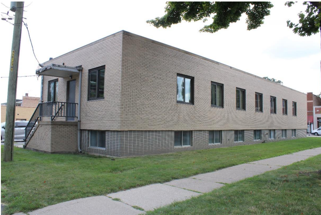
Figure 15: West façade, view southeast.
