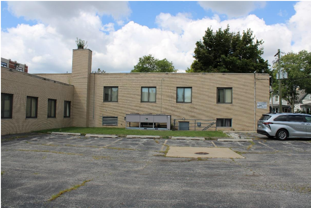
Figure 18: East façade of west wing, view west.
