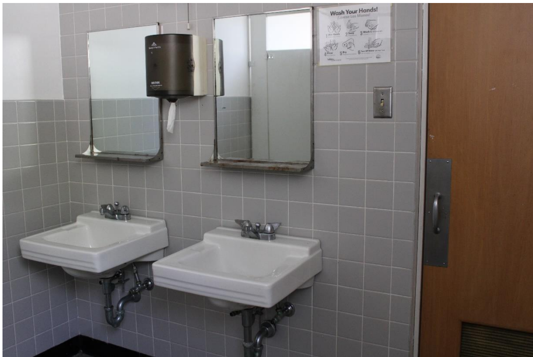
Figure 43: Women's restroom on lower level.
