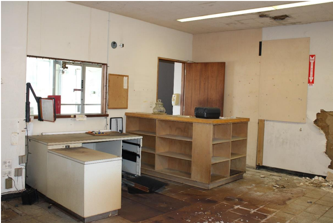
Figure 26: Administrative office off the lobby.
