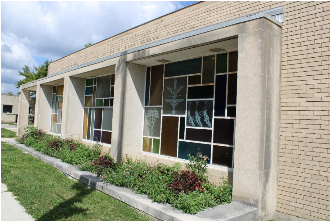
Figure 6: Front façade detail, view northwest.
