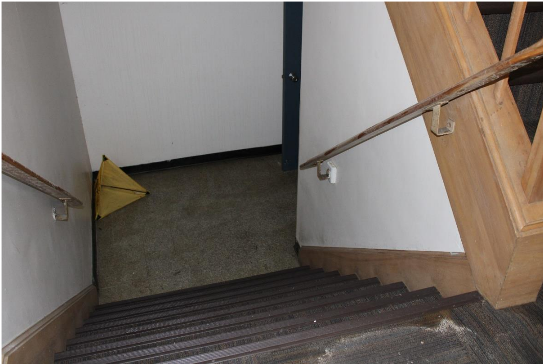
Figure 40: Stairway to lower level.
