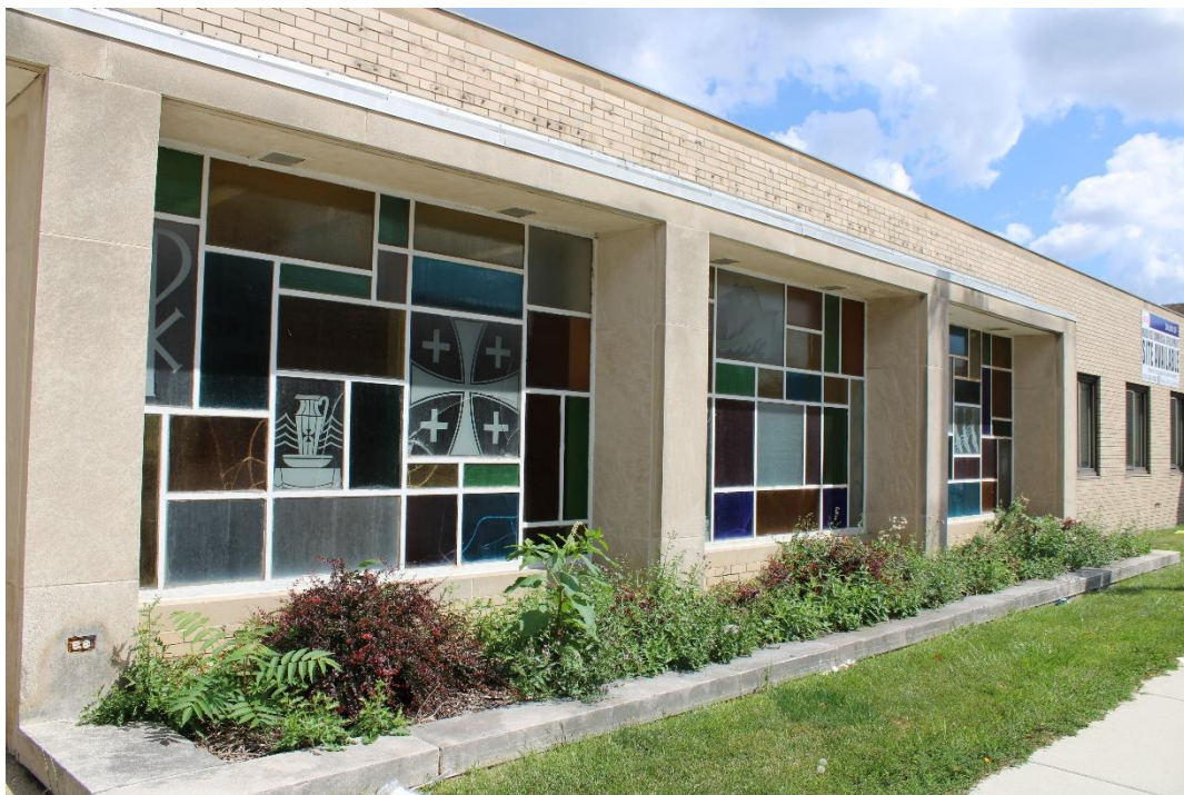
Figure 9: Front façade, stained glass window bays, view northeast.
