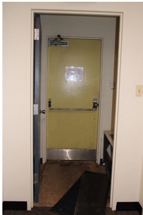
Figure 61: Exit at the north end of the upper level.
