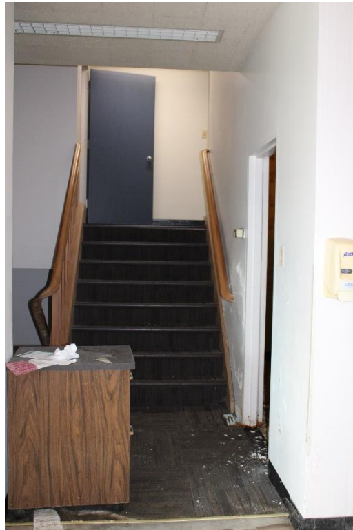
Figure 38: Staircase to upper level with door to women’s restroom on right.
