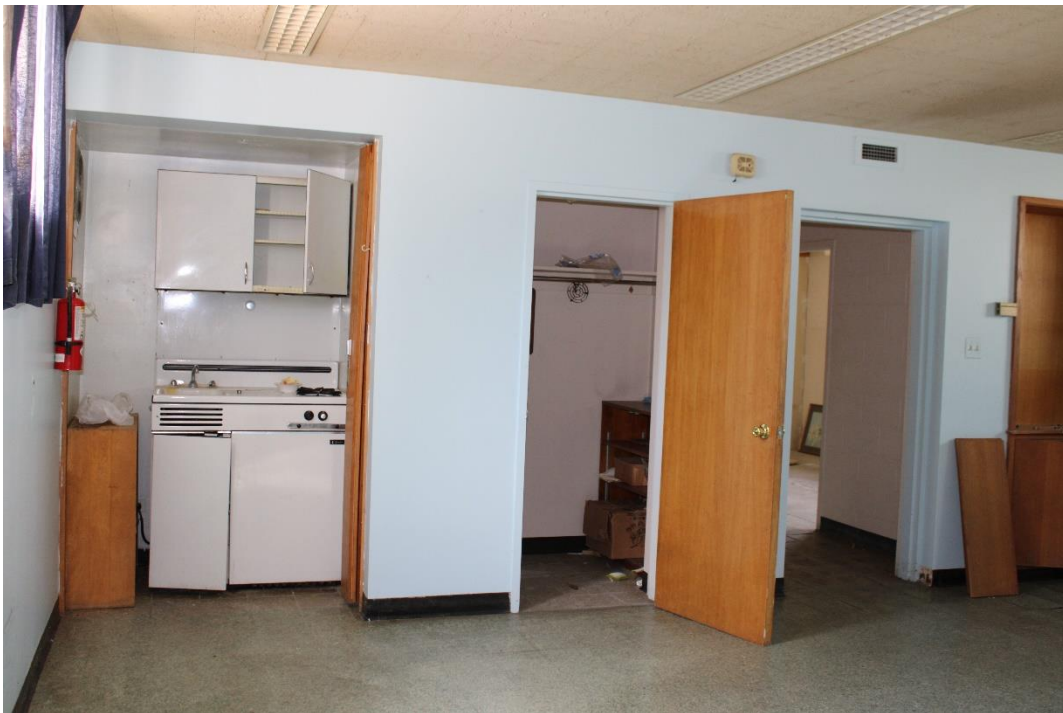
Figure 51: Meeting room on lower level showing original metal kitchenette.
