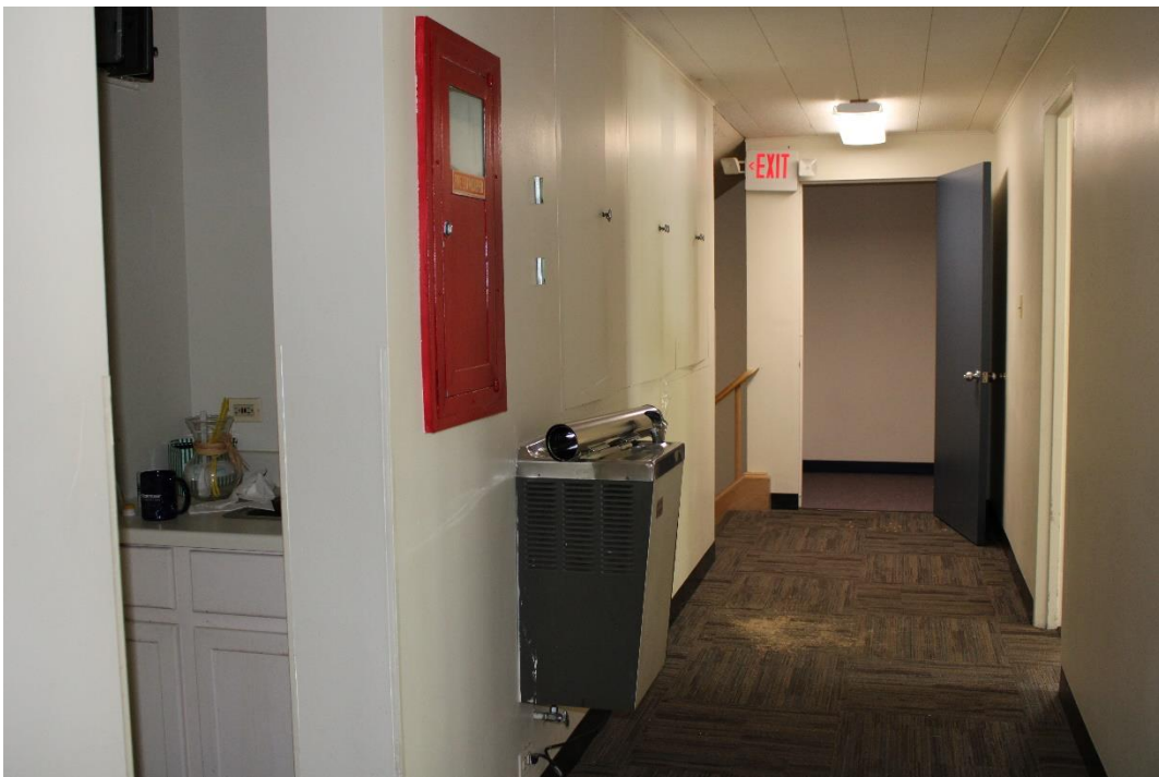
Figure 63: Corridor on the upper level, view south.
