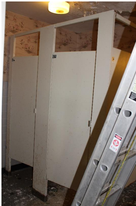
Figure 39: First floor women’s restroom.
