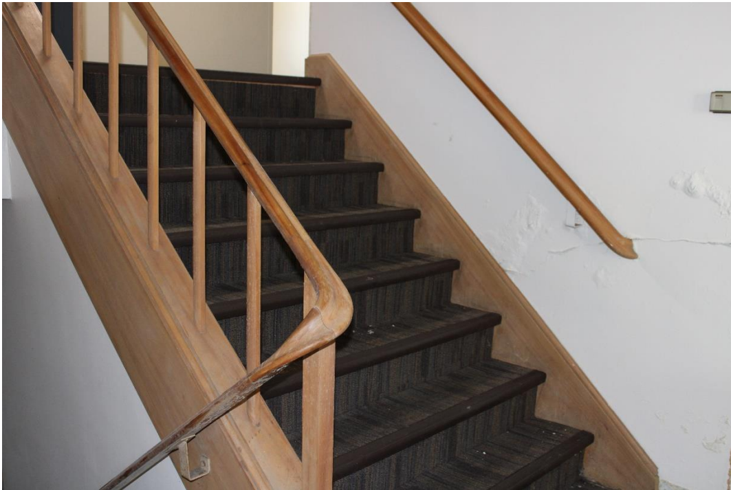
Figure 54: Stairway from first floor to upper level.
