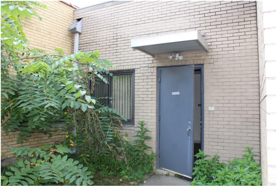
Figure 20: Rear entrance to Madison Street wing.
