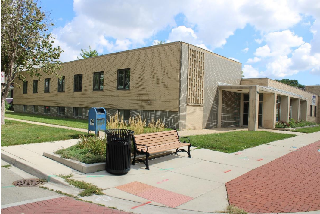
Figure 14: Front (south) and west facades, view northeast.
