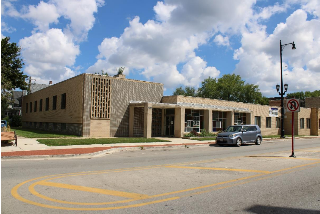
Figure 4: Front façade, view northeast.
