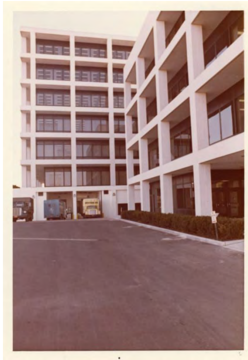
Figure 68: Rear view of G building, 1975, view east. Source: Allstate Corporate Archive.
