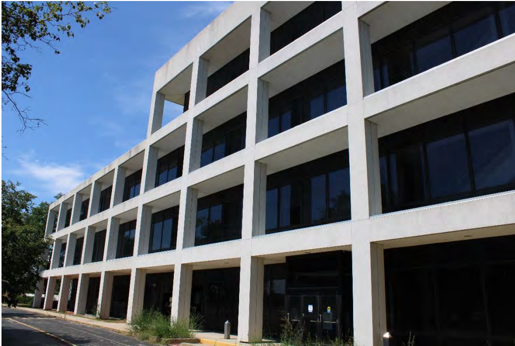
Figure 13: South Plaza Complex, rear section of G building showing its 1992 addition on the left, view northwest.
