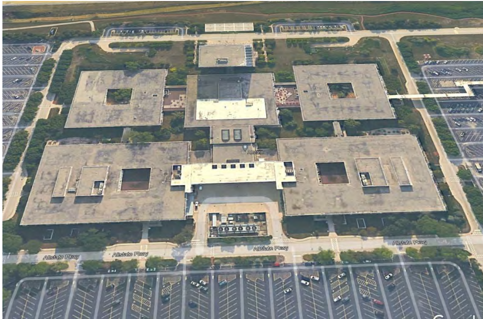
Figure 1: Aerial view of the North Plaza Complex, view east. Source: Google Earth.
