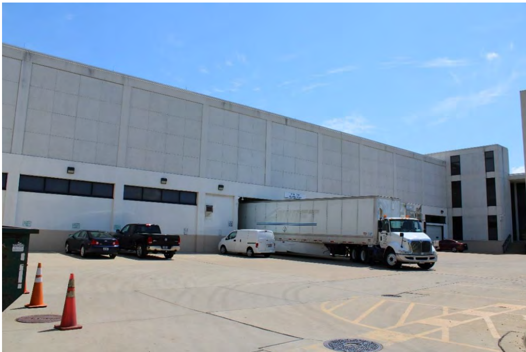
Figure 14: North Plaza Complex, C building loading dock, view southeast.
