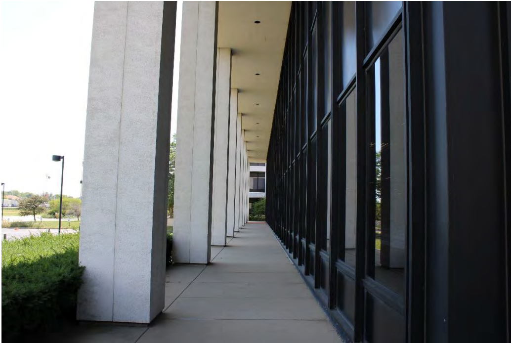
Figure 21: South Plaza Complex, portico of I building, view south.
