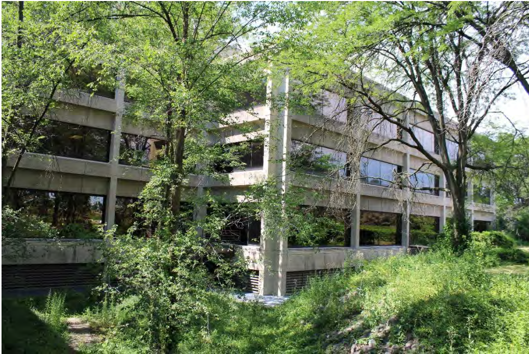
Figure 13: Willow (aka Nielsen) Plaza Building, view of Y (left) and X wings, view northwest.
