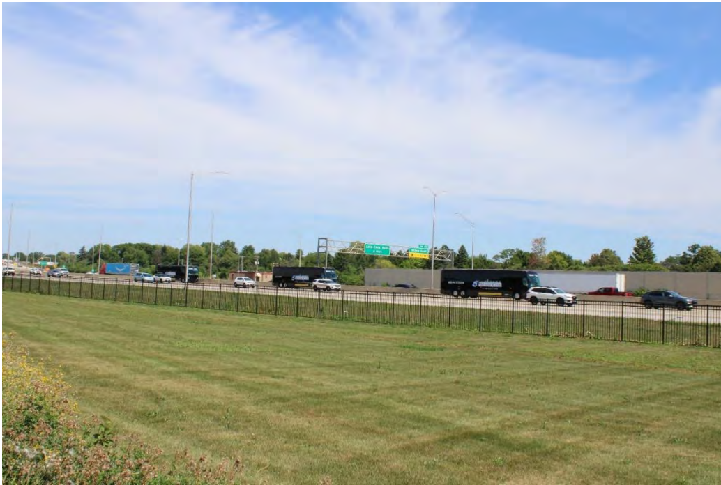
Figure 16: I-294 Tollway as seen from Allstate campus, view northeast, August 2022.
