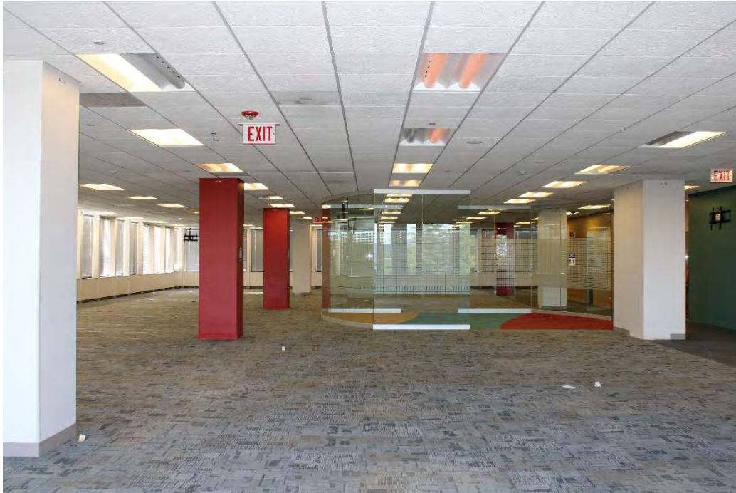
Figure 29: North Plaza Complex, fourth floor of F building showing typical open plan.
