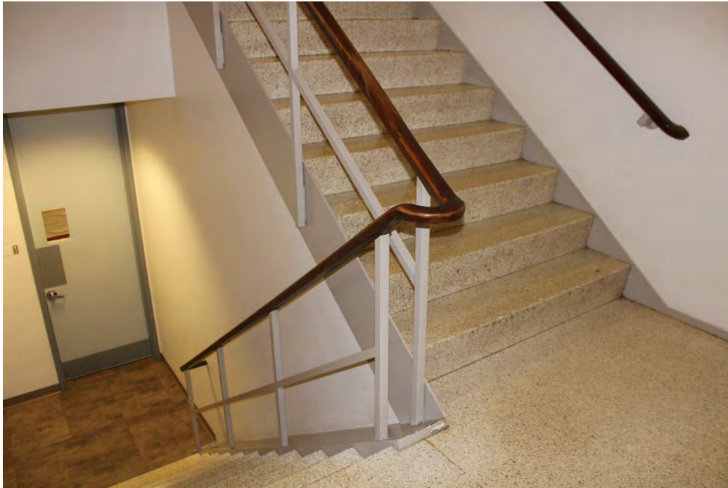
Figure 41: North Plaza Complex, typical stairway
