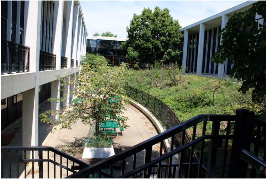
Figure 19: North Plaza Complex, courtyard between B building (left) and A building (right), view north.
