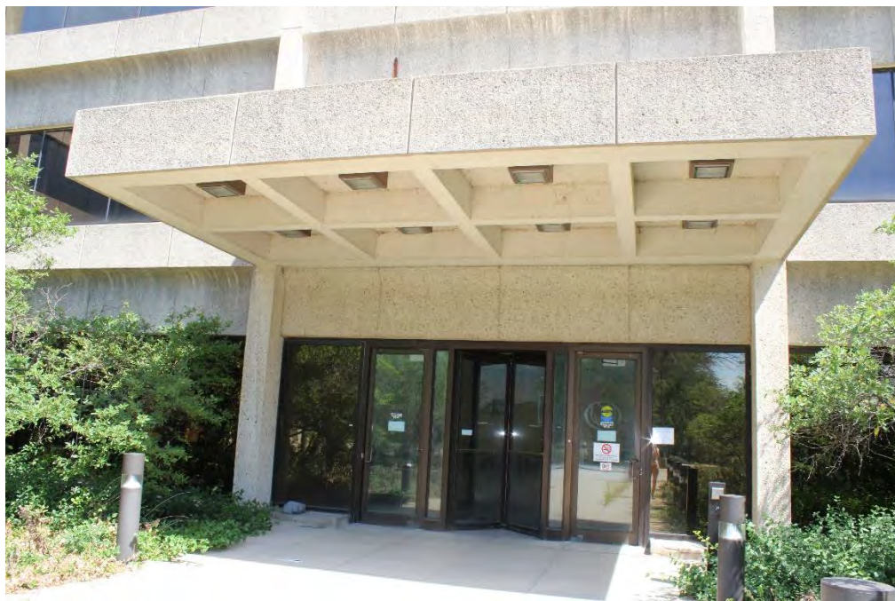
Figure 4: Willow (aka Nielsen) Plaza Building, main entrance on W wing with concrete coffered canopy, view northeast.
