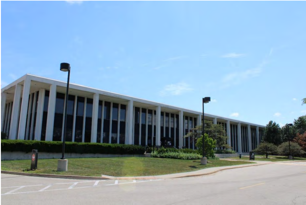
Figure 15: North Plaza Complex, B building, view northeast.
