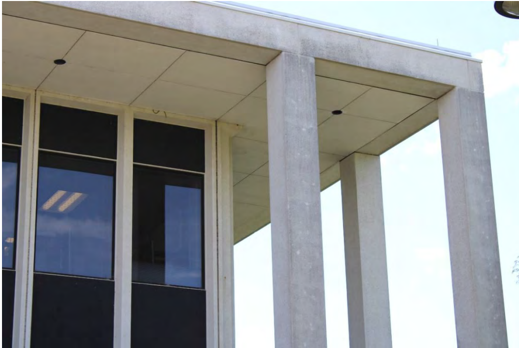
Figure 13: North Plaza Complex, D building detail.
