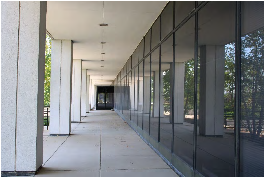
Figure 3: South Plaza Complex, G building portico, view south.
