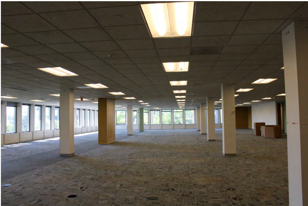
Figure 36: North Plaza Complex, 2 nd floor of E building showing typical open plan.
