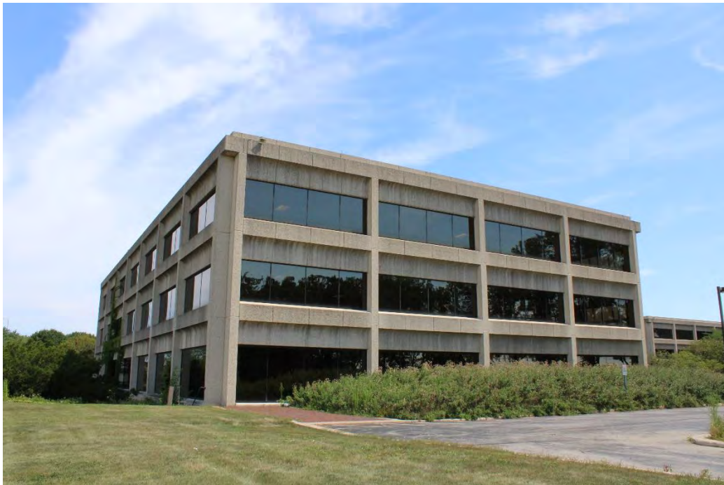
Figure 2: Willow (aka Nielsen) Plaza Building, U wing, view southeast.
