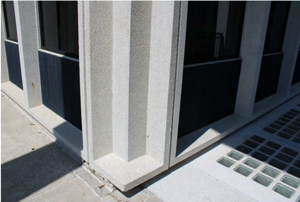
Figure 17: North Plaza Complex, B building corner detail.
