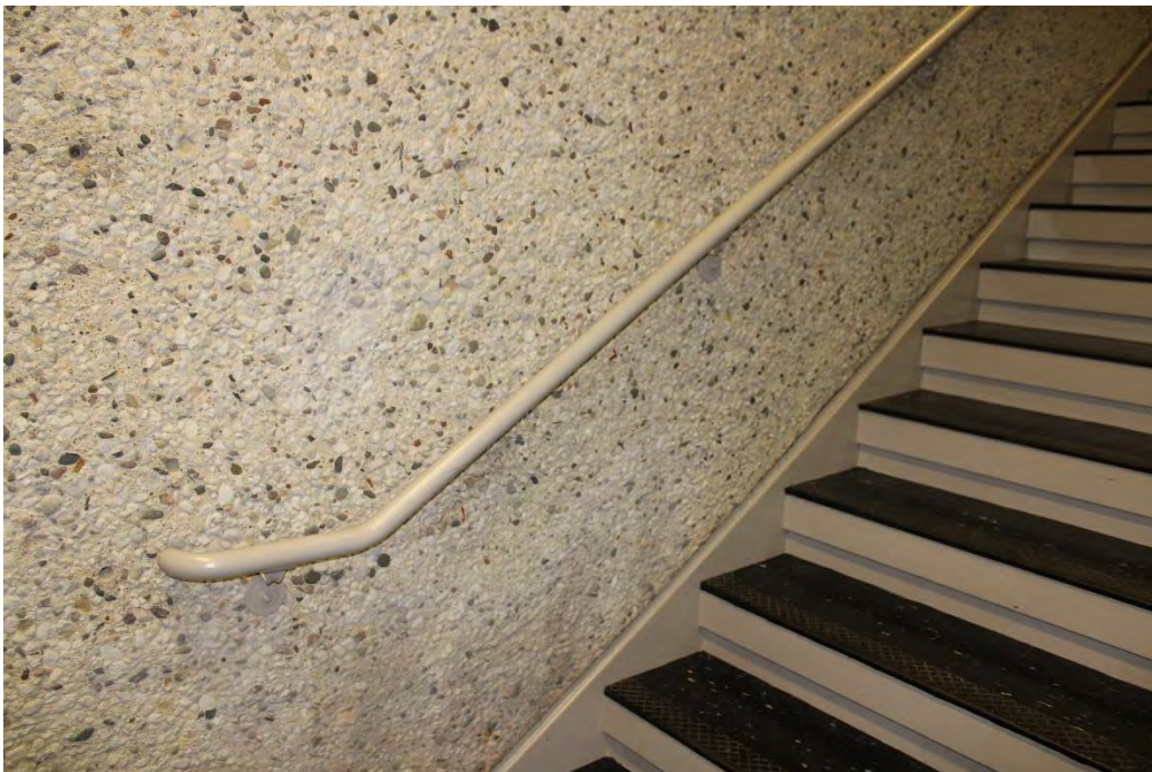
Figure 30: Willow (aka Nielsen) Plaza Building, wall detail showing concrete aggregate in stairwell.
