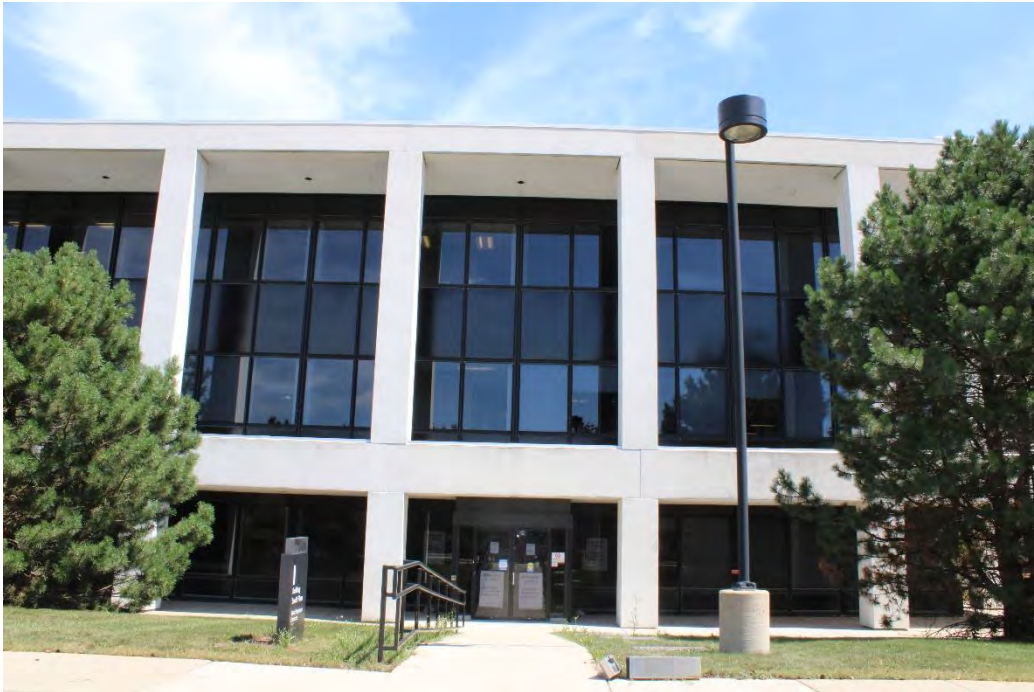
Figure 17: South Plaza Complex, entrance to I building, view east.
