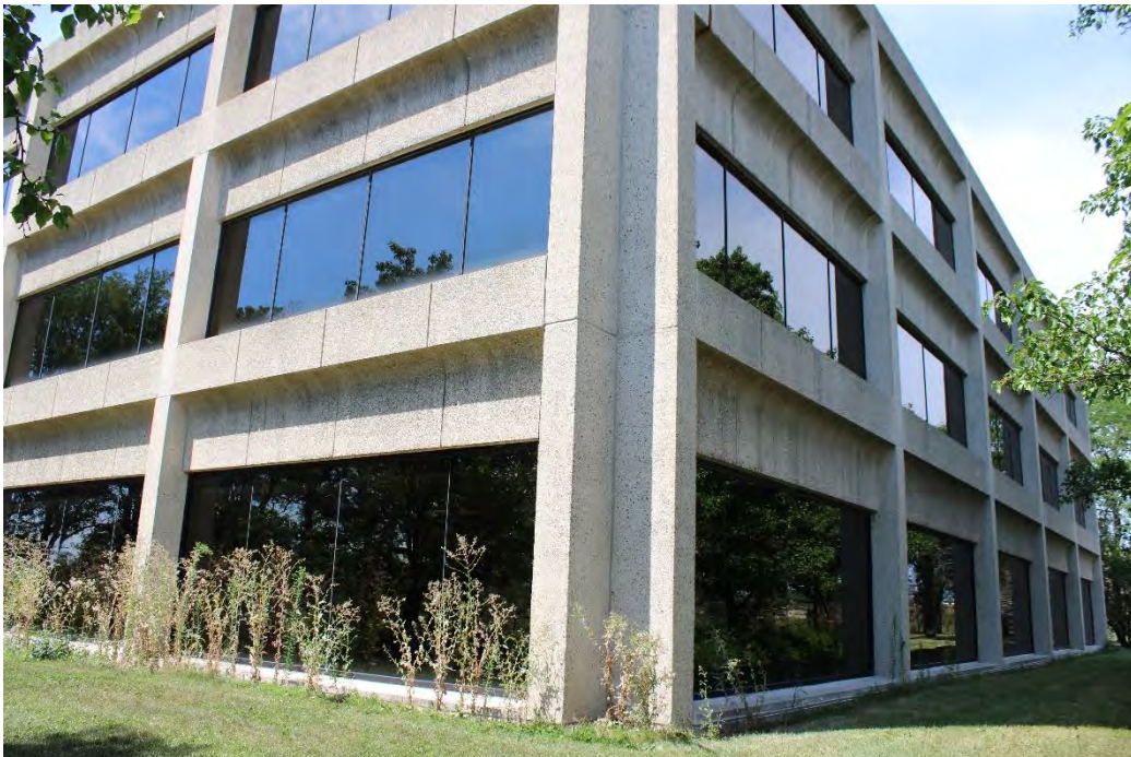
Figure 12: Willow (aka Nielsen) Plaza Building, corner of Z wing, view northwest.
