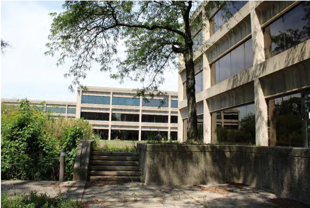
Figure 9: Willow (aka Nielsen) Plaza Building, view north.
