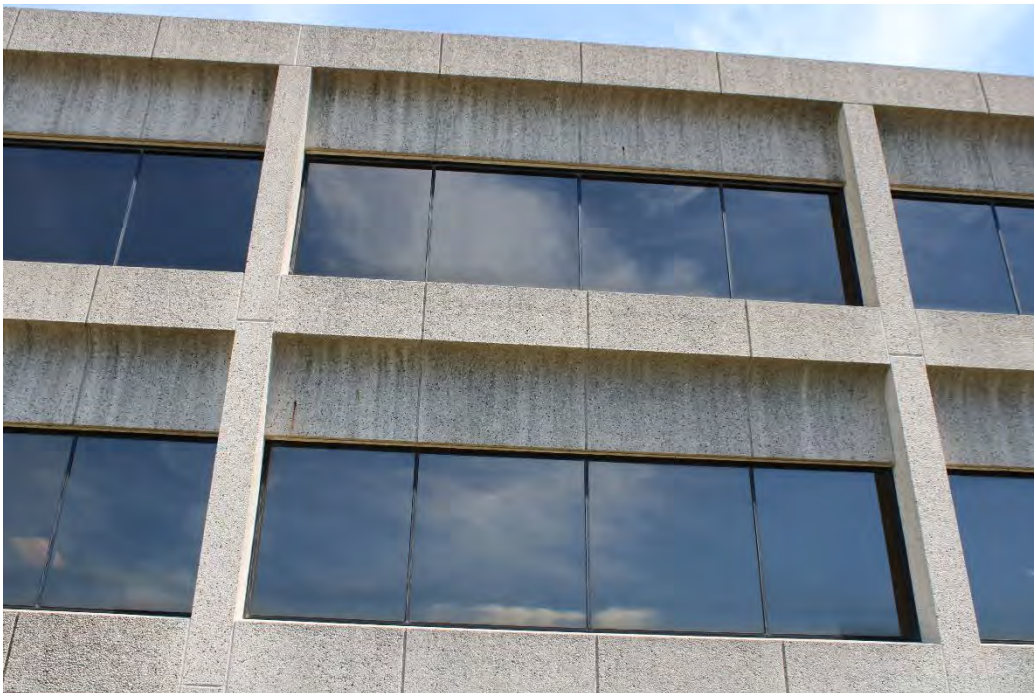
Figure 6: Willow (aka Nielsen) Plaza Building, detail of precast concrete panels.
