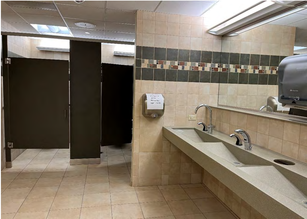
Figure 37: Willow (aka Nielsen) Plaza Building, third floor women's restroom.
