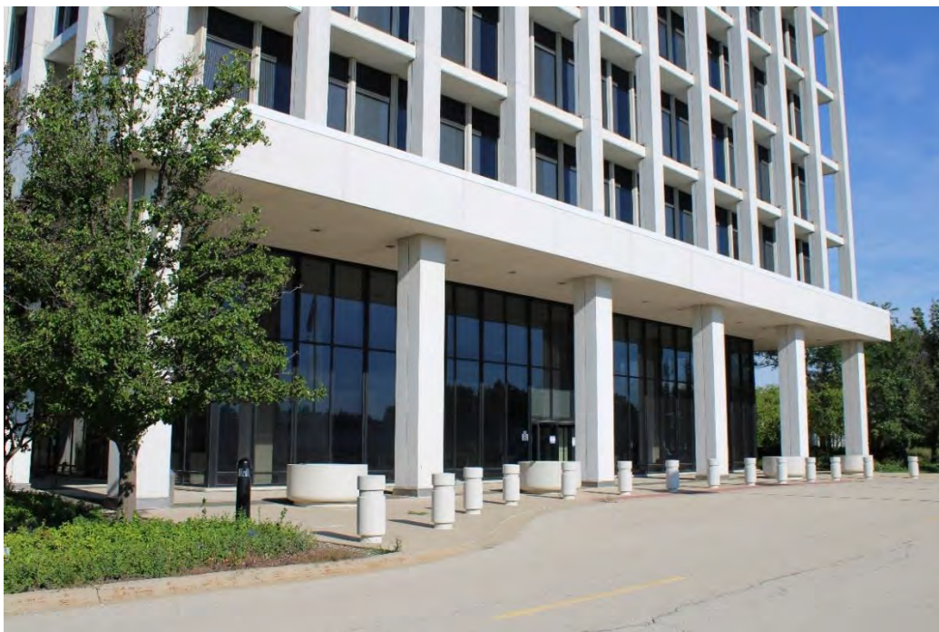
Figure 4: North Plaza Complex, F building's front façade, view northwest.
