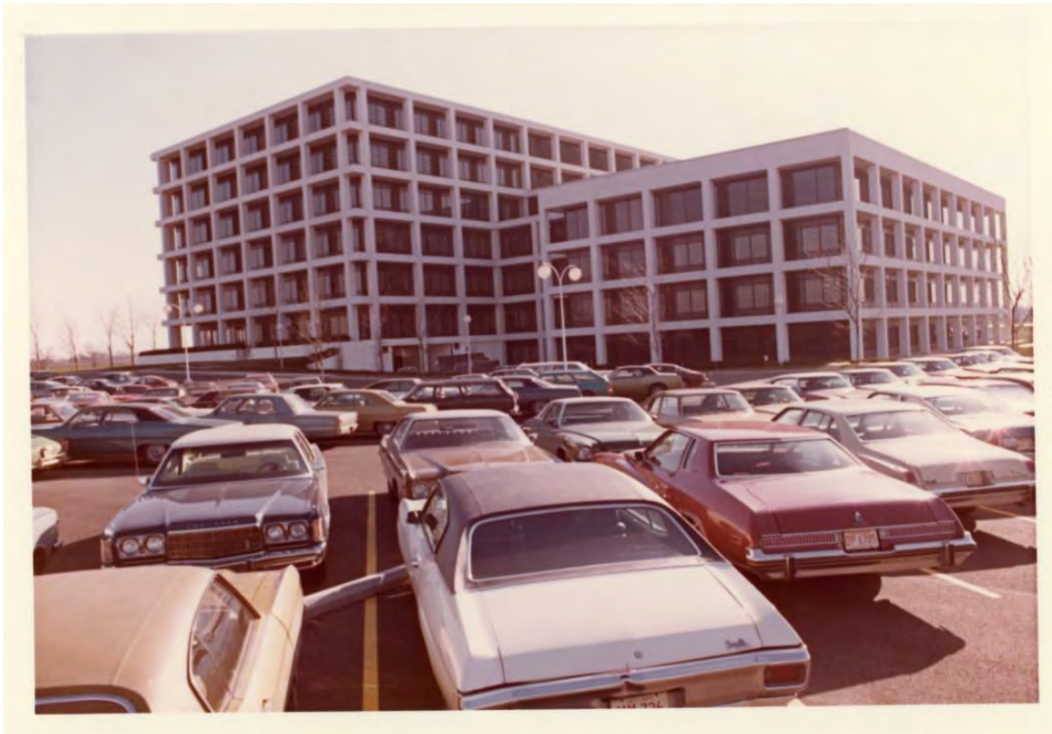
Figure 67: G building, 1975, view southeast. Source: Allstate Corporate Archive.
