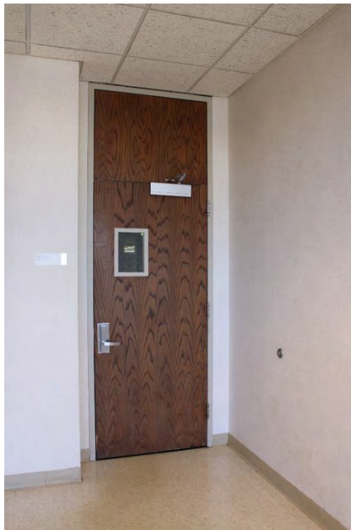
Figure 34: Typical interior door in South Plaza Complex.
