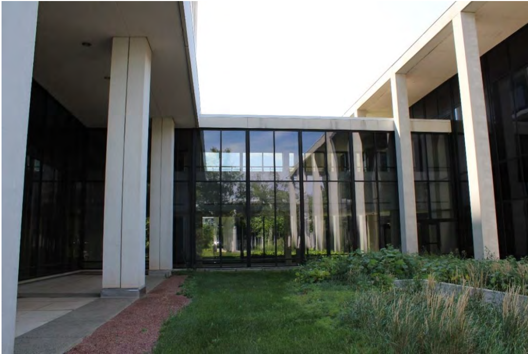
Figure 9: North Plaza Complex, link between F (left) and C (right) buildings.
