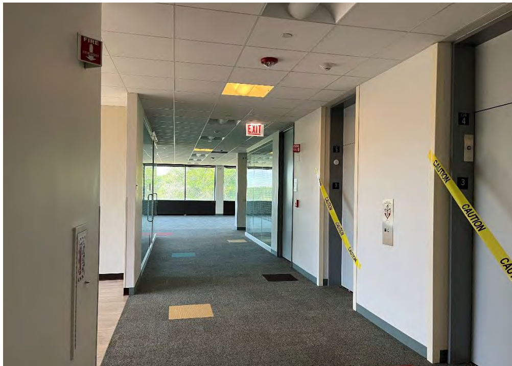
Figure 36: Willow (aka Nielsen) Plaza Building, third floor elevator bank.
