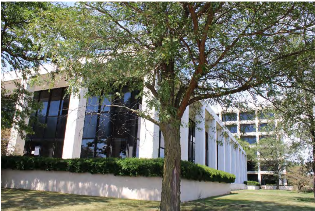
Figure 8: South Plaza Complex, H building (foreground) and G building (background), view northwest.
