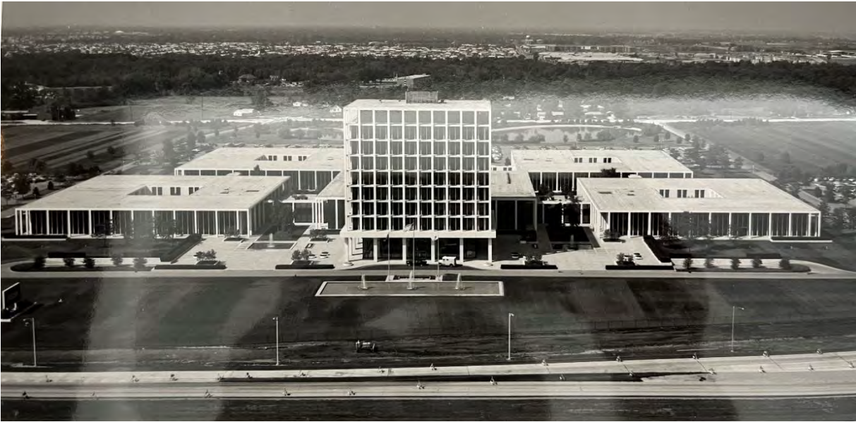
Figure 66: North Plaza Complex, view west. Photographer: Hedrich Blessing. Source: Chicago History Museum.
