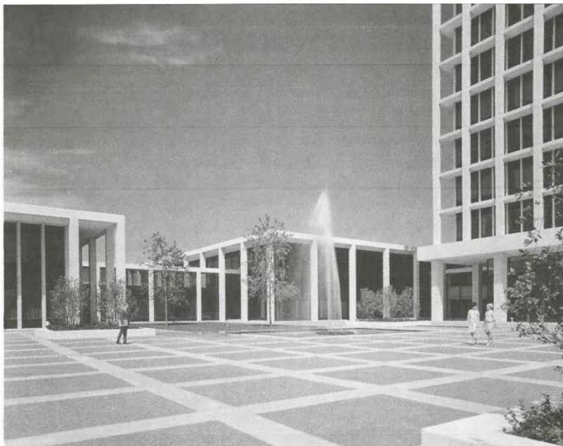
Figure 37: North Plaza courtyard with reflecting pool and fountain. Photo courtesy of the Allstate Corporation Archive.
