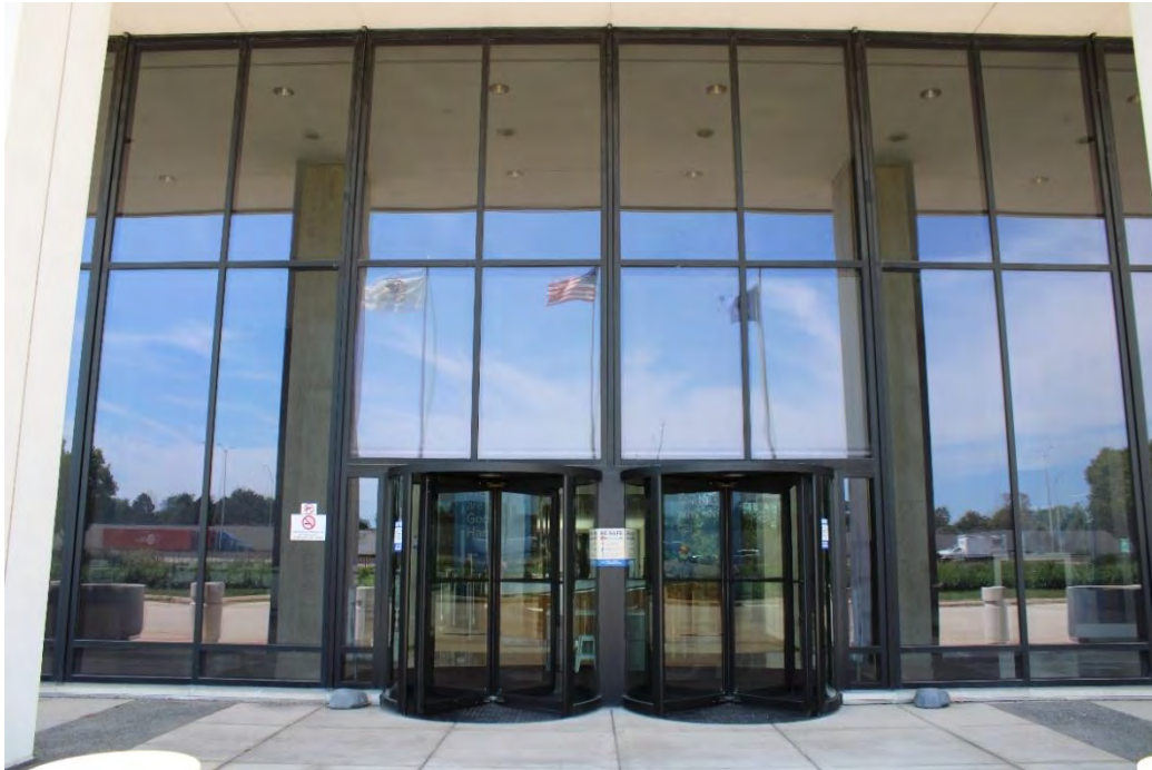
Figure 5: North Plaza Complex, F building's main entrance, view west.
