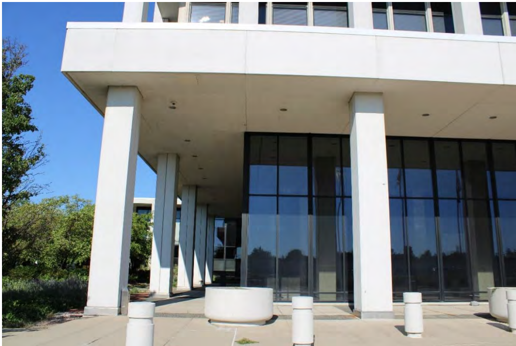
Figure 6: North Plaza Complex, F building detail, view west.
