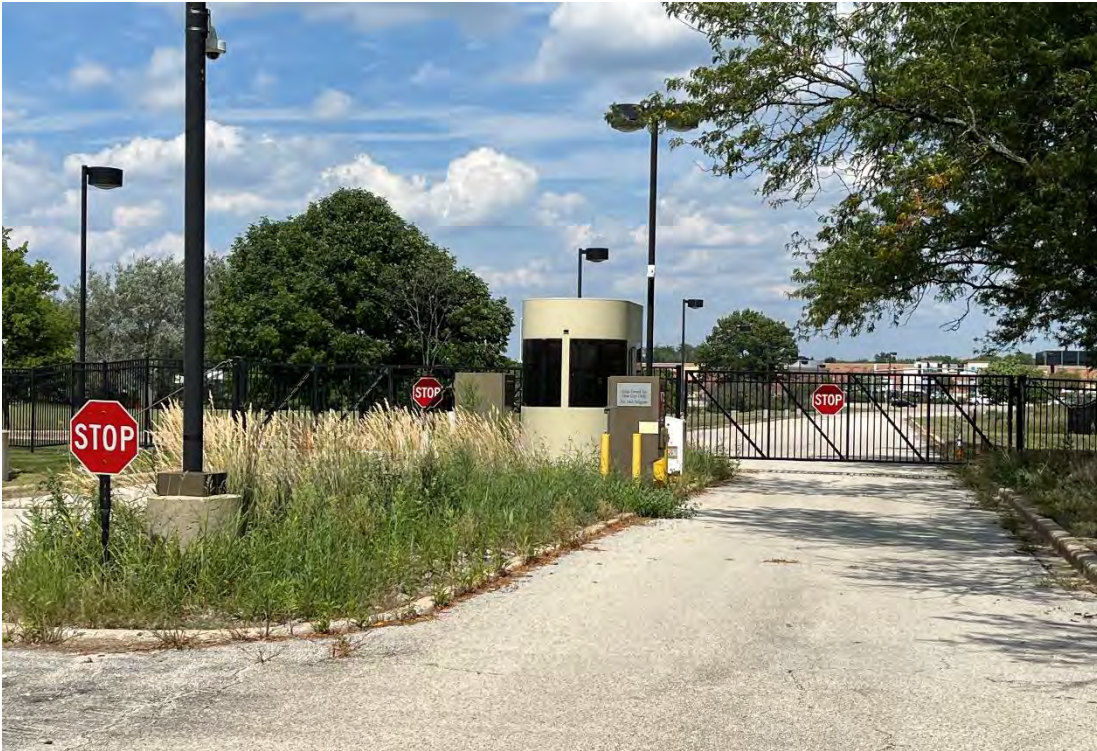
Figure 2: Guard house at the main entrance to the campus on Sanders Road, August 2022.
