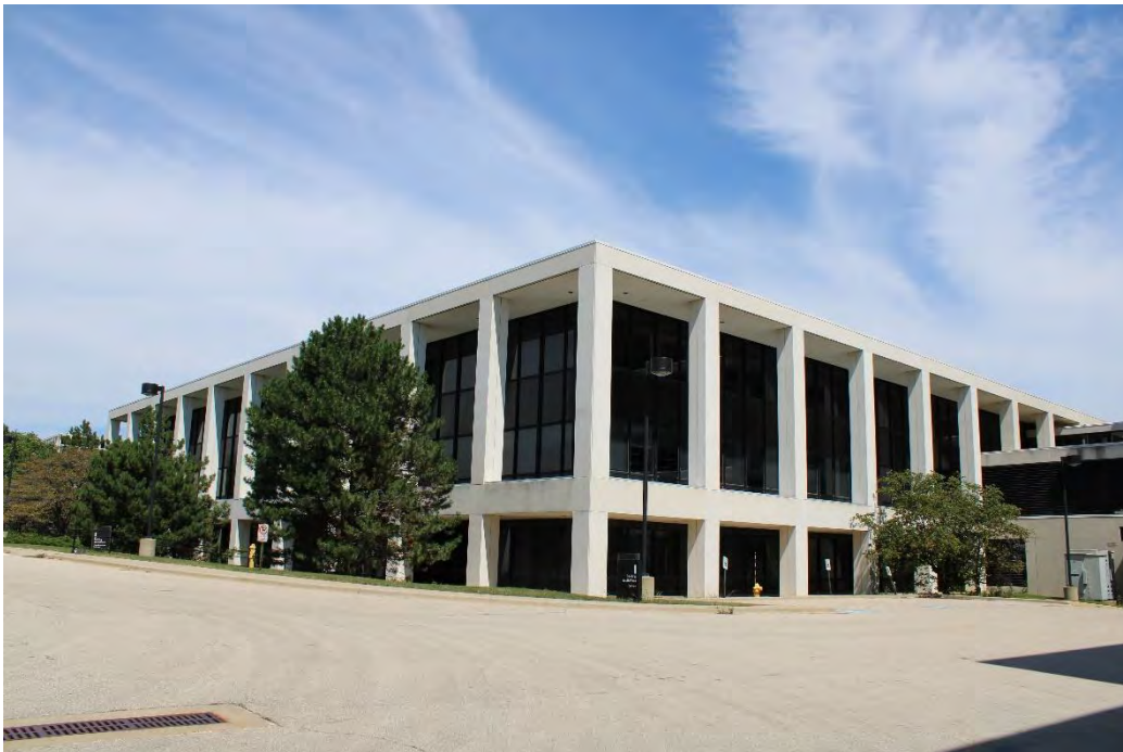
Figure 16: South Plaza Complex, I building, view northeast.
