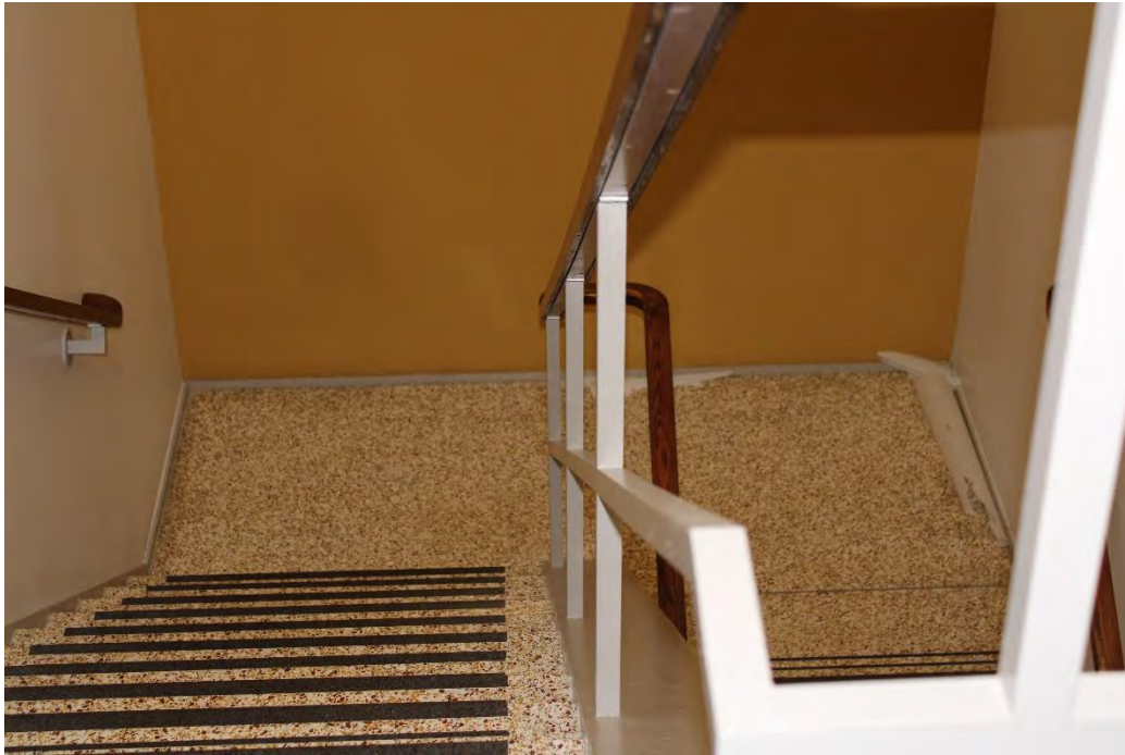
Figure 27: Typical stairwell in South Plaza Complex.
