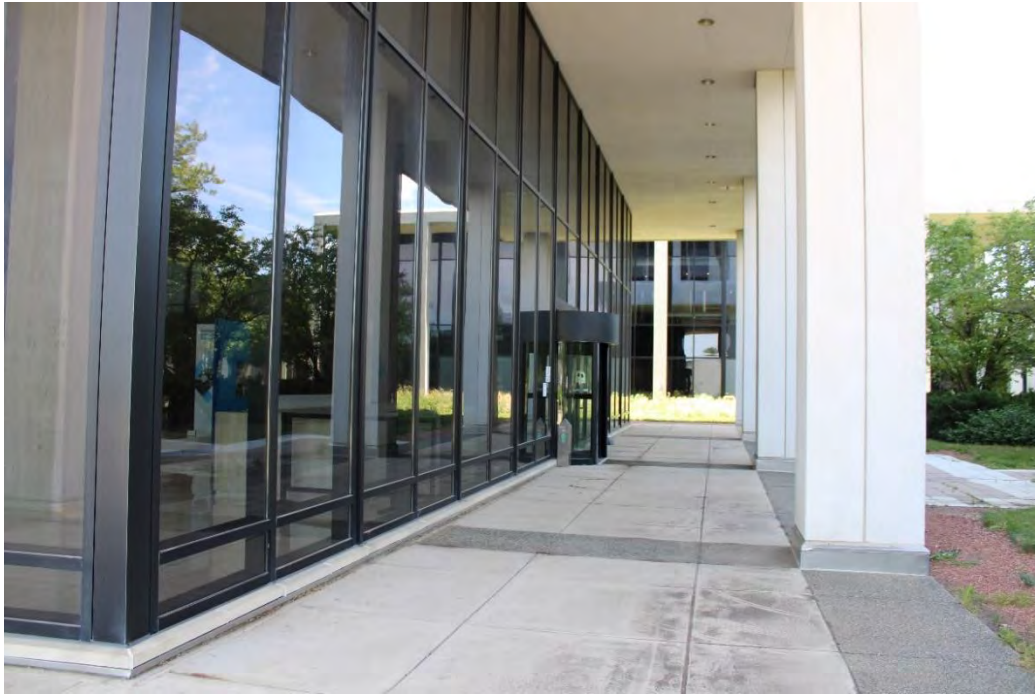
Figure 7: North Plaza Complex, F building's north lobby wall, view west.
