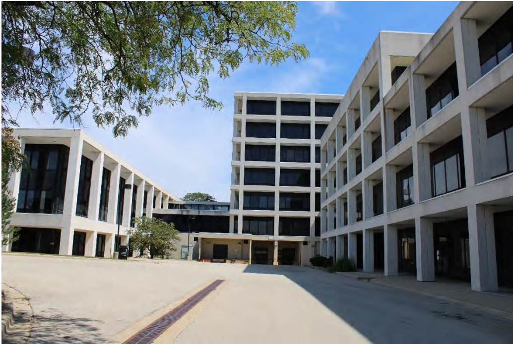
Figure 15: South Plaza Complex showing I building (left) and G building (right), view east.
