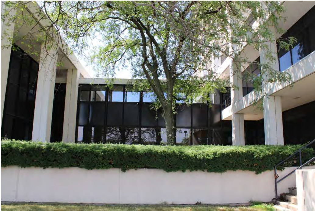
Figure 7: South Plaza Complex, link between the G building (right) and H building (left).
