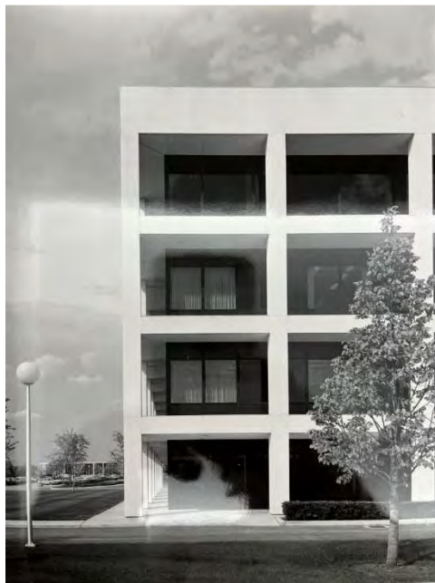
Figure 95: Detail of G building portico, 1975, view north. Photographer: Hedrich Blessing. Source: Chicago History Museum.
