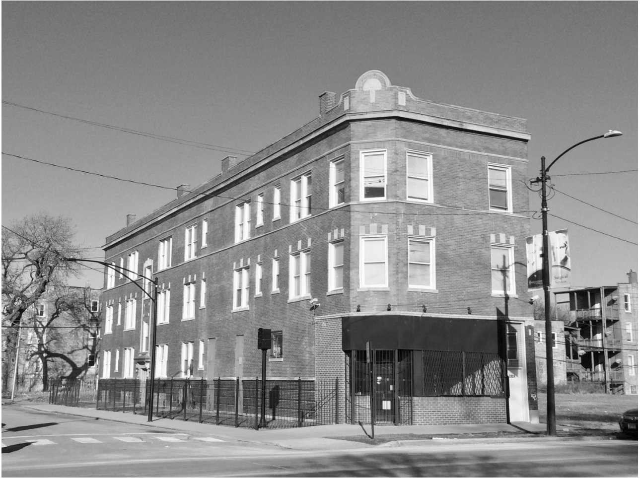
General view of south and west façades from south southwest.
