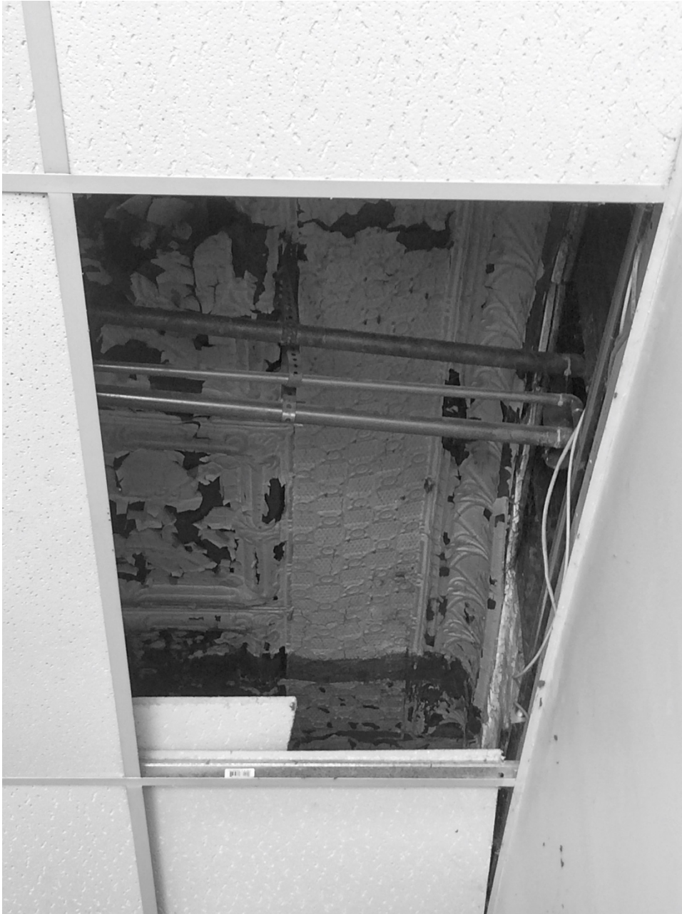
Detail of historic tin ceiling in storefront space.
