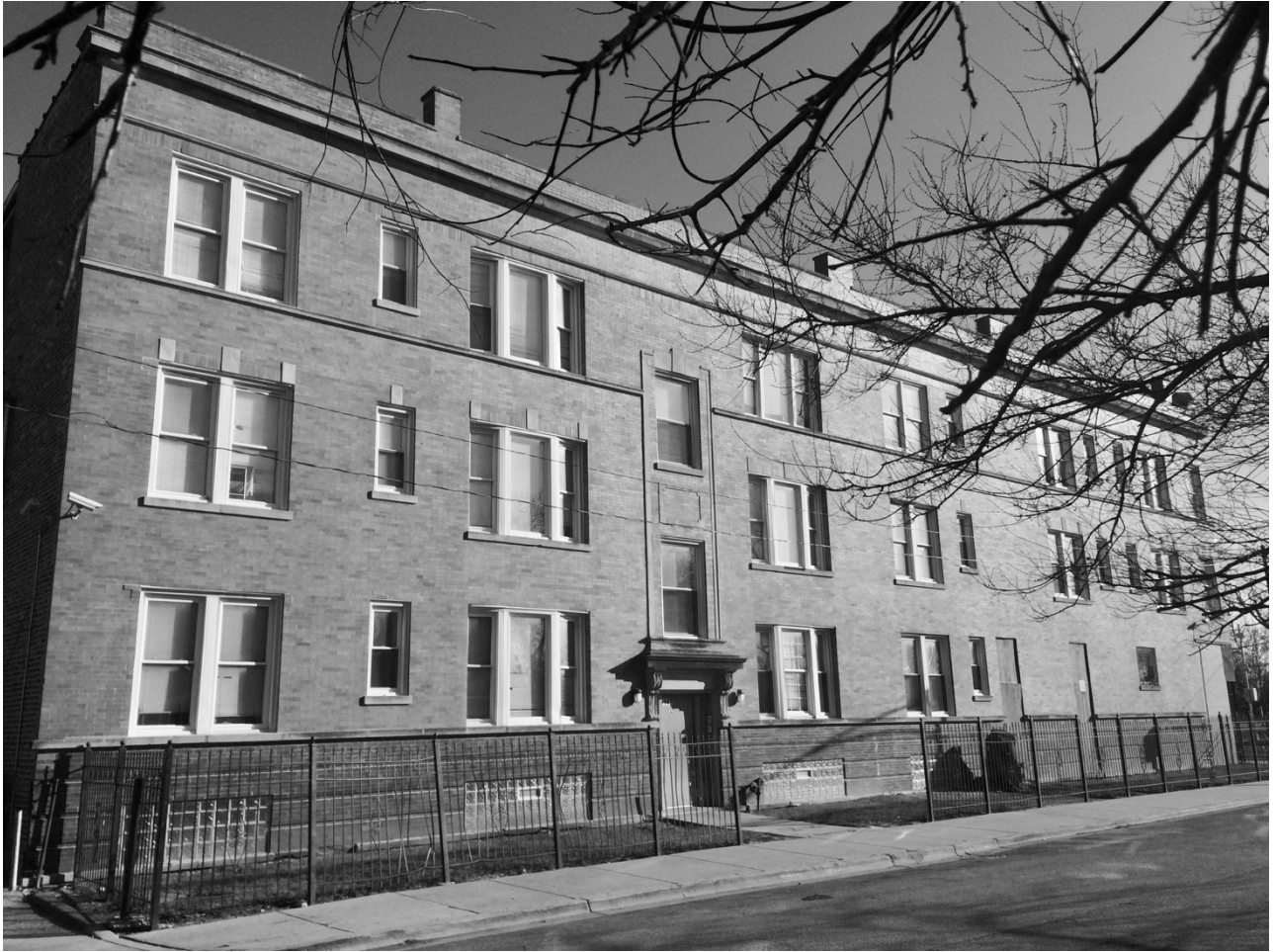
General view of west façade from northwest.
