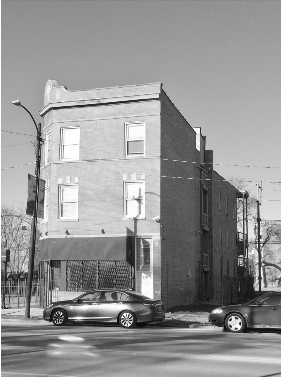
General view of south and east façades from south southeast.
