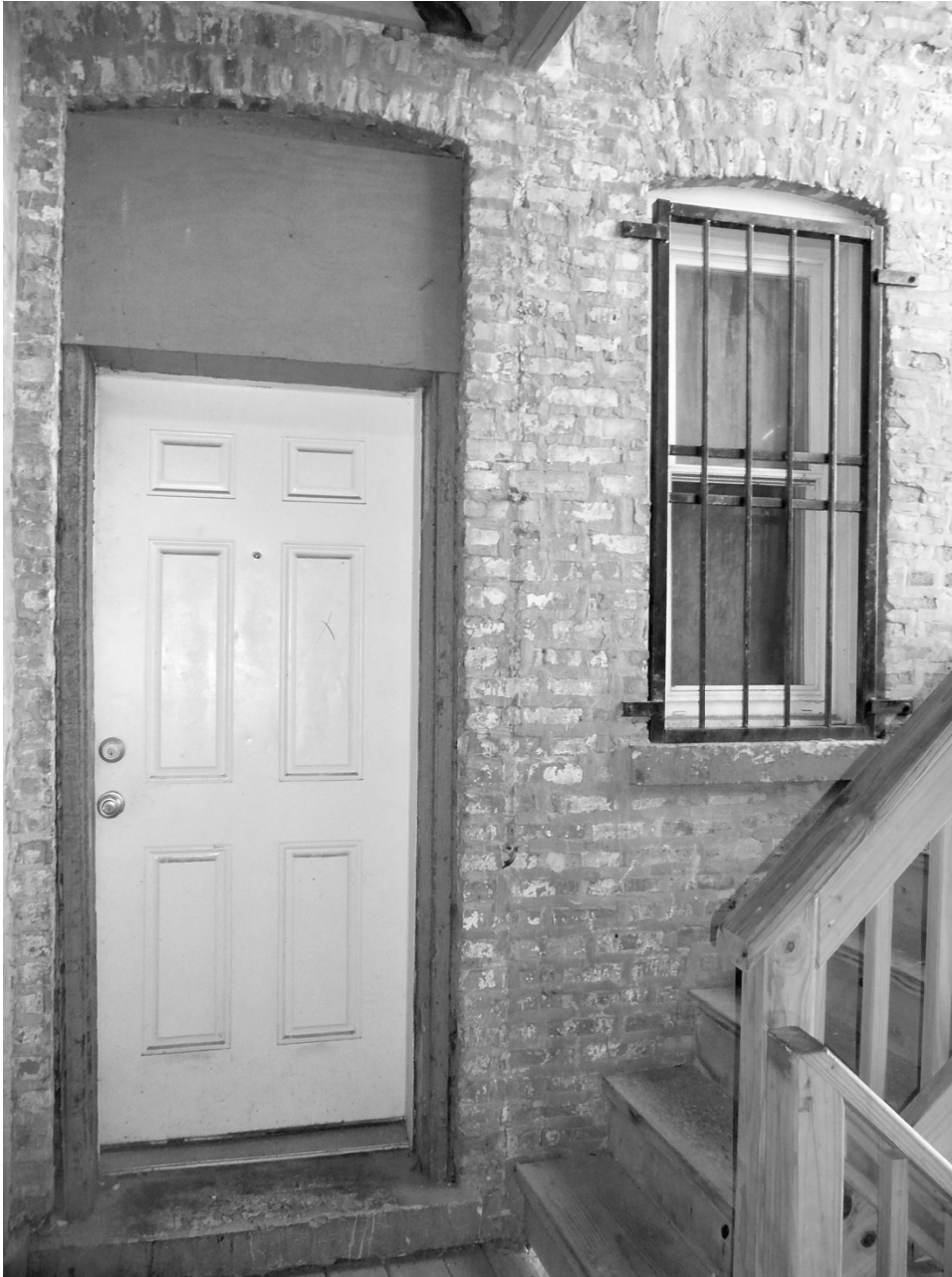
Detail view of rear apartment entrance from eastern external stairwell.
