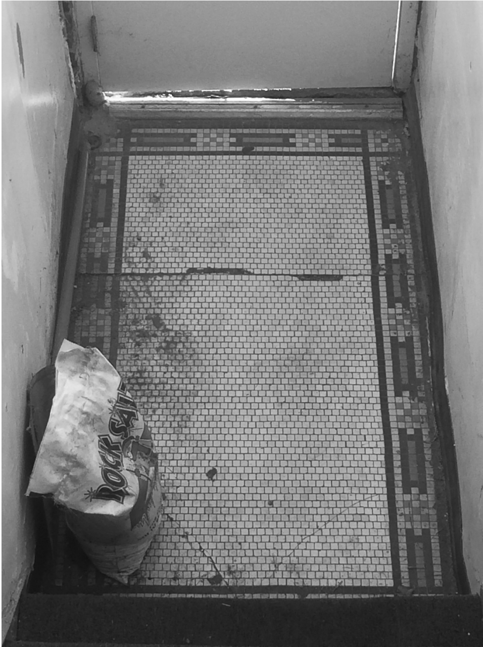
View of south vestibule floor, showing original mosaic tilework.
