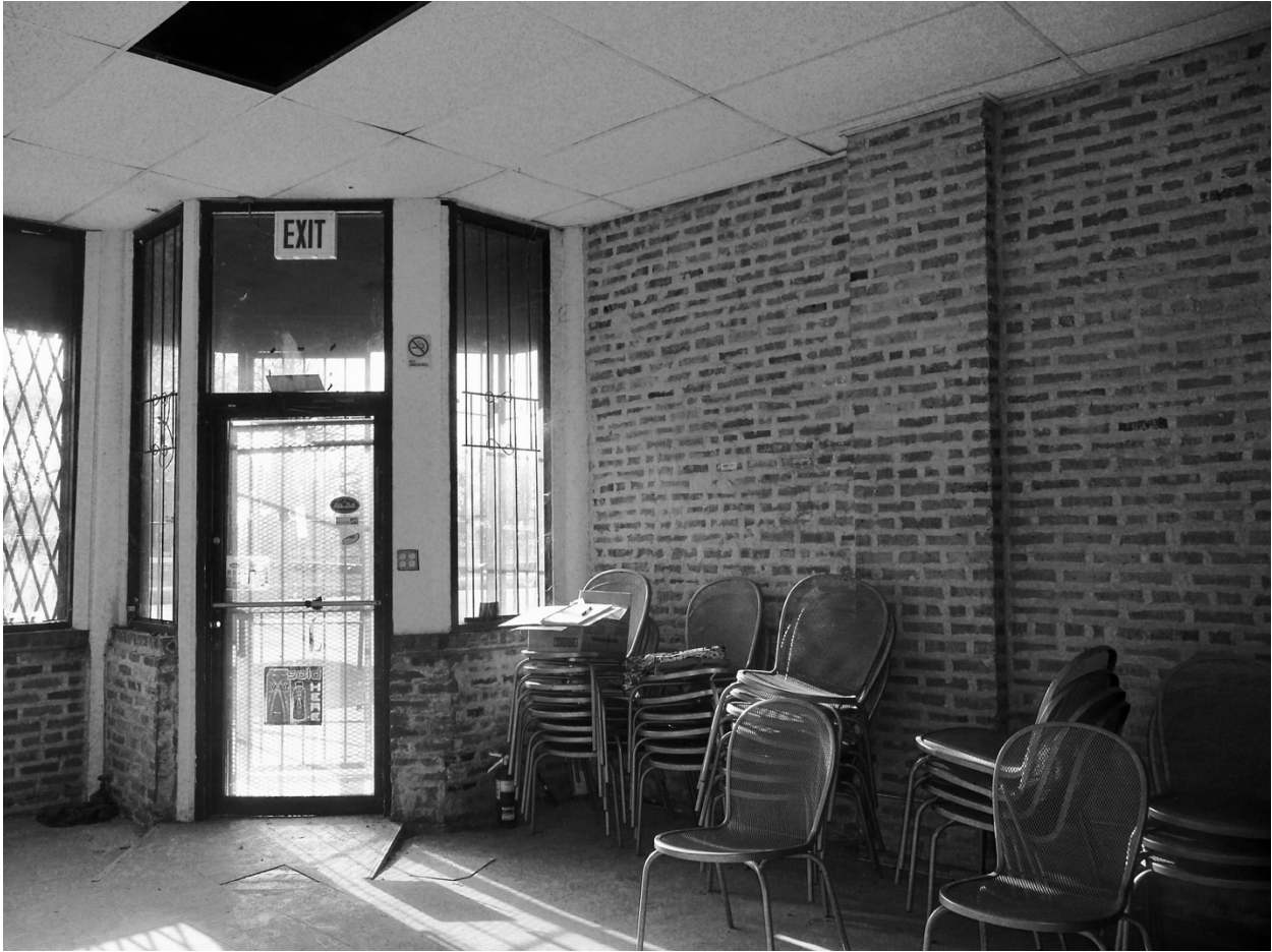
General view of storefront entrance from northeast.
