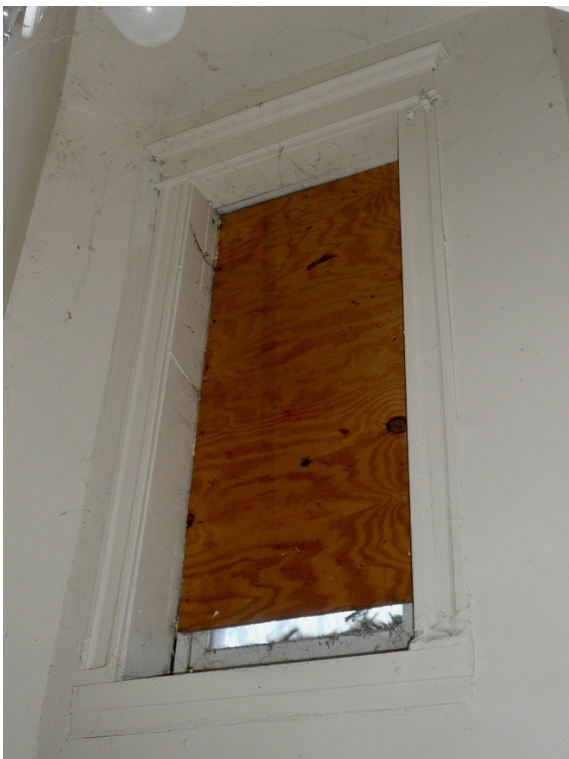
Original window trim scheme
