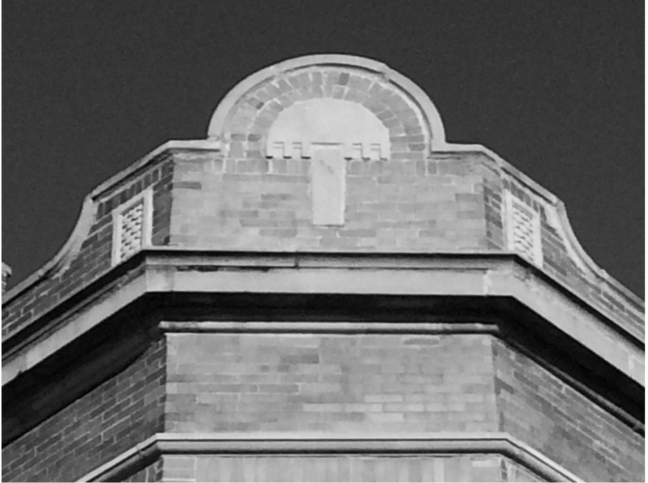
Detail view of southwest corner parapet from southwest.
