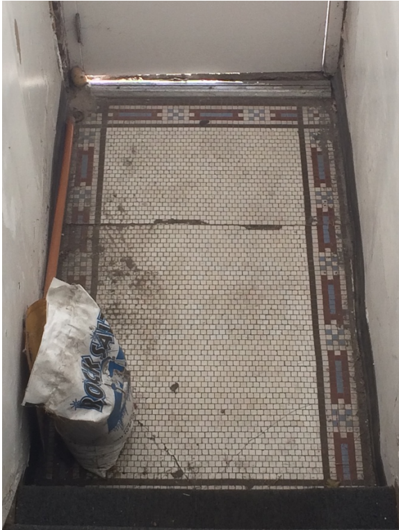
Original tile vestibule floor
