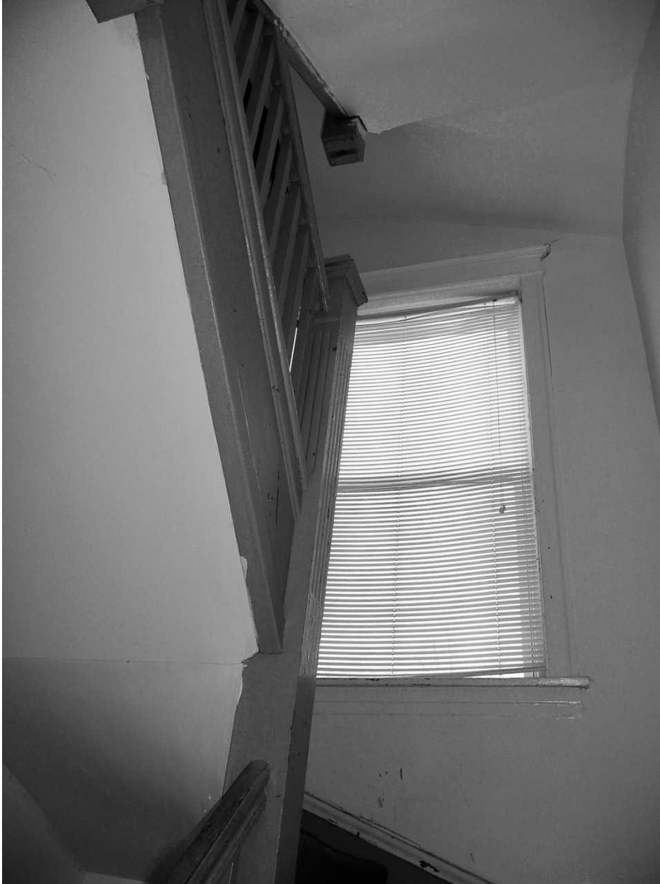
View of apartment staircase, showing original banisters, newel, and window trim.
