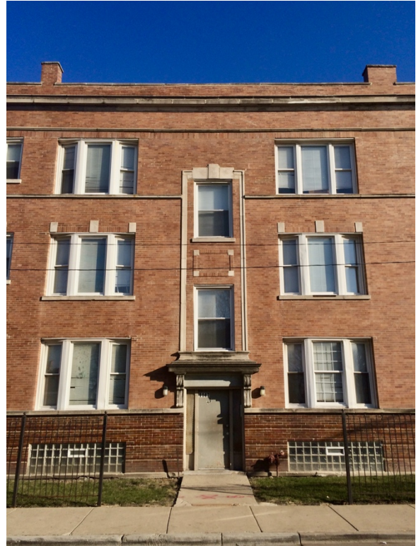
Apartment entrance bay detail
