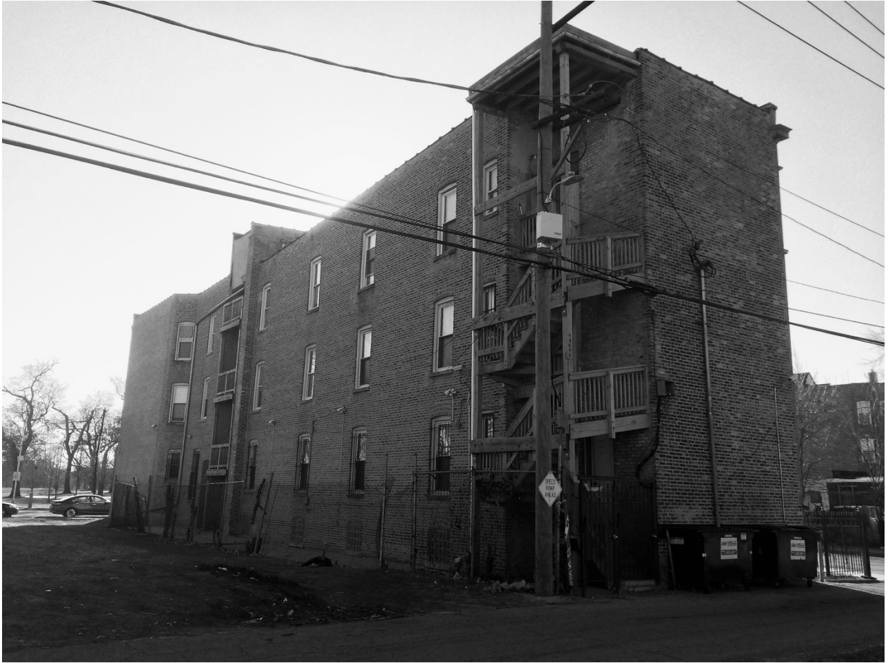
General view of north and east façades from north northeast.
