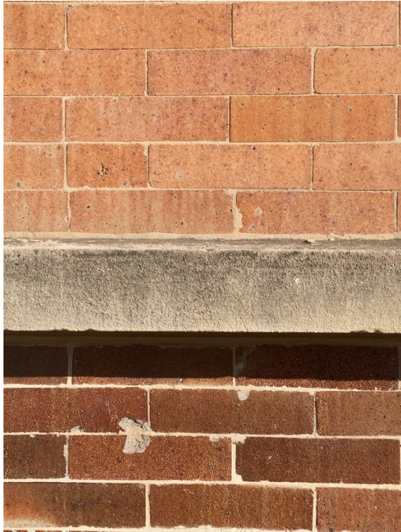
Exterior brick detail
