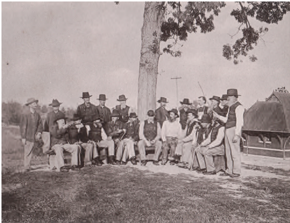
More 1889 views of the Home. Top: View of the power plant and commissary building. Bottom: Group of veterans gathered around a tree by the railroad depot.
