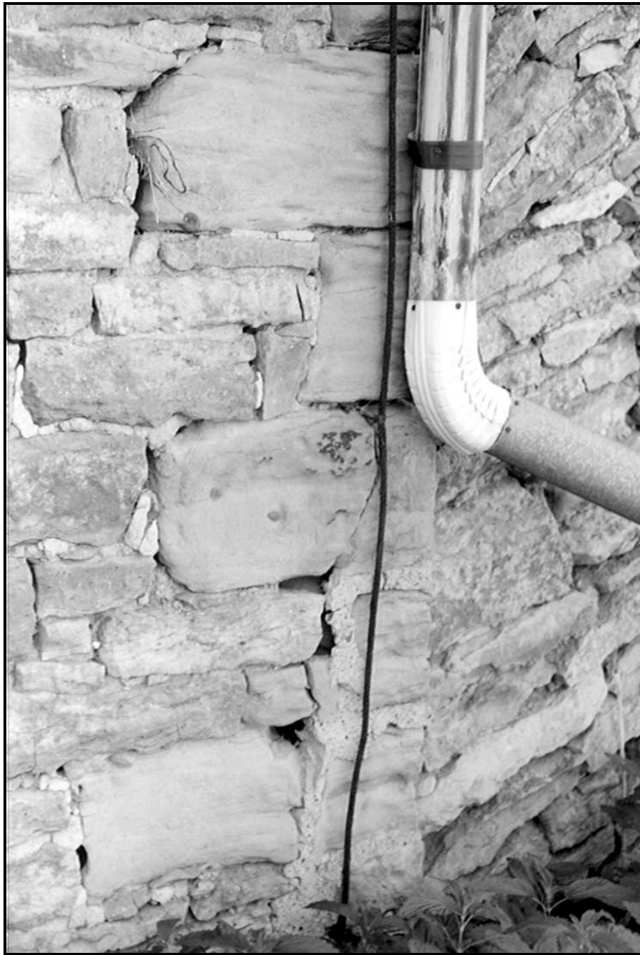
Figure 89. Poor drainage in the past has contributed to the deterioration of the exterior stonework on the barn. This view is of the northeast corner of the barn (FRR May 2001).
