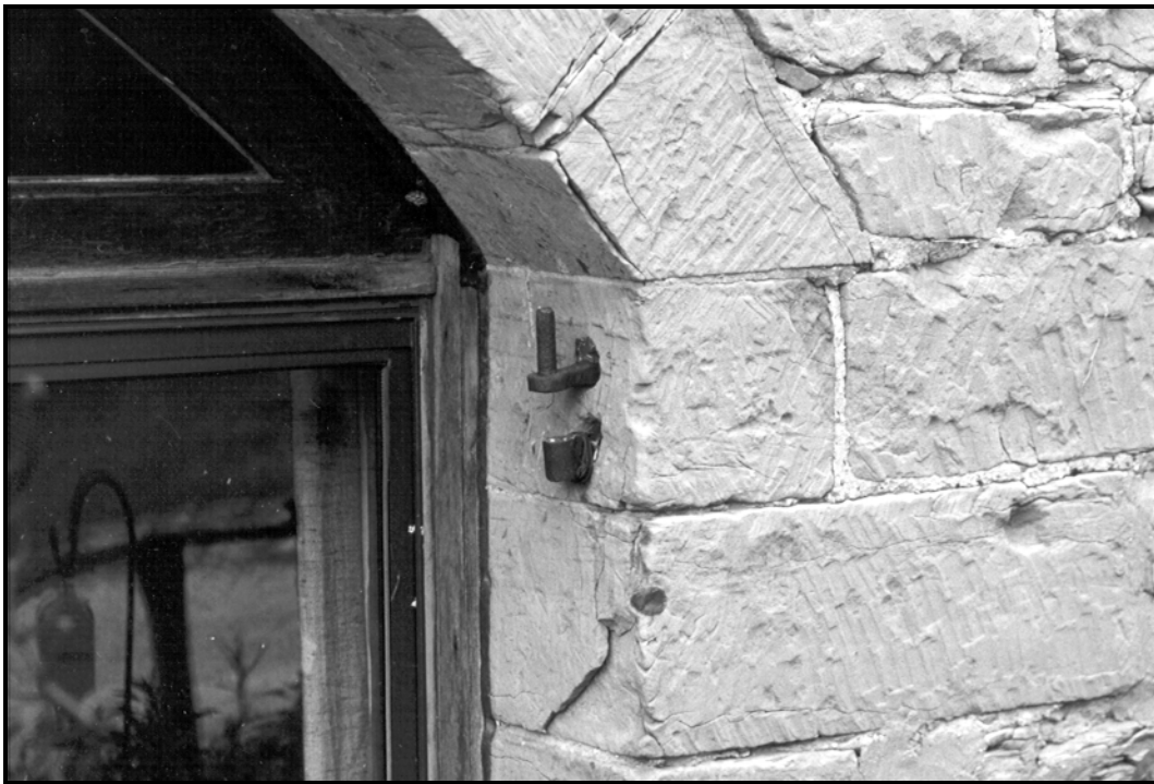
Figure 71. (Top) View of the central arched entrance in the cow house. The doors have been removed and the opening converted into a window. (Bottom) Detail of the arched doorway for the cow house, showing one of the pintels on which the original doors were hung (FRR June 2001).
