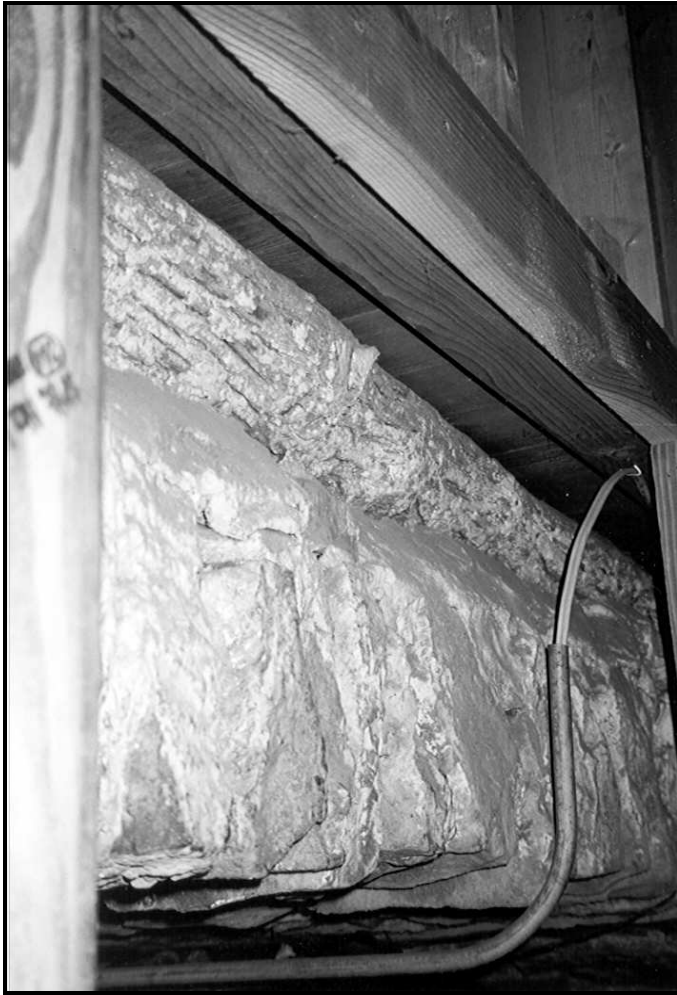
Figure 58. (Left) View of the top of the stone vault over the original cellar room. Note the log floor joist (or “sleeper”) above the vault. (Right) The interior stairway leading between first floor and original cellar room. The stone steps are tied into the foundations and are suspended without the aid of a stringer.
