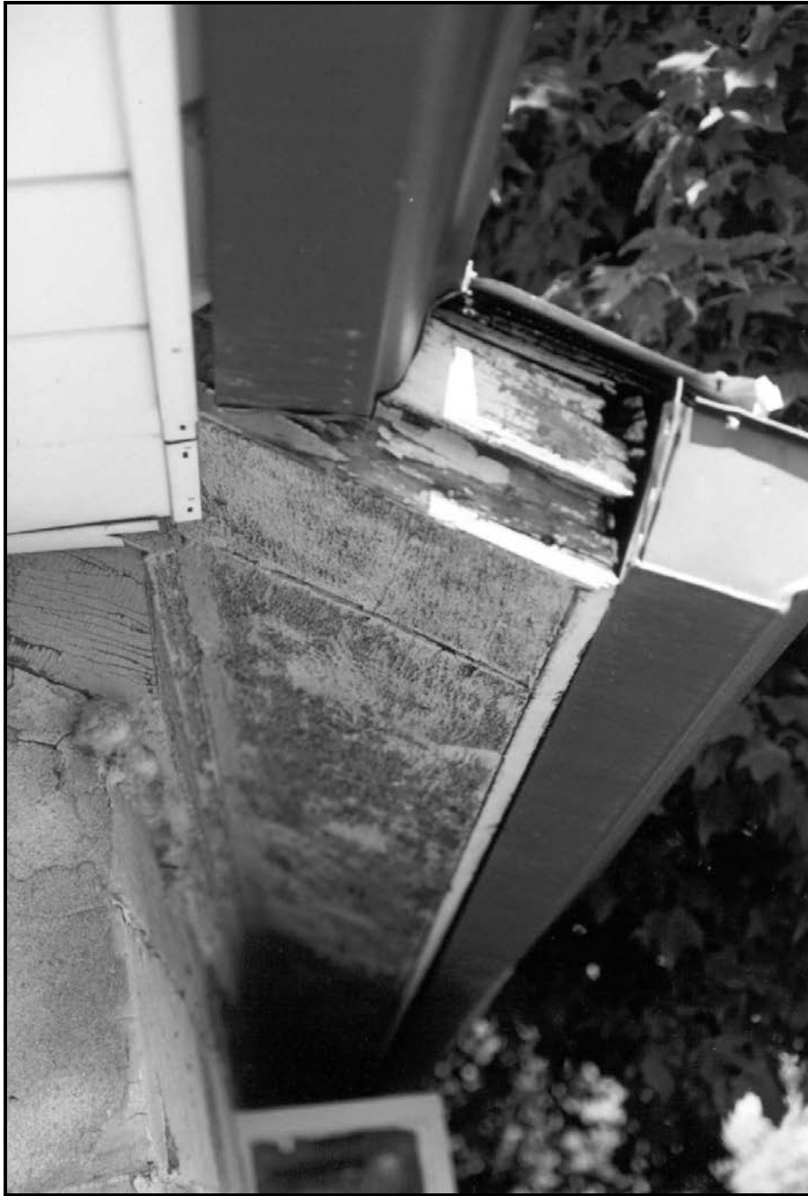
Figure 84. View of the eave at the southwest corner of the original house, illustrating the poor condition of the paint. The eaves on the original house and north addition should be scraped, primed, and painted (FRR July 2001).
