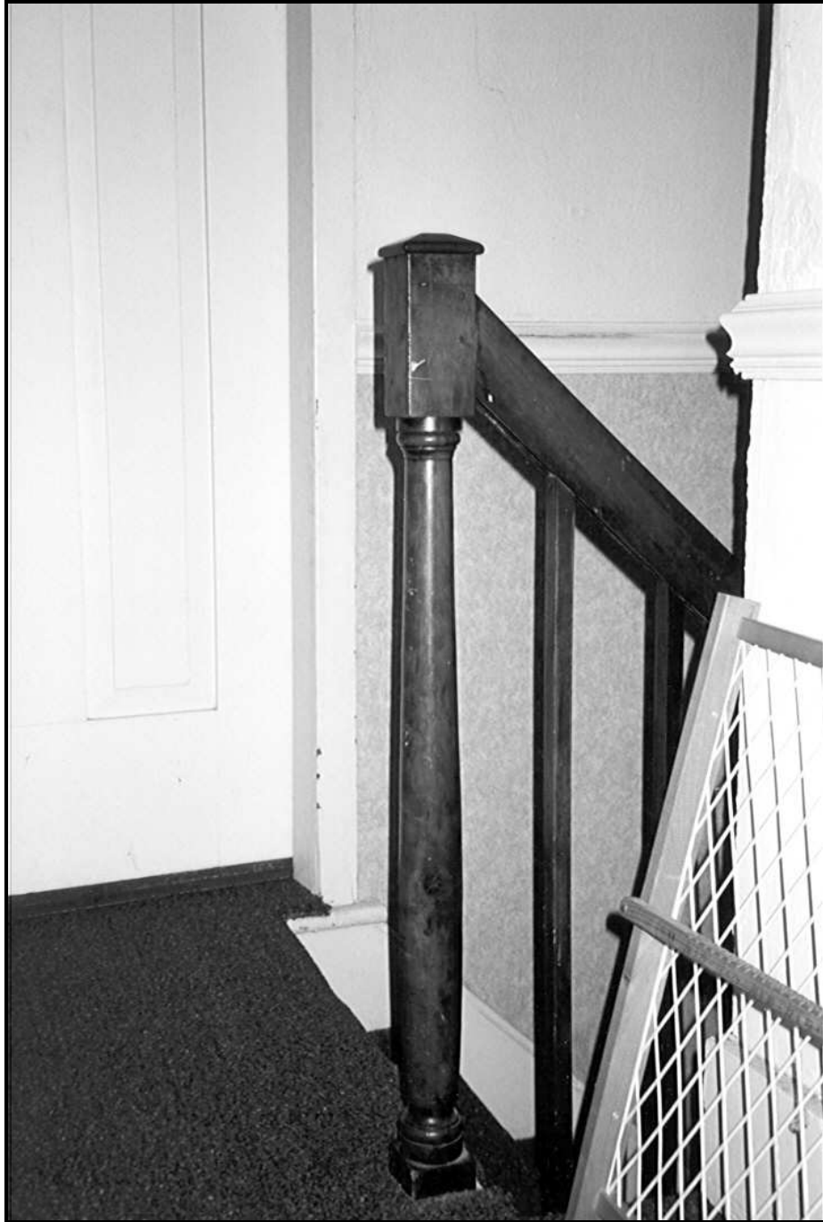
Figure 59. View of the newel post and balustrade present at the top of the second-floor stairway (FRR June 2001).
