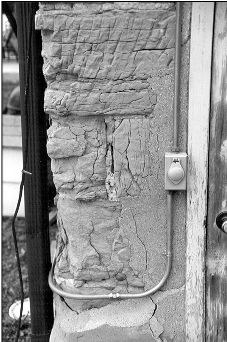
Figure 88. View of concrete parging that has been applied at the southwest corner of the barn. Future conservation efforts should avoid using such methods (FRR June 2001).
