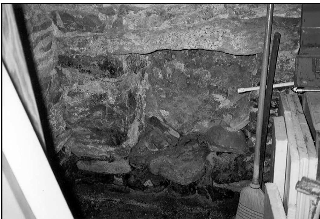
Figure 57. (TOP) View of vaulted cellar room located beneath original house, looking west. (BOTTOM) View of one of the two wall niches that are present along the south side of the vaulted cellar room. Niches of this type often were used as cold storage chambers for food and/or drink (FRR June 2001).
