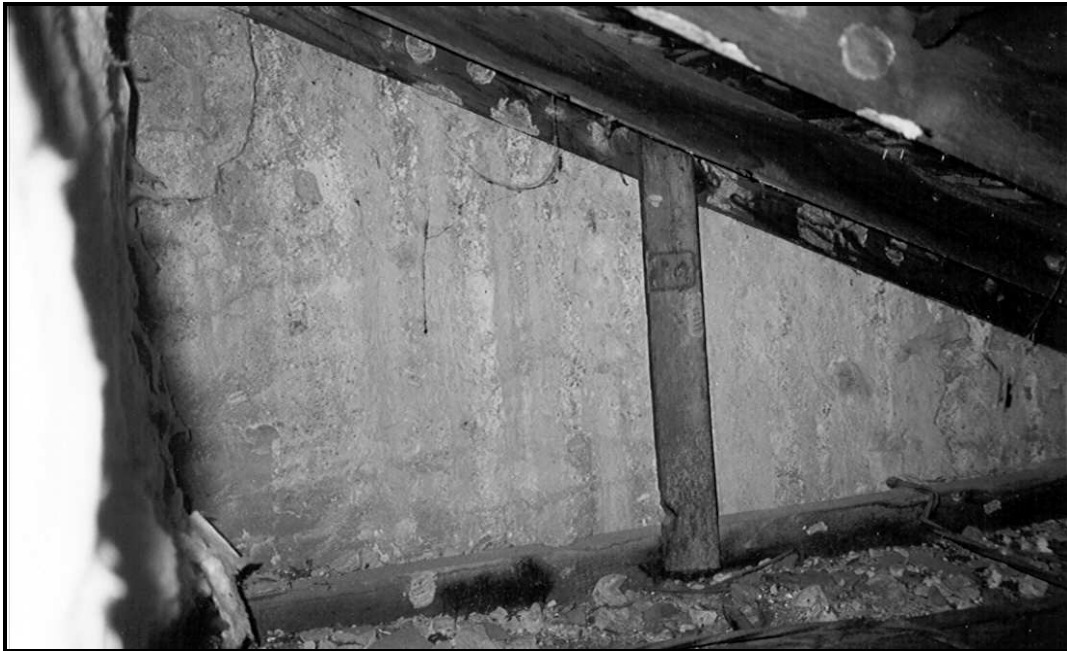
Figure 34. (TOP) Detail of the stonework on the southwest corner of the Howarth House, illustrating the different dressing techniques used. The stones to the right face east and have been roughly dressed with pointwork, while those on the far left are associated with the façade of the original house and have a finer finish. (BOTTOM) View of the stucco that covers the north elevation of the original house, looking from the attic of the porch that stretches across the west side of the north wing. The date of the stucco's application has yet to be determined (FRR June 2001).
