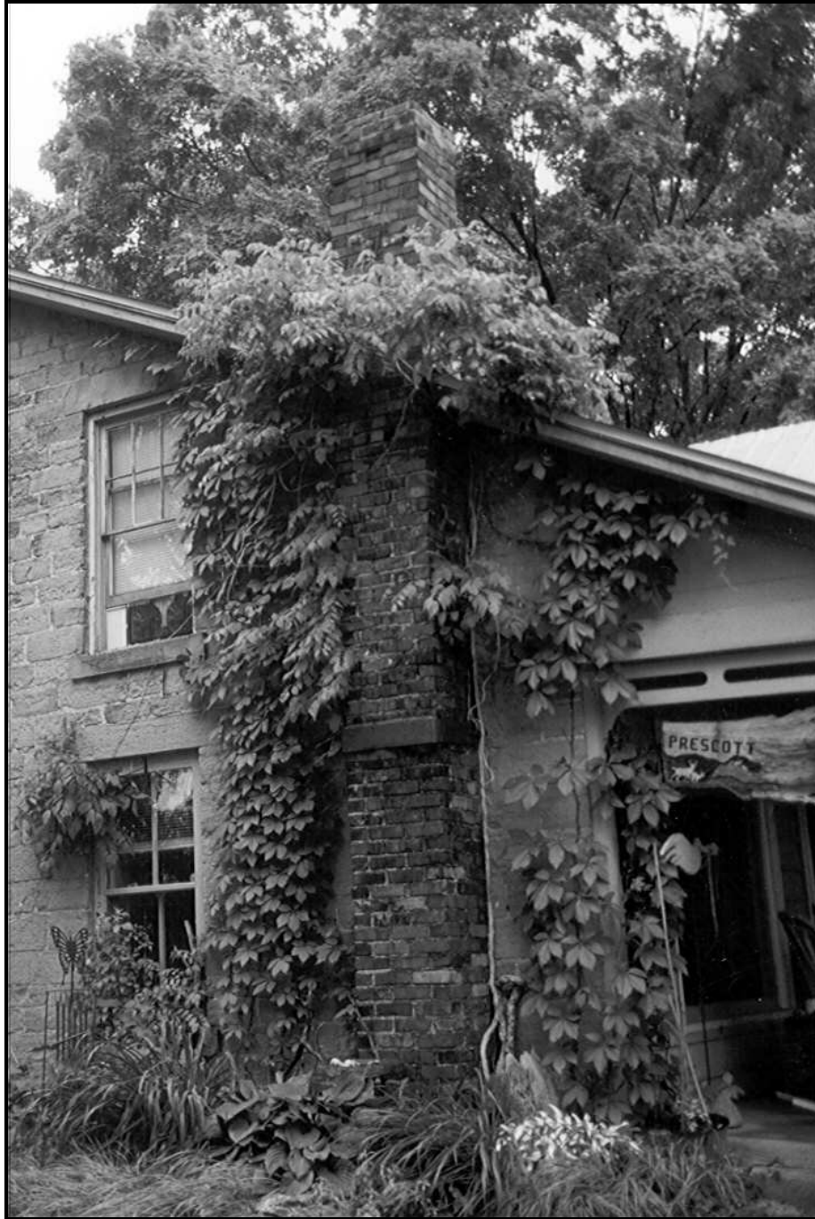
Figure 46. Photograph of the northwest corner of the north wing, showing the exterior brick chimney that vents the boiler currently used to heat the house. A hot-water heating system was installed in the house during the early twentieth century (FRR June 2001).
