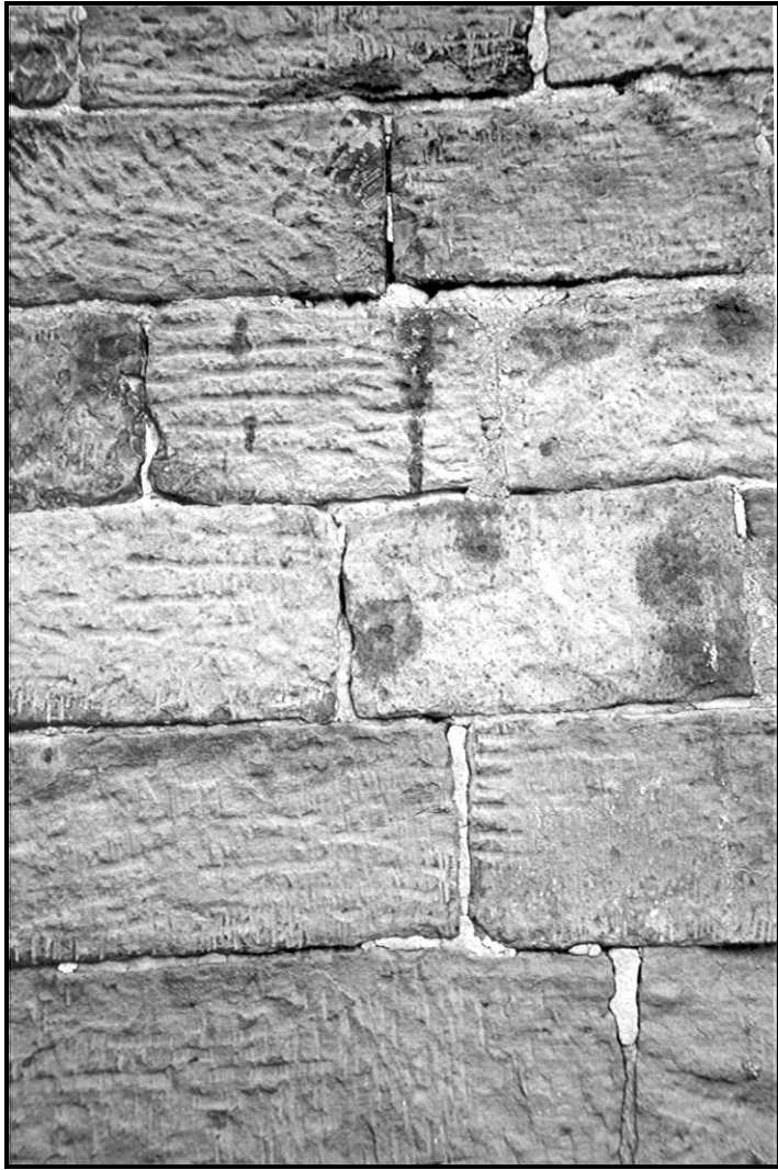
Figure 37. Comparison of the different dressings used on the stone sections of the Howarth House. The stones on the left are found on the east elevation of the original house, while those on the right are from the north wing (FRR June 2001).
