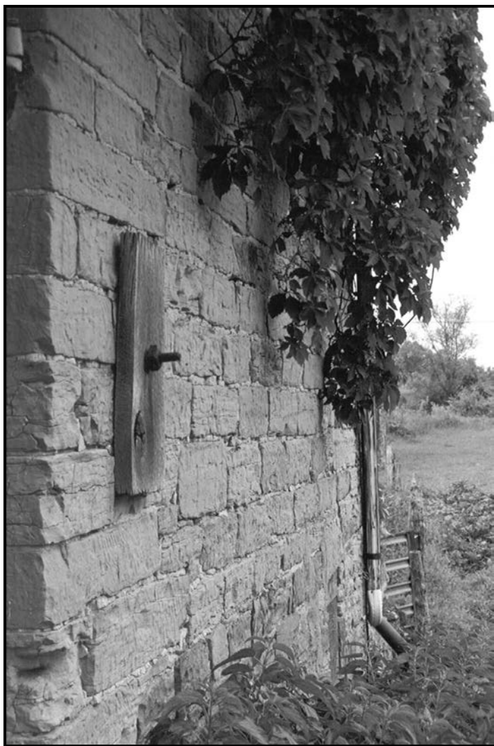
Figure 86. (Left) Section of wall on east side of barn that is bulging out. (Right) Stress fractures on interior of the west wall of barn (FRR June 2001).
