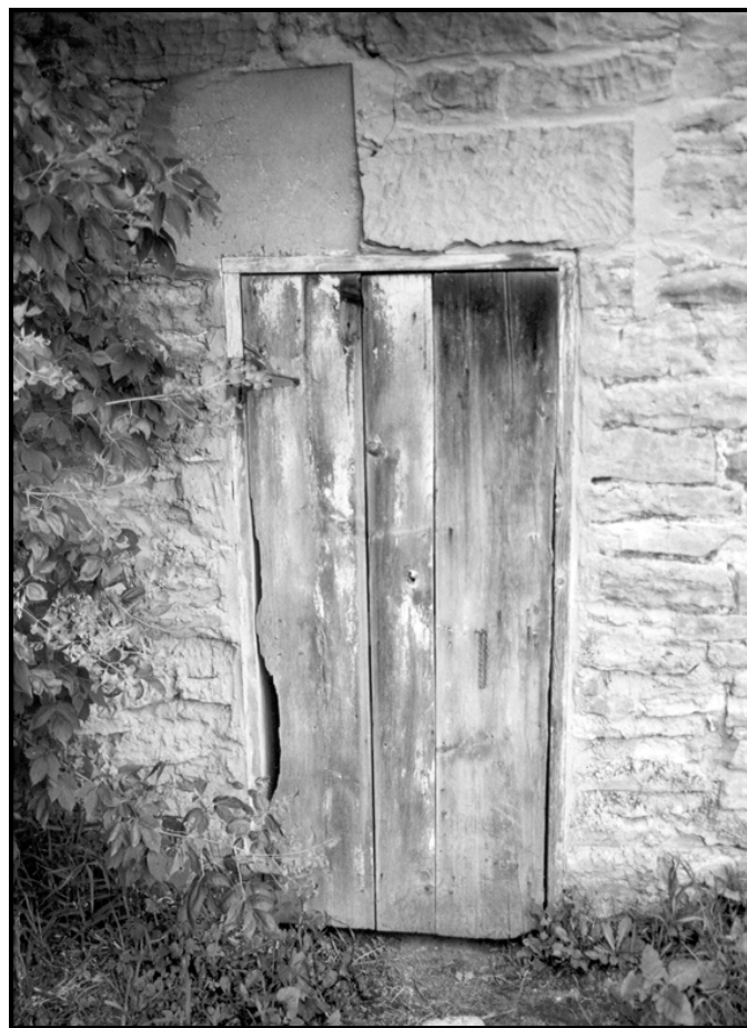
Figure 72. (Left) View of the western door that accesses the cow house section of the barn. This doorway originally serviced livestock, but now functions as the principal entrance to the living quarters that have been installed in the cow house. (Right) View of the personnel door on the west side of the barn. The plank construction of this door was probably typical of the original doors on the barn (FRR June 2001).
