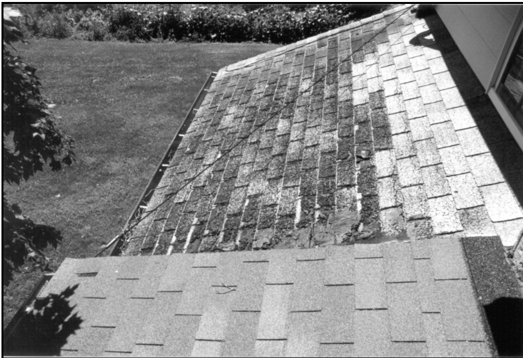
Figure 83. (Top) Cracked and fissured window sill on the south elevation of the house. (Bottom) Deteriorated roofing over the bathroom/laundry room addition (FRR July 2001).
