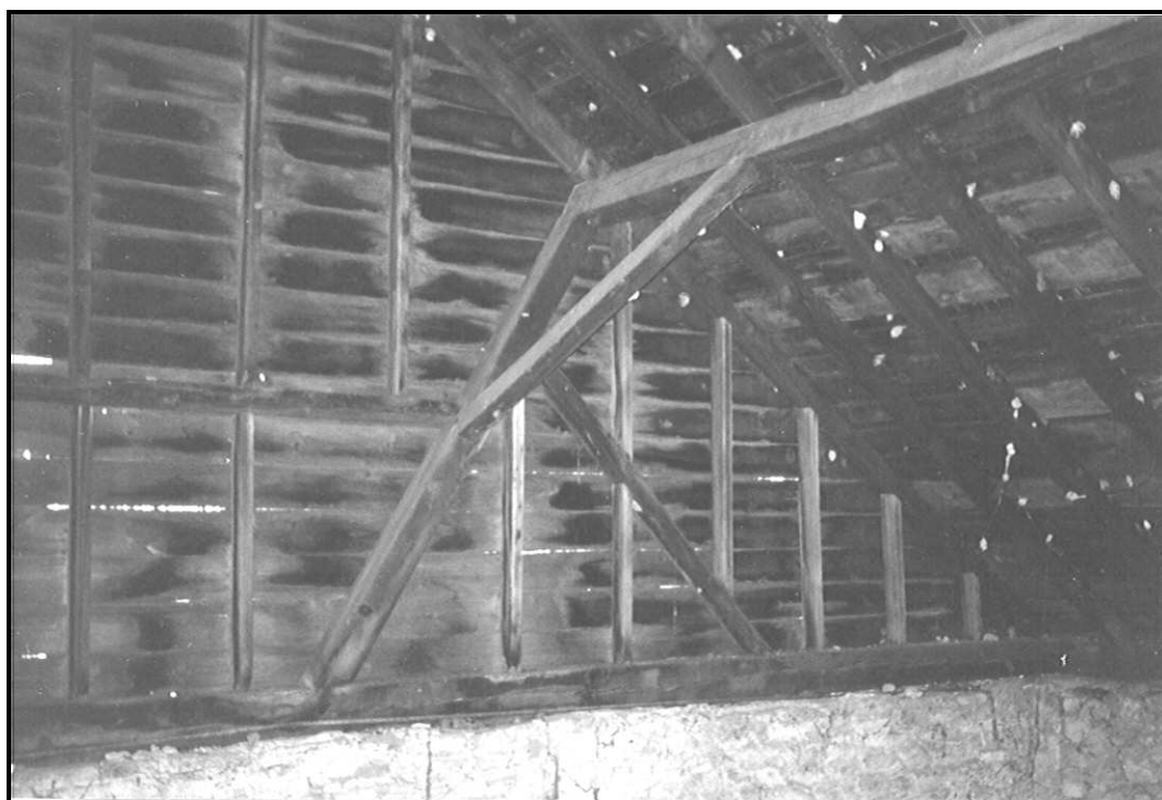
Figure 69. (Top) View of the roof system in the main barn, showing the underframing. (Bottom) View of the framing at the north gable. The stonework originally present in the gable has been removed down the level of the rafter plate (FRR June 2001).
