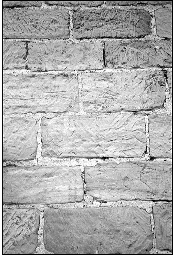
Figure 37. Comparison of the different dressings used on the stone sections of the Howarth House. The stones on the left are found on the east elevation of the original house, while those on the right are from the north wing (FRR June 2001).
