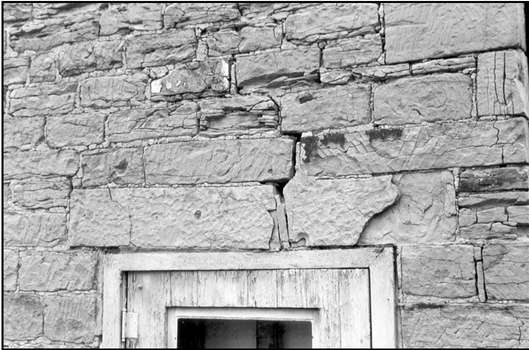
Figure 87. Two views of the differential weathering seen on the exterior of the barn. Cracking and spalling is prevalent (FRR June 2001).
