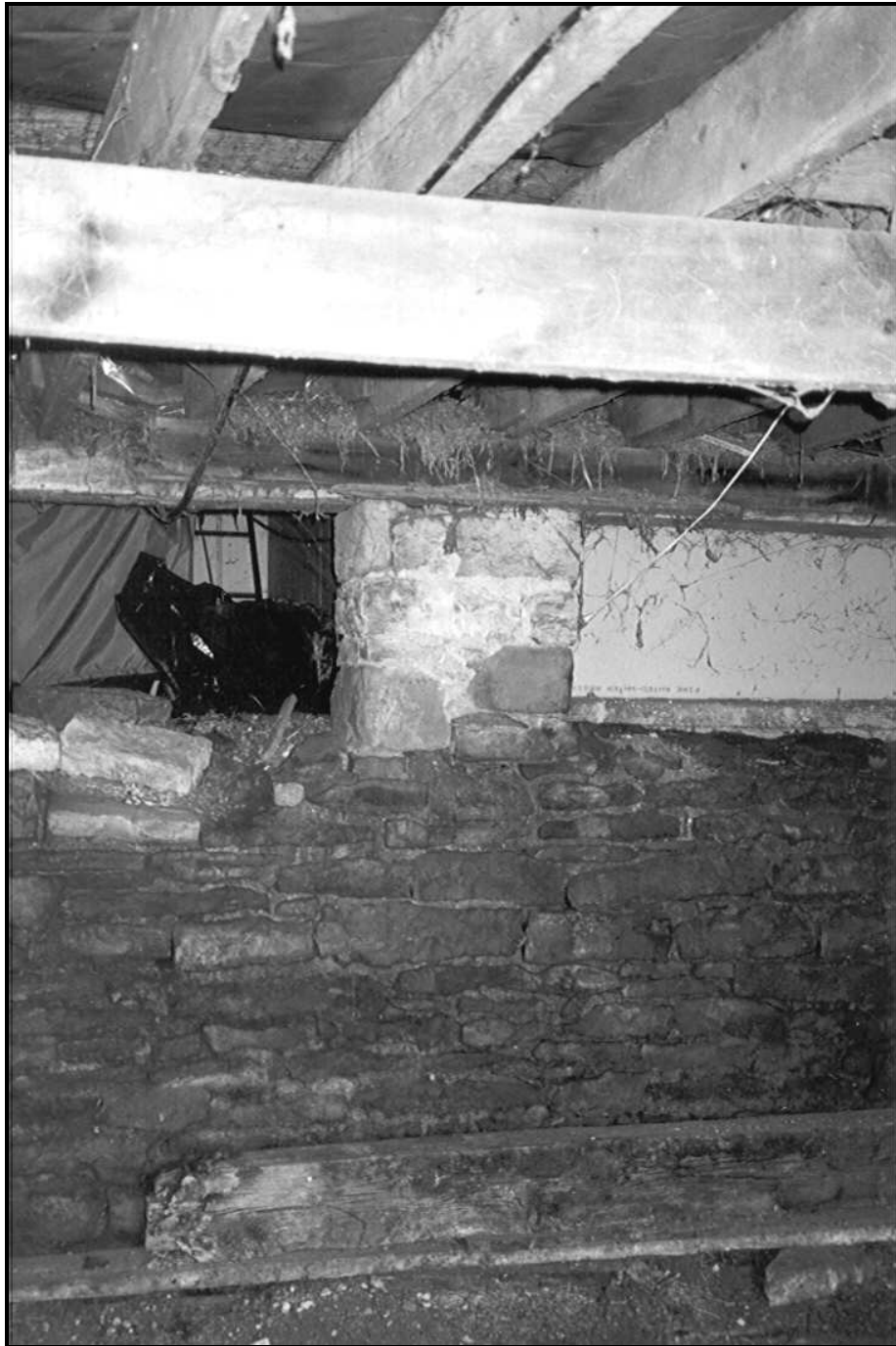
Figure 67. View of the interior foundations along the south side of the basement. The pier on top of the foundation wall helps support the north framing bent in the barn (FRR June 2001).
