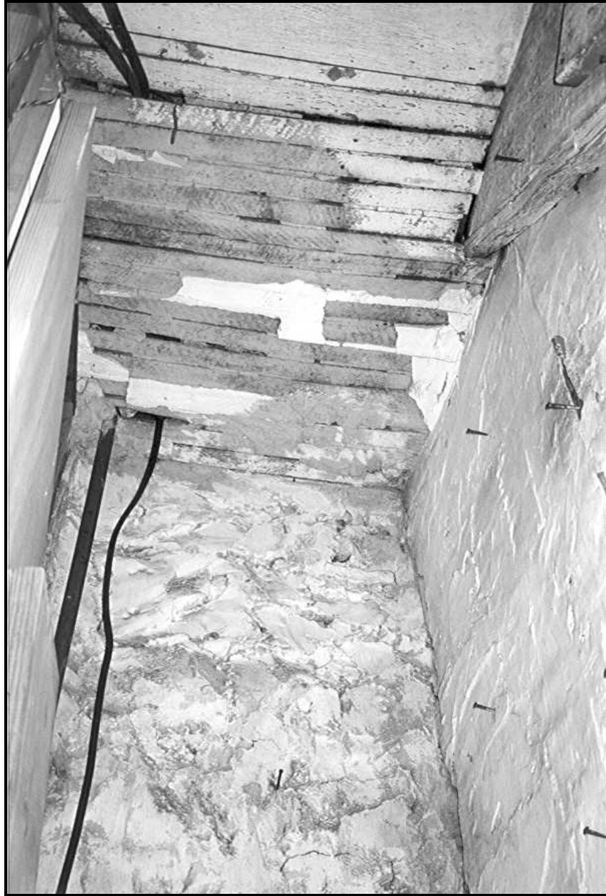
Figure 60. View of the area beneath the second-story stairway, illustrating the character of the original wall and ceiling finishes in the house. The ceiling was covered with sawn wood and plaster. The wall to the right of the view, which separates Rooms 101 and 102, was covered with a thin coat of plaster and then whitewashed; no lath was required on account of the brick nogging between the studs. The wall at the center of the view is the rear (north) wall of the original house, and its interior face was covered with a rough coat of plaster applied directly over the stone (FRR September 2001).
