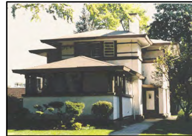
Figure 26: Flori Blondeel House #1 - 1913. From Martin Hackl's unpublished book: The Work of John S. Van Bergen, Architect .
