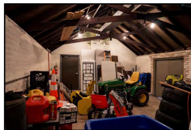
Figure 114: Warming Hut interior - entrance and fireplace, which is covered with equipment. Photograph by Susan Ryan Kalina.
