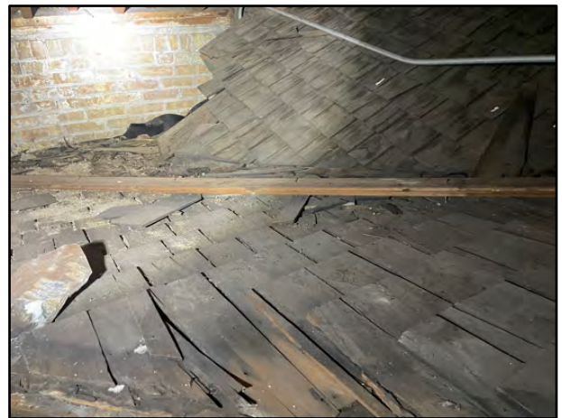
Figure 63: Original roof. Photo by Wight & Co.
