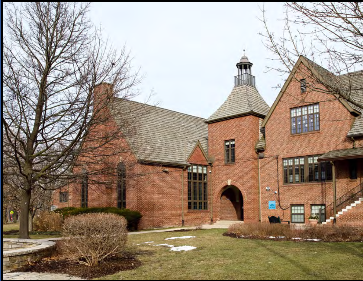
Photo 05 Entrance to Gymnasium/Auditorium
