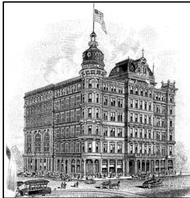
Figure 32: Caldwell Hotel - 1889. Demolished due to fire in 1894. From bhamwiki.com.
