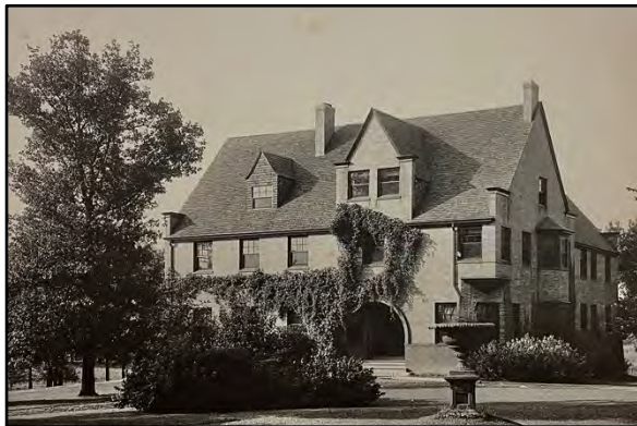
Figure 14: Durand Cottage - Dormitory - 1893. Demolished mid-1960s. From Ryerson and Burnham Art and Architecture Archives.
