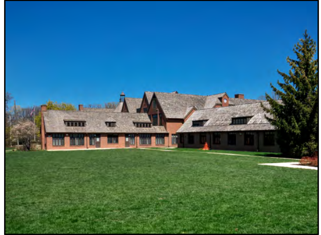
Figure 61: Southside of West Wing along with the 1998 South Wing Addition. Photograph by Susan Ryan Kalina.
