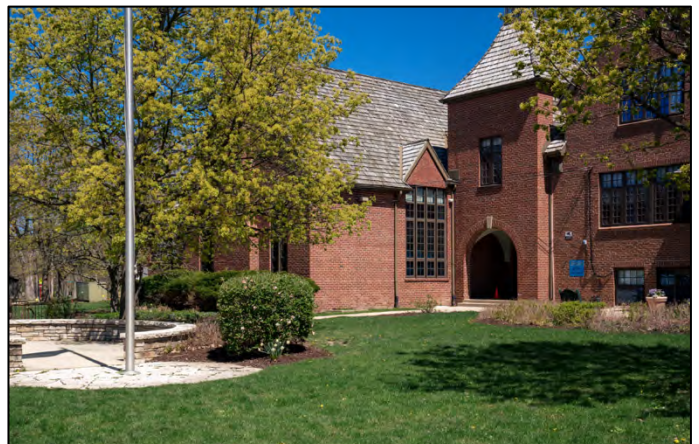
Figure 71: 1927 Addition with view of auditorium and entrance. Photograph by Susan Benjamin.
