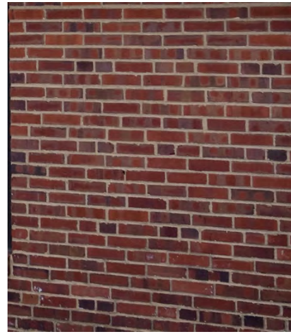
Figure 51: Brick detail. Photograph by Susan Ryan Kalina.
