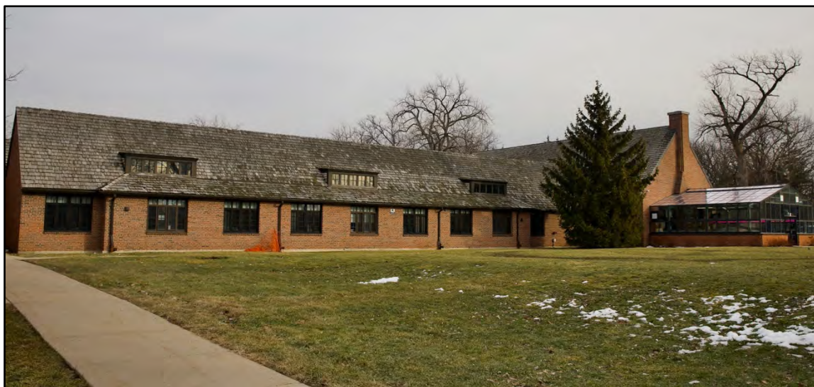
Figure 89: 1998 South Wing addition. Photograph by Deb Carey McIlvain.
