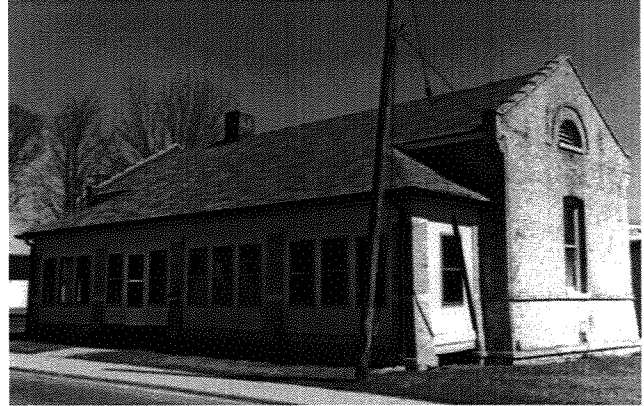
Quartermaster Stables Guardhouse (#37), 1997. Photograph by Victoria Granacki
