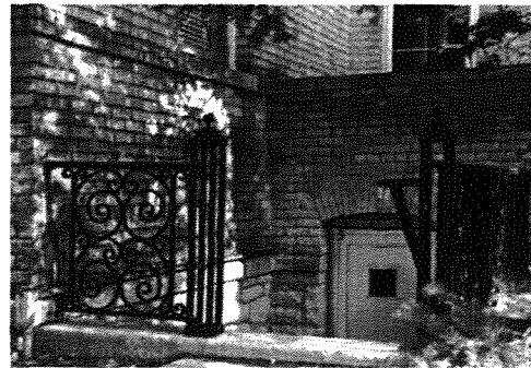
Barracks, railing detail (#50), 1997. Photograph by Victoria Granacki
