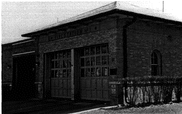
Fire Station (#79), 1997. Photograph by Victoria Granacki
