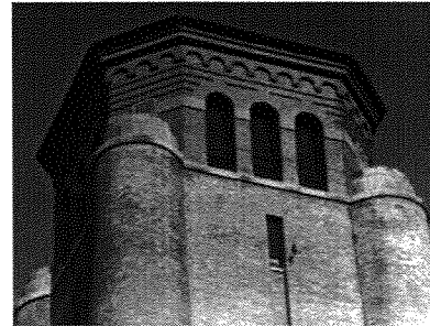
Water Tower, roof (#49), 1997. Photograph by Victoria Granacki
