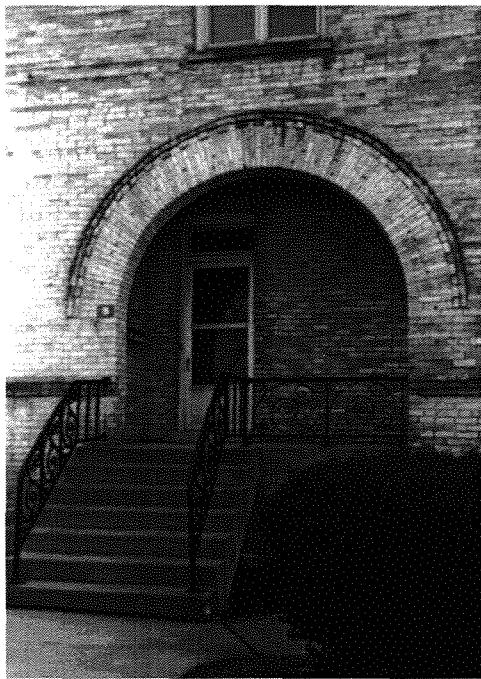
Front entrance to Lieutenants' Quarters (#5), 1997. Photograph by Victoria Granacki
