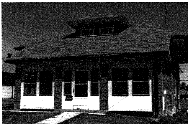
Saddler's and Stable Sergeant's Building (#72), 1997 Photograph by Susan S. Benjamin
