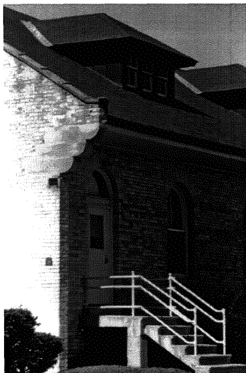
Quartermaster and Commissary Storehouse (#35), 1997. Photograph by Victoria Granacki
