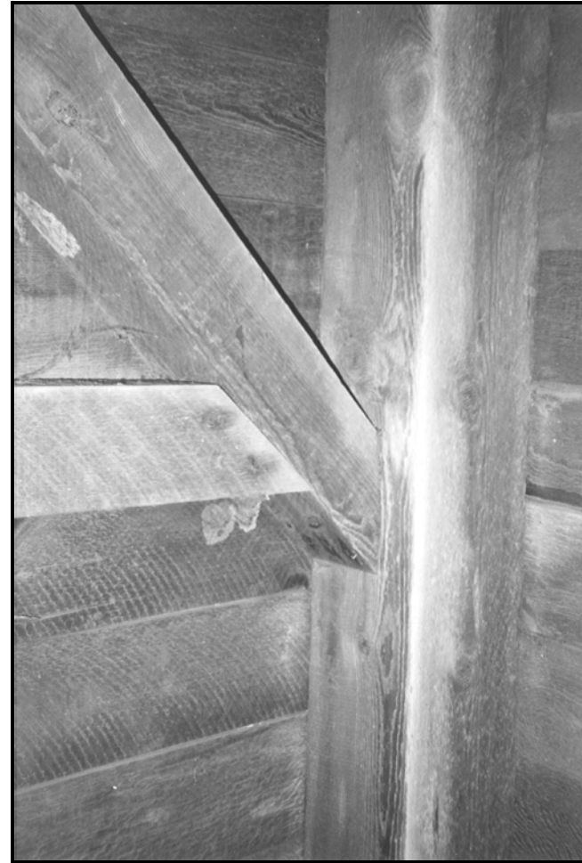
Figure 17. Additional framing details on the interior of the grain bins. In contrast to the north and south bents, the diagonal bracing on the two center bents are nailed together, rather than being connected with mortise and tenon. Note the heavy cross bracing used on the walls of the grain bins. The walls bore a great deal of weight and pressure when the bins were filled with grain (FRR October 2002).
