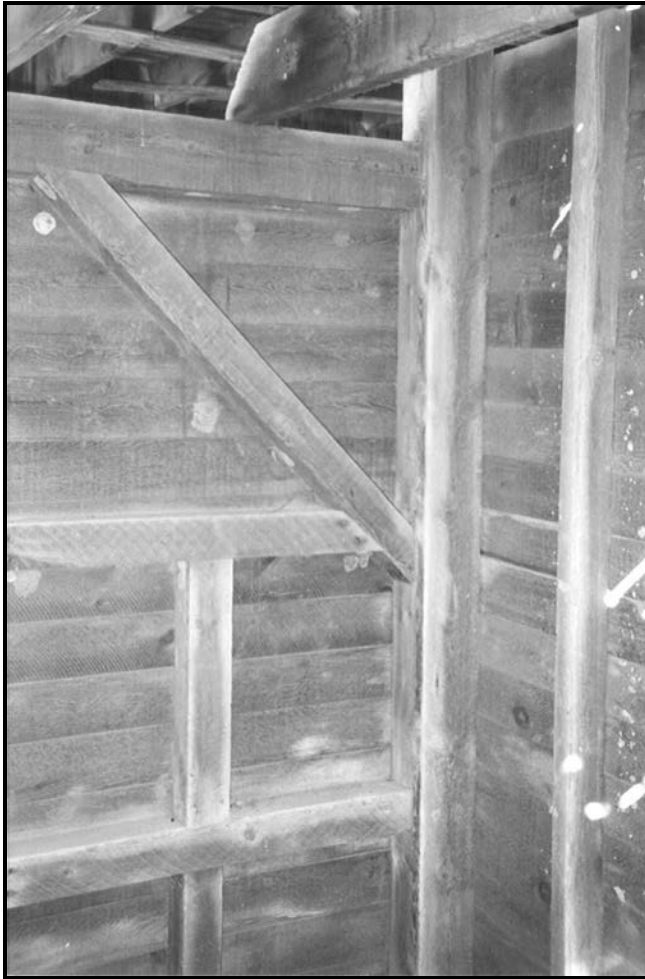
Figure 17. Additional framing details on the interior of the grain bins. In contrast to the north and south bents, the diagonal bracing on the two center bents are nailed together, rather than being connected with mortise and tenon. Note the heavy cross bracing used on the walls of the grain bins. The walls bore a great deal of weight and pressure when the bins were filled with grain (FRR October 2002).
