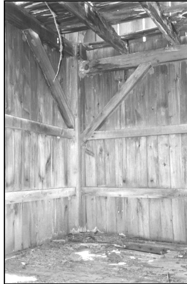
Figure 16. Framing details in the south bay of the barn. (LEFT) Larger framing members in the barn are joined with mortise-and-tenon joints, such as the pictured here, which connects a post and two girts in the interior bent along the south side of the central drive. (RIGHT) Interior view of easternmost grain bin, showing the framing at the southeast corner of the barn. The corner posts are supported by diagonal braces, set at 45-degrees, and by horizontal braces that double as nailers for the exterior siding (FRR October 2002).
