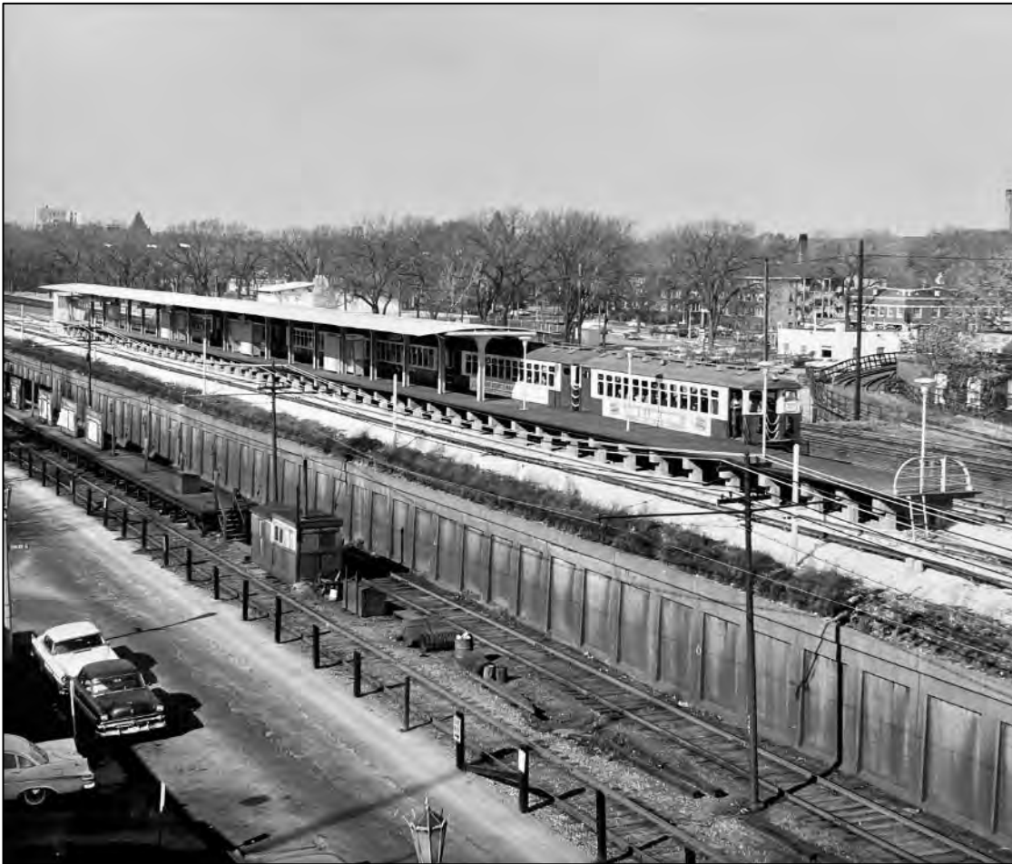
Figure 9: View of Ridgeland Station looking west (1962) showing the new platform and canopy on the embankment and the at-grades tracks. CTA Photo 366-62 #1.
