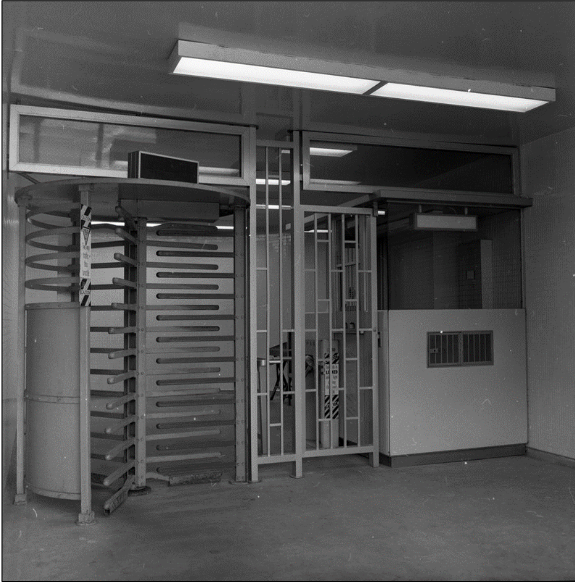
Figure 17: Interior view of the Secondary (Mason) Stationhouse, 1964. CTA Photo 437-64 #13.
