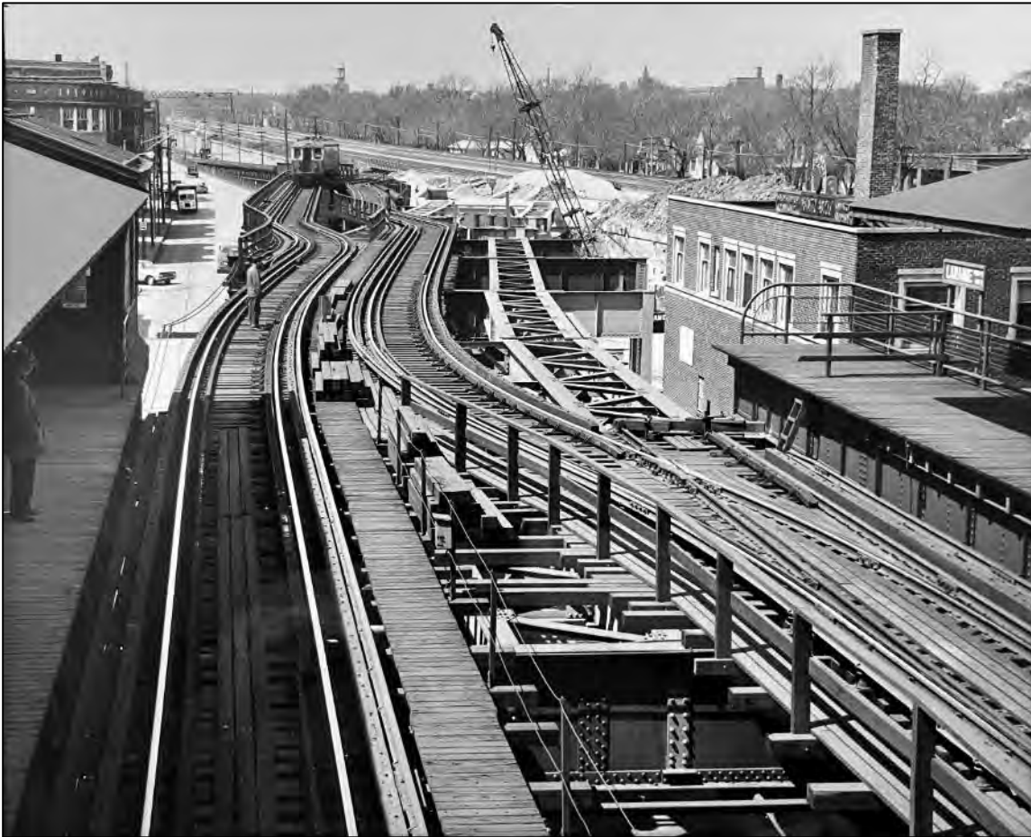
Figure 7: This 1962 view looks west from the Laramie Avenue Elevated Station. On the right a new steel structure connects the tracks to the Northwest Railway embankment. CTA Photo 182-62 #14.
