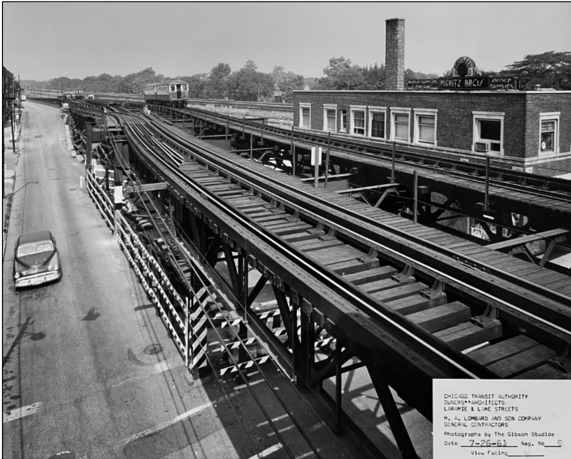
Figure 6: This 1961 photo (prior to work beginning) shows the elevated tracks west of Laramie Station, which parallel the Northwest Railway embankment on the right (north). In the distance on the left is the ramp down to the at-grade portion of the line. CTA Photo from general contractor (No. 9).
