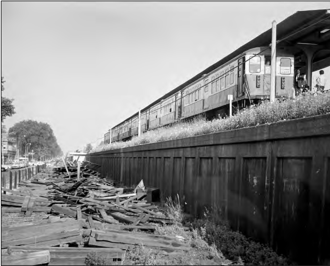
Figure 12: Demolition of the Oak Park station, platform and canopy with completion of the new Oak Park Station, 1963. CTA Photo 266-63 #12.
