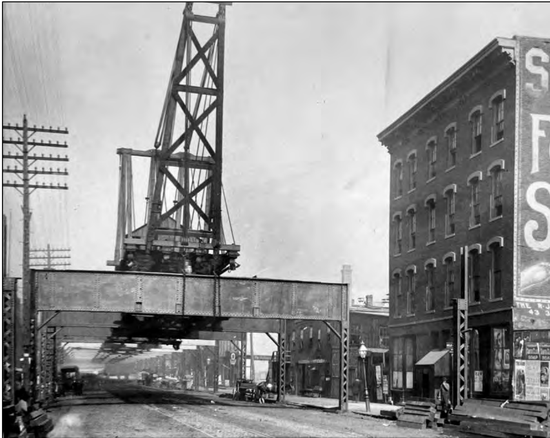
Figure 2: View of the 1892 construction of the Lake Street L between N. Halsted Avenue and N. Western Boulevard. Collection of George Krambles. CTA Photo H292.
