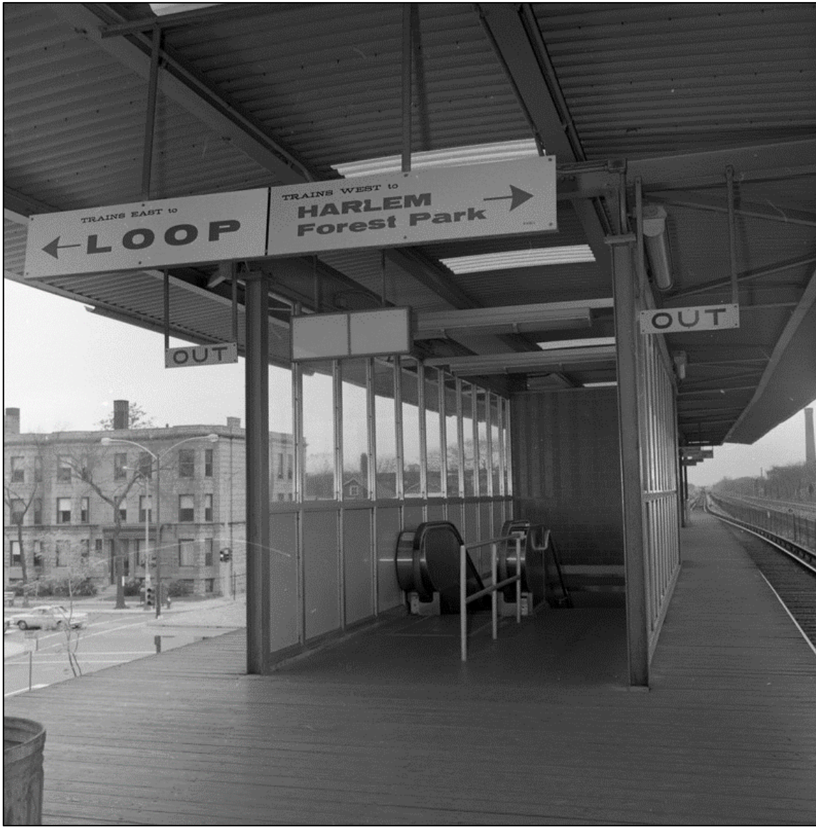
Figure 18: View of the Austin Station platform enclosure with stairs and escalator in 1964. CTA Photo 437-64 #8.
