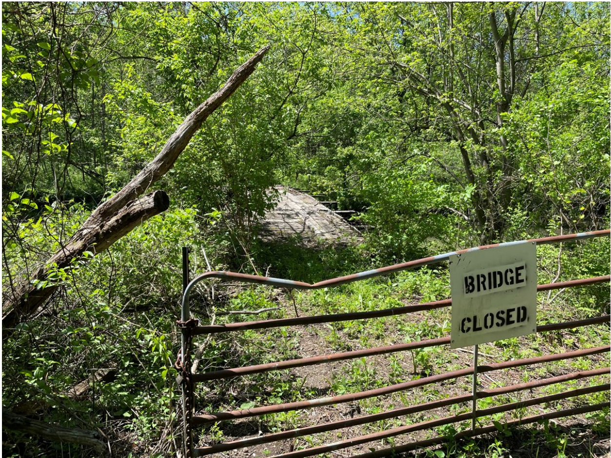
Figure 2. Approach view of the footbridge looking south from the north bank of Jackson Creek. Photograph by Joseph S. Murphey, USACE.
