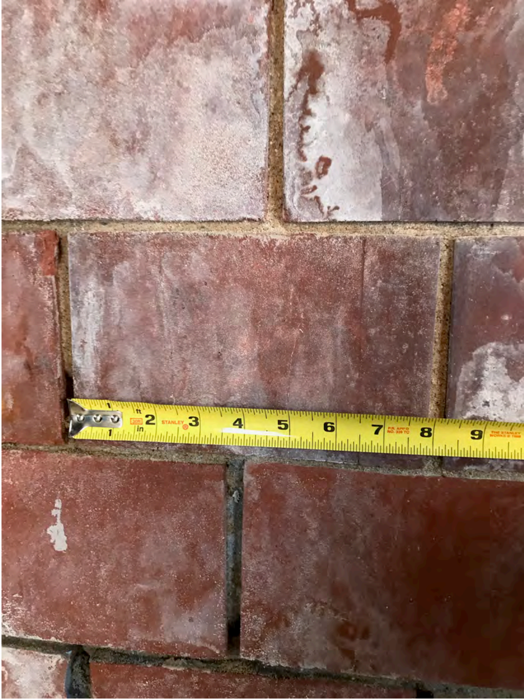
HAER No. IL-1201-17: 14" Pumphouse wall
