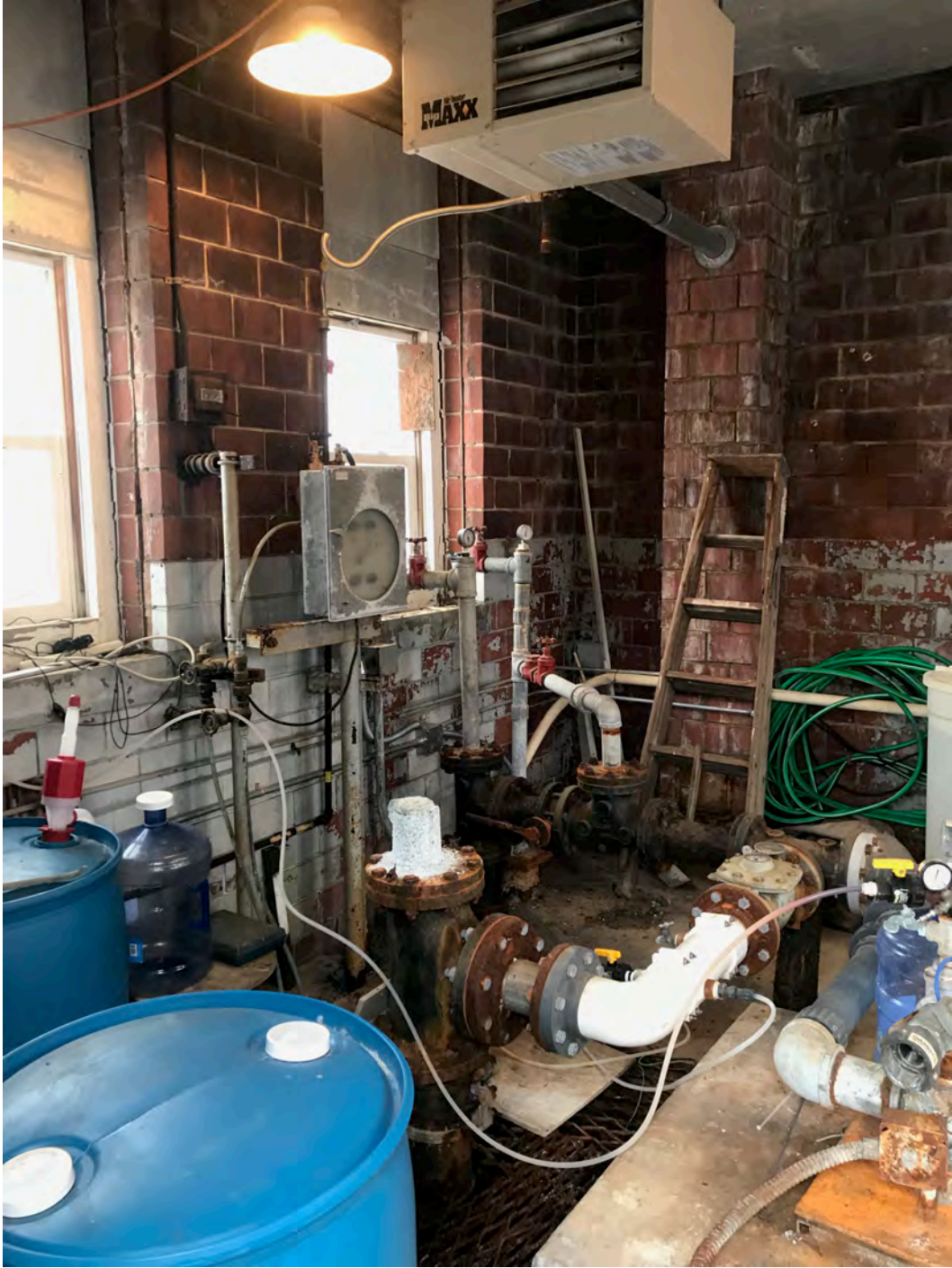
HAER No. IL-1201-14: Pumphouse interior 1
