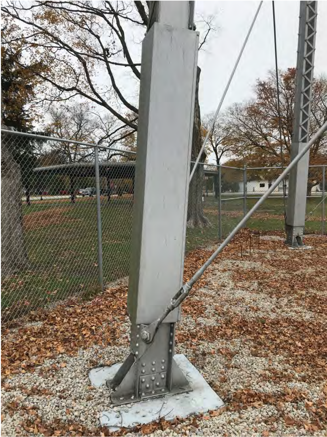
HAER No. IL-1201-21: 14" Plate connecting tower rod to base of column
