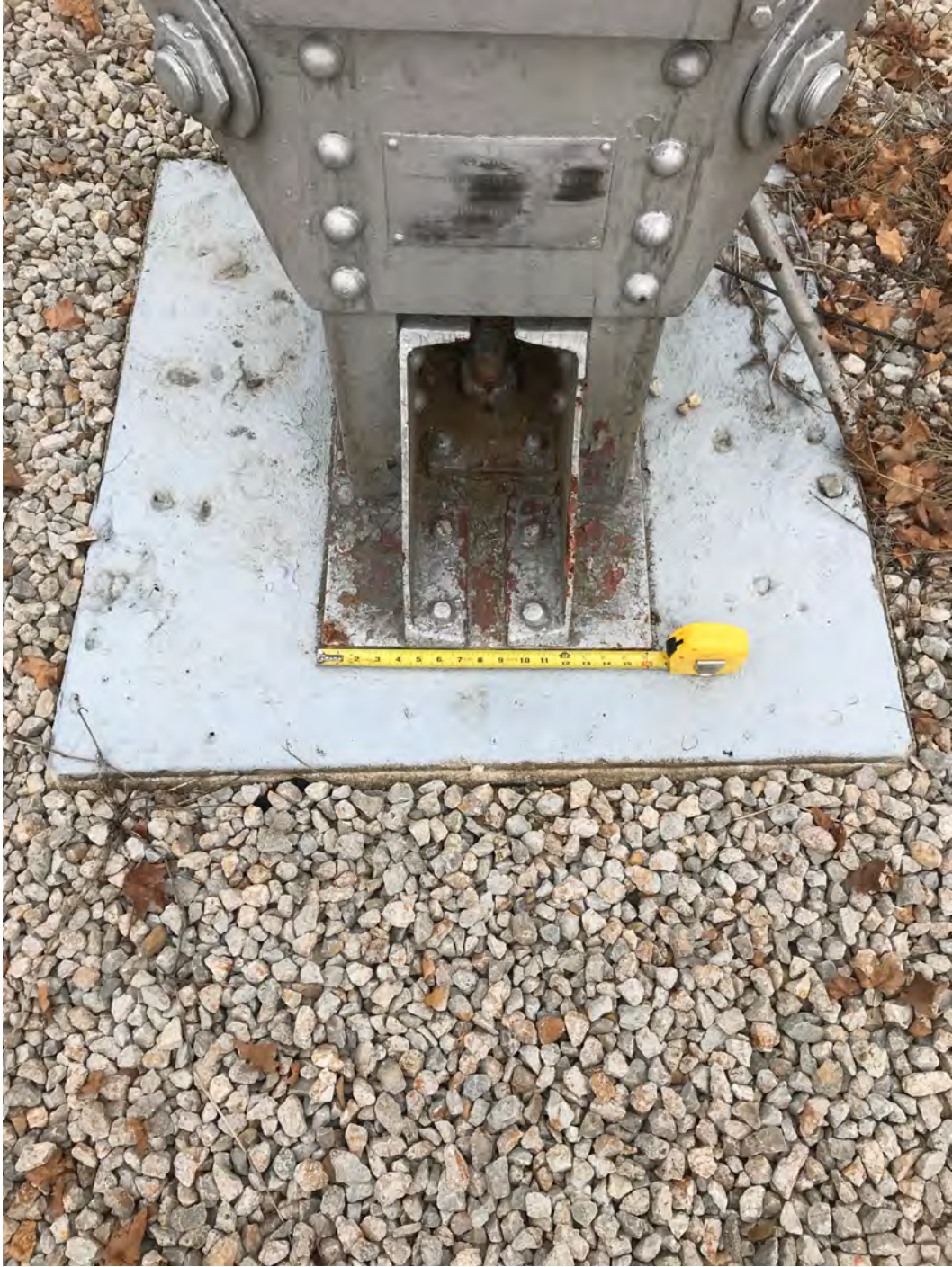
HAER No. IL-1201-25: Column boot and anchor bolt
