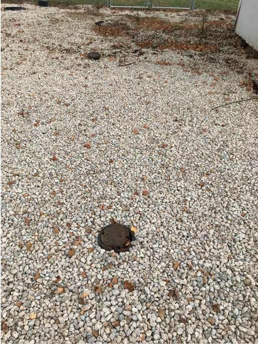
HAER No. IL-1201-24: Capped water pipes
