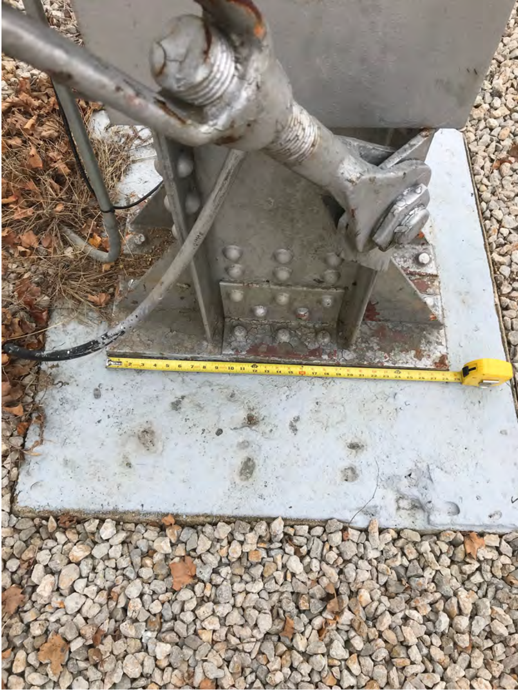
HAER No. IL-1201-26: Side view of column boot and tower rod
