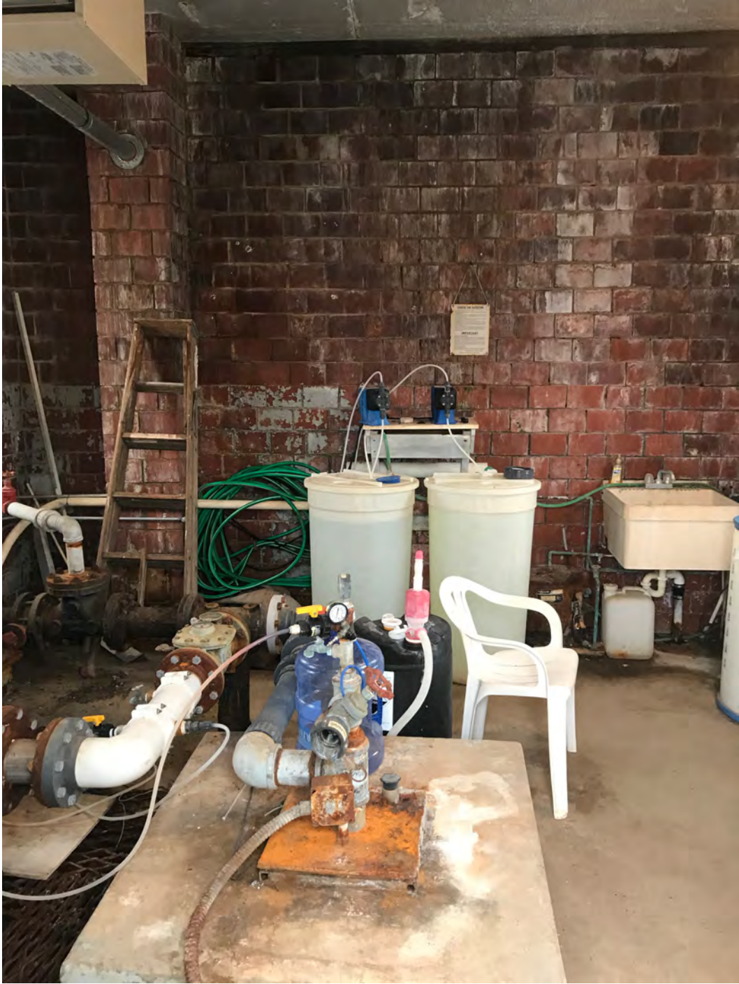
HAER No. IL-1201-15: Pumphouse interior 2
