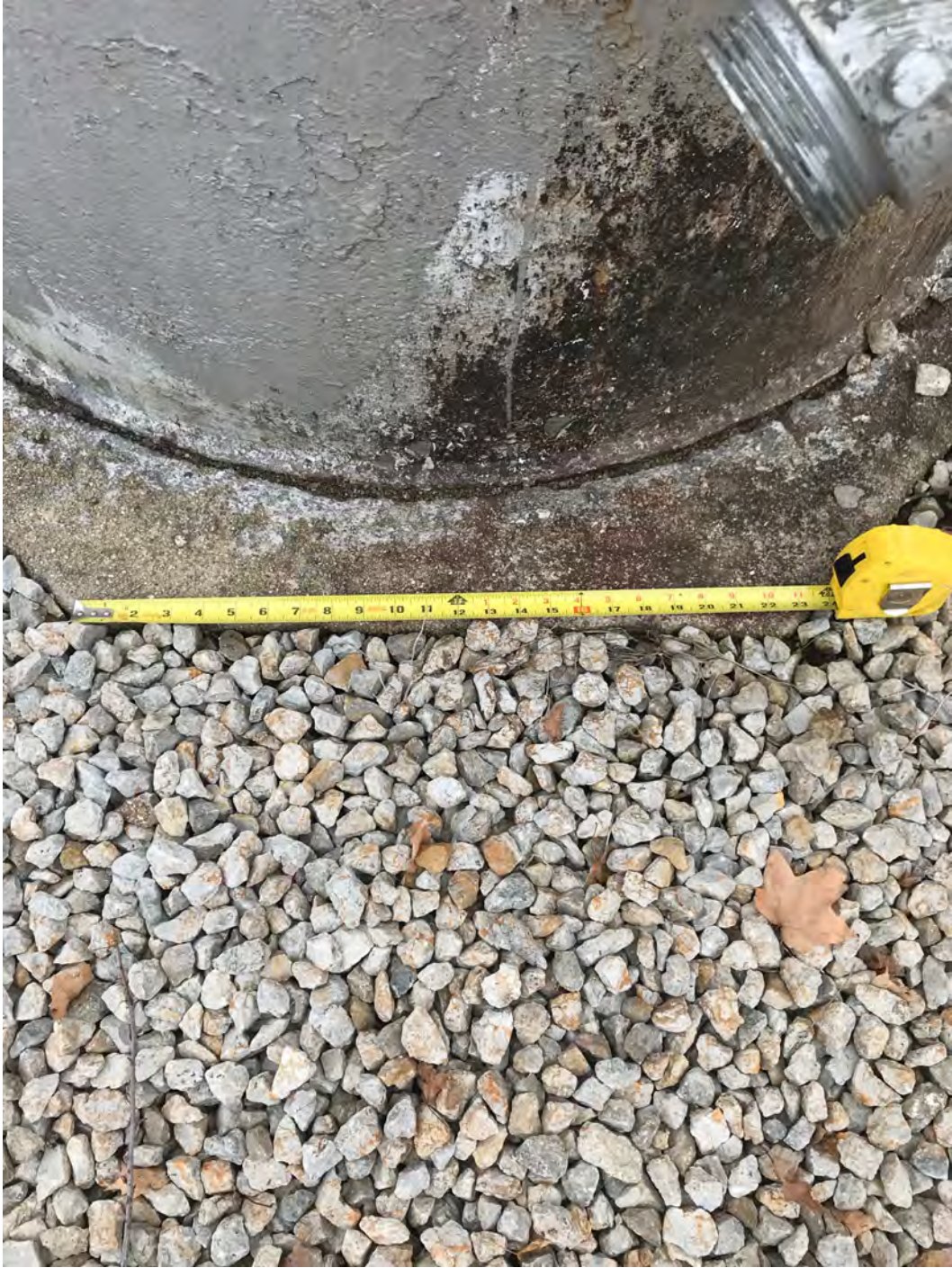
HAER No. IL-1201-22: Octagonal riser foundation, 23" on each side
