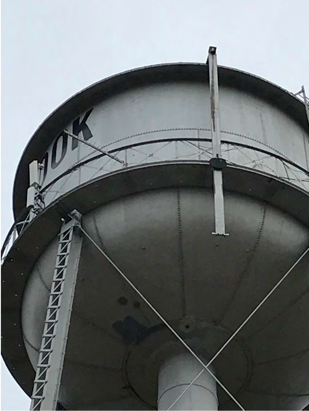
HAER No. IL-1201-28: Connection of column to balcony and tank
