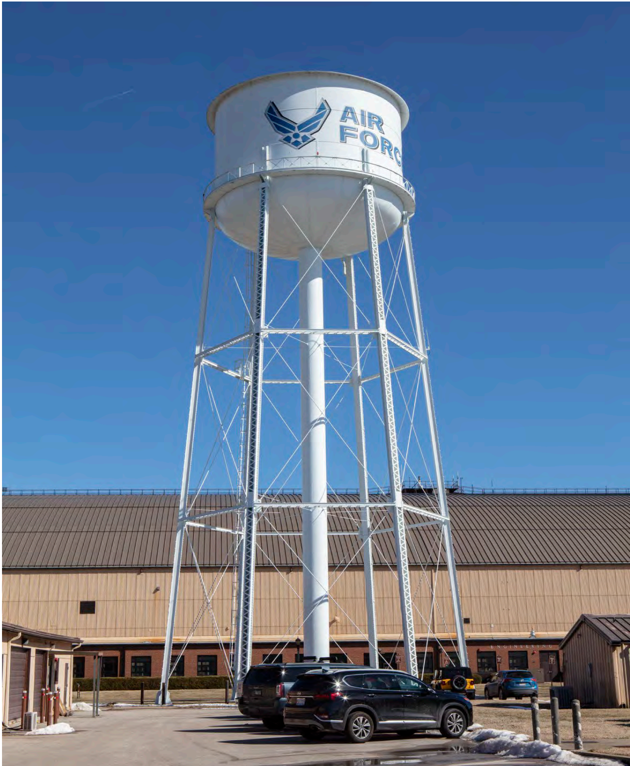
Figure 8: View of Water Tower 8020 looking east from the parking lot immediately to the west of the tower, January 2020.
