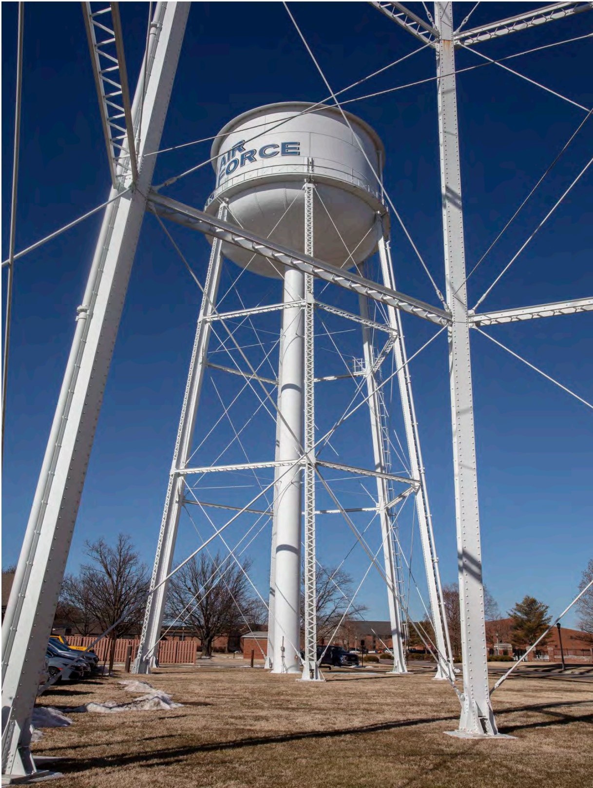
Figure 10: View of Water Tower 8020 looking north from the center of Water Tower 8010, January 2020.
