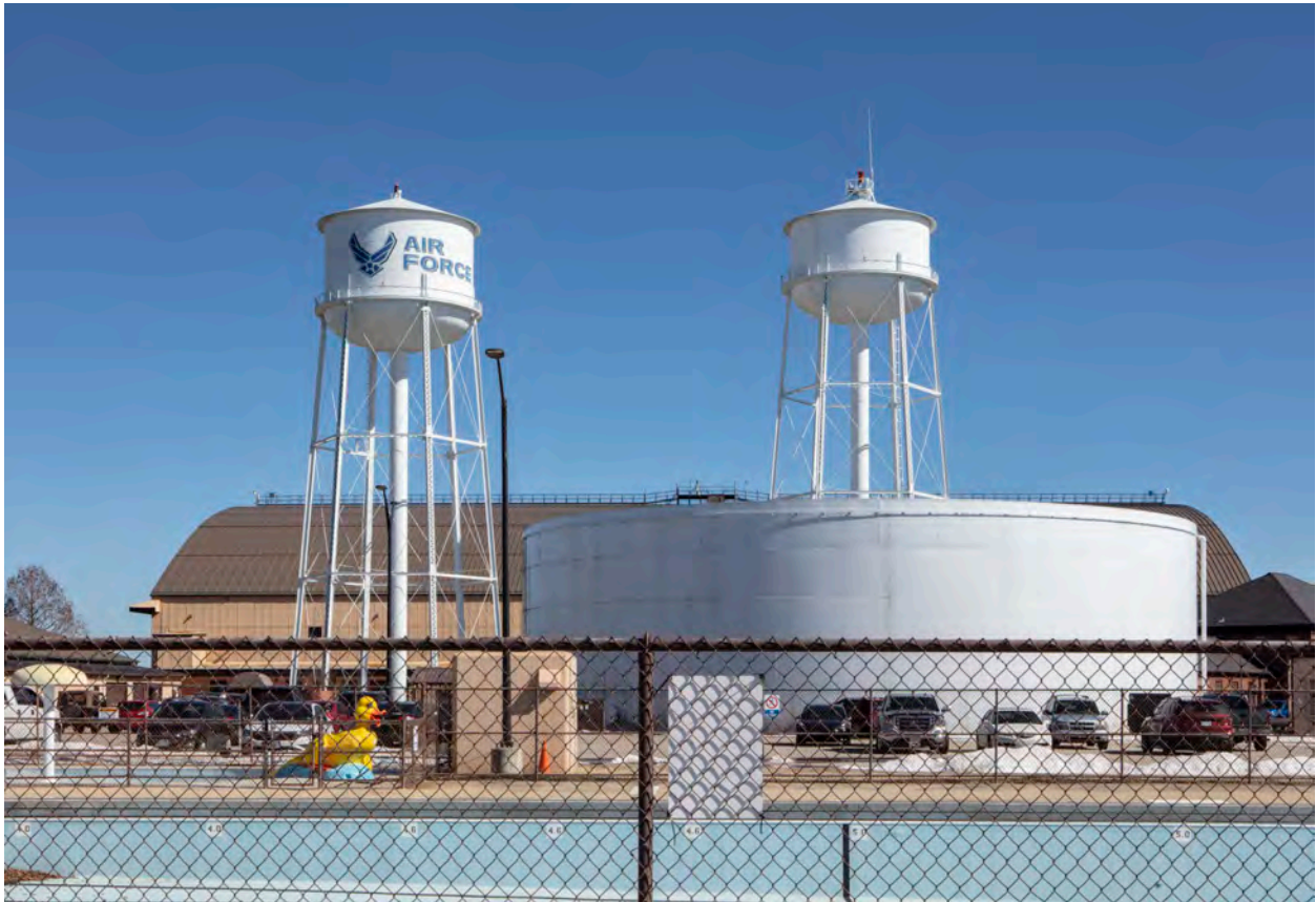
Figure 5: View of Water Towers 8010 and 8020 looking east from E Street, January 2020.
