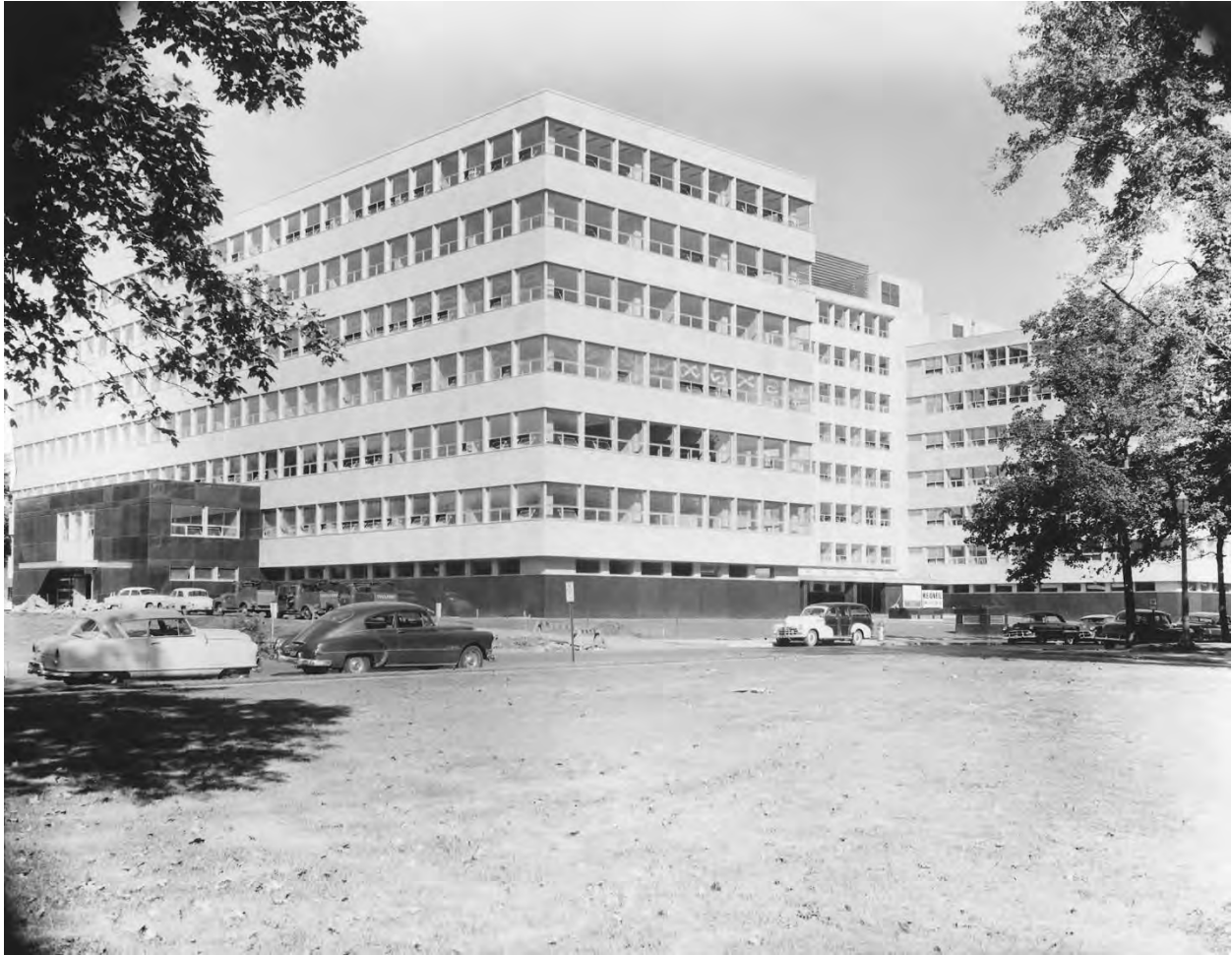
Figure 17. The building nears completion, 1955, view from the southeast. Source: Sangamon Valley Collection, Lincoln Library, City of Springfield.
