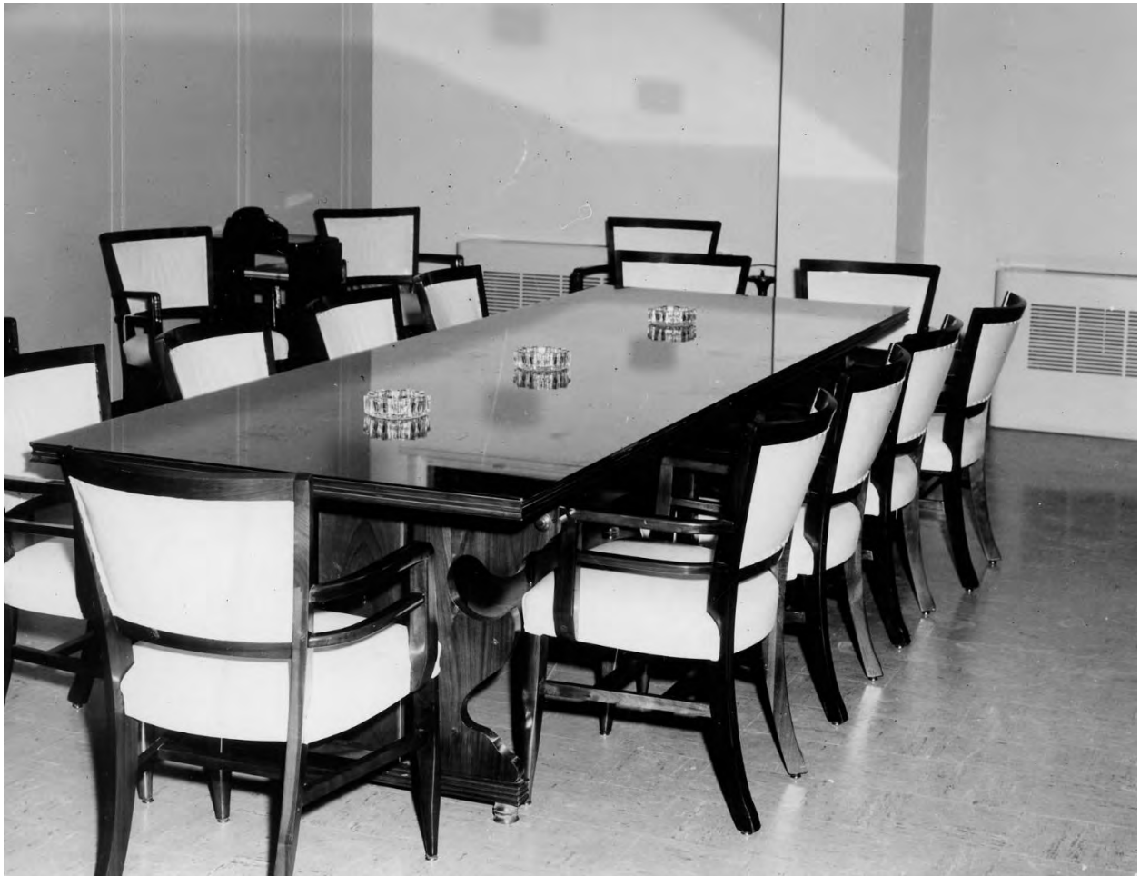
Figure 7. Conference room, circa 1956. Source: Sangamon Valley Collection, Lincoln Library, City of Springfield.
