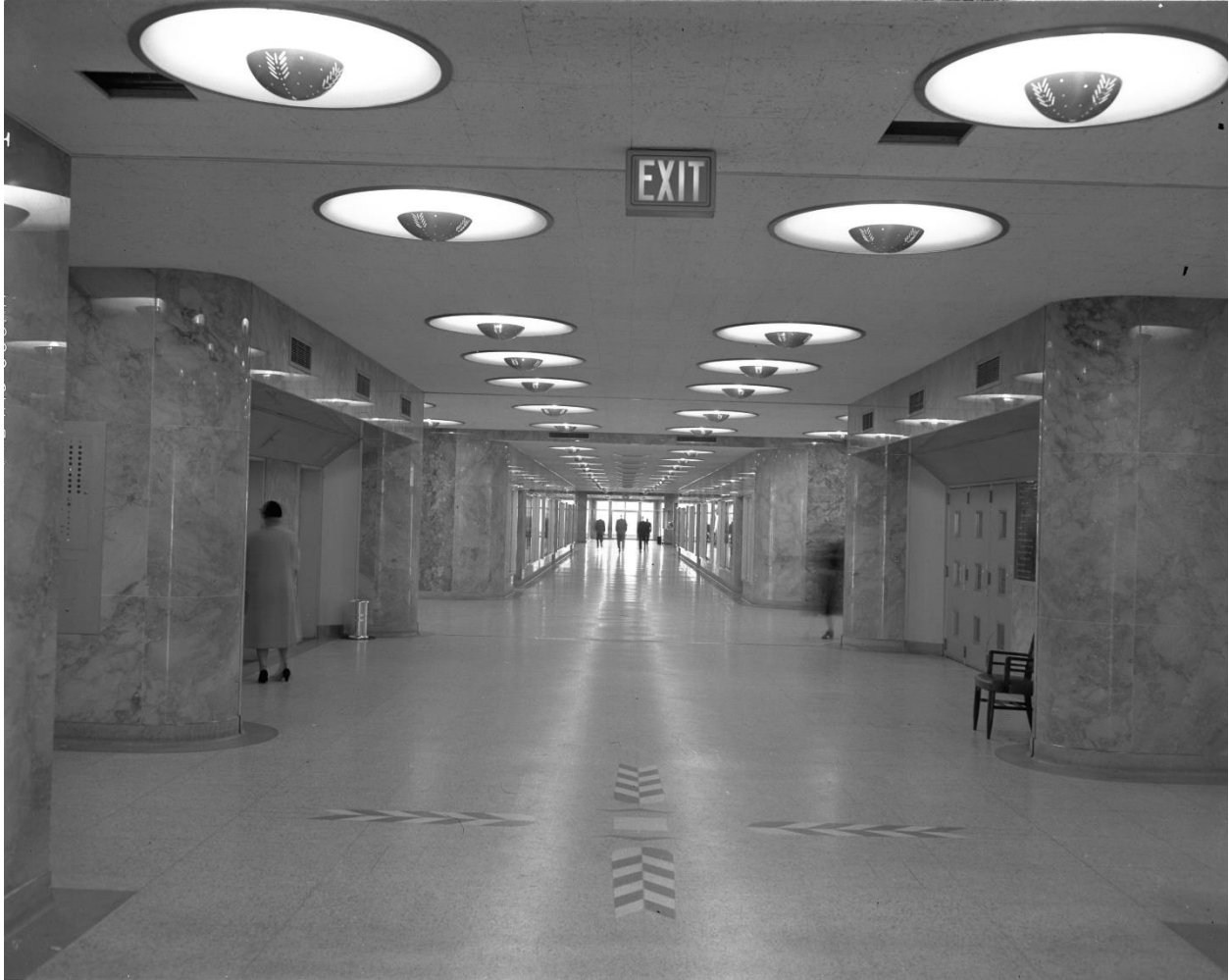
Figure 1. First floor main corridor, looking north, circa 1956. Source: All images from Architect of the Capitol files unless noted otherwise.
