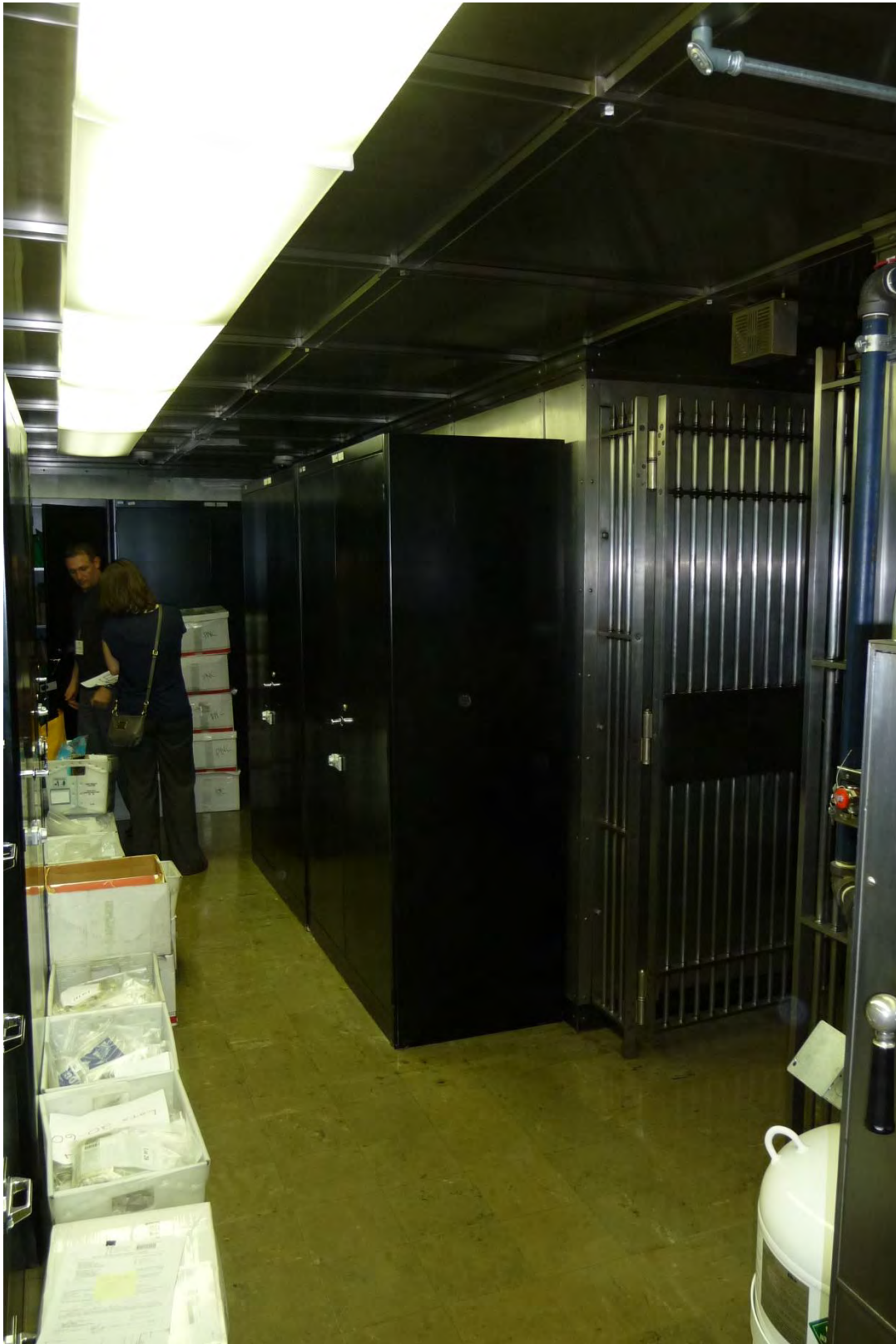
Figure 33. Inside Treasurer's vault at south door, facing north.
