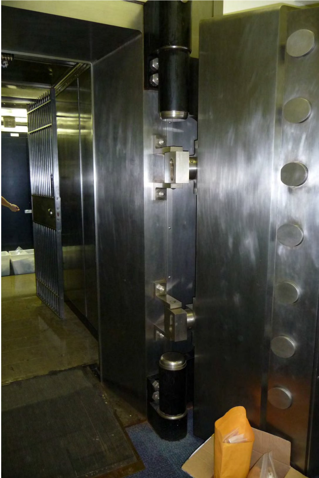
Figure 31. Detail of South door of Treasurer's vault, facing west.
