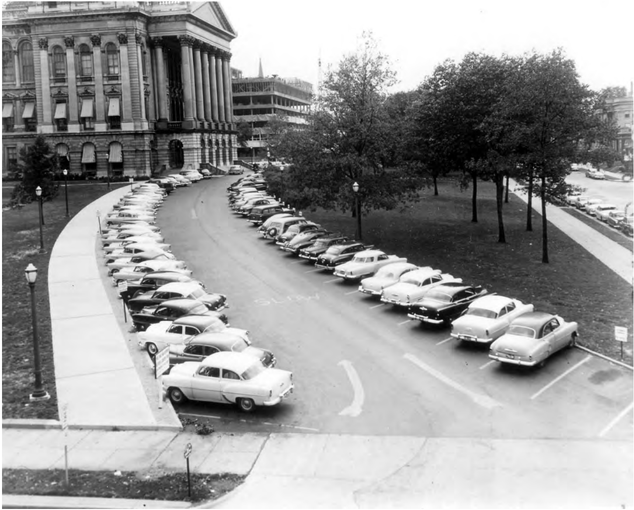
Figure 25. View of the north approach drive after widening, 1955.
