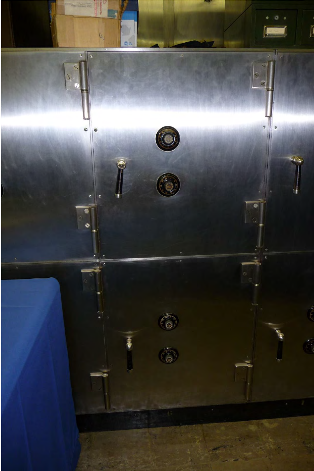
Figure 38. Detail of exterior face individual safe, within Treasurer's vault.
