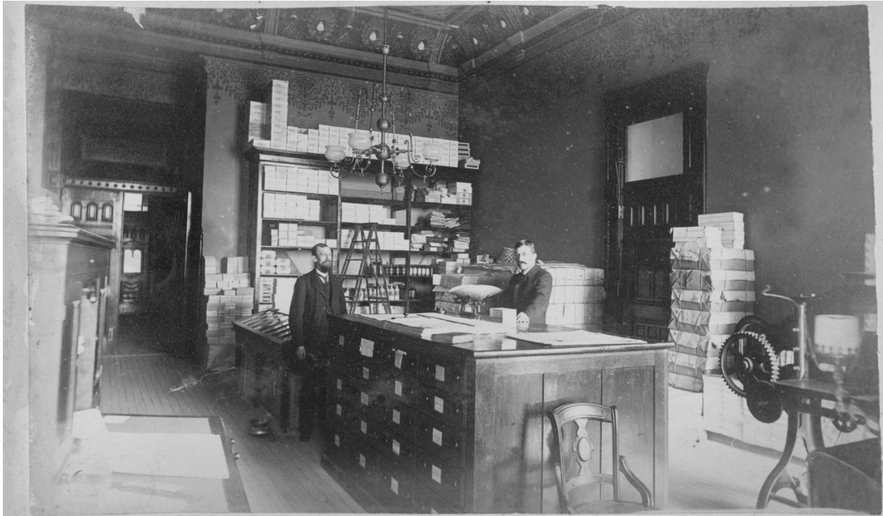
Figure 3. Photograph dated 1886, showing the Shipping Department on the first floor of the Illinois Capitol. Image shows the original first floor plaster cornice and ceiling ornamentation, dating from era of W.W. Boyington's work on the first floor of the Capitol during the 1880s. This ornamentation is the same as shown in repair drawings dated October 10, 1923. See Figure 27 and Figure 28 below.
