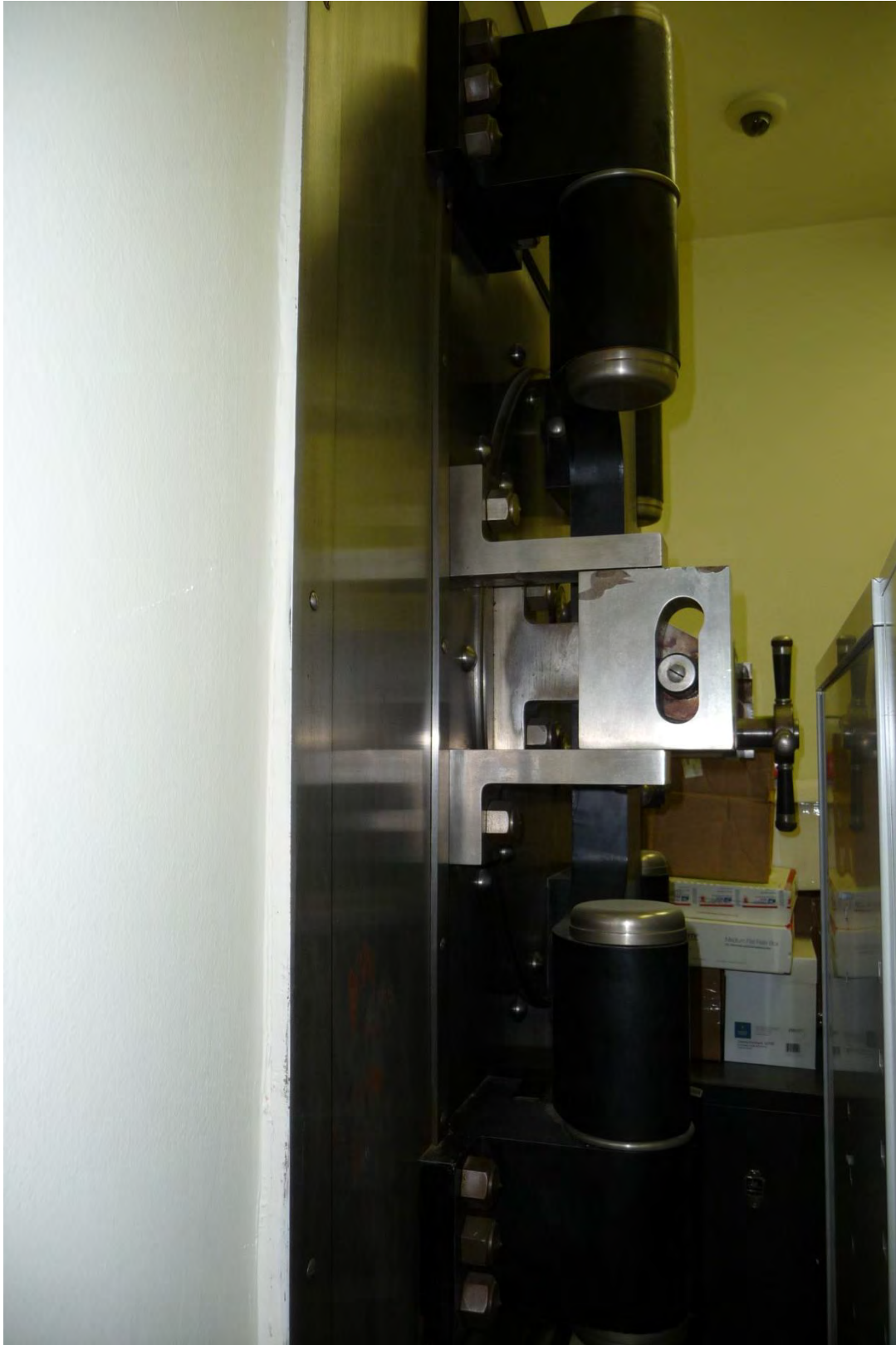
Figure 32. Detail of Treasurer's vault south door hinge.
