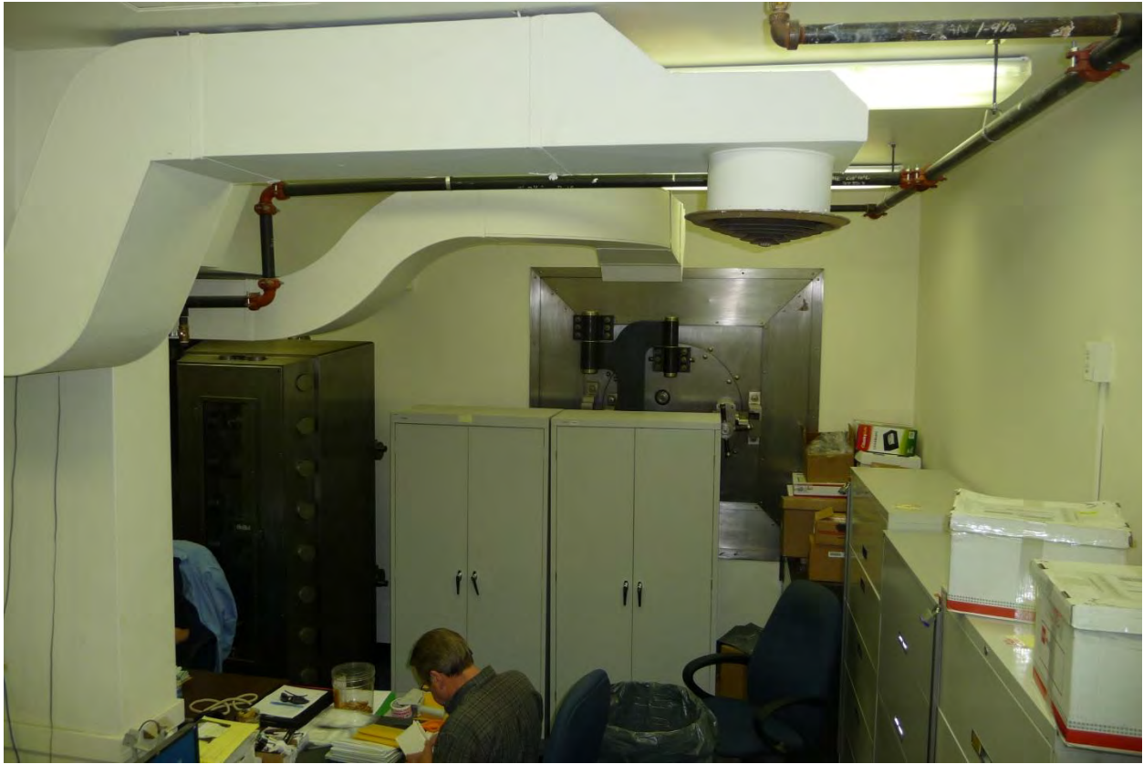
Figure 29. Bank Vault Ante Room, within North Wing of original Capitol, facing west toward north door to non-original, external subgrade Treasurer's Vault. Figure 29 through Figure 38 were taken by the HABS project team prior to the demolition of these vaults.
