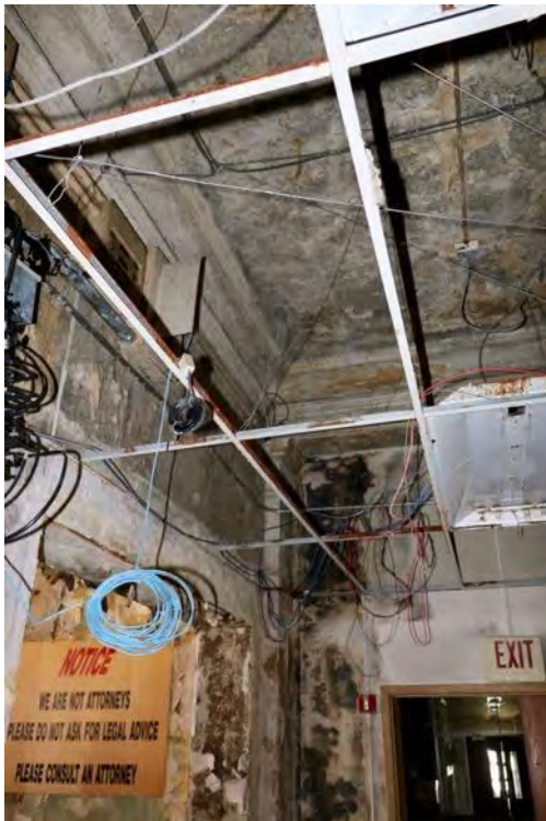
Exhibit N - Original plaster cornice in second floor corridor
