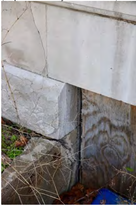
Exhibit A - Detail of Carthage Marble water table
