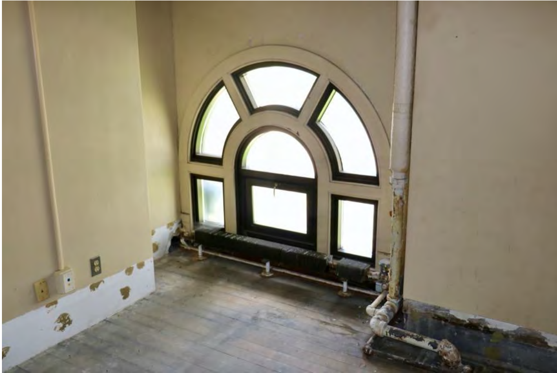
Exhibit H - Second floor office with original arched window
