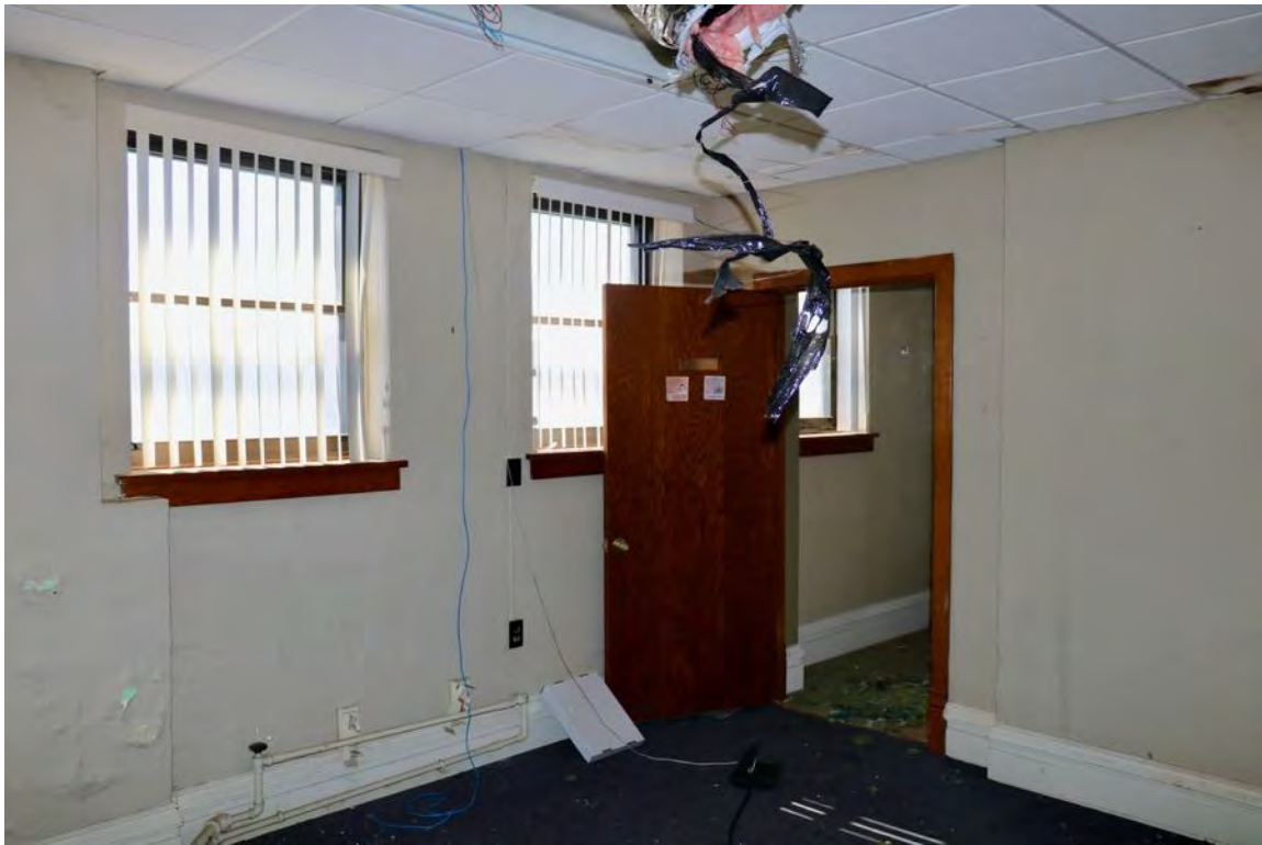
Exhibit U - Fourth floor office
