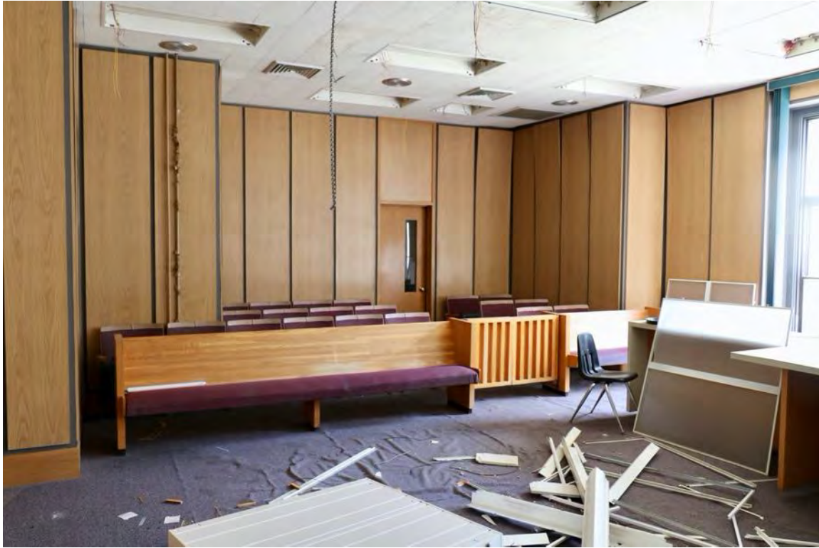
Exhibit J - Second floor northwest courtroom, showing plastic laminate wall panels
