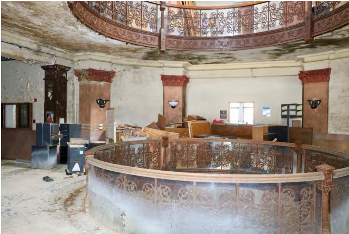
Exhibit P - Third floor rotunda, looking east
