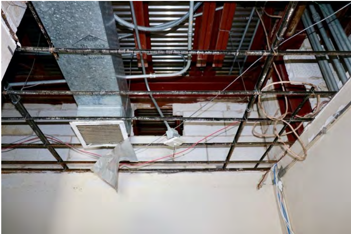
Exhibit S - Third floor wall construction of Pyrobar fireproofing blocks
