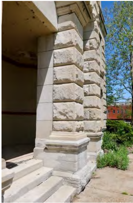
Exhibit B - Detail of south porch, showing blue and buff Bedford stone
