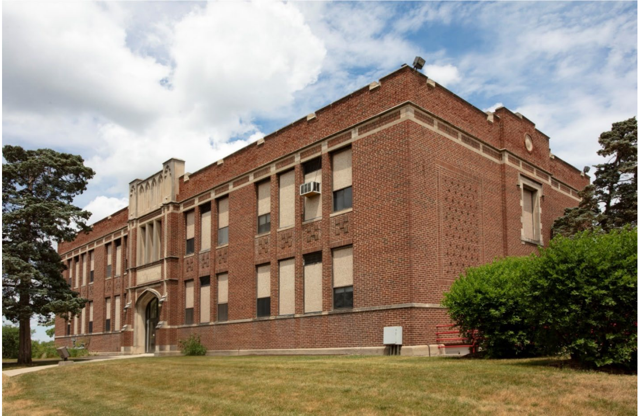
Figure 3. West façade of original 1929 building, view looking northeast. (JLK Architects, 2021)
