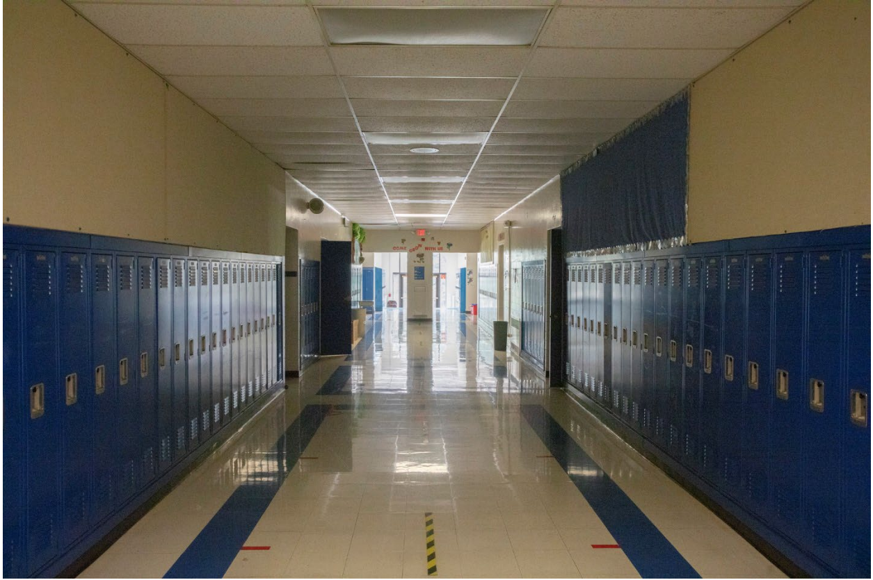
Figure 7. Interior view of hallway and student lockers within 1952 addition, view looking southeast toward south entrance. (JLK Architects, 2021)
