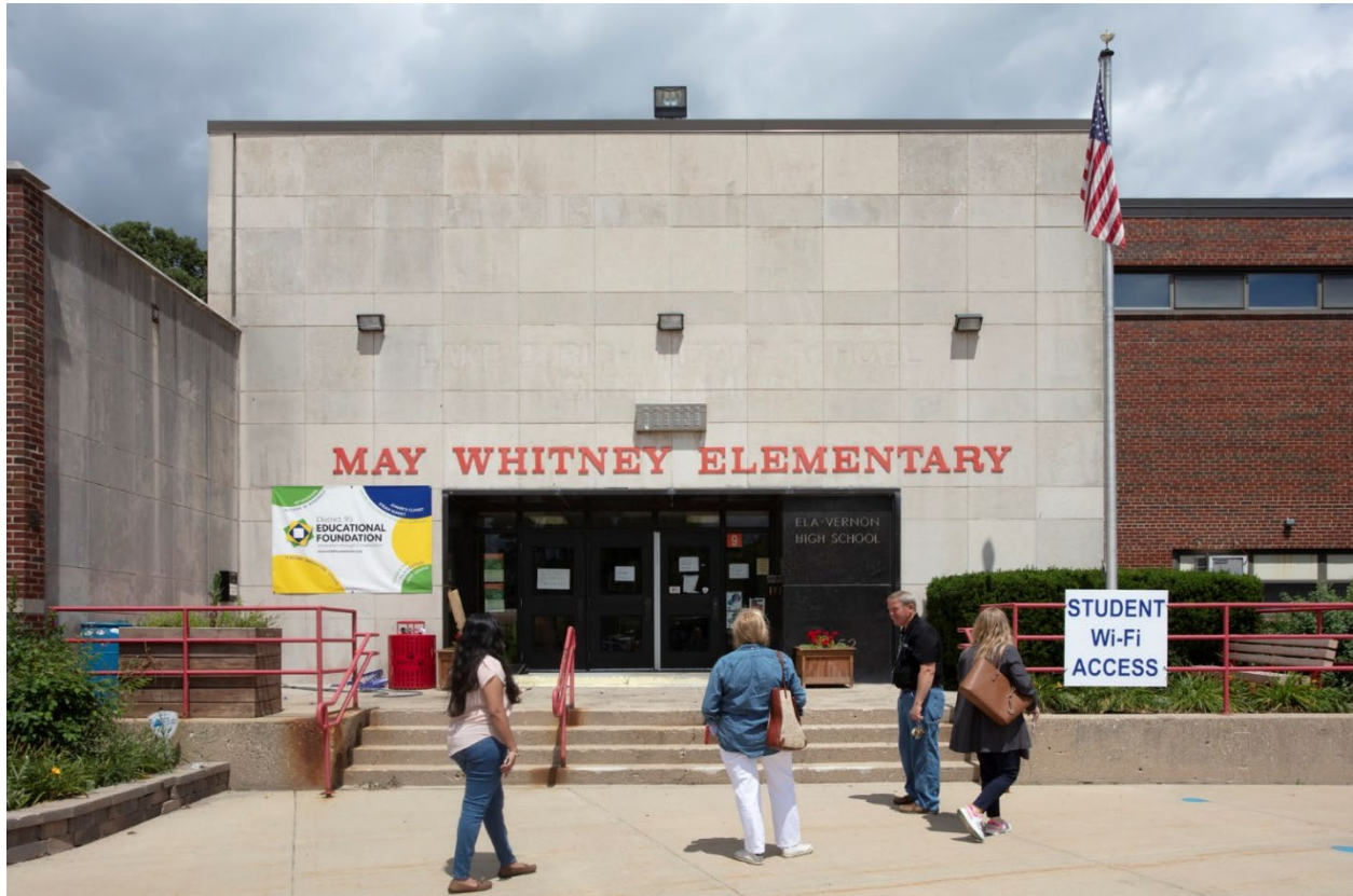
Figure 1. North entrance at 1952 addition, view looking northwest. (JLK Architects, 2021)
