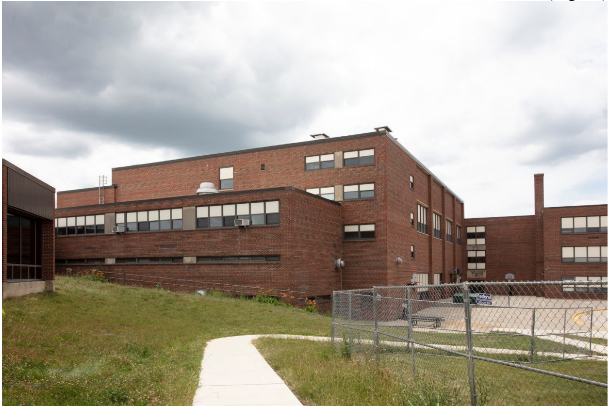
Figure 5. East façade of 1952 addition, view looking southwest. (JLK Architects, 2021)
