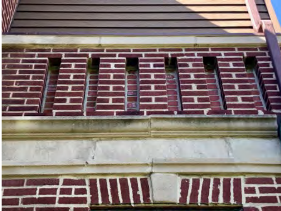
View of rear balcony parapet, showing later brick infill
