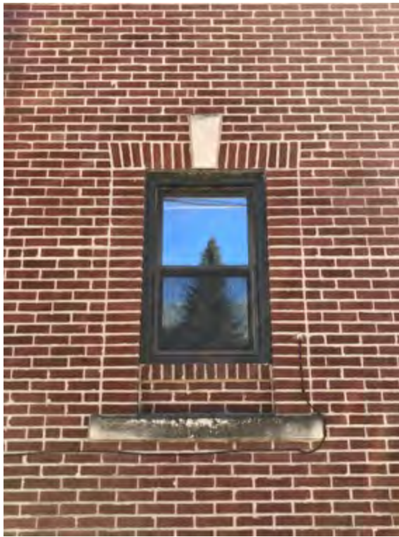
North kitchen window, showing brickwork surround
