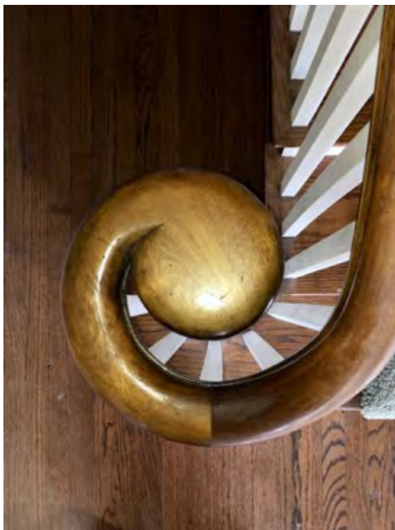
Stairway detail, showing volute
