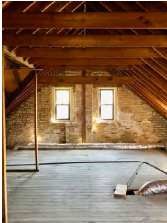
Attic, looking south
