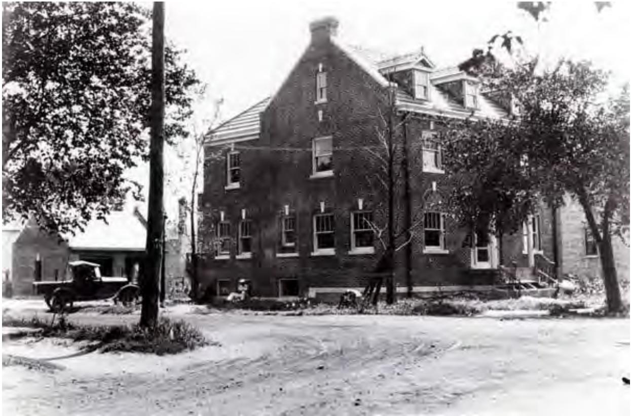
1926 photo during construction, looking southeast.
