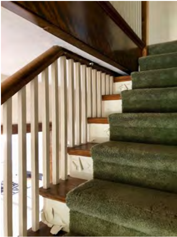
Stairway detail, showing transition from first floor to second
