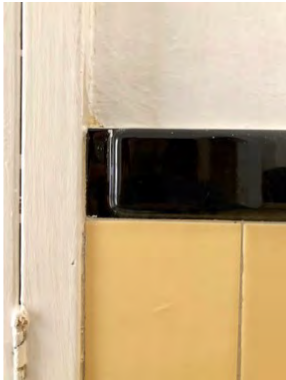
First floor powder room, original tile detail
