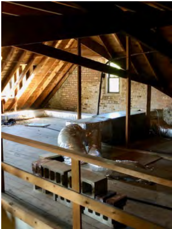
Attic, looking northwest
