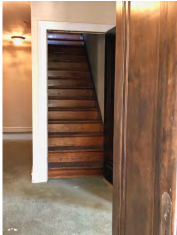
Second floor hall looking east from hall bath to attic stairs
