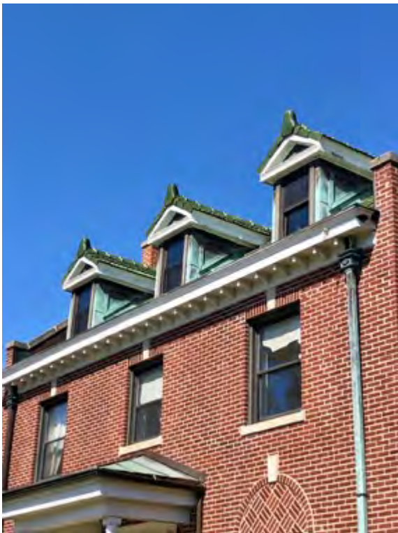
Front façade detail, showing cornice and dormers
