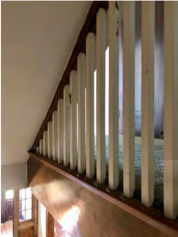
Detail of balusters under attic stairway
