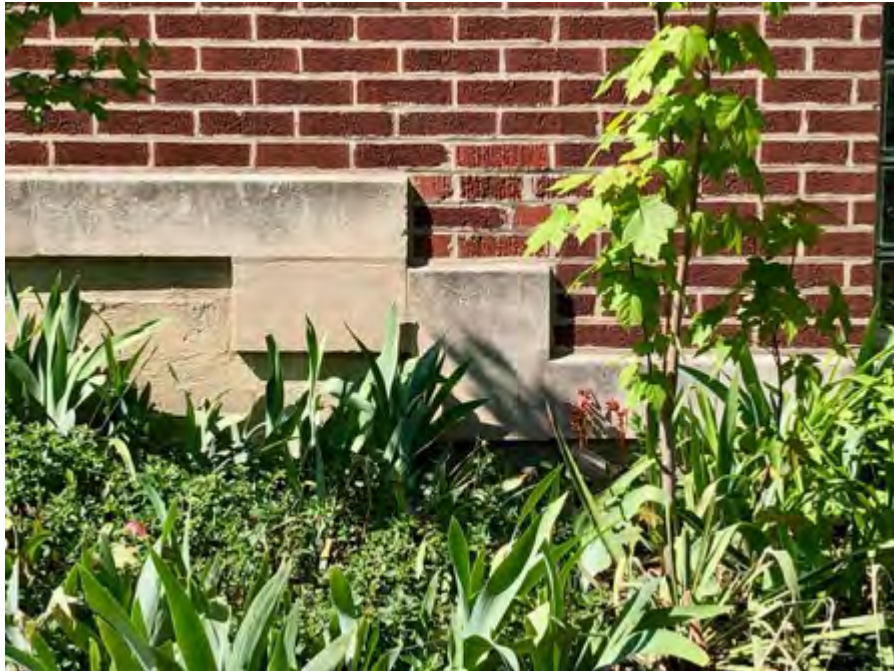
Detail of water table, showing step-down in levels
