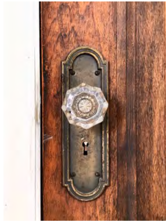
Original door hardware throughout house
