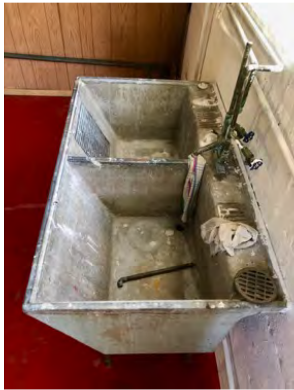
Detail of original laundry sink on north wall
