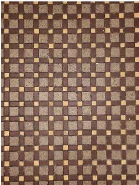
First floor powder room, original tile floor detail
