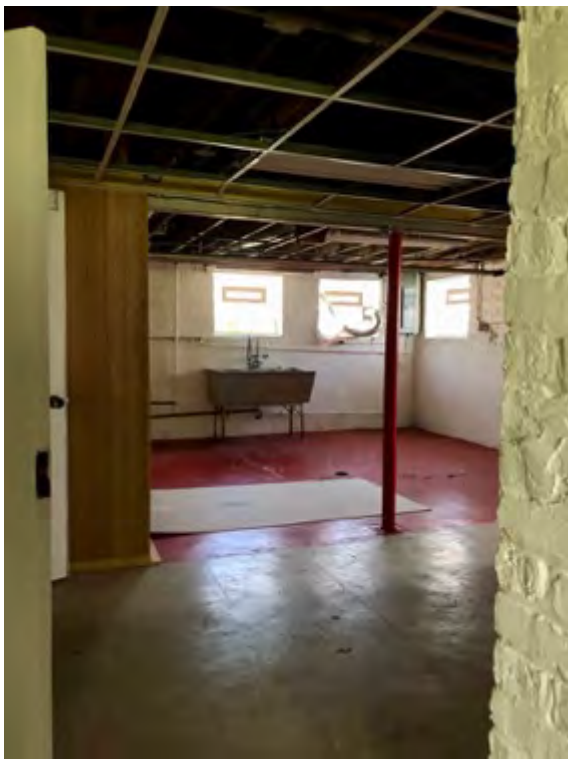
Basement laundry room, looking north
