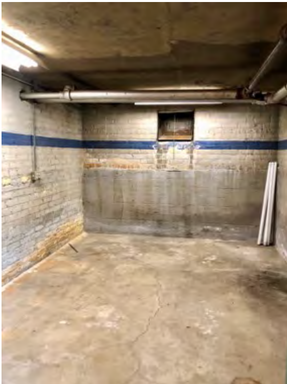
Coal room looking east, showing poured concrete footings with brick above
