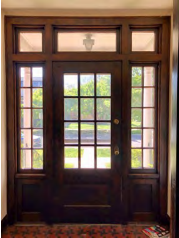
Front door from vestibule, looking west
