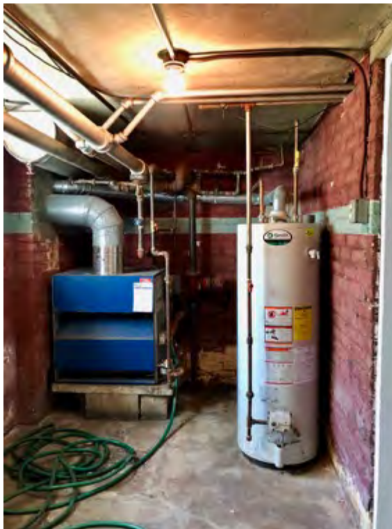
Furnace room looking west
