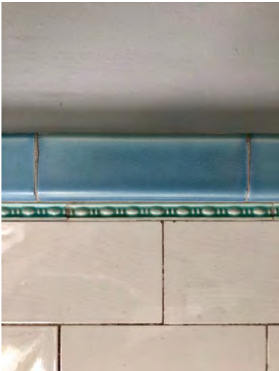
Second floor hall bath, detail showing original trim tiles
