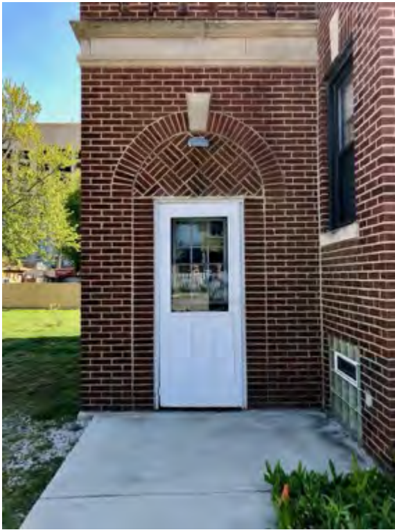
Rear entrance, showing blind arch with basketweave brickwork
