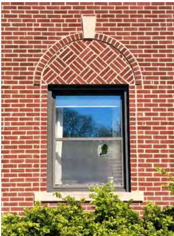
Front façade window, showing blind arch with basketweave brickwork
