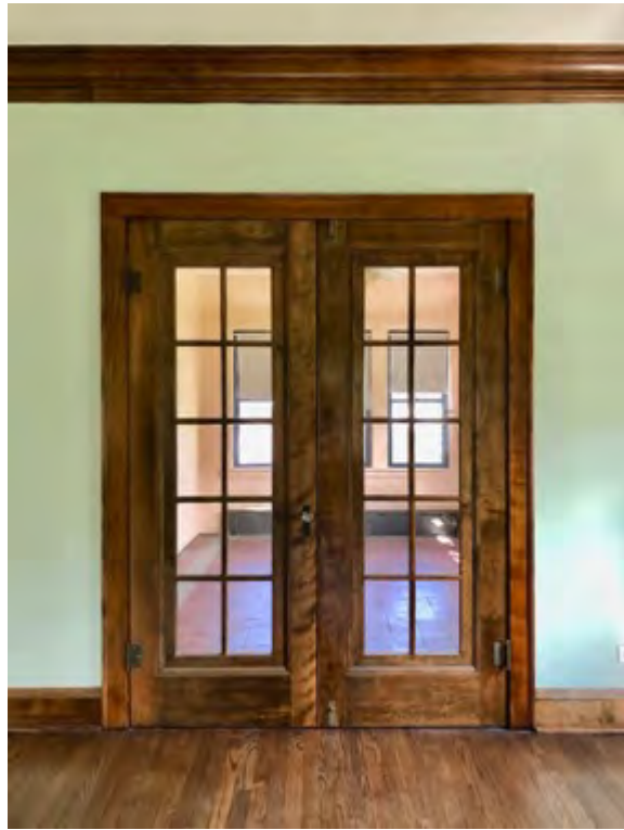
French doors from living room into sun room, looking east
