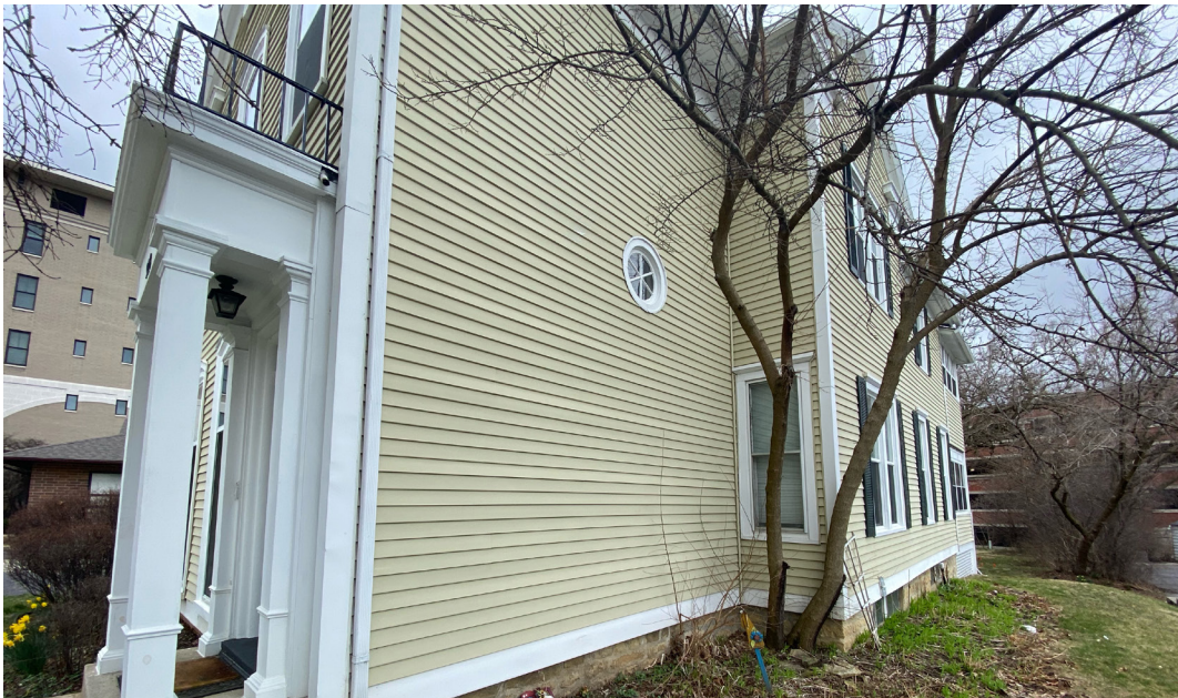
6: General view of the east side of the house, taken from the southeast corner. Image includes detail of the portico at the main entrance, and a divided light circular window is at center.
