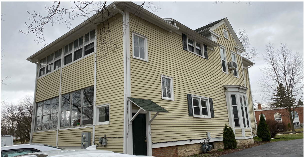
4: Oblique view of the north and west sides of the house. The two-story sleeping porch, rear entrance to the house, and foundation is visible in the foreground. The dining room bay window is visible in the background.
