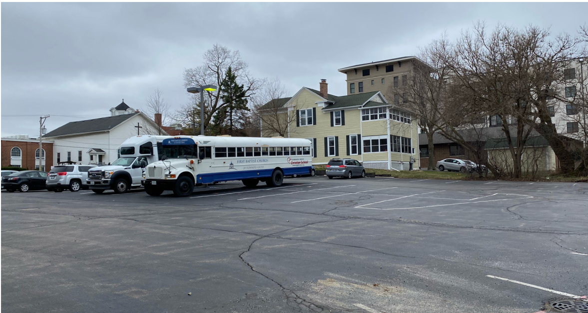
8: General view of the east and north walls in the background. The image includes a view of a surface parking lot in the foreground, which is owned by a neighboring church.
