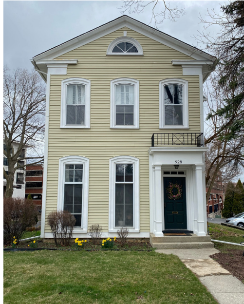
1: General view of the primary south facade of the house. Looking north. Features associated with the 1940 remodel are present, including a semi-circular window, cornice returns, and portico to the main entrance with a transom window.
