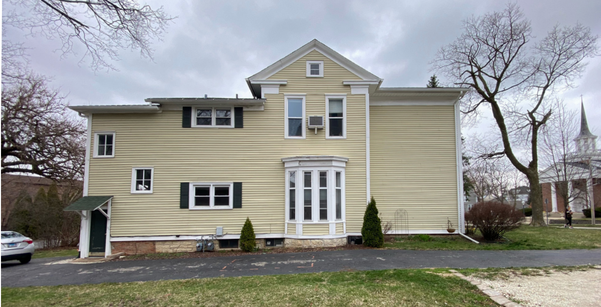
3: General view of the west wall of the house. A portion of limestone and brick masonry foundation is visible, and the rear entrance to the property is visible left of center.
