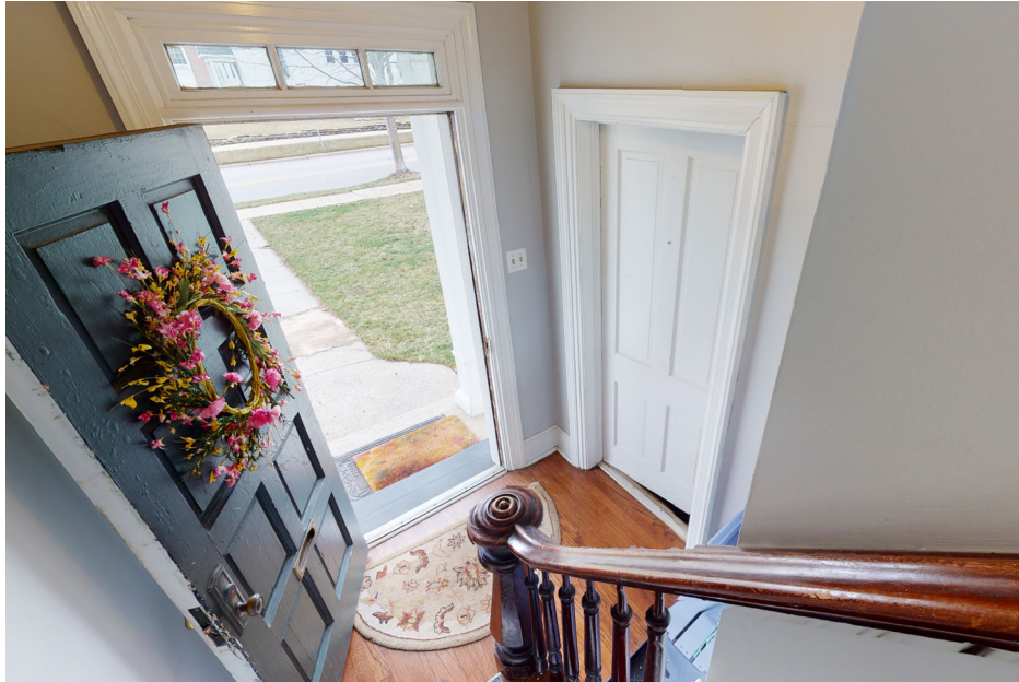
9: Close-up view of the interior entrance, vestibule, and staircase, looking south. A view of the original newel post and balustrade is present, and the interior door leading to the first floor living room is visible in the background.
