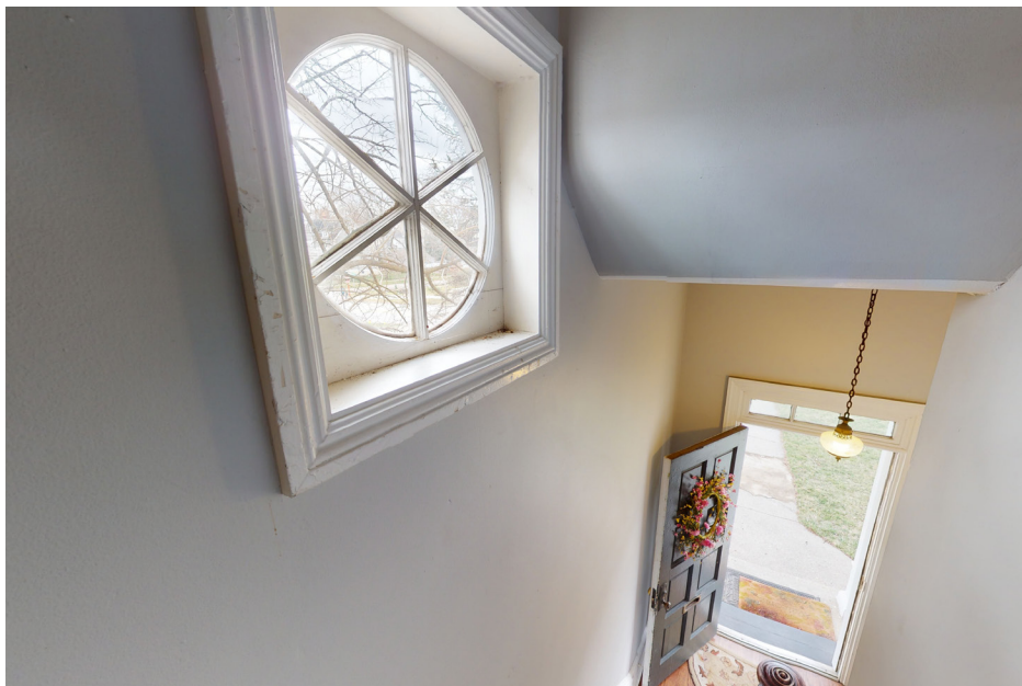
10: Close-up view of original divided light circular window in the main staircase, looking south. The main entrance is visible in the background.
