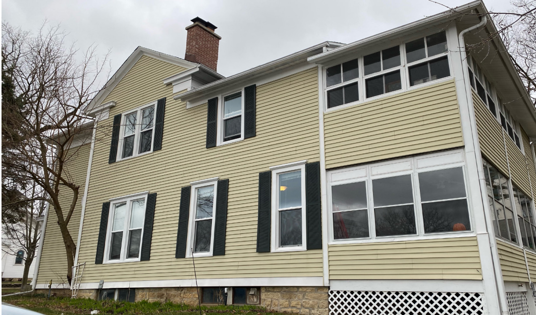
5: General view of the east and north sides of the house. The two-story sleeping porch extends to the north, and a large portion of the limestone foundation is visible.
