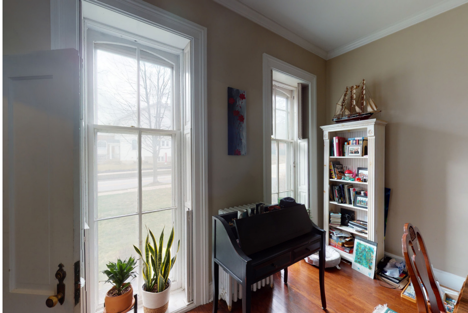
11: General view of first floor living room, looking southwest. Double-hung windows with arched upper sashes, interior shutters, and heavy casing are visible.
