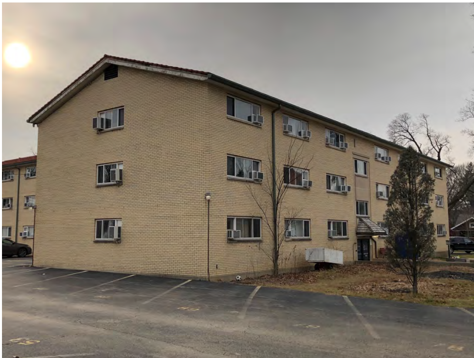
Figure 6: North wall, looking southwest
