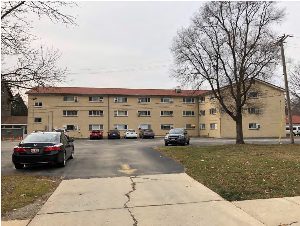
Figure 5: East side of the building, looking west
