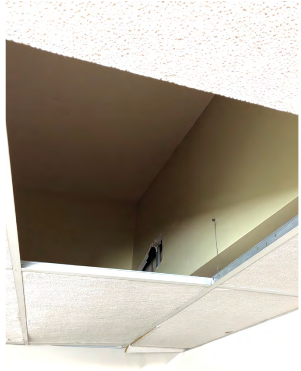
Figure 16: Original cathedral ceiling above dropped grid
