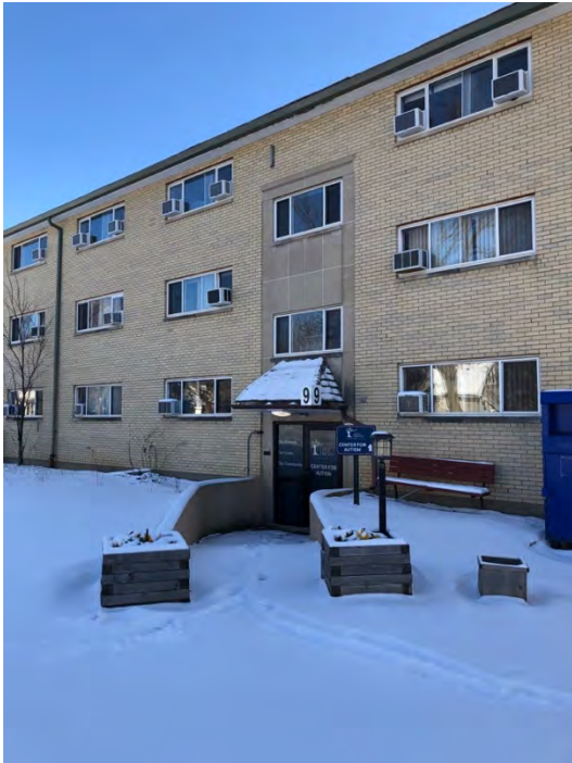
Figure 11: North entrance detail, looking southeast
