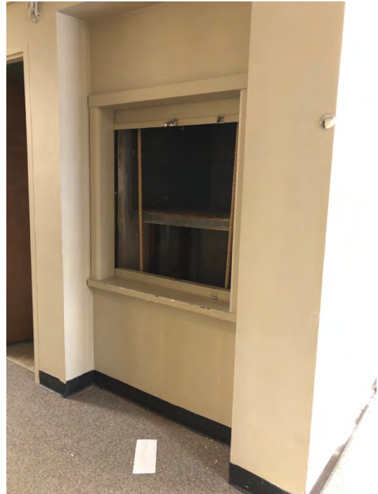
Figure 12: Dumbwaiter in corridor
