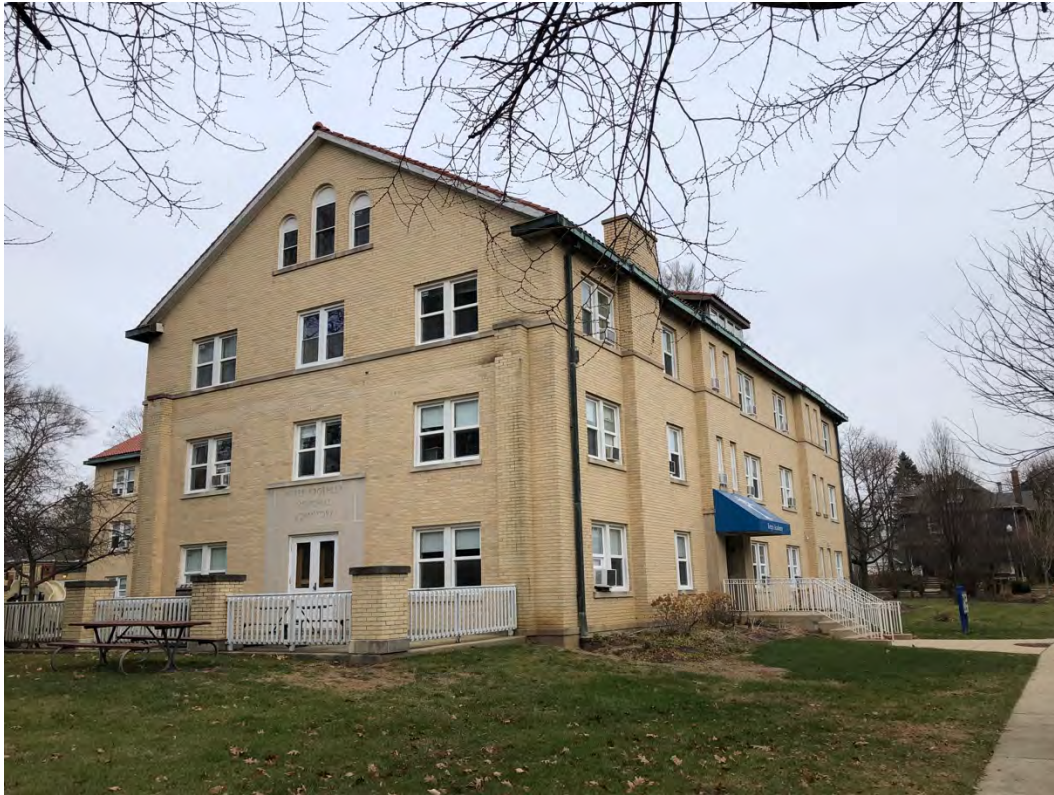
Figure 8: West and south walls, looking northeast Source: author
