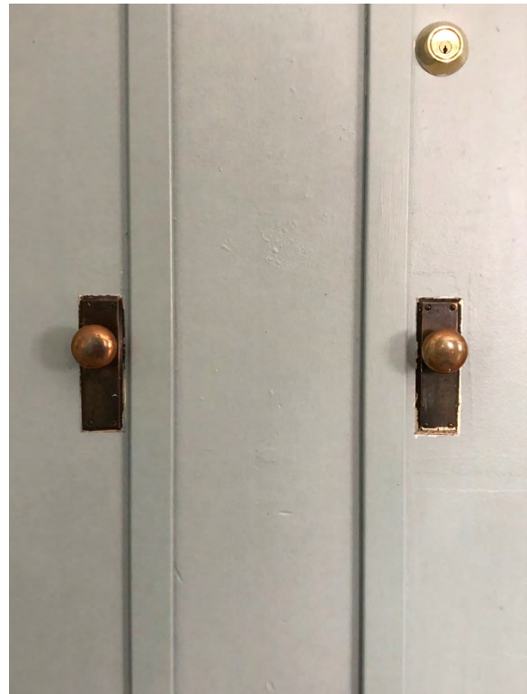
Figure 14: Original closet door hardware
