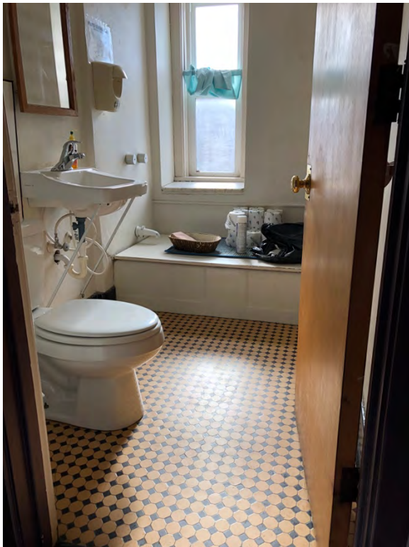
Figure 13: Original bathroom tile floor
