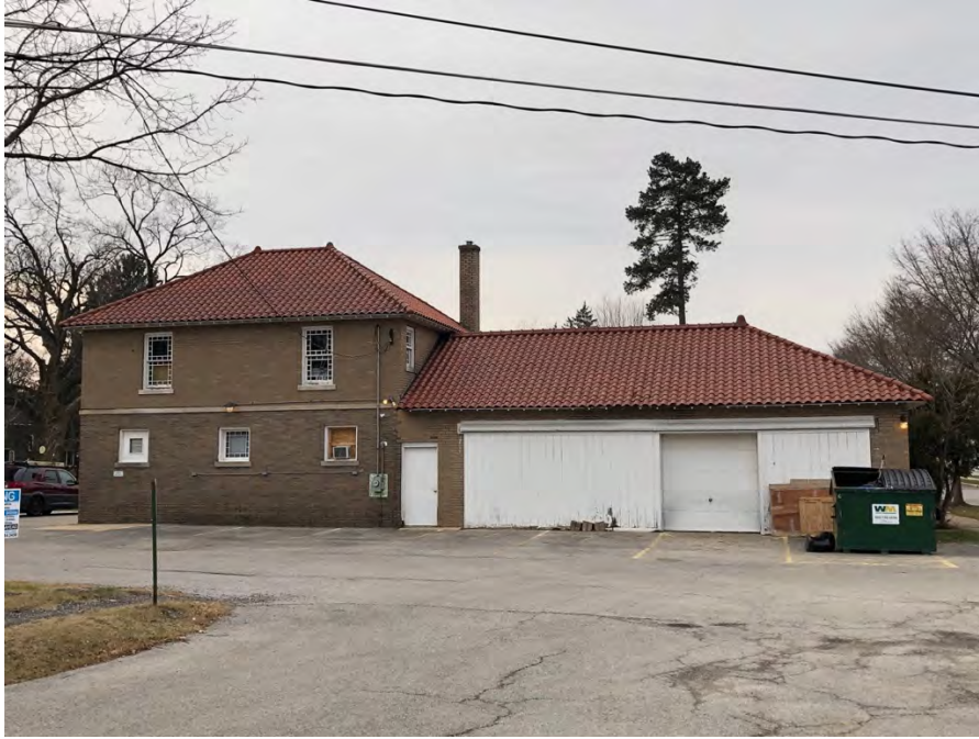
Figure 4: East wall, showing four-car extension to the right, looking west
