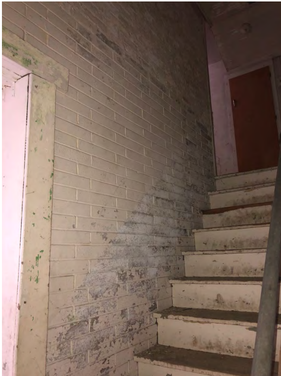
Figure 10: Stairs looking southwest with original exterior wall
