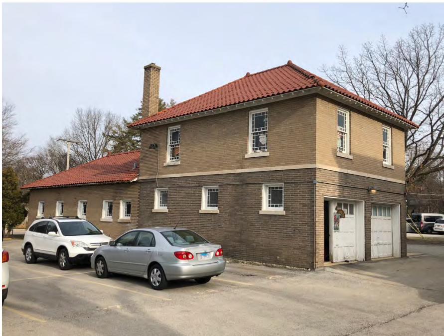
Figure 5: West wall, showing original building in darker brick, looking northeast
