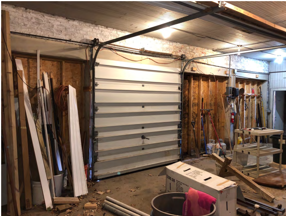
Figure 7: Interior of four-car section, looking southeast
