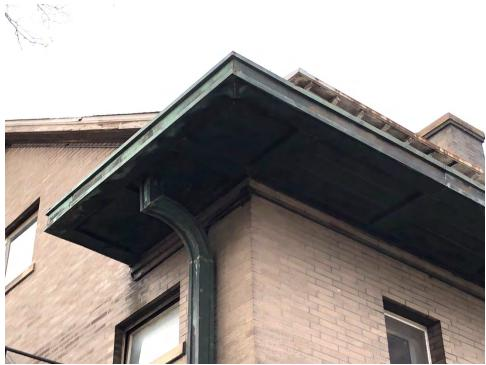
Figure 8: Detail of exterior cantilevered gutter system
