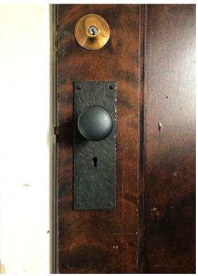
Figure 28: Detail of hammered metal door hardware
