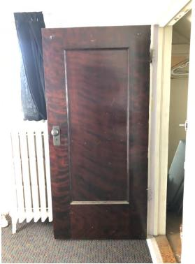
Figure 27: Single-panel closet door with original finish
