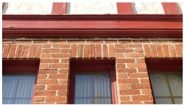
Figure 9: Detail of brickwork and the stucco and wood half-timbering on parsonage wall.
