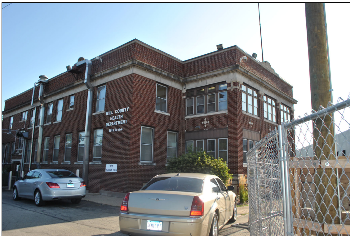
1. Administration block, view northeast
