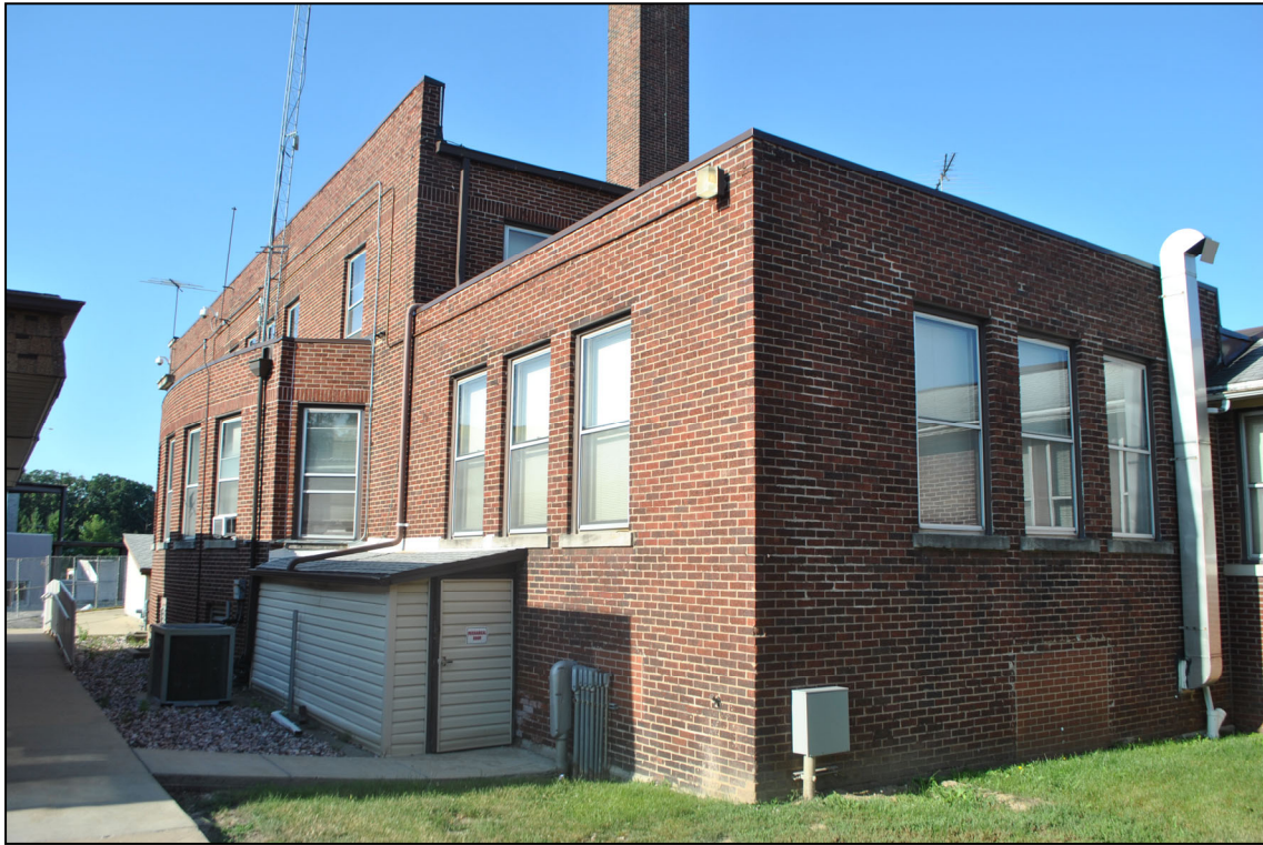
5. Administration block, east and north elevations, view southwest
