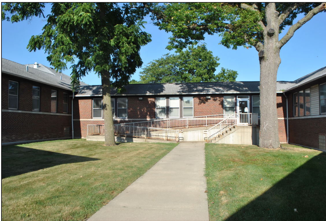
7. Infirmary, courtyard between the east wings of the first and second division, view west
