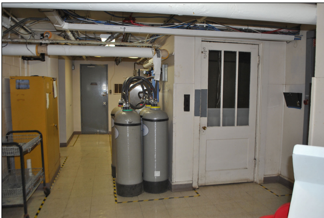
22. Administration block, basement, north-center room, view north
