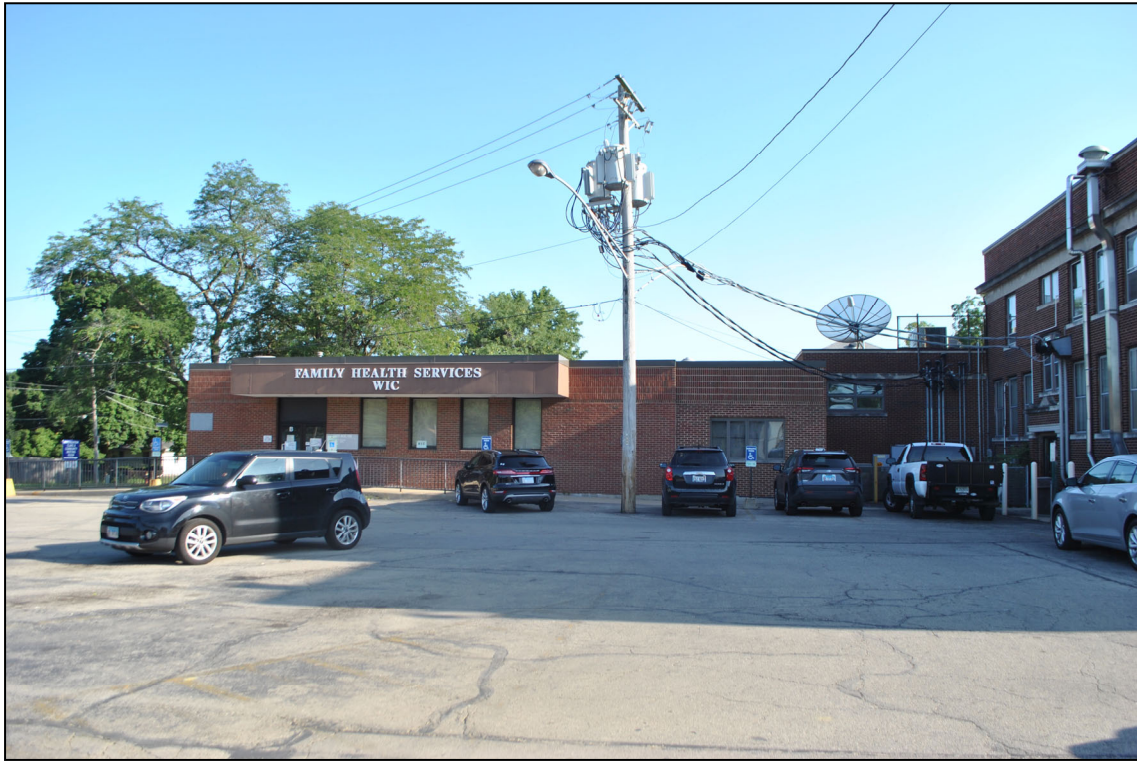
3. 1990 southwest addition, view north
