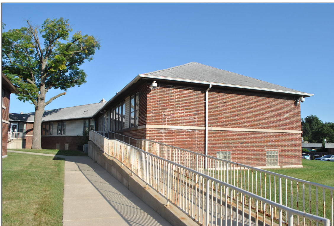
10. Infirmary, third division, east wing, southeast and southwest elevations, view northwest
