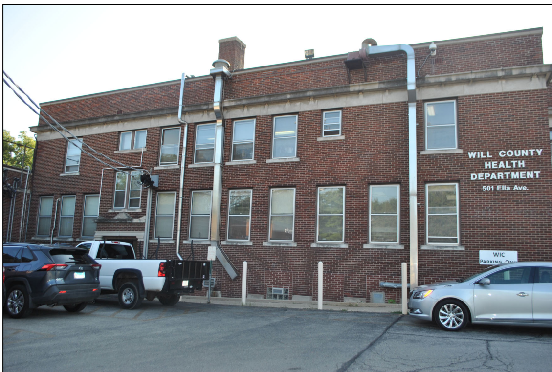
2. Administration block, west elevation, view east
