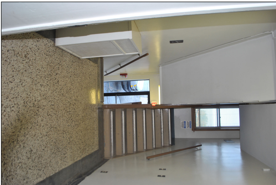
16. Administration block, first floor, west stairwell, view west
