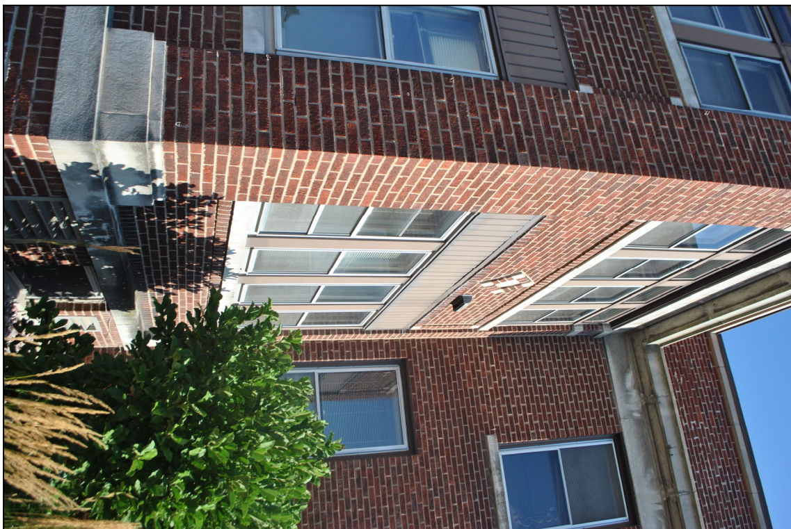
4. Administration block, southeast corner, view northwest
