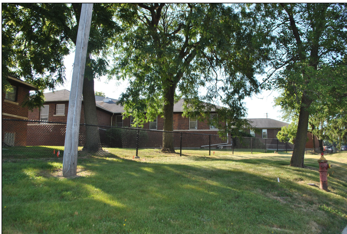
12. Infirmary, west wings, view south
