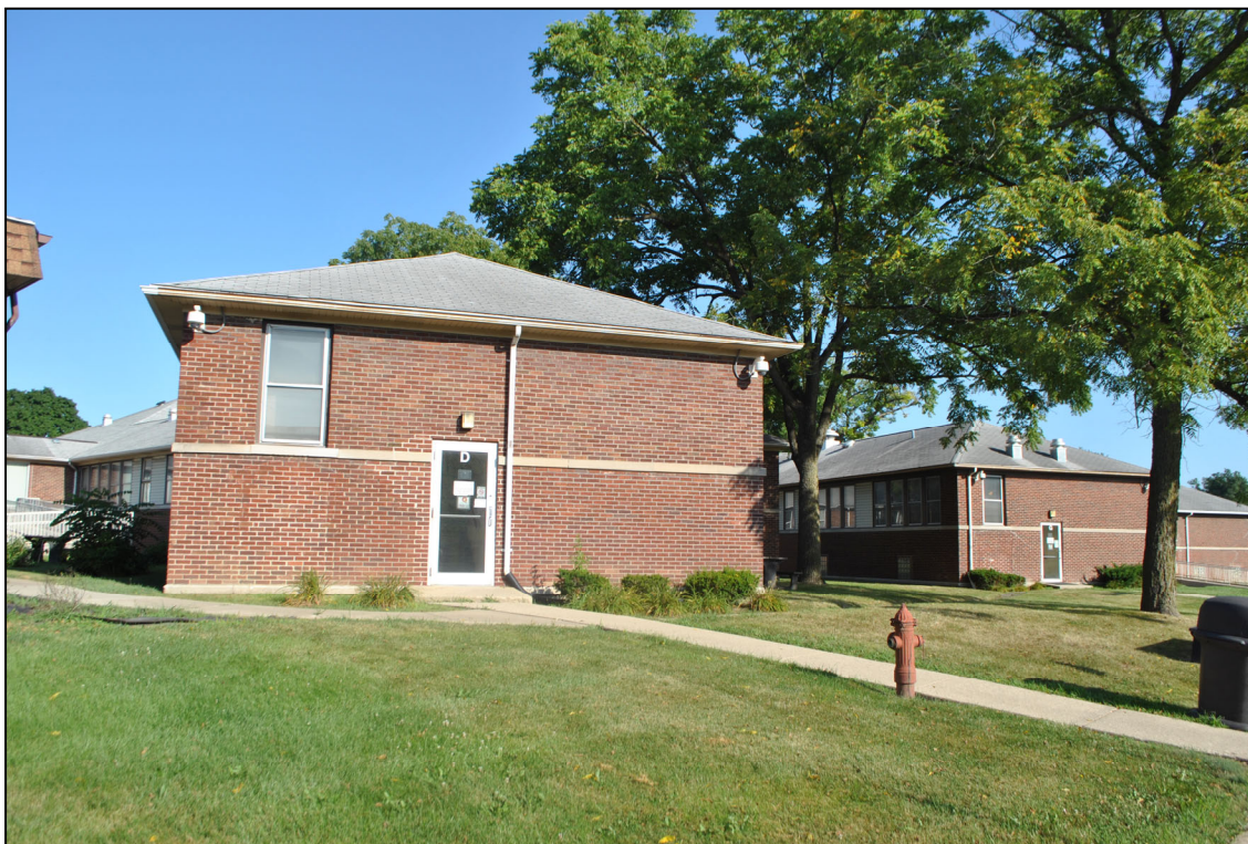
8. Infirmary, first and second division, east wings, view west
