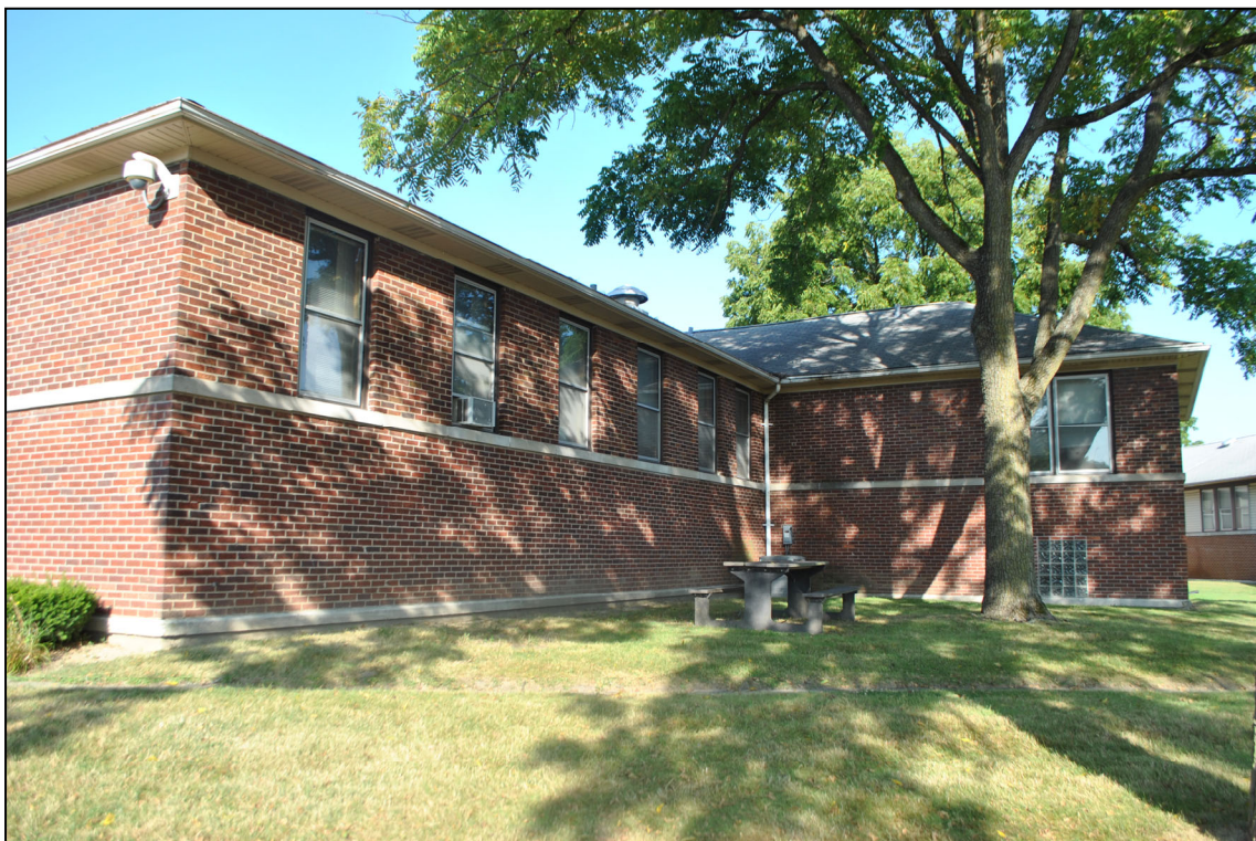
6. Infirmary, first division, east wing, view west
