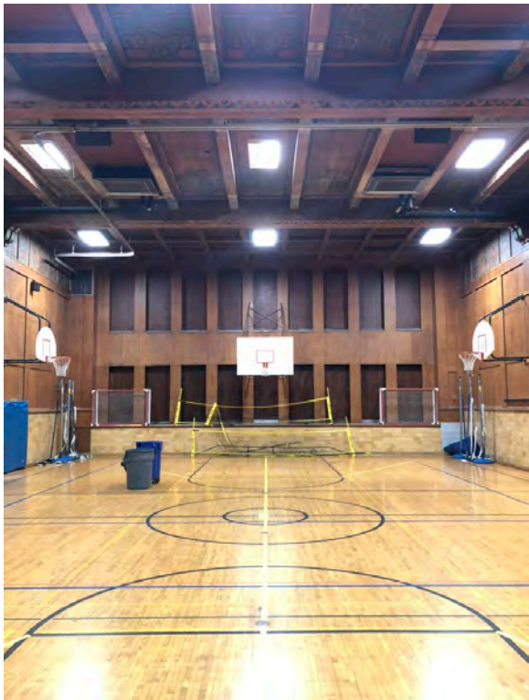
North wall of gym, showing filled windows
