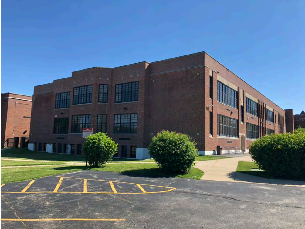
View to south of 1952 addition
