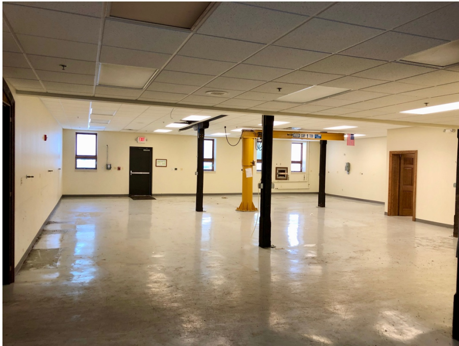
Room C in Section 61a (to be demolished), looking east
