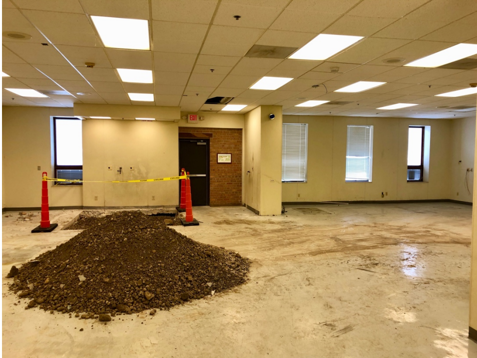
Secondary Operations in Section 61 (to be demolished), looking east
