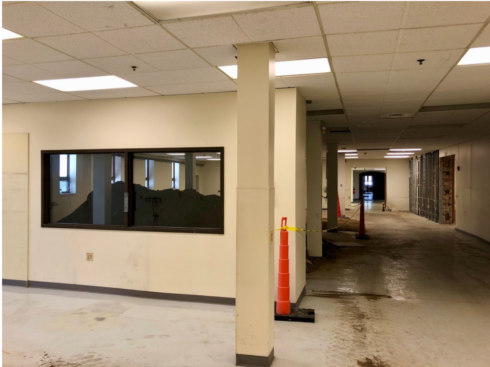
Secondary Operations in Section 61 (to be demolished), looking north
