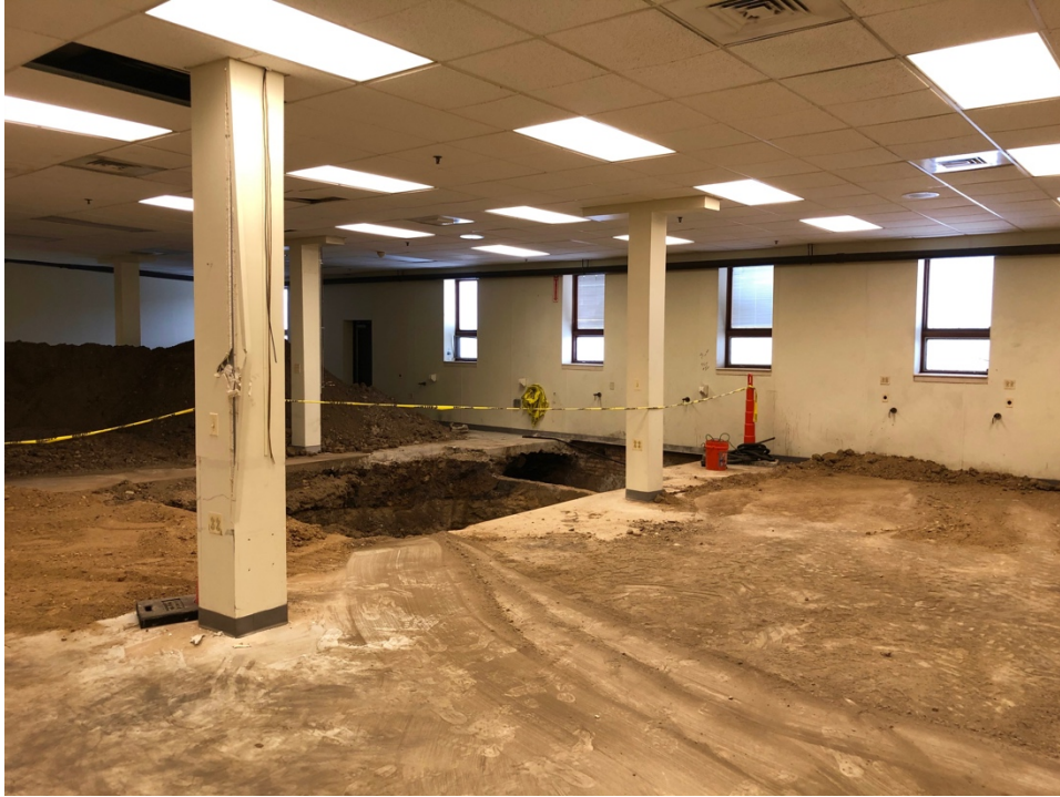
Tool & Die in Section 61a (to be demolished), looking northeast
