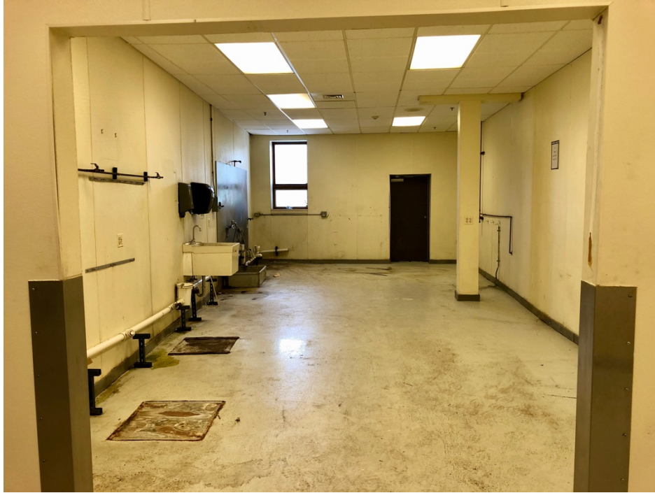
Room A in Section 61a (to be demolished), looking west
