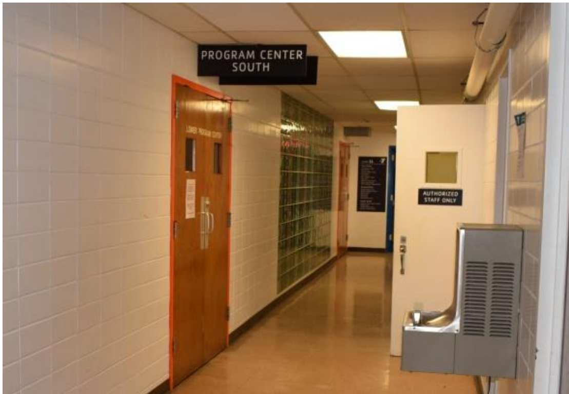
Figure 76. Use of decorative glass blocks in the Youth Center. (Top) Interior view of room illustrating use of clear and colored glass block. (Bottom) Detail of hall illustrating use of glass block and painted concrete block walls, and acoustical tile ceilings (2020).
