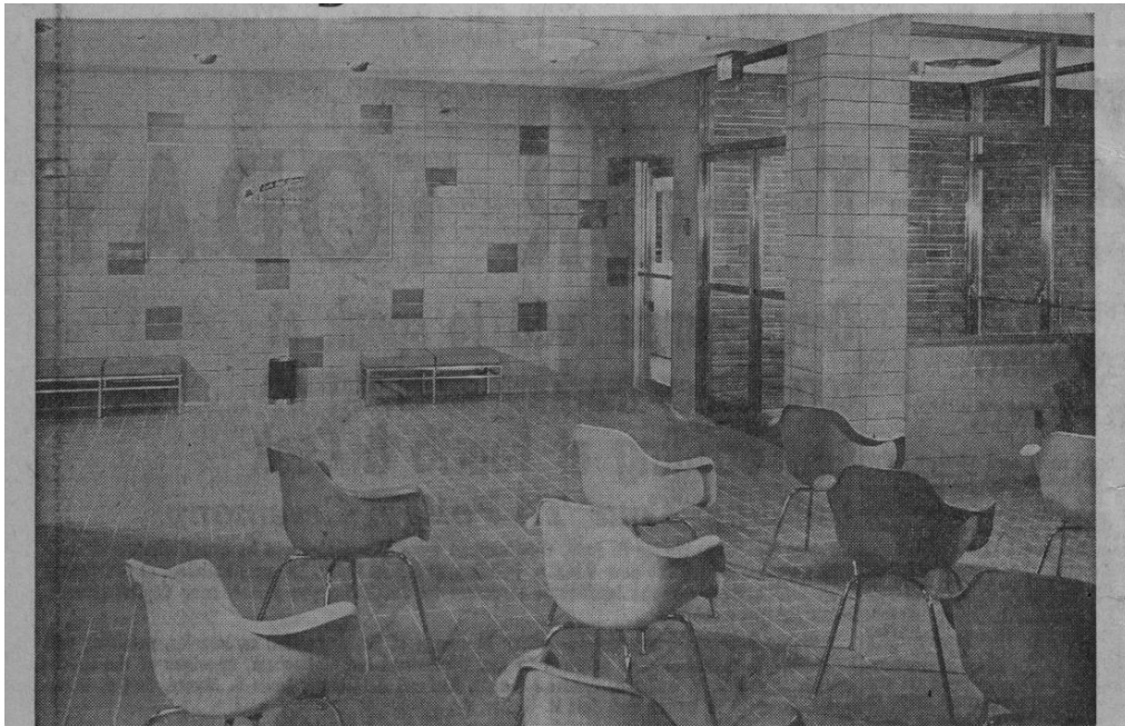
Boys will be boys, but in spite of heavy traffic, this wall, being scuff resistant and virtually dust free, will require only infrequent cleaning. Arketex ceramic glazed structural facing tile is shown above in the main lobby youth entrance.
