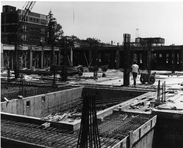
Figure 40. Concrete and steel work framing superstructure (late 1959) (YMCA Black and White Prints 1959).
