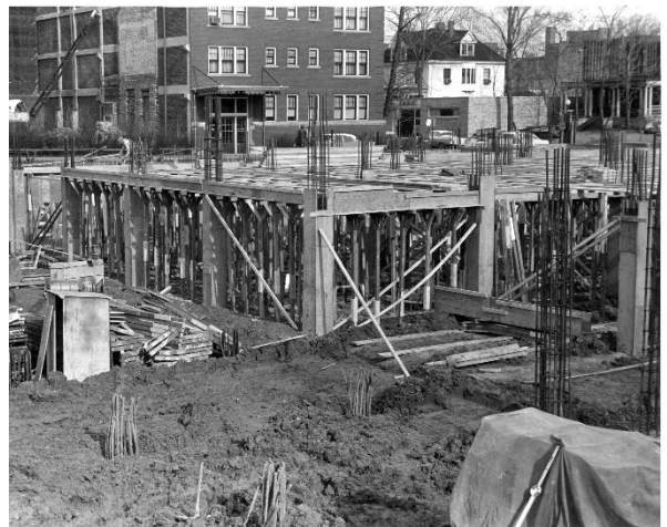
Figure 39. Excavations, foundation work, and forming columns and first floor deck (fall 1958/early 1959) (YMCA Black and White Prints 1958-59).
