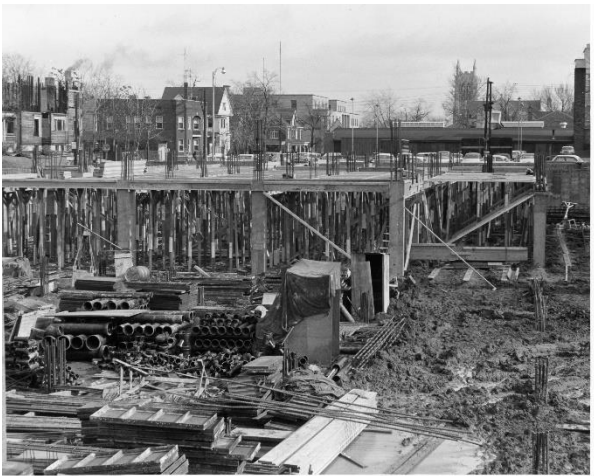
Figure 39. Excavations, foundation work, and forming columns and first floor deck (fall 1958/early 1959) (YMCA Black and White Prints 1958-59).
