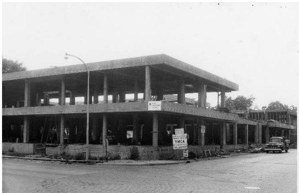
Figure 40. Concrete and steel work framing superstructure (late 1959) (YMCA Black and White Prints 1959).
