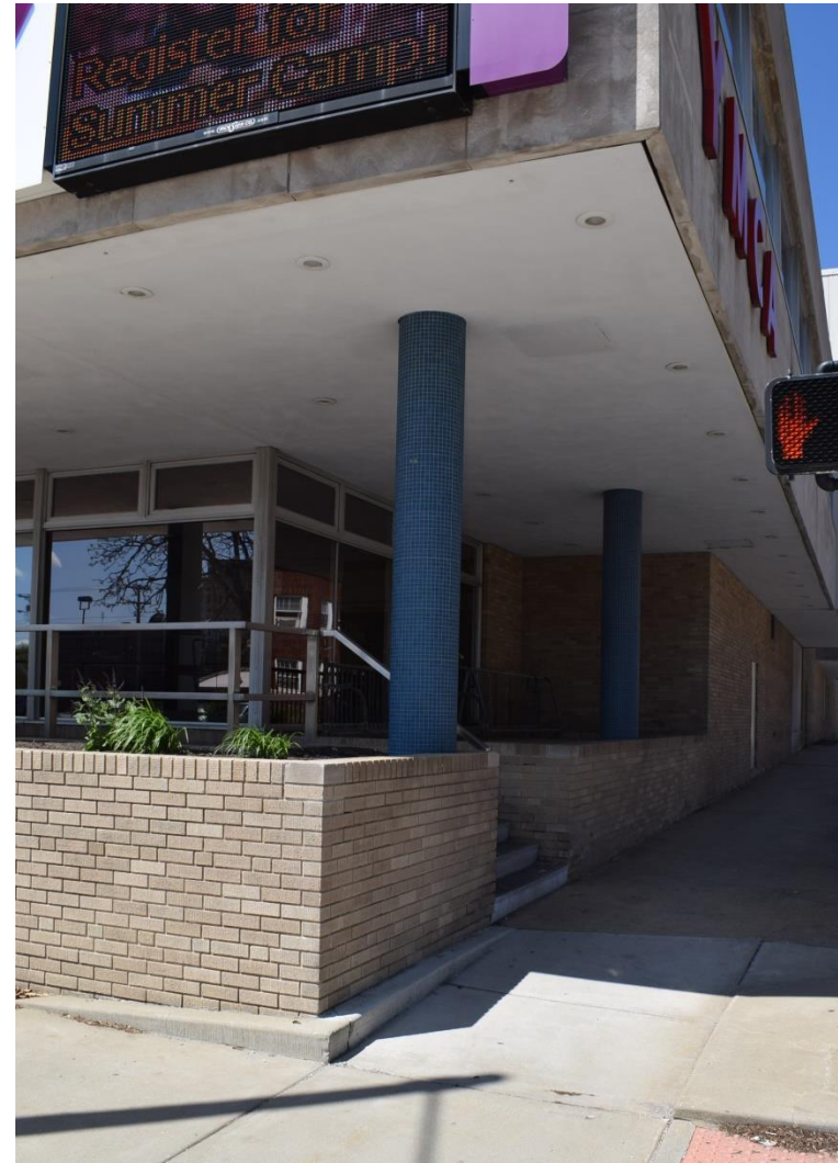
Figure 72. Two views of the Adult Entrance's recessed terrace with brick planters and round columns (with blue-glazed tile). (Left) Looking south along Fourth Street elevation. (Right) Looking west along Cook Street elevation (2020).
