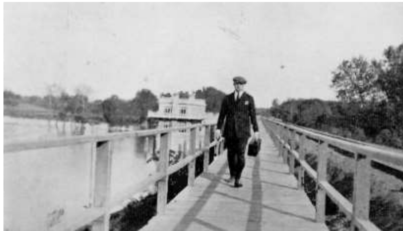
Figure 28. (Top) Boardwalk under construction (Staley Museum). (Middle and Bottom) Photographs taken in 1921 looking down the boardwalk leading to the Staley Club House, which appears in the distance ( Staley Journal [June 1921], pp. 1, 8). Note the slight difference in construction, with the use of diagonal corner blocks in the top photograph.
