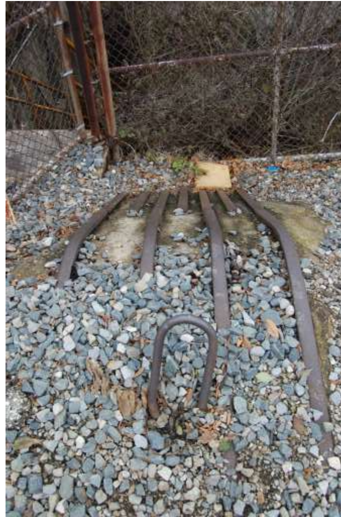
Figure 76. (Left) Close-up detail of the exterior finished concrete surface on the building, emulating ashlar masonry. (Right) Rail incline located along east side of causeway bridge, for raising and lowering heavy machinery into the pump floor level.
