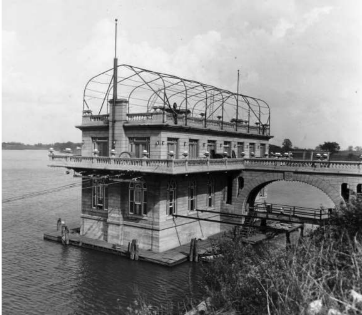
Figure 33. Ca. 1928 image of the Staley Pumping Station and Club House, looking northeast (Staley Museum). Note the presence of the canopy, with chimney flue extension only on the west chimney. This would suggest that the east fireplace was not used as much as the west one. The frame canopy is present over the two side-by-side privies present along the north side of the building, adjacent to the steps at the northeast corner of the structure.
