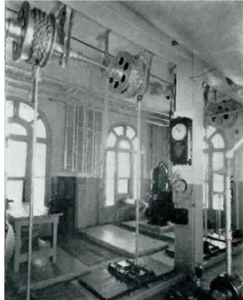
Figure 62. (Left) “These four pumps, C and D units, are in almost continuous service.” (Right) “The hoisting mechanism shown here raises and lowers the screens between the intake and suction chambers in the level below this shown” ( Staley Journal [September 1938], p 5).
