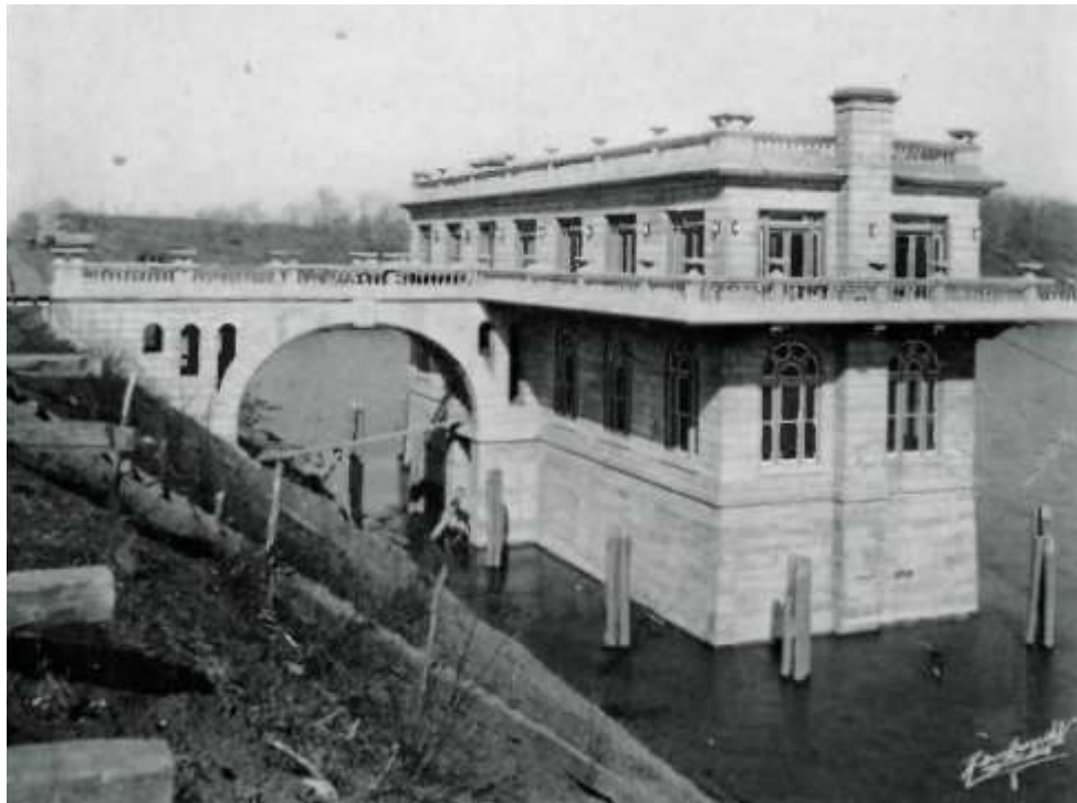
Figure 23. (Top) Photograph of the Staley Pumping Station and Club House, illustrating the filling of the impoundment. Original picture, as published in article discussing the Staley Company's annual picnic, with pictures of Nelson Park and captioned "Down this walk to the Staley Club House for the Dance. Please Shine, Mr. Moon." Staley Journal [September 1921], p. 7; Staley Museum). (Bottom) The Pumping Station and Club House, as seen early in February 1921. The pilings seen around the perimeter of the building were intended to hold in place a floating dock that was not, as yet, installed. The level of the lake was quite low when this photograph was taken, in February 1921 ( Staley Journal [March 1921], p. 8).
