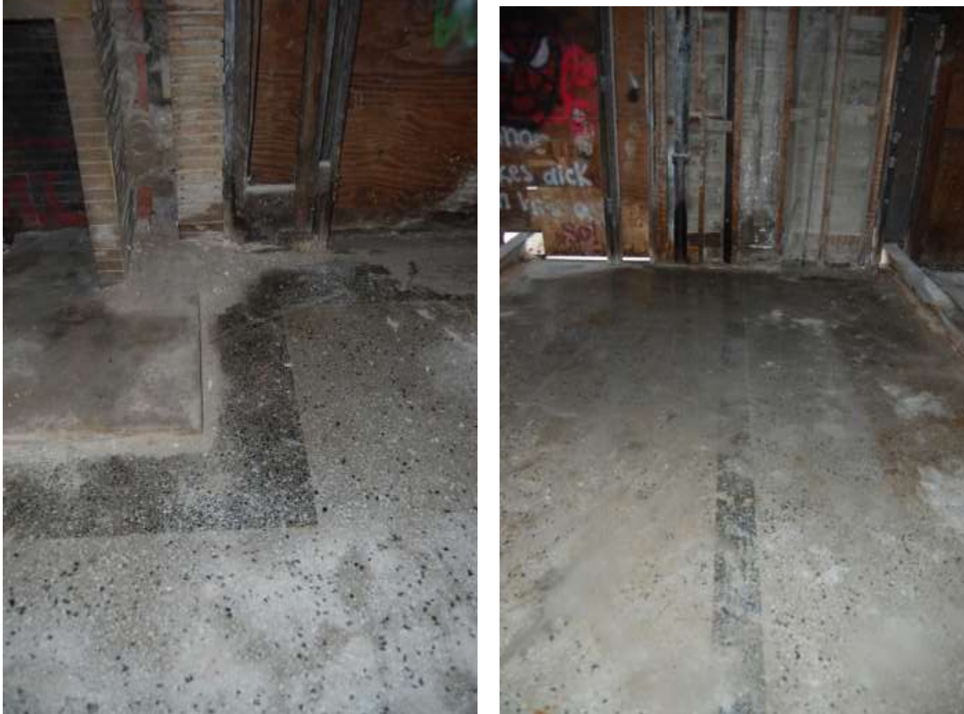
Figure 77. Two views of the darker border used on the terrazzo floor in the Club Room. (Left) Wide border around the perimeter of the room, and the edge of the fireplaces. (Right) Narrow band across the rooms, dividing the large floor into panels (See also Figures 63, 64, and 66 for historic views of floor).
