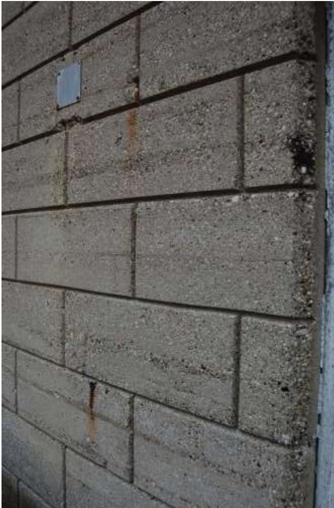
Figure 76. (Left) Close-up detail of the exterior finished concrete surface on the building, emulating ashlar masonry. (Right) Rail incline located along east side of causeway bridge, for raising and lowering heavy machinery into the pump floor level.
