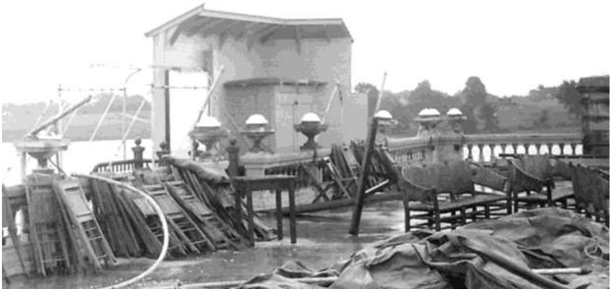
Figure 32. (Top) View showing the pre-canopy, frame structure located at northeast corner of the Roof Level. Note what appears to be a boxed vent along the west side of this structure (Staley Museum). (Bottom) Post-canopy frame structure located immediately east of the stair landing, after storm damage (Staley Museum). This small, frame structure had two doors (presumably accessing separate men's and women's toilets), and was accessed from the adjacent stair landing. By this time, a frame screen had been constructed on the lake-side of the enlarged landing, partially covering the smaller structure and protecting it from the lake-side winds. This structure probably represents side-by-side toilets (or "privies") with a protective frame canopy.
