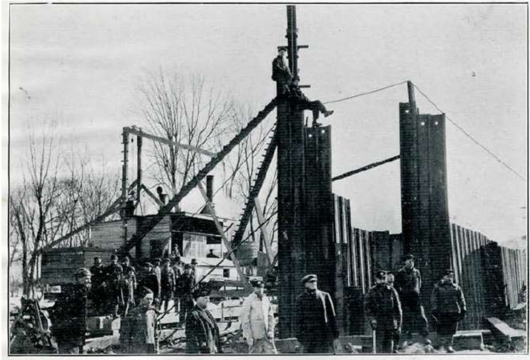
Figure 18. (Top) “A winter scene along the banks of the Sangamon” ( Staley Fellowship Journal [February 1920], p. 5). (Bottom) “Driving the last sheet of steel bulkhead for the 36-inch intake from the river” ( Staley Fellowship Journal [February 1920], p. 9).
