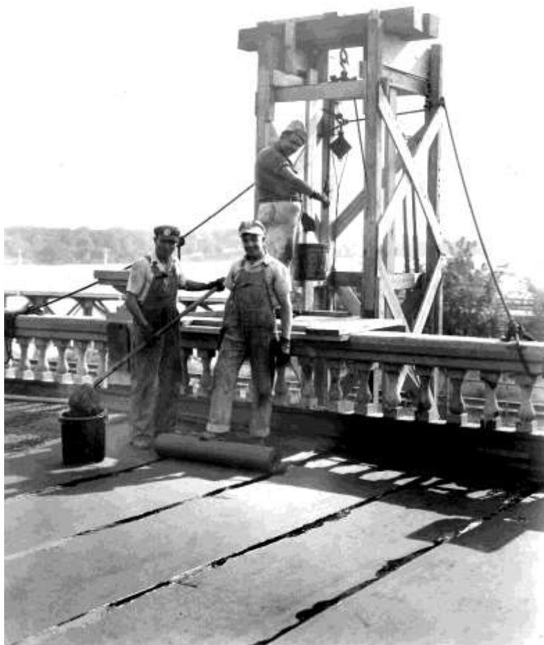
Figure 69. New tar roof being applied to the upper deck of the Staley Pumping Station and Club House, during renovation work of late 1944. By this time, the canopy had disappeared, and the use of the upper floor as a social space had been abandoned (Staley Museum). According to the Staley Journal , the use of the roof top of the Club House had been abandoned sometime ca. 1929 (“Work Starts on Renovation of Club House,” Staley Journal [October 1944], pp 25-26).
