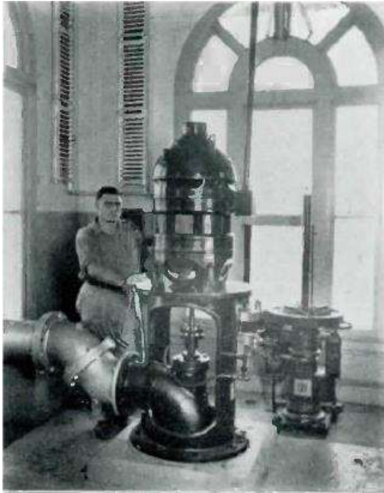
Figure 61. (Left) “Henry Meyer polishing the deep well pump.” (Right) “A and B pumps at the south end of the pump room” ( Staley Journal [September 1938], p 5).
