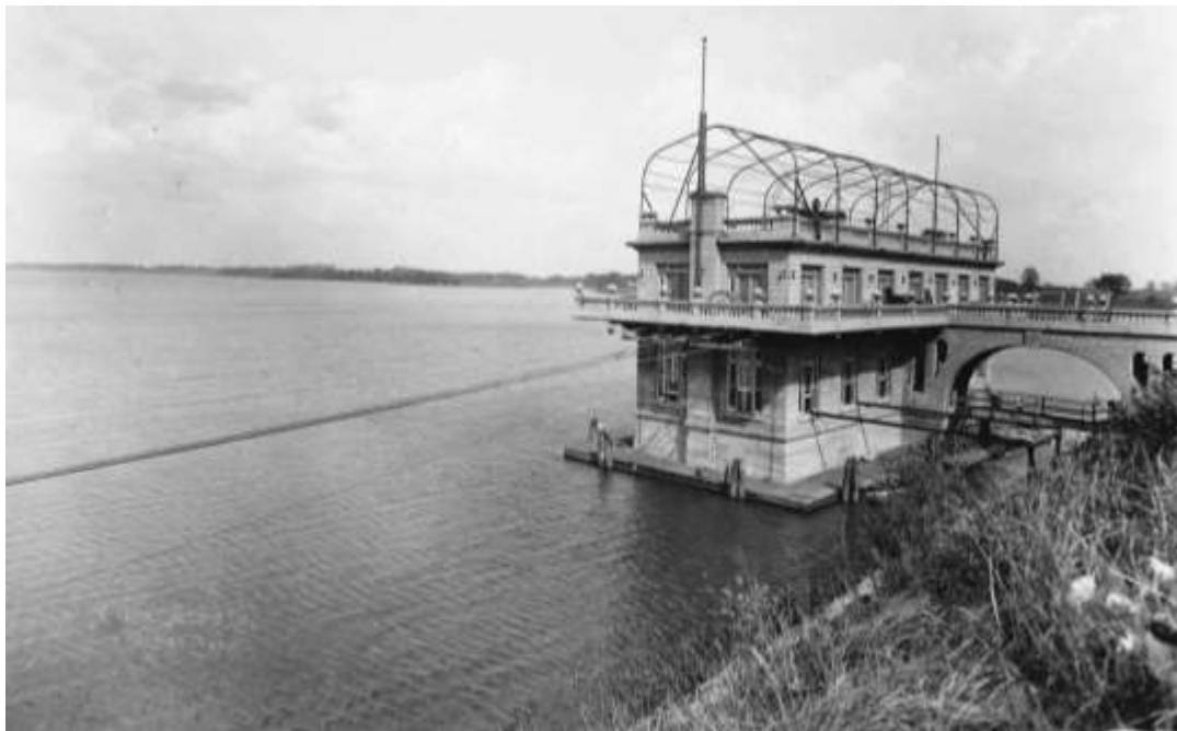
Figure 30. (Top) Picture similar to one published in Staley Journal in 1923 (Coyle 1923:4). (Bottom) Ca. 1928 view looking northwest. This image shows the framework for the roof-top canopy, as well as the frame of the boat shelter on the south (or landward) side of the building. The canopy and boat shelter were installed in late 1923, or perhaps the following year.
