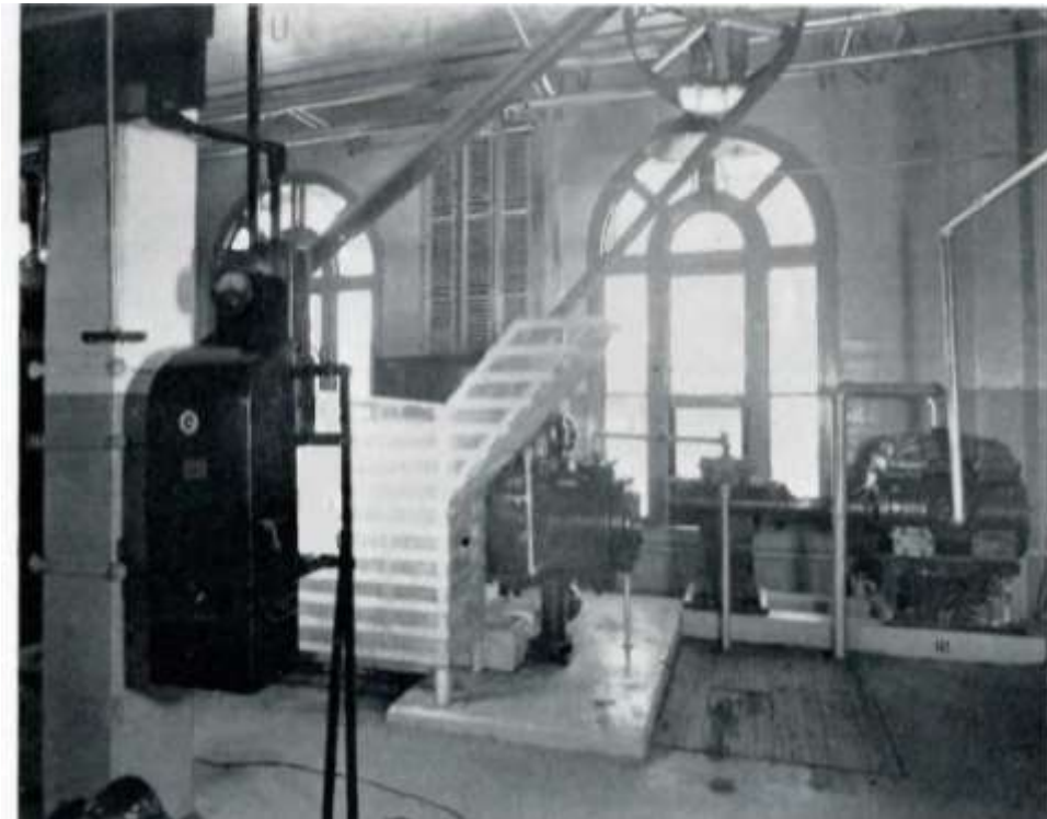
Figure 56. (Top) “Pumps and Intake Gates Above Intake Pits at Pumping Plant,” presumably on the pump room (or “landing”) level (Watson 1923:7). (Bottom) “Part of air compressor and vacuum pumps used to prime centrifugals” ( Staley Journal [September 1938], p. 4).
