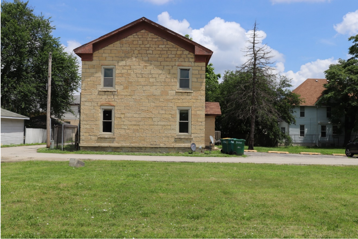
West elevation and site context
