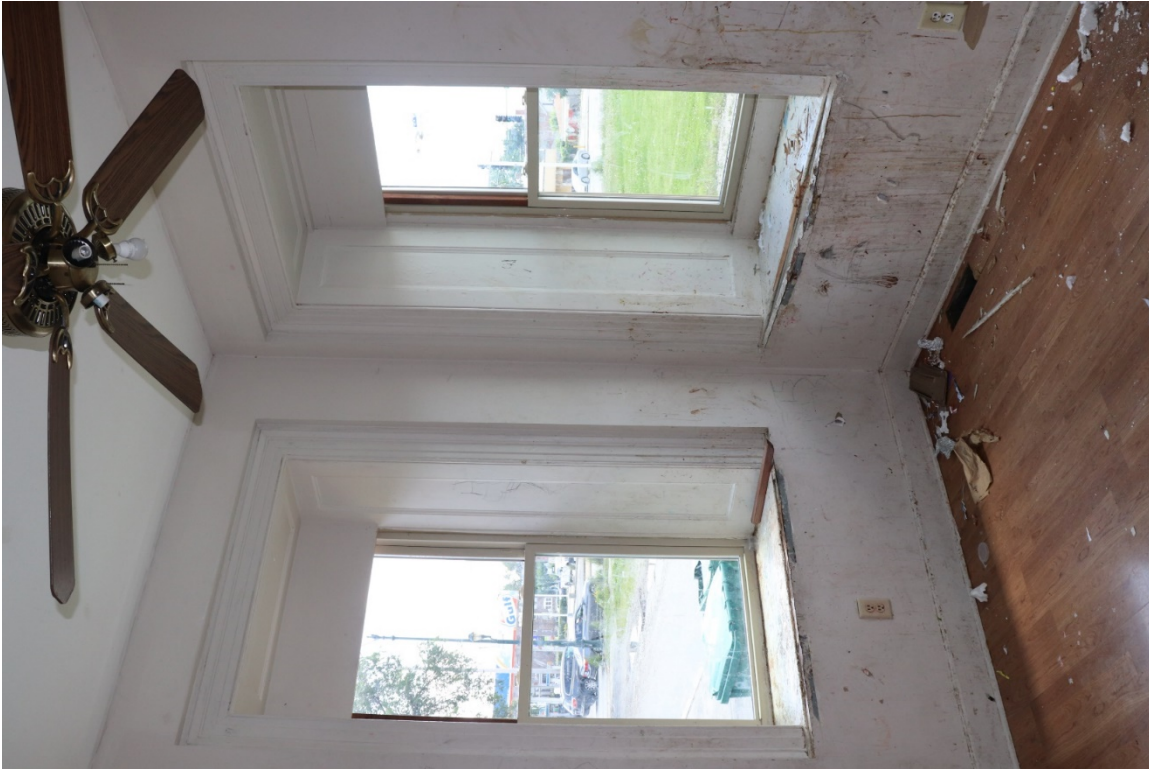
Apartment 1 southwest corner bedroom showing historic window casings
