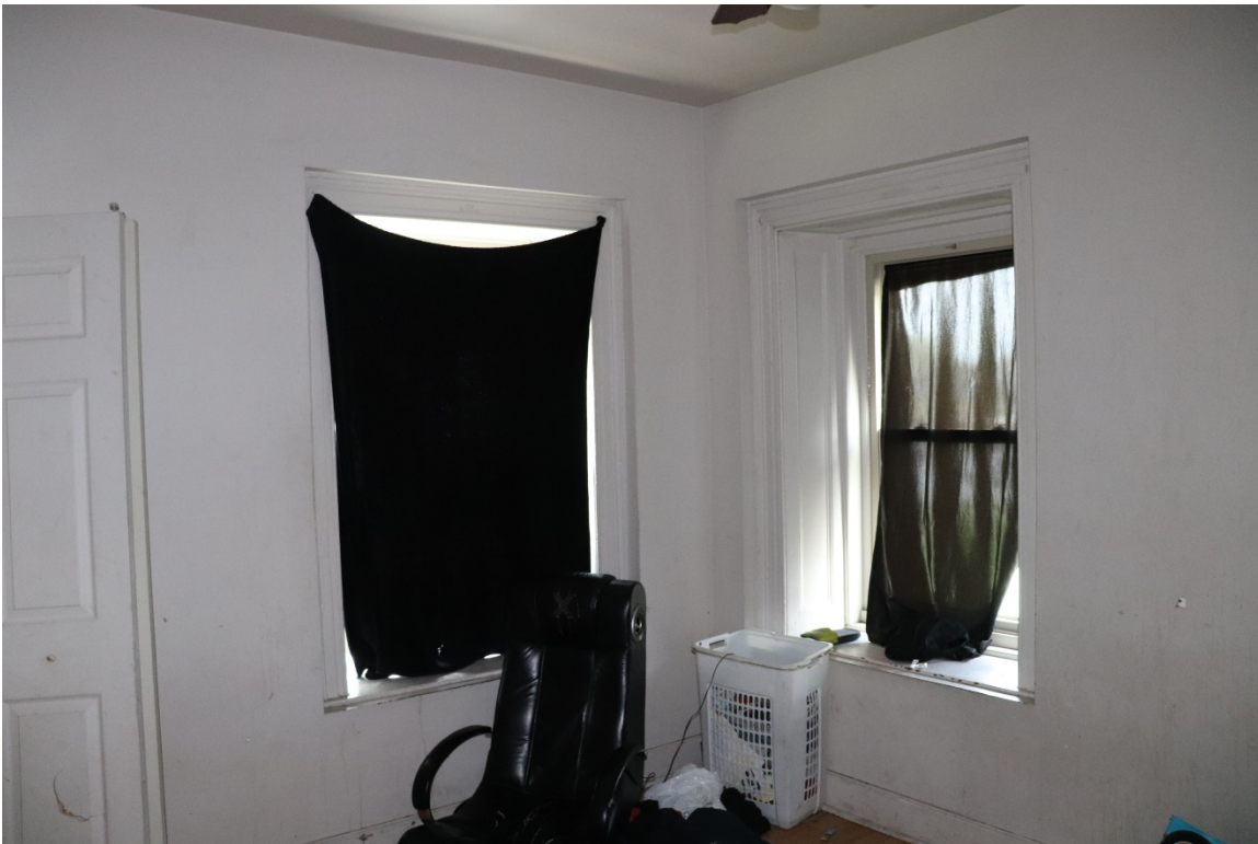
Apartment 2 southwest corner bedroom
