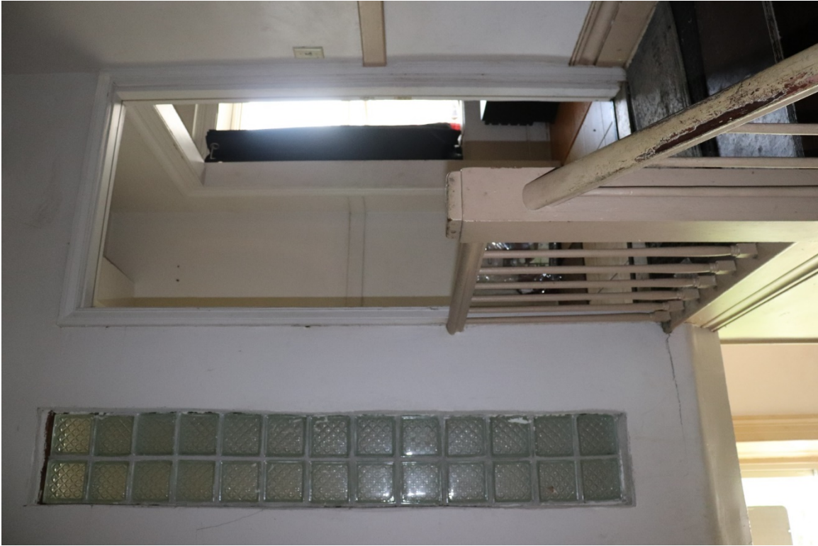
Stair and entry to 2 nd floor apartment
