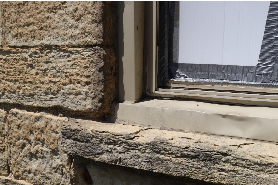
Window sill at south elevation, west end
