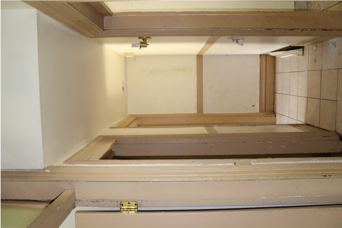
Apartment 1 hallway view west
