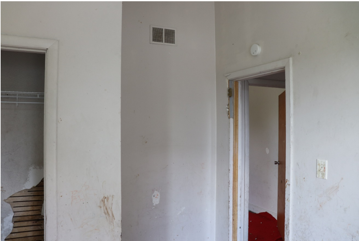
Apartment 1 bedroom at southwest corner
