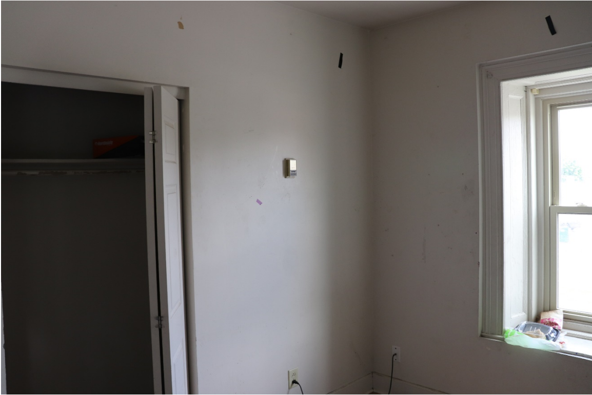
Apartment 2 northwest corner bedroom
