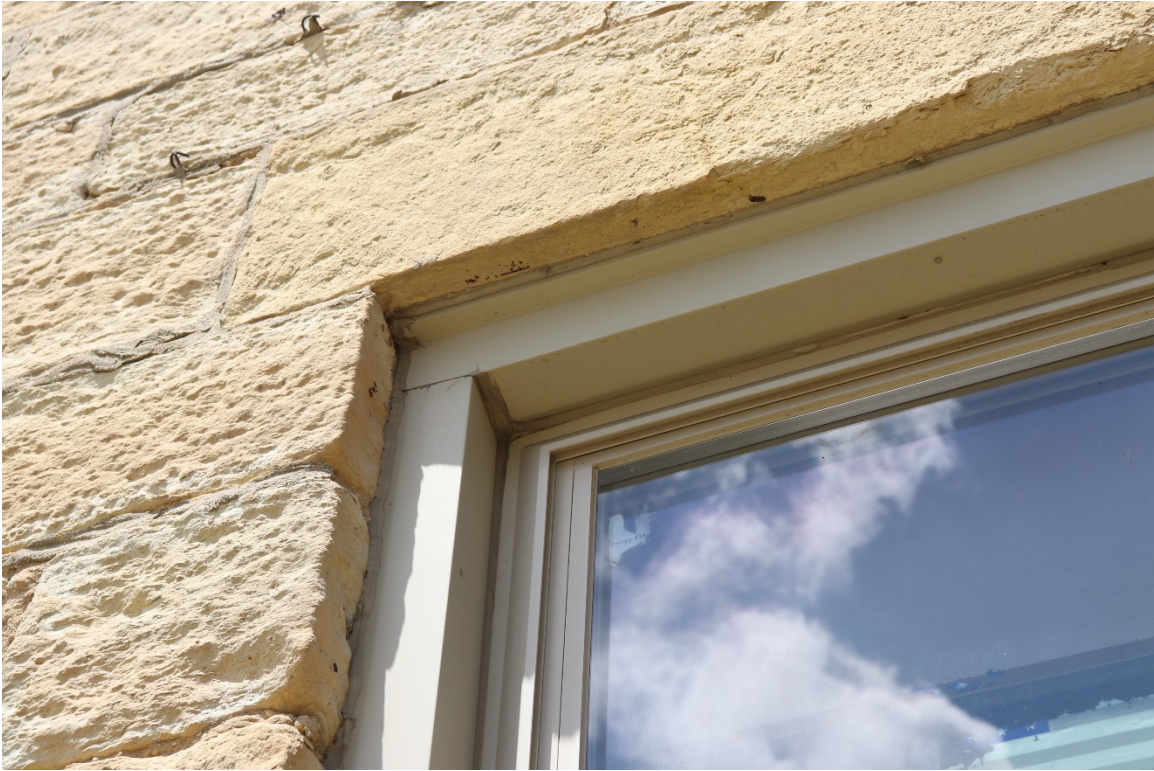
Window head at south elevation, west end
