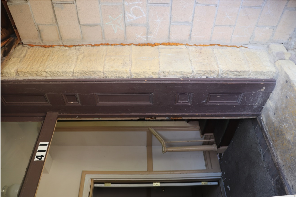
Entry casing and stair hall
