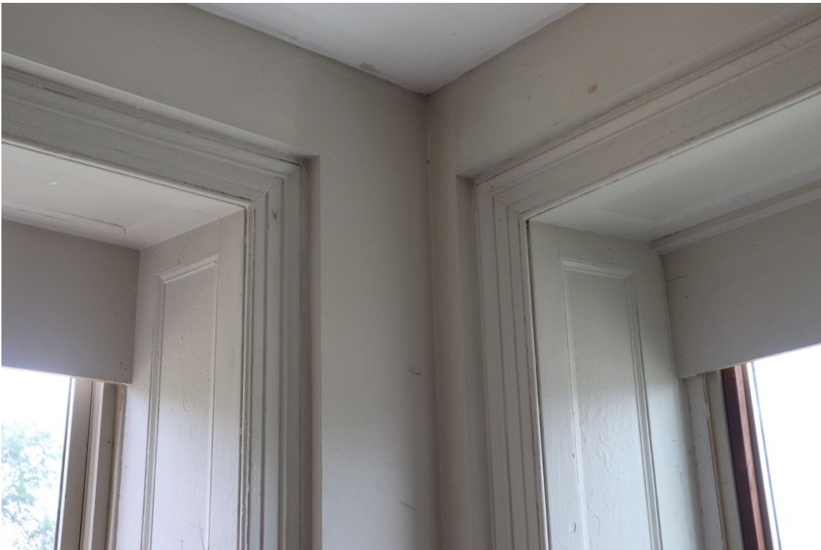
Historic window casings in southwest bedroom of Apartment 1
