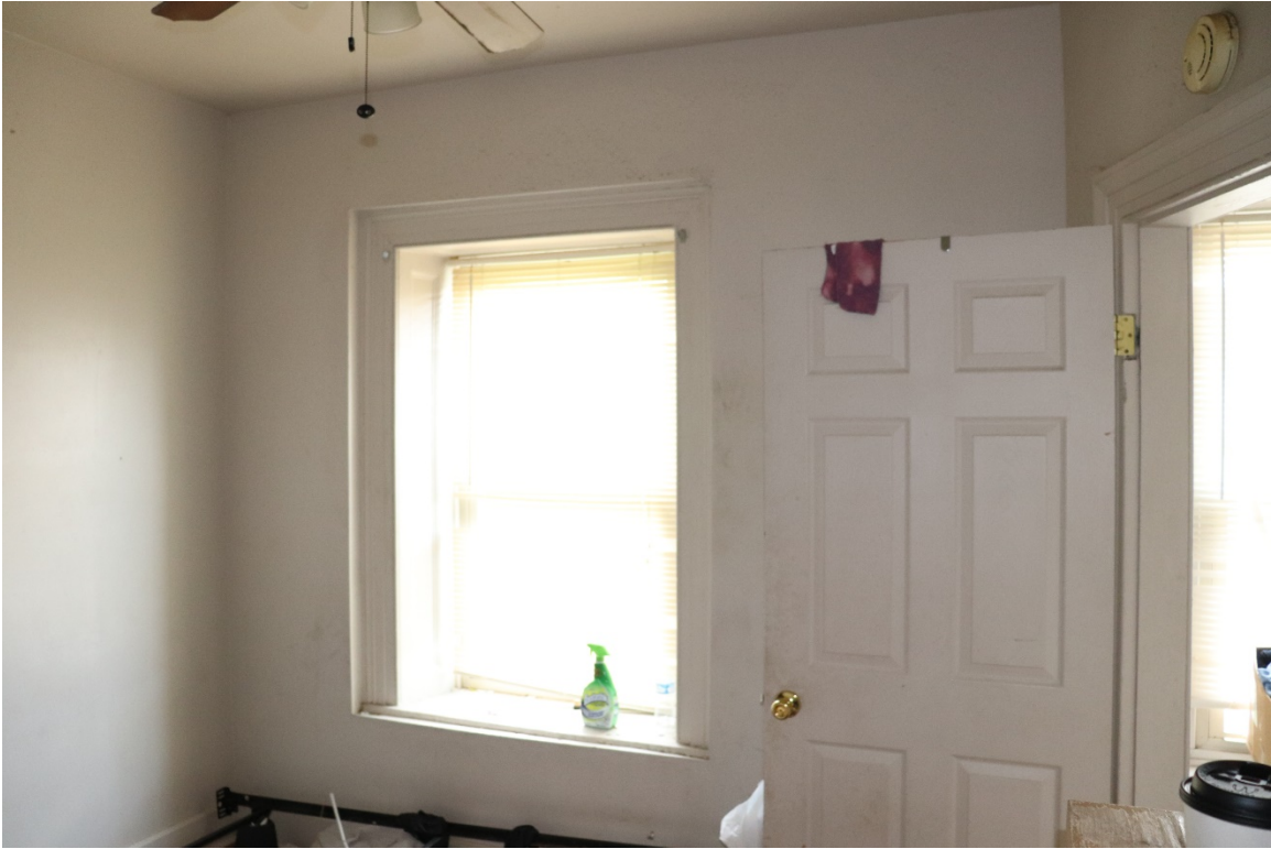
Apartment 2 southeast corner bedroom
