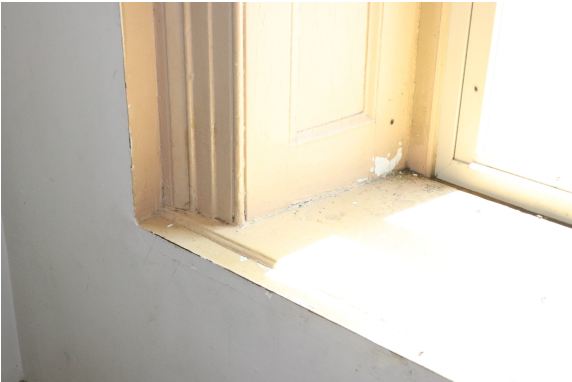
Historic window casings in southeast bedroom of Apartment 1
