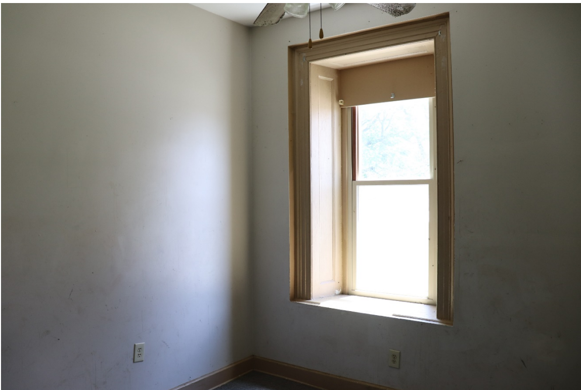
Apartment 1 southeast corner bedroom
