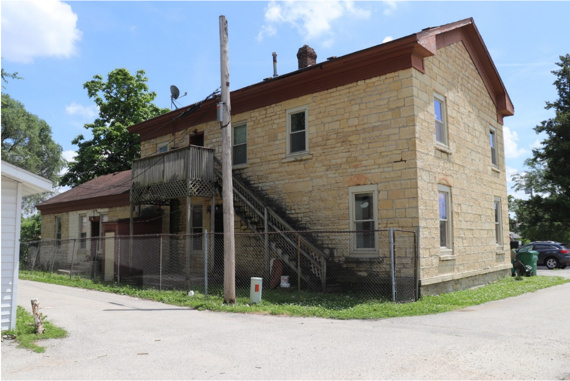
Northwest corner showing north elevation
