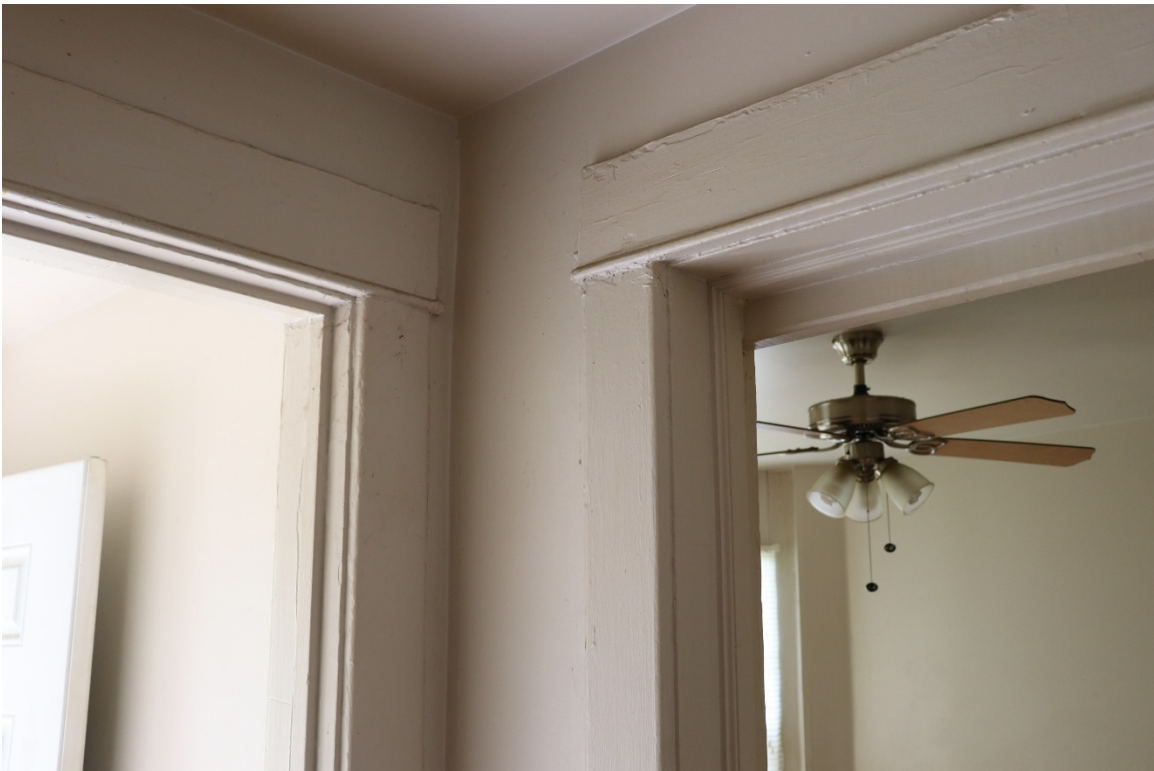
Detail of interior door casings in Apartment 3 hallway
