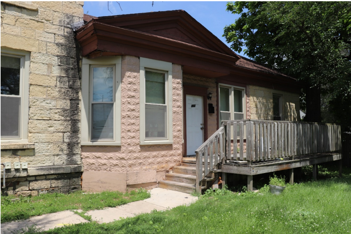
Detail view of south elevation of addition
