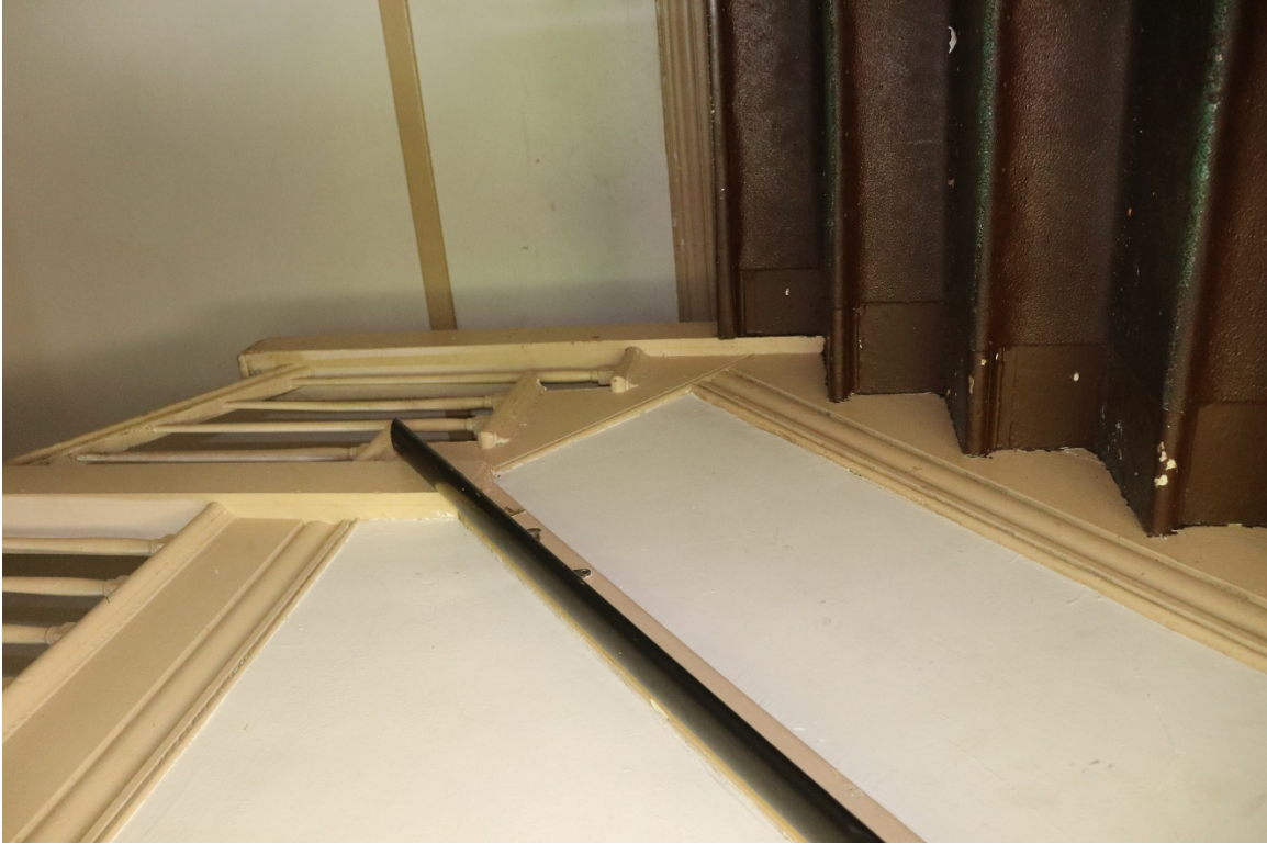
Stair view to landing
