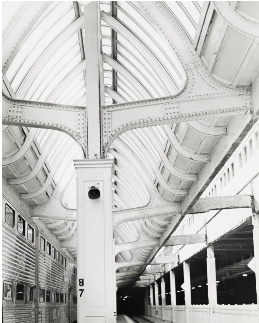
Historic Image 15 Union Station Train Shed Canopies Chicago History Museum IChi-i176253
