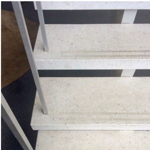
Detail of floating terrazzo staircase
