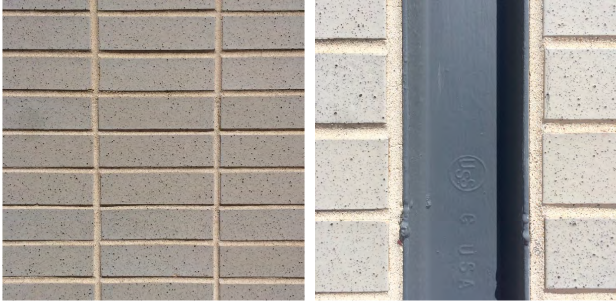
Glazed brick and steel channels in south wall of 1962 building
