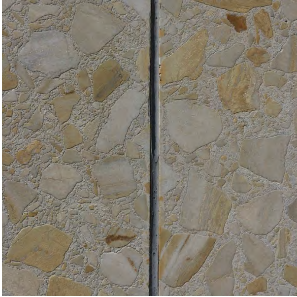
Terrazzo cladding and cornerstone on front of 1971 addition
