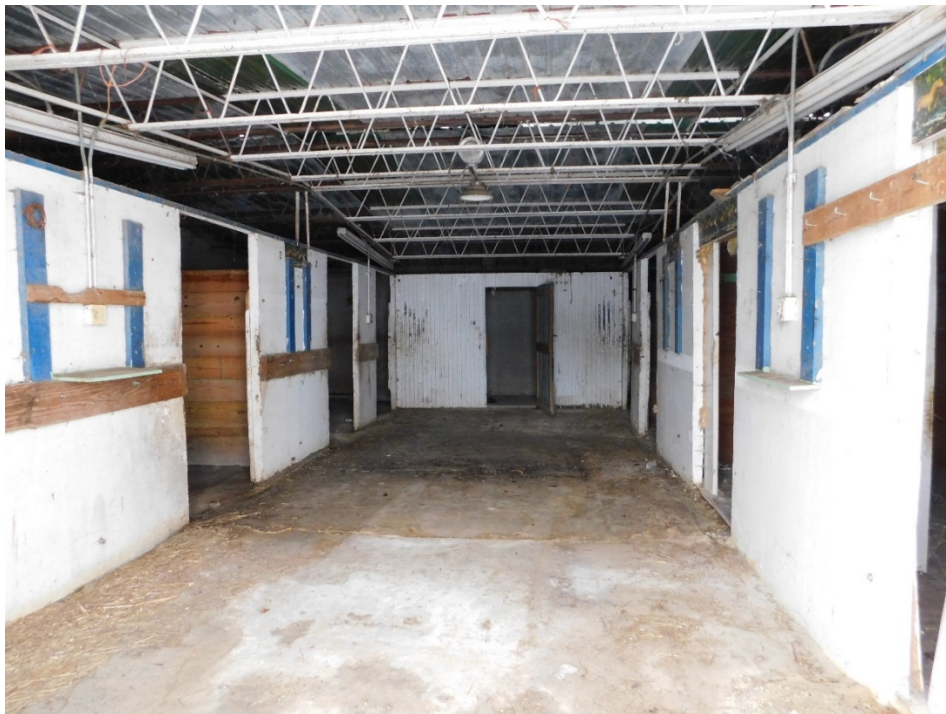
Figure 17: Typical six-stall interior within Stable Building 7b.
