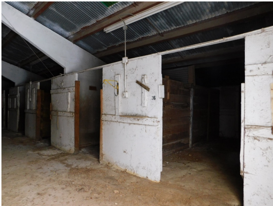
Figure 13: Horse stall within typical tiered Stable Building group.
