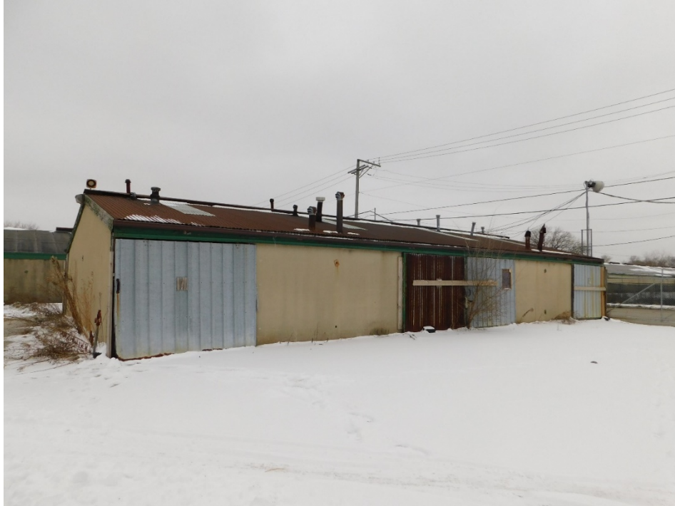
Figure 18: Stable Building 7d on west side of racetrack.
