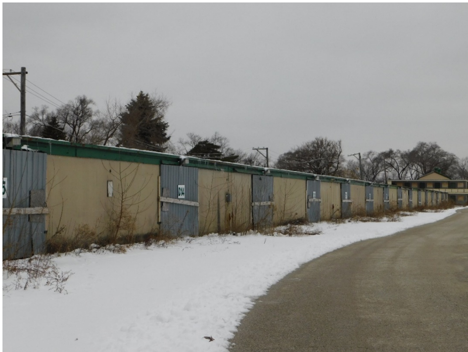
Figure 15: Stable Building Group 7b on south side of racetrack.
