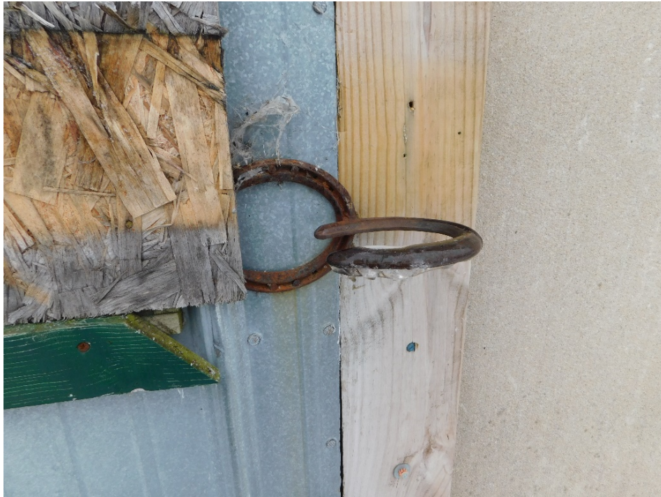
Figure 16: Horseshoe handles on entrances to stalls on Stable Building 7b.
